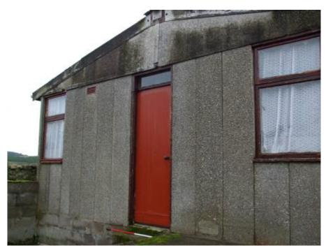
Concrete panels cut horizontally for the insertion of a window; NW wall
