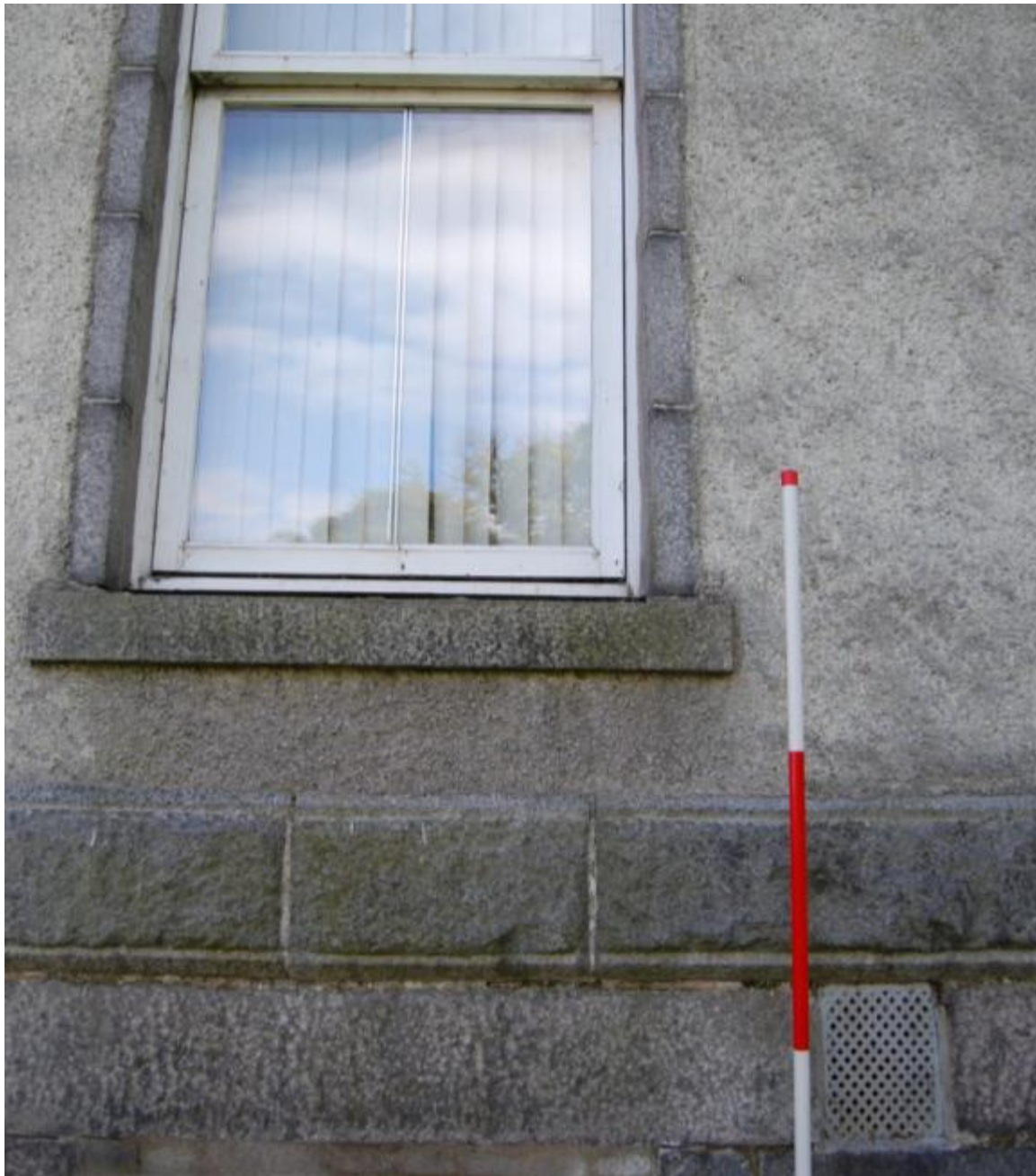
III 7 Detail of original window with plain granite quoin and lintel, rustic granite string course and cast iron vent (bottom right)
