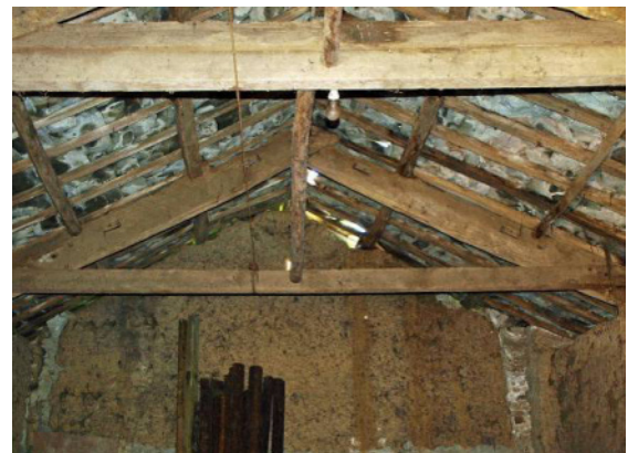
Fig 22 Barn roof E truss (one of 3 similar trusses with reused C16 blades)
