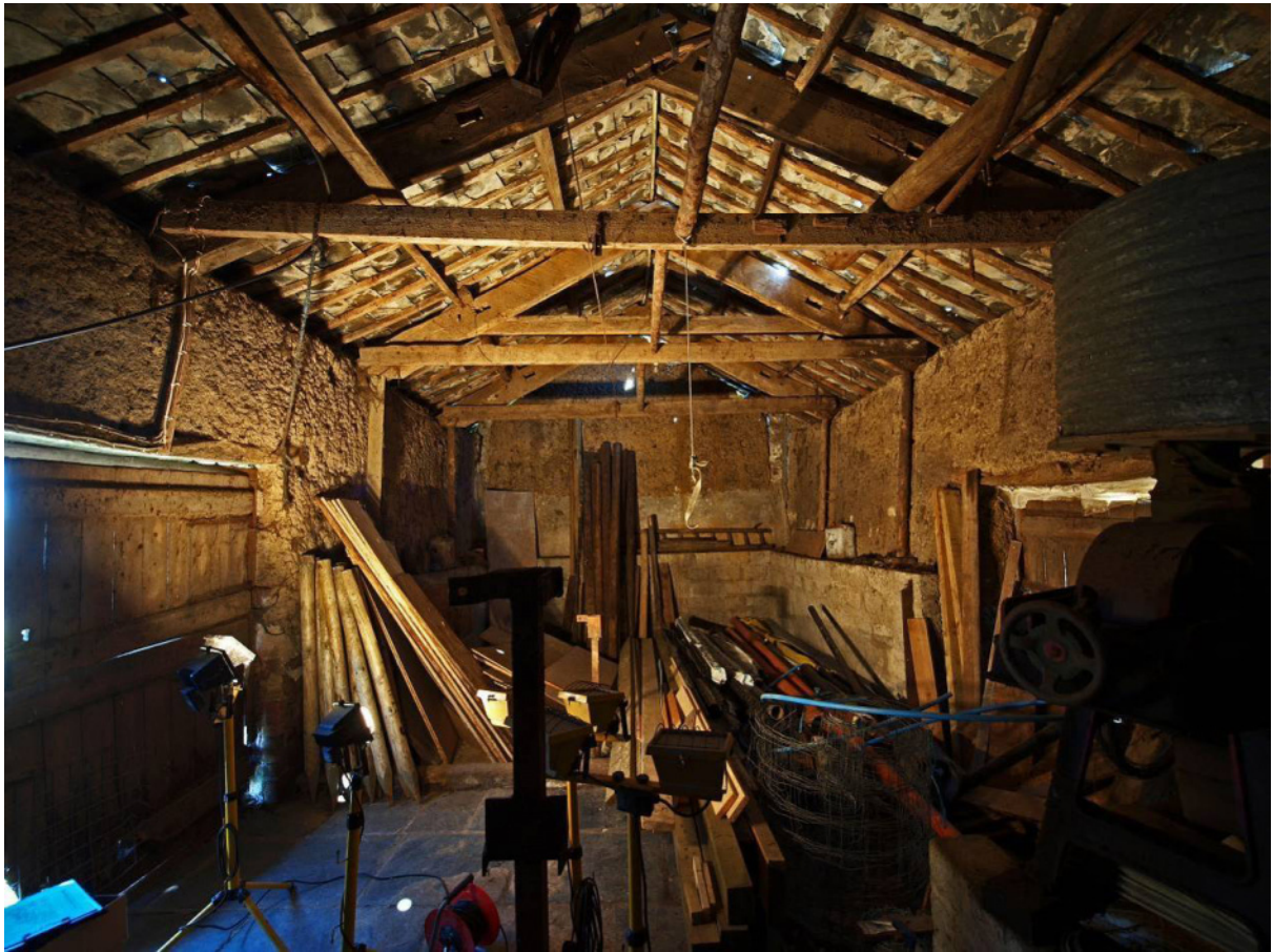
Fig 11 Barn interior from west (note three trusses to east end of barn incorporate truncated blades from a 16 th century roof structure)
