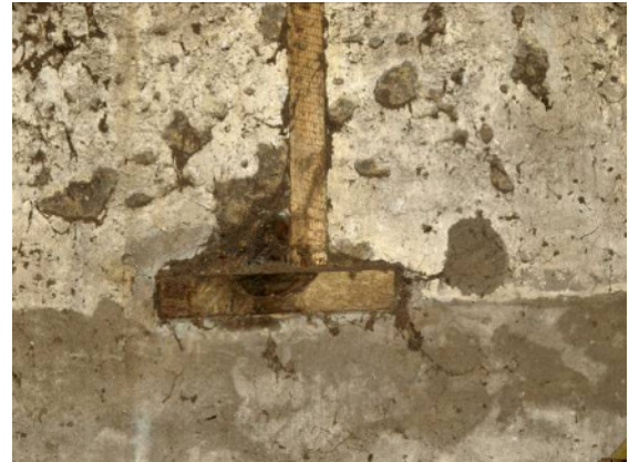
Fig 20 S wall former drive shaft location
