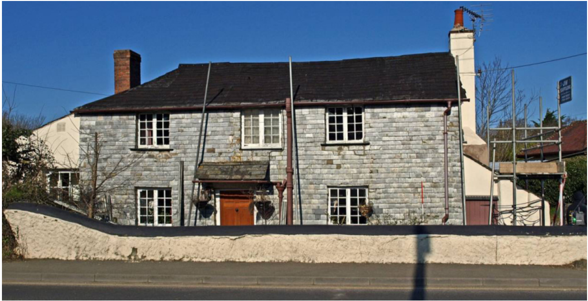
Fig 6 Hillhead Farm Cottage SE front
