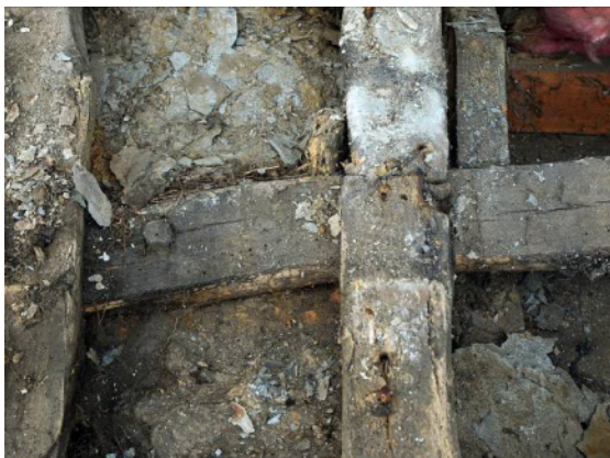
Fig 25: E wall: purlin pegged to cob wall
