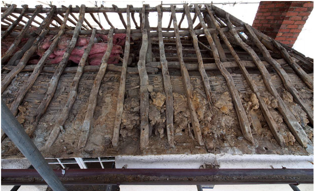
Fig 14 North roof slope towards right (SW): hip coeval with main part of roof (note lath and plaster ceiling at this end of house); two short lengths of common rafter cut away to remove water tank
