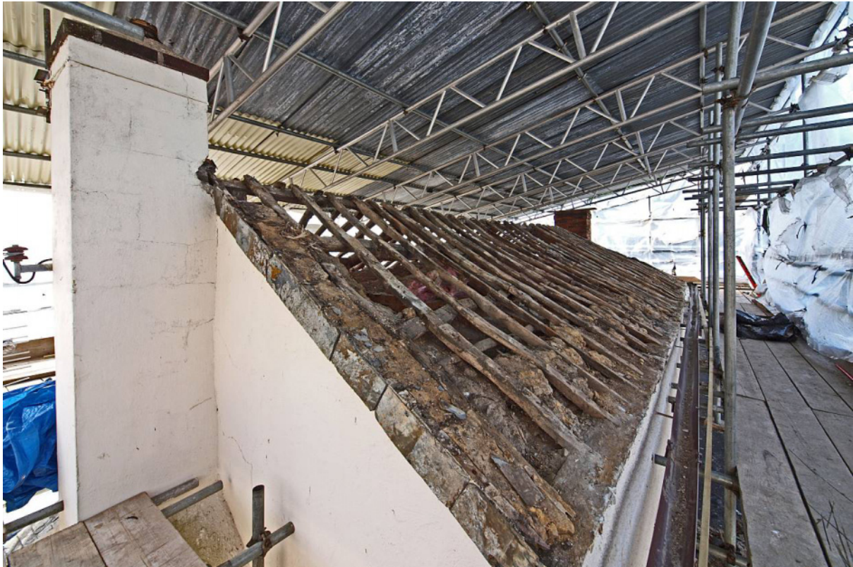
Fig 11 Roof timbers stripped of slates from N
