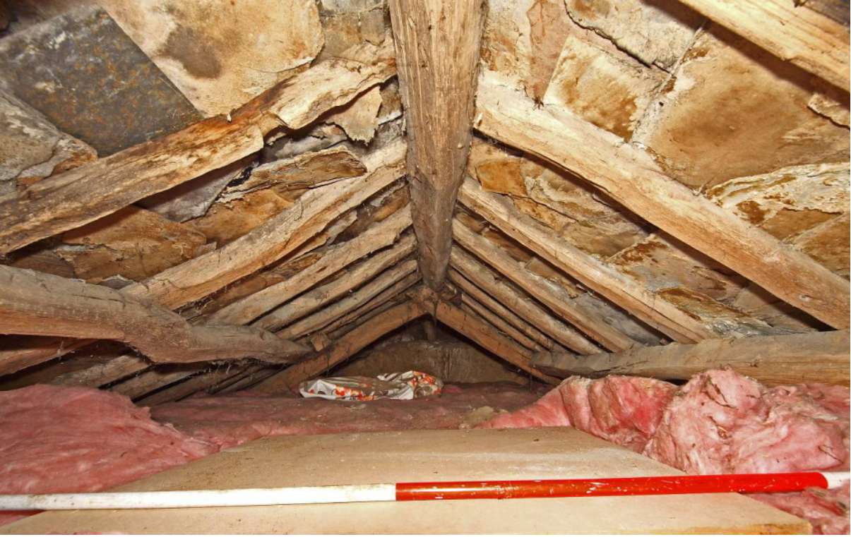
Fig 9 Roof space from SW with original rag slates in situ
