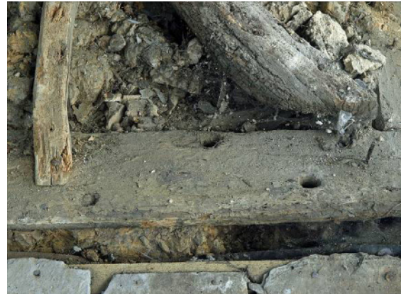
Fig 28 W wall-plate: reused ship's timber
