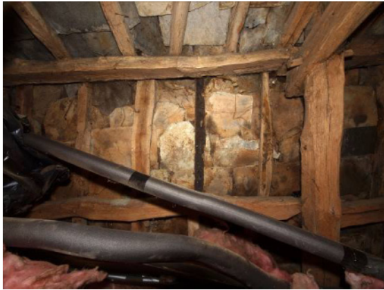
Fig 23: 4 rafters: reused ship's timbers
