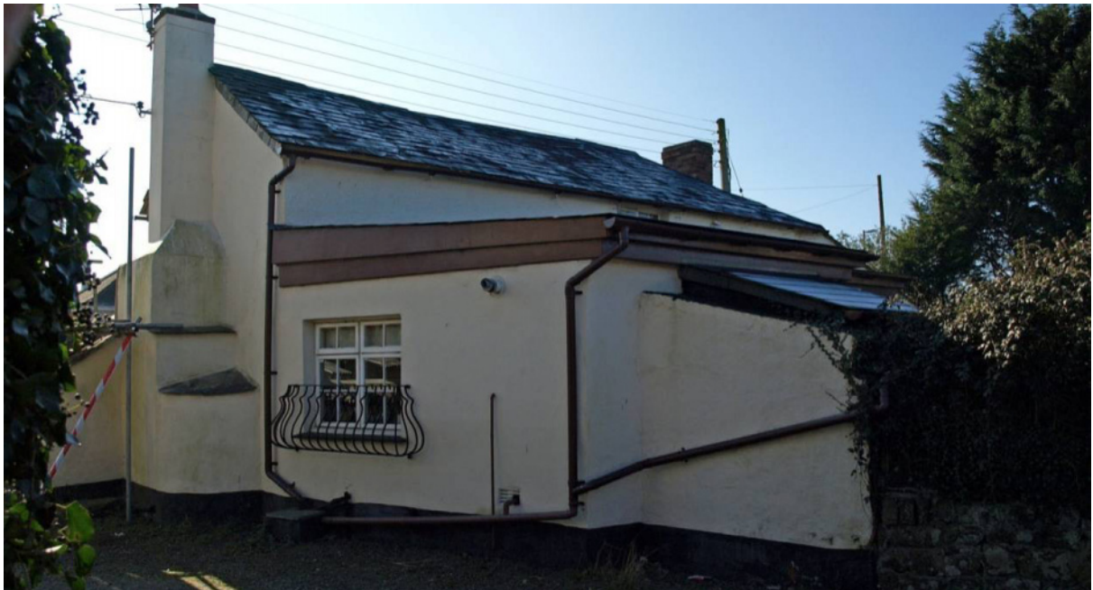
Fig 7 East elevation from N
