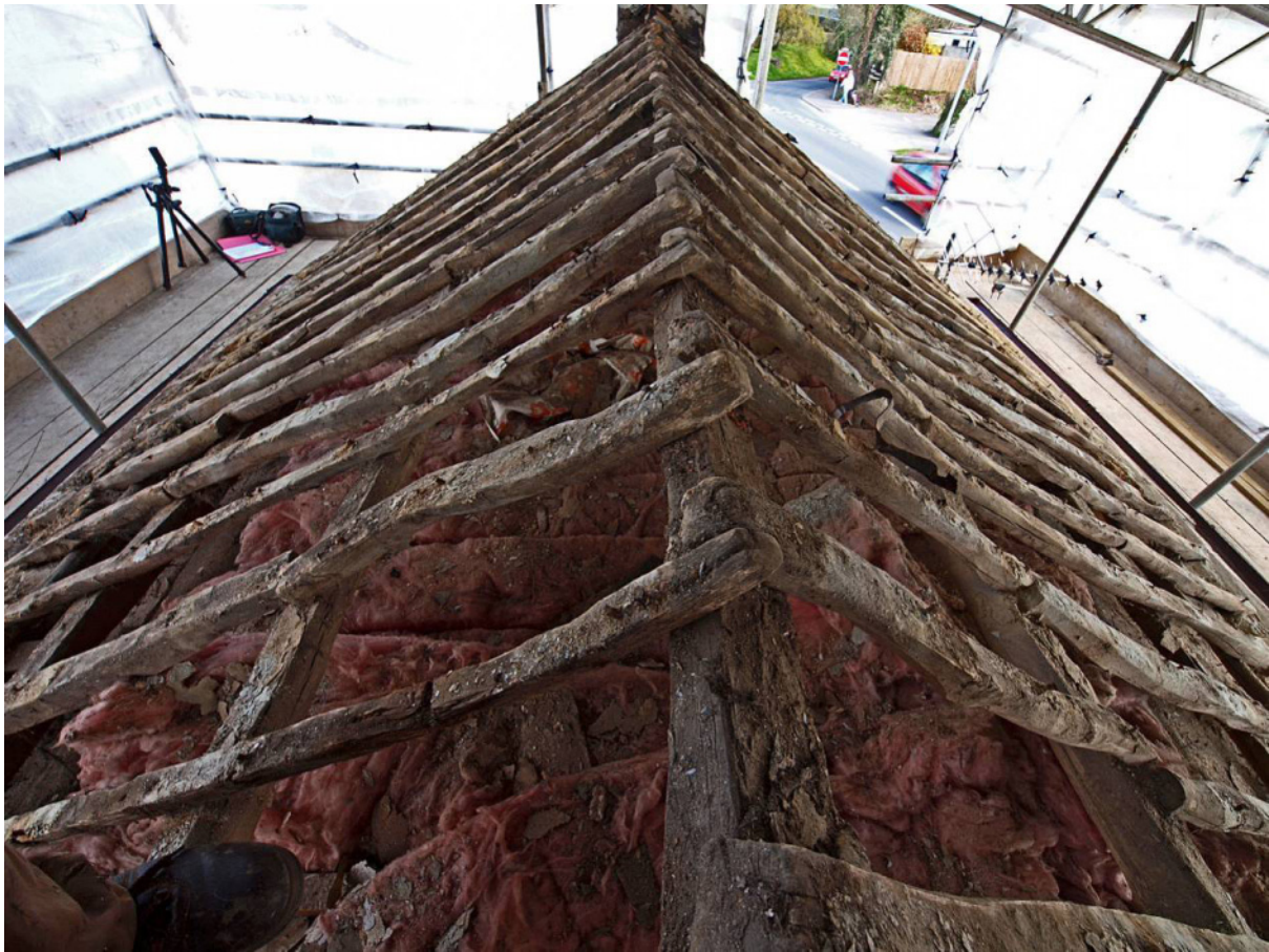
Fig 22 Roof from above towards east gable end
