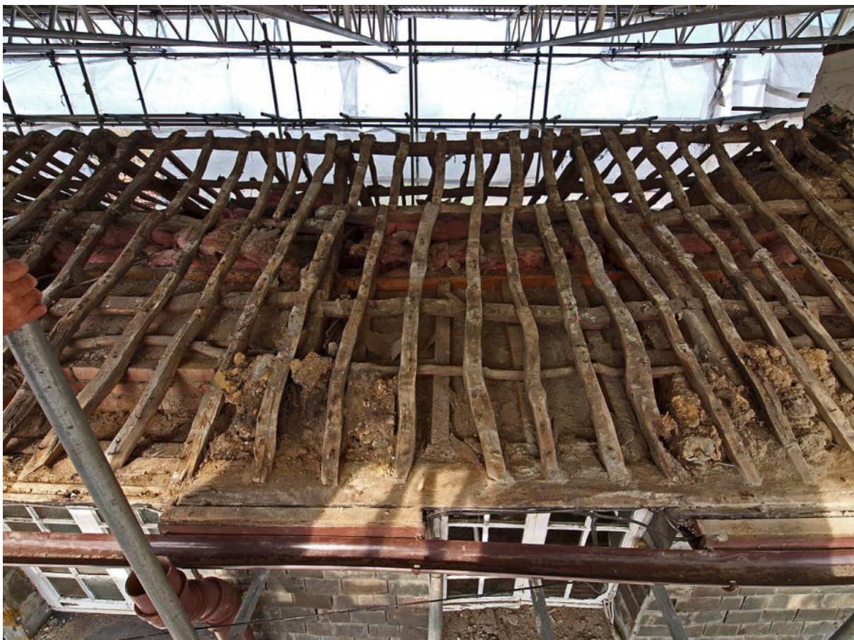
Fig 20 South roof slope left of centre (note cob walling between rafters)
