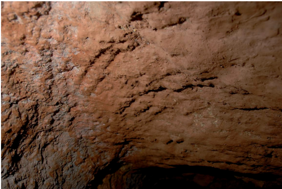
Fig 46. A section of the wall of the western drive showing evidence for having been dressed with a pick.
