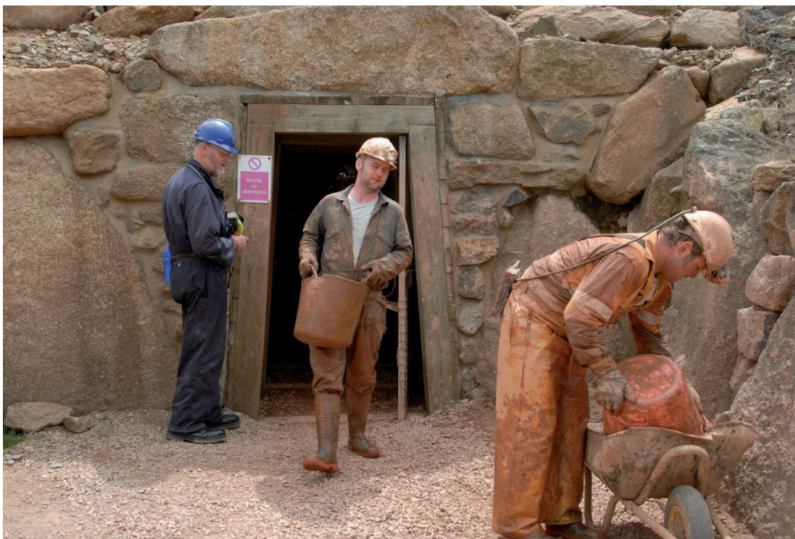
Fig 27. All material excavated from the western drive had to be manually removed using a bucket chain (here showing John Dowling and Luke Anstice). AJ, one of the Geevor guides, looks on.
