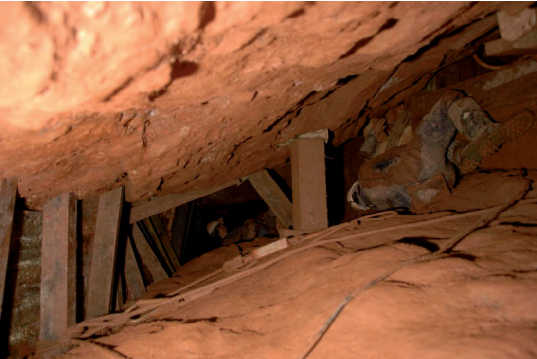
Fig 29. This view southwards in the eastern drive gives a good impression of the amount of timberwork needed to support the hanging wall during clearance operations. Further low-level props are being installed in this view.
