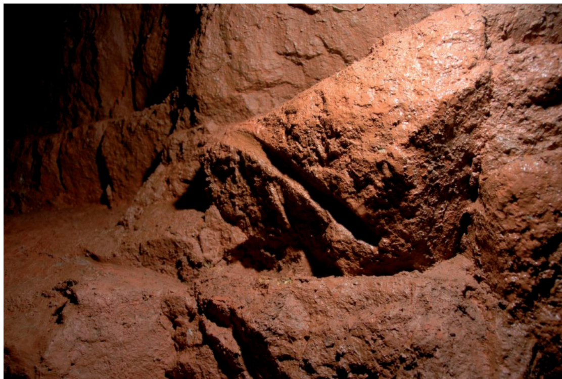
Fig 45. A hand-cut drill hole in the roof of the western adit near its southern end.
