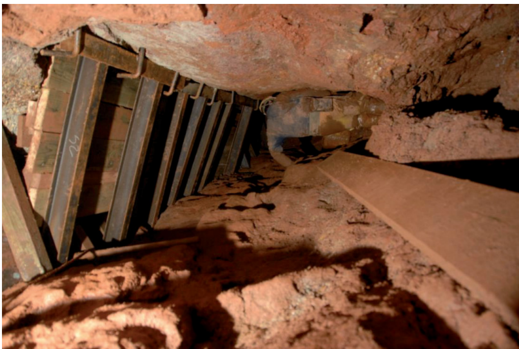
Fig 35. Looking south in the eastern stope. The plank is resting on the rock pillar found at this point.
