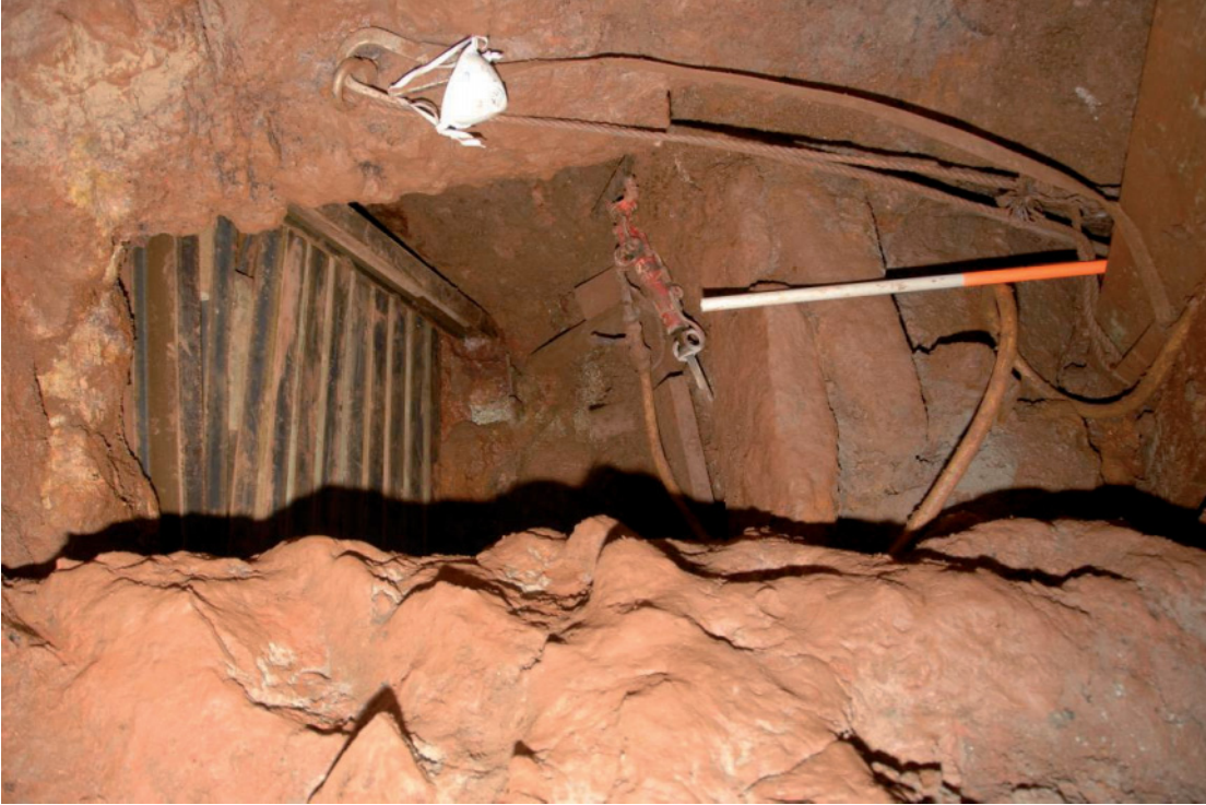
Fig 30. Looking from the southern end of the western drive into the connection with the eastern stope. The steelwork in the roof was installed to support the loose material above, which runs to surface. The stone wall between the two tunnels survived at this time.
