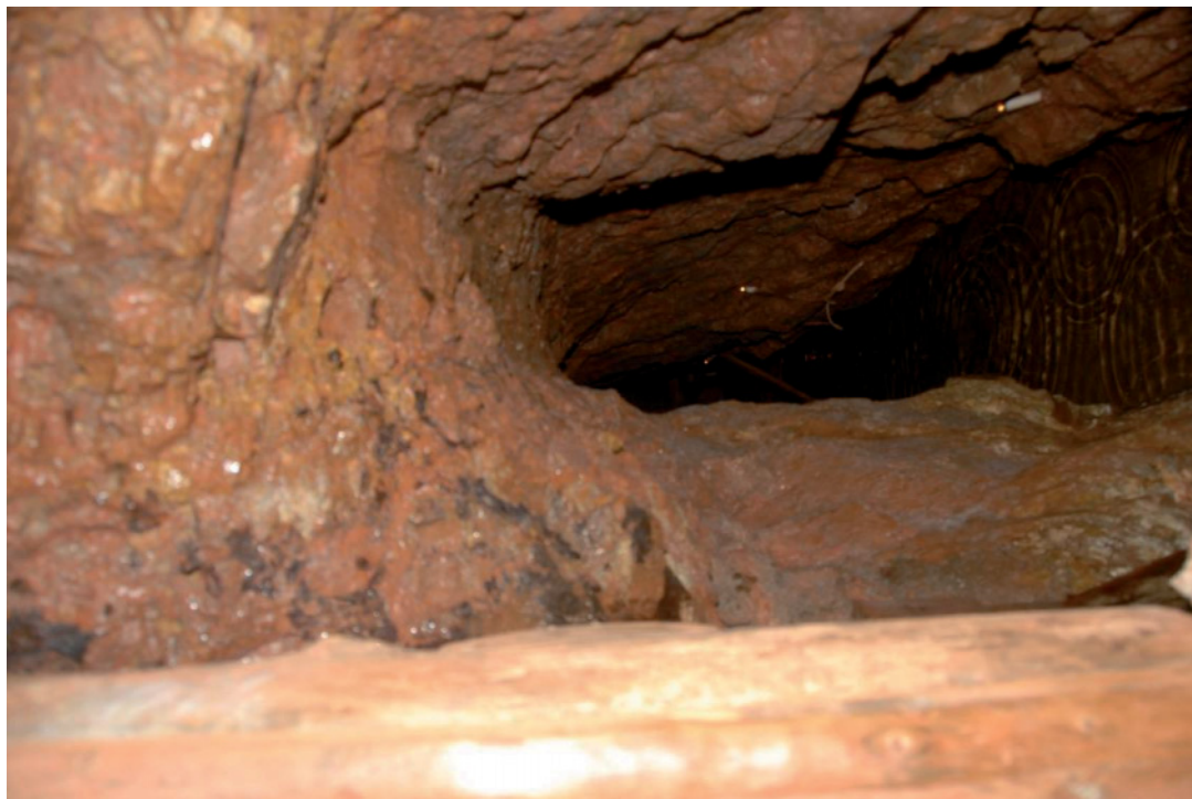
Fig 18. Looking south from Old Mexico Shaft into the western drive before work began, showing the water standing in it and the 'candles' installed by PCH. The drive was blocked a few metres upslope.
