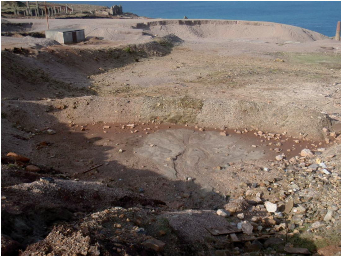
Fig 21. The area at the toe of the waste dump agreed as the site for the disposal of the material excavated from the Wheal Mexico adit system.
