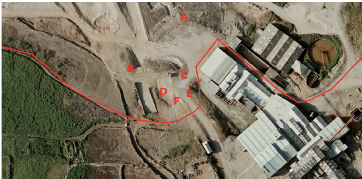
Fig 13. A 2005 Cornwall County Council aerial photograph of the lower part of the Geevor site showing (red line) the route of the main sewer and the locations of A) Mexico adit entrance, B) Mexico adit exit, C) New Mexico Shaft, D) Old Mexico Shaft, E) Mexico Ladderway Shaft, F) Sulphide Bay East Shaft. © Cornwall Council.
