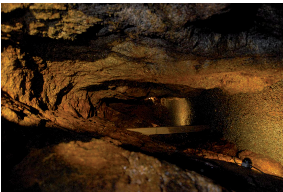
Fig 66. Looking north along the western drive showing the gravel flooring and a timber prop supporting the wall.
