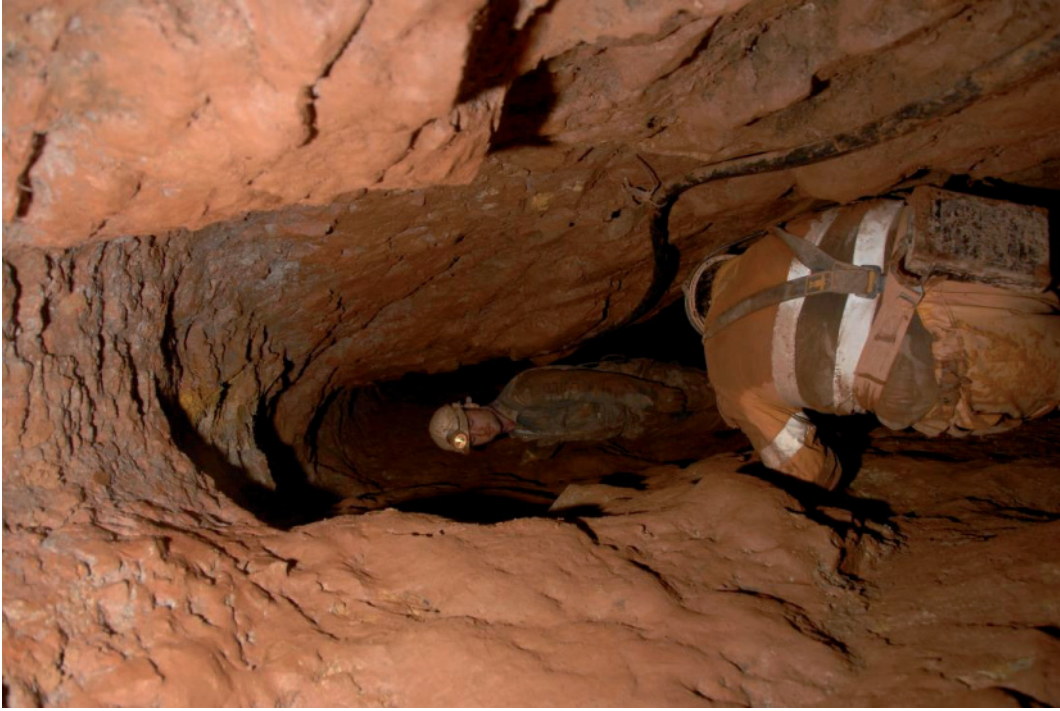
Fig 24. A chain of contractors (here Luke Anstice and Colin Davies) hauled buckets of material excavated from the western drive back to Old Mexico Shaft, from where it was carried to surface for disposal. The narrowness of the adit is readily apparent.
