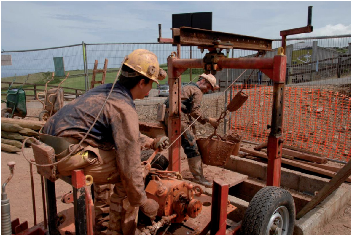
Fig 25. Douglas Wheatcroft and John Dowling using a compressed-air Holmans' winch and gantry to haul buckets of spoil up from the eastern drive via Sulphide Bay East Shaft. This approach greatly reduced the amount of manual work involved in clearing the spoil in this drive, as well as limiting impacts on the visitor tour.
