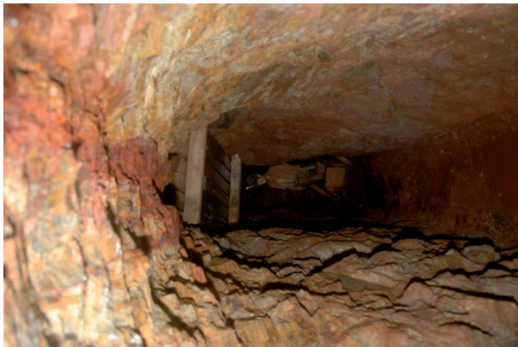
Fig 17. A view from the crosscut on the original visitor tour to Sulphide Bay East Shaft on the eastern drive prior to works, where PCH had set up a tableau including this mannequin.
