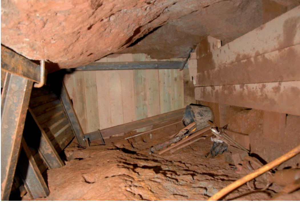
Fig 34. The limits of excavation on the eastern stope once the unexcavated fills had been bratticed off and the timber floor had been partially constructed.
