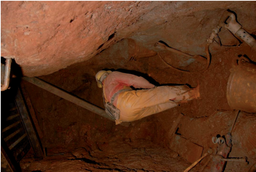
Fig 33. Work under way at the southernmost extent of the excavated part of the eastern stope. Mervyn Brakespear is standing on the fills of 'Windlass Shaft', whose curved eastern wall is just visible to his left.
