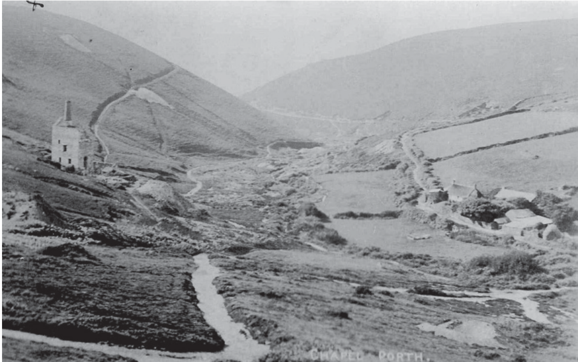
Fig 125. A late 19 th century or early 20 th century archive view looking westwards down Chapel Combe showing the abandoned pumping engine house on Charlotte United Mine. A comparison with the view today makes it clearly evident how much willow and scrub vegetation has subsequently developed in the valley base. Clive Benney Collection.
