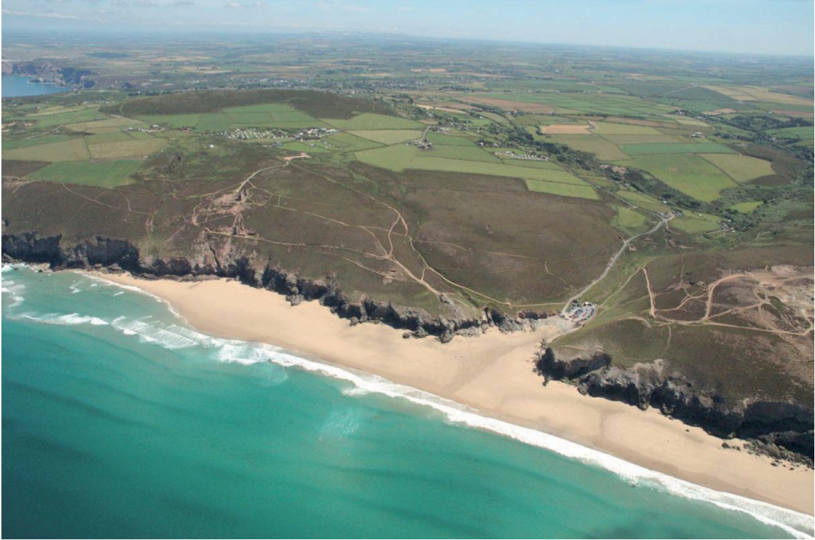
Fig 16. An aerial view of the central part of the project area from the sea, with St. Agnes Beacon in the distance (upper left), Wheal Coates (left), Chapel Porth and Chapel Combe (centre) and Great Wheal Charlotte (right). HE Photograph F69-011.
