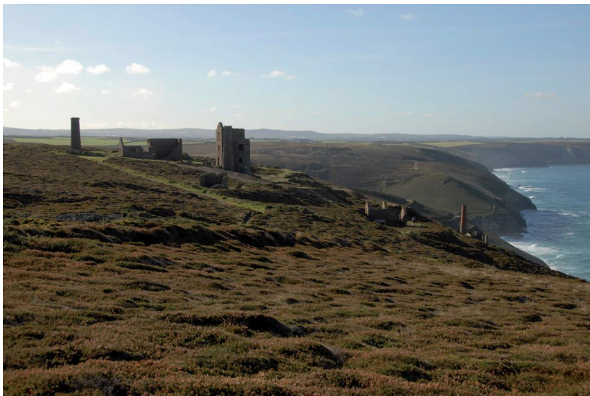
Fig 91. The clifftop buildings of Wheal Coates from the north, including (left to right) the chimney [190373], the horizontal whim engine house [190376], the all-indoor whim engine house [190378], Smithy [190343], the stamps engine house [190381], calciner [190346] and pumping engine house [190390]. HE Archive.
