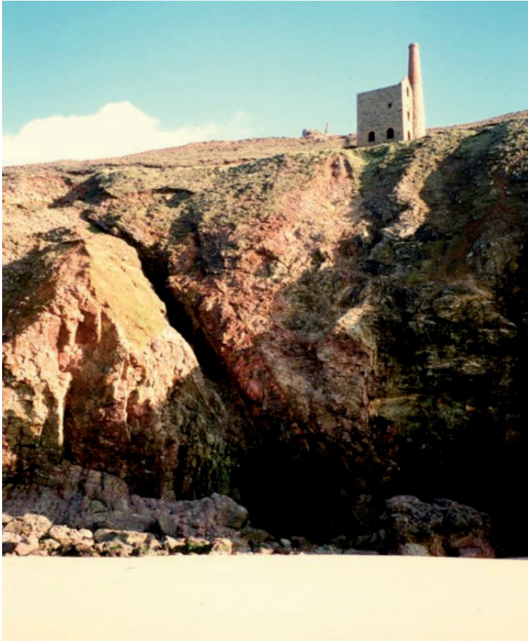
Fig 78. The cliff-face outcrop workings on the Towanroath Lode, showing its south-dipping nature. Towanroath Vugga is at its base, whilst the vertical upper section of Towanroath Shaft intersects the lode below sea level. HE Archive.
