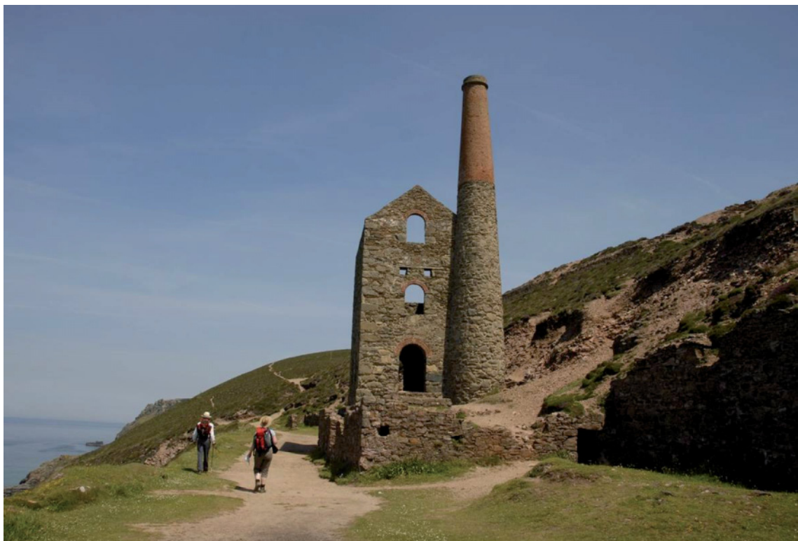
Fig 87. Towanroath pumping engine house from the south, with the remains of the boiler house eastern wall (right) and the walling around the concrete base for the 20 th century horizontal pumping engine (lower centre). A comparison with Fig 86 indicates the extent of the rebuilding of this elevation. HE Archive.
