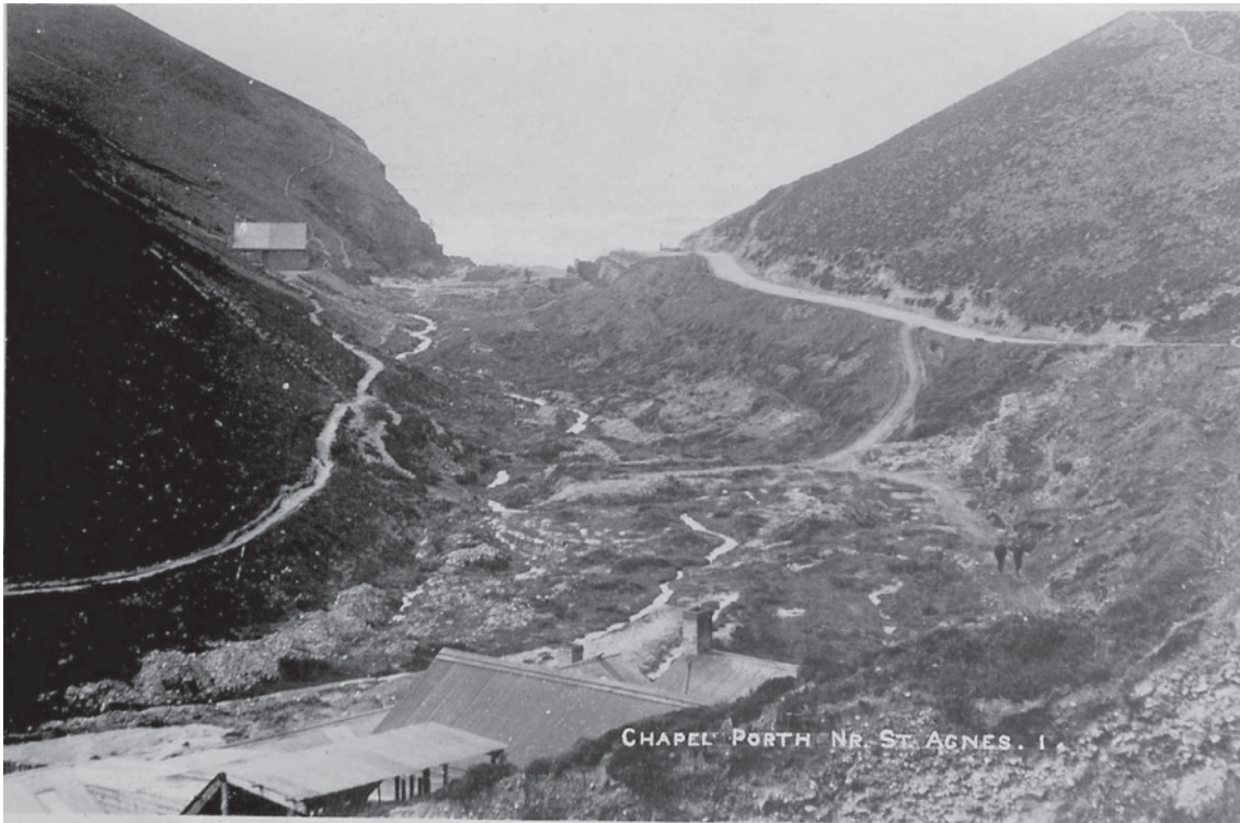
Fig 108. A probably early 20 th century archive view looking down Chapel Combe across the Old Century tin works [190510]. The disturbed nature of the valley bottom indicates abandoned tin streaming activity. In the background (left) can be seen the bungalow [198501]. Clive Benney Collection
