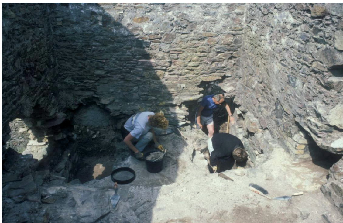
Fig 98. Volunteers excavating the interior of the northern part of the calciner [190346] prior to its conservation during 1986. Adam Sharpe Collection.
