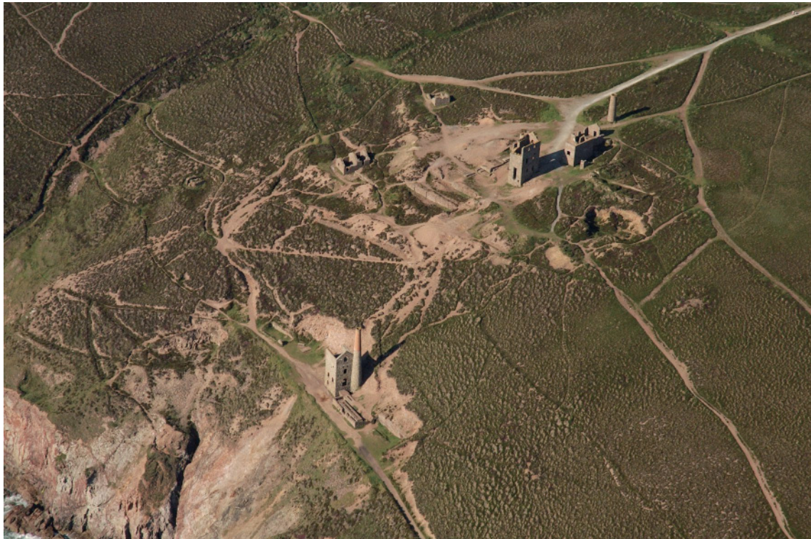
Fig 149. The effects of visitor pressure on thin soils can be found at many points within the project area, but are particularly evident in this aerial photograph of Wheal Coates. Multiple, braided paths have developed on thin soils, removing the vegetation and topsoil and promoting erosion. HE Archive.
