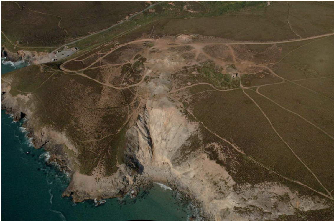
Fig 131. A recent aerial view of Porthgwidden Cove and the remains of Great Wheal Charlotte. Much of the spoil deriving from mining operations seems likely to have been dumped over the cliff into the back of the cove. HE F68-043.
