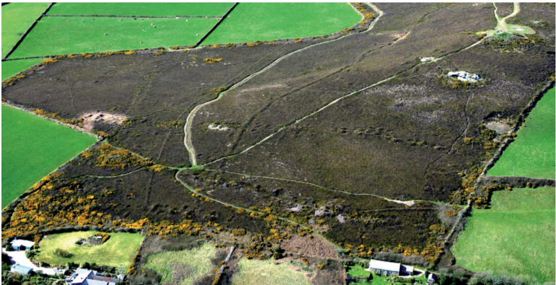
Fig 152. Much of the complex of historic mining activity in the south-west corner of the Beacon rough ground is concealed under dense furze and scrub, and furze and bracken are also encroaching around the fringes of the NT property. NT Archive.
