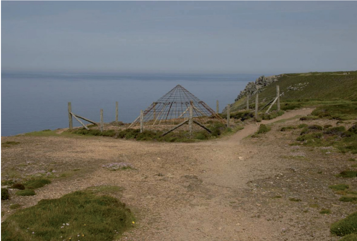
Fig 66. The large Chmyd Cap over open shaft [90048] in Wheal Bungay. The cobbled dressing floor [96758] is in the foreground. HE Archive.
