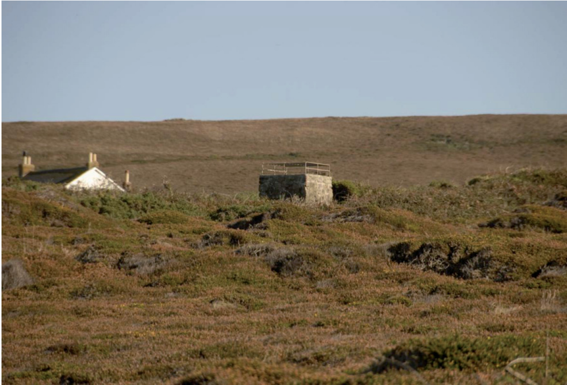
Fig 104. Water Shaft [190332] at Wheal Coates, one of the few shafts on this site to have been maintained as an open feature, in this case having been fitted with a bat castle. HE Archive.
