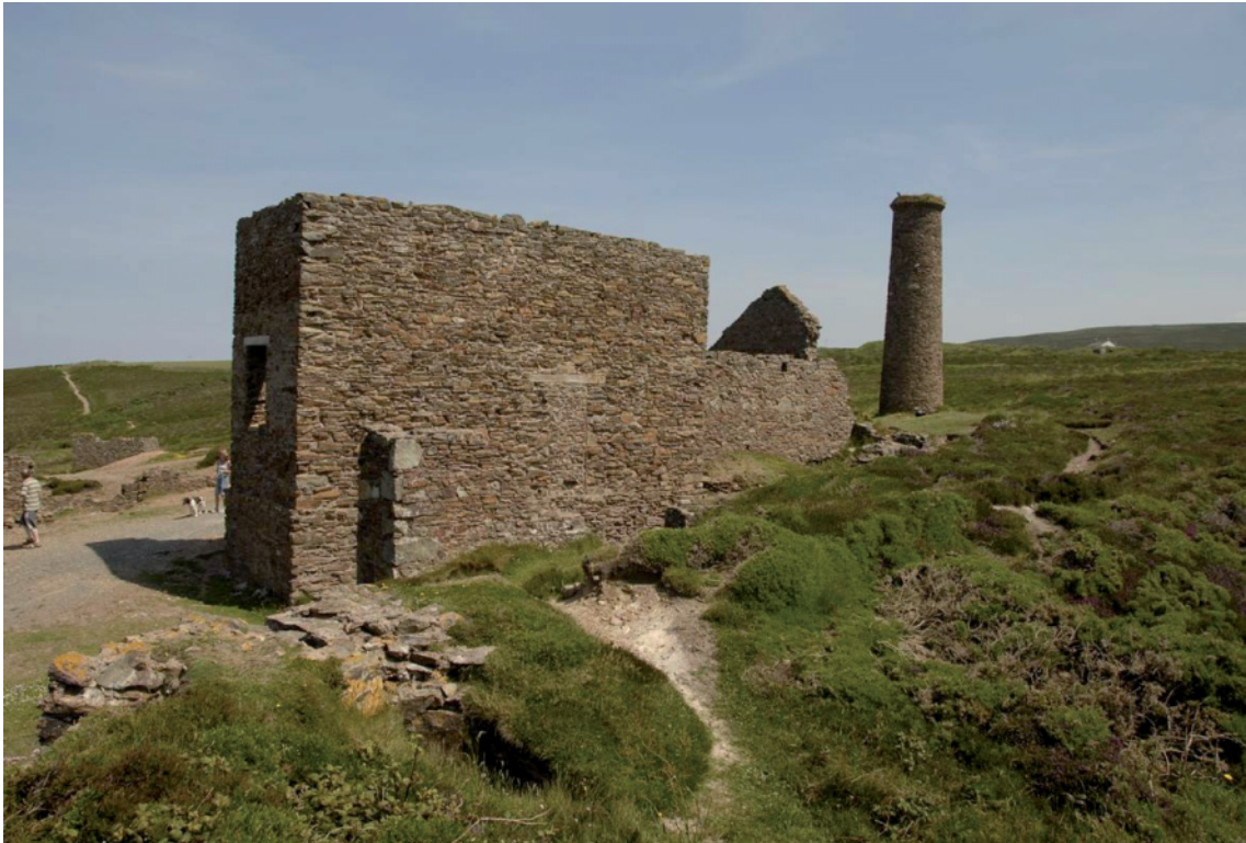
Fig 94. The boiler house [190377] (foreground), the all-indoor beam whim engine house [19037] (immediately behind) and the chimney [190373] seen from the reservoir [190394]. HE Archive.
