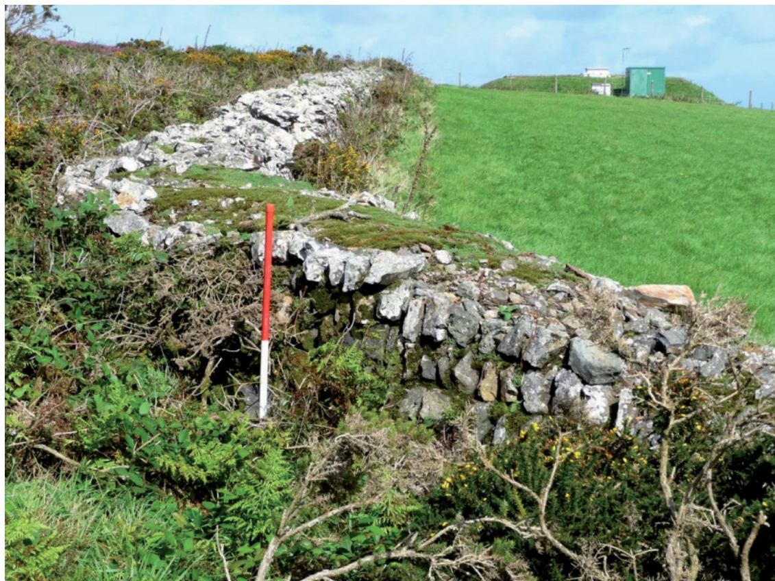
Fig 46. A stone-faced hedge [190101] bounding enclosed land on the east side of the Beacon. Stone for these boundaries would have been obtained from clearing the land but also from the prehistoric cairns on the Beacon and from a number of small quarries. HE Archive.
