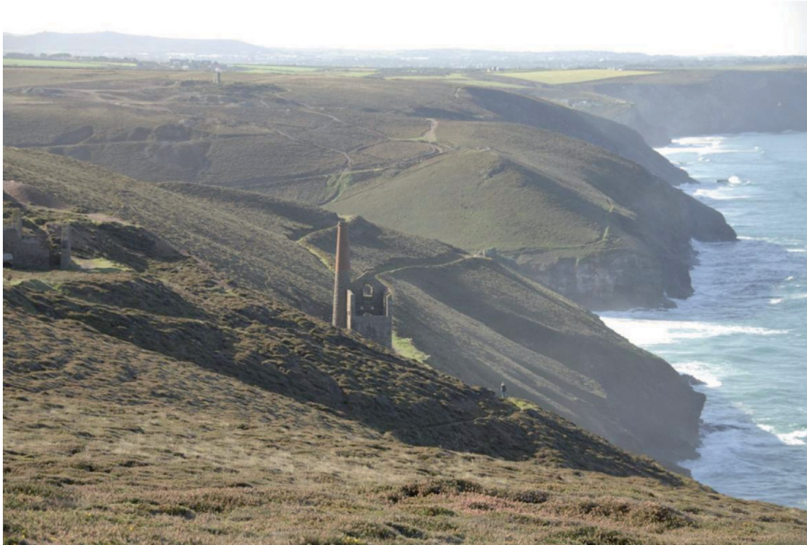
Fig 71. Towanroath shaft pumping engine house from the north, with Mulgram Hill and Charlotte Moor in the background. Two roadways can be seen running diagonally up from the left towards the summit of Mulgram Hill, the lower of these having been re-cut by the US Army in 1944. HE Archive.
