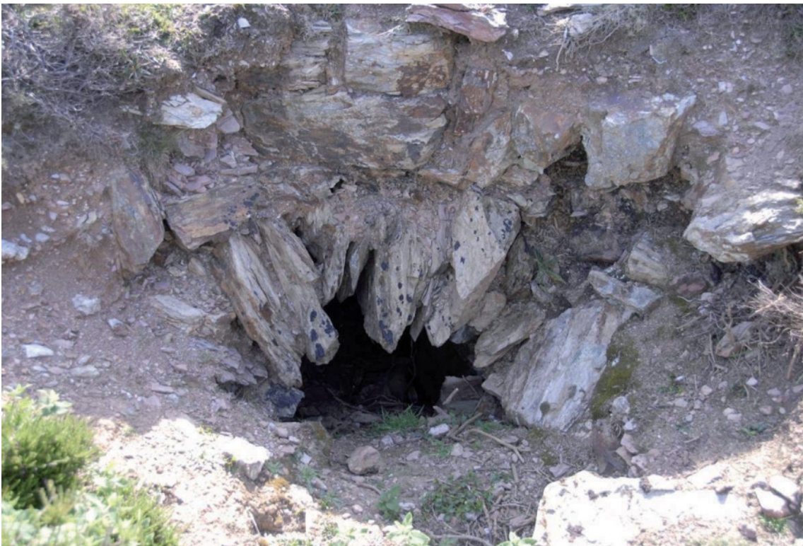
Fig 128. The almost completely blocked stone-arched portal to a high level adit [190557] in Great Wheal Charlotte, not far to the west of the remains of the pumping engine house. This adit might have channelled water pumped by the engine to dressing floors sited just down slope. HE Archive.
