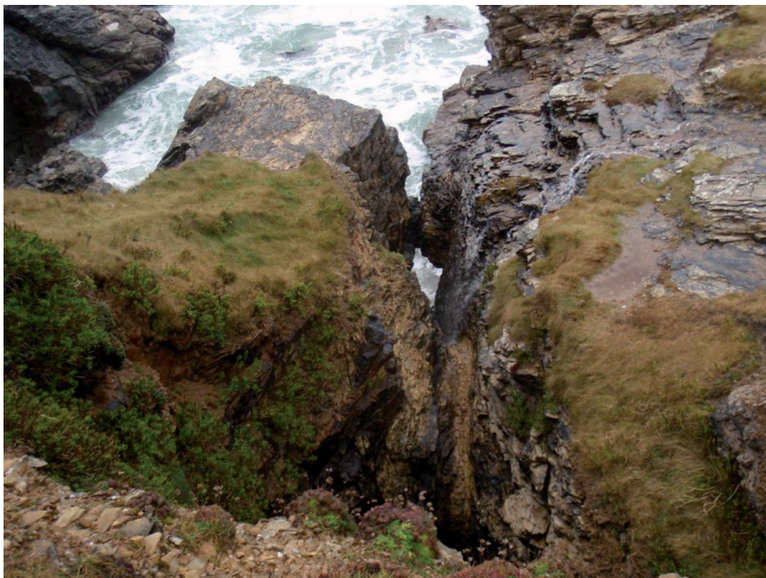
Fig 118. The site of St. Agnes Chapel [190469] was probably over the non-eroded top of one of the two sea caves at Chapel Porth called the Two Vugs [190470]. HE Archive.
