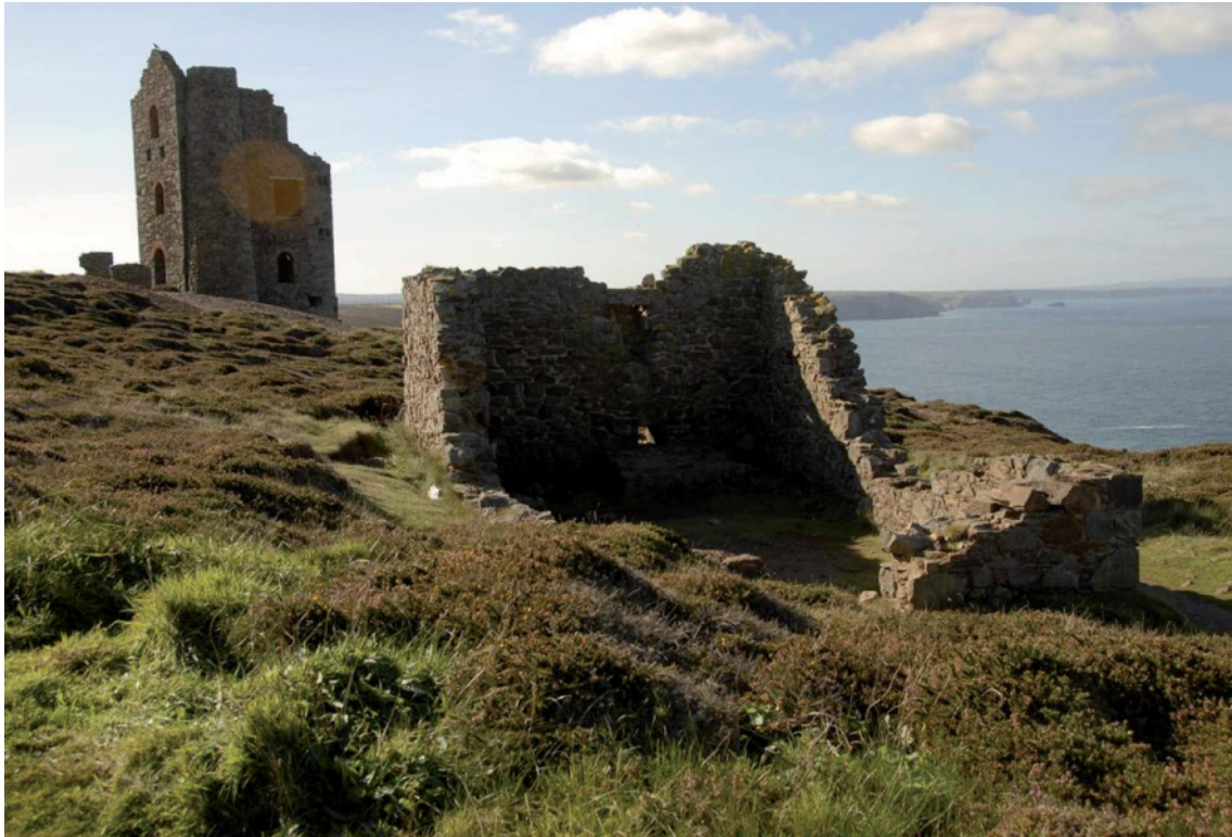
Fig 100. The mine smithy [190343] with its forge base (inside rear wall) seen from the north, with the stamps engine house [190381] in the background. HE Archive.
