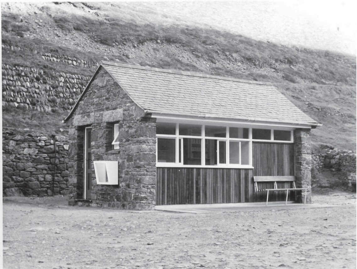
Fig 115. The first purpose-built café [190499] constructed at Chapel Porth in 1957 by the NT. This was destroyed by arson in 1984. NT Photo Archive.
