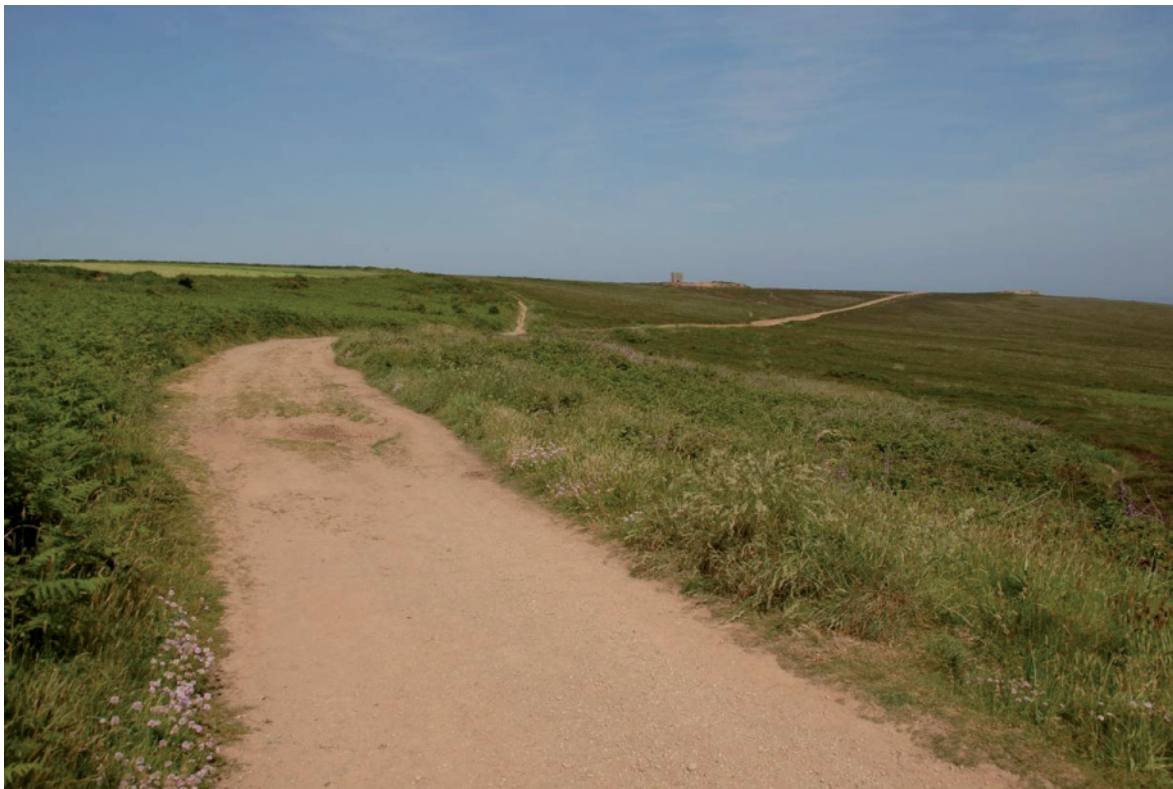
Fig 140. A section of the roadway linking Great Wheal Charlotte (on the skyline) with Towan Cross, most of this route having been upgraded by US Army Engineers in June 1944 to allow the downs to be used for the temporary accommodation of troops awaiting embarkation to the Normandy beaches on D Day. HE Archive.
