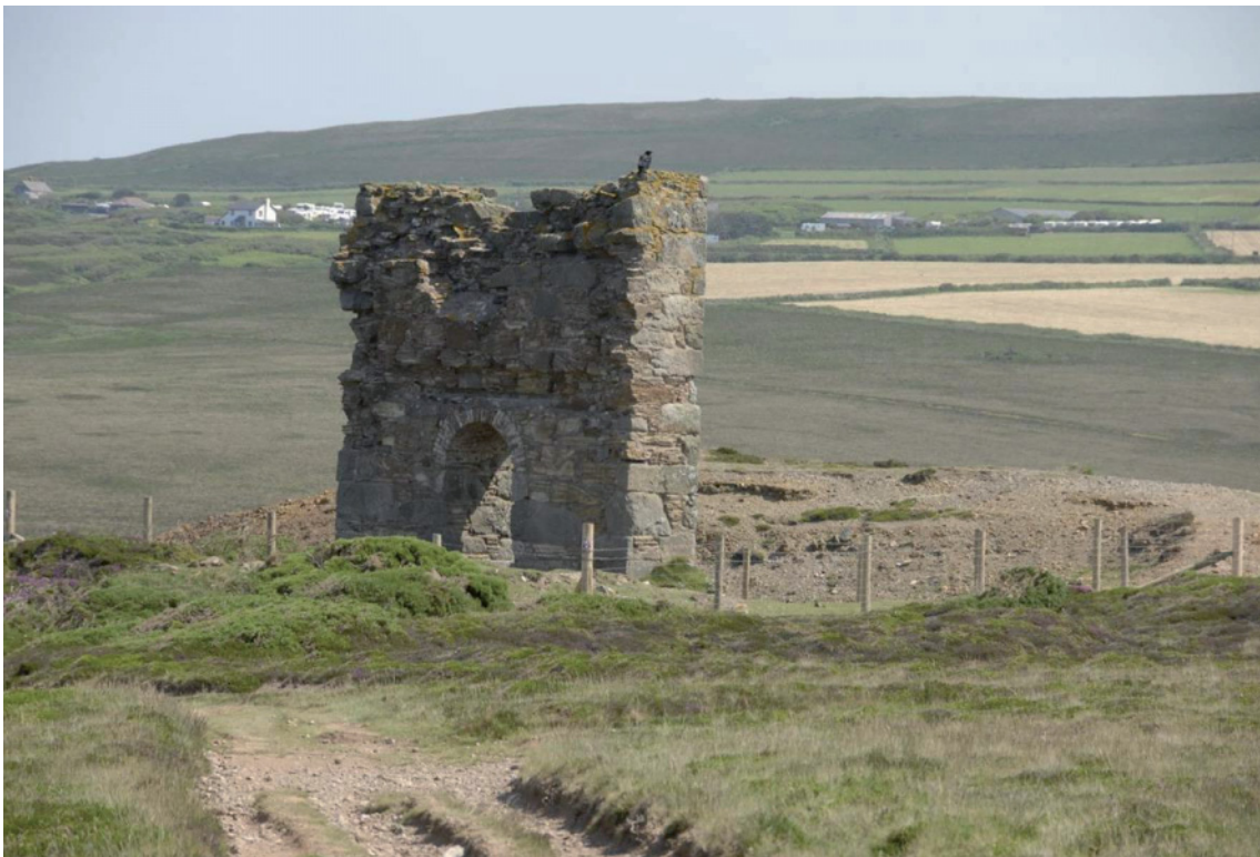
Fig 136. Great Wheal Charlotte engine house bob wall today, the remains of the engine house and boiler house, together with the associated shaft site having been recently enclosed within a post and barbed wire fence. HE Archive.
