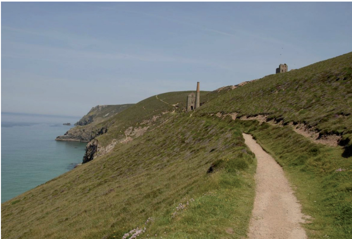
Fig 85. Towanroath pumping engine house viewed from the coast path approaching it from the south, the first view of the site gained by most visitors to the site. HE Archive.
