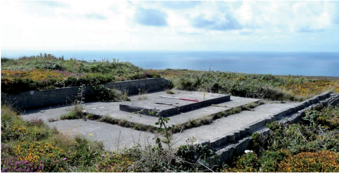
Fig 56. The concrete base of a building [190069] forming part of the World War II radar installation on the Beacon. The central plinth, on which fixing bolts are still visible, is likely to have been the base for some form of machinery. HE Archive.4
