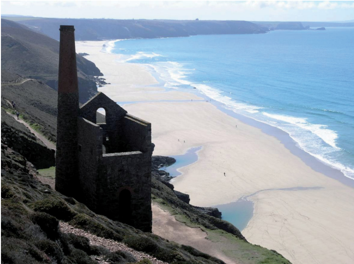
Fig 86. Towanroath pumping engine house and a section of the path (lower left) which leads to it from the clifftop buildings of Wheal Coates. HE Archive.
