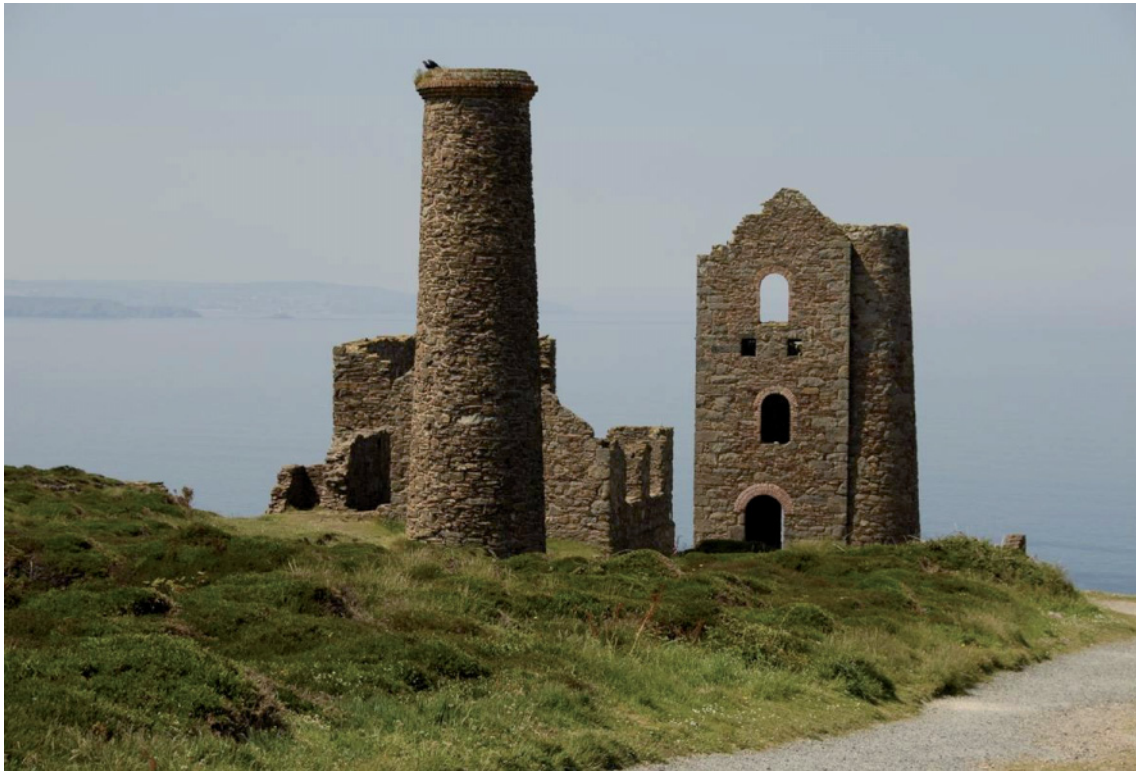
Fig 90. The clifftop building group at Wheal Coates, including (right to left) the boiler house [190377], all-indoor beam whim engine house [190378], chimney [190373], the horizontal whim engine house [190376] and the stamps engine house [190381]. HE Archive.
