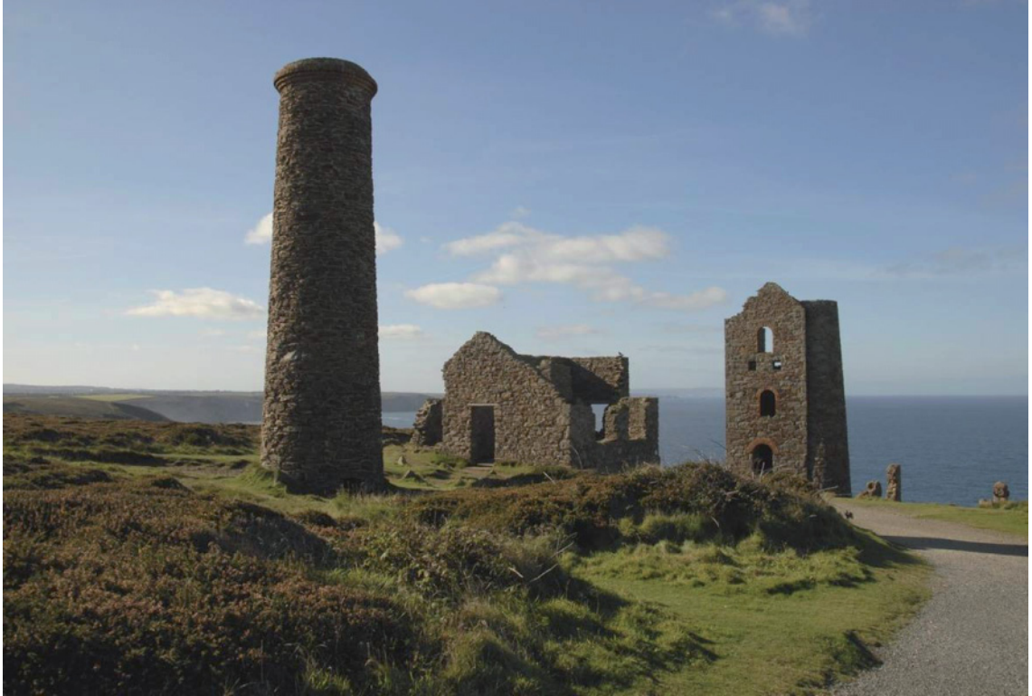
Fig 74. The cliff-top group of buildings at Wheal Coates as seen from the western end of the path from the visitor car park on Beacon Drive. This path is virtually DDA compliant. HE Archive.
