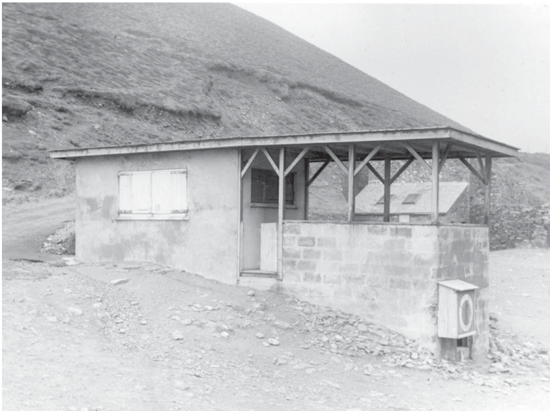
Fig 113. The blockwork-built café [190487] at the head of Chapel Porth beach, possibly adapted from a wartime structure. NT Photo Archive.
