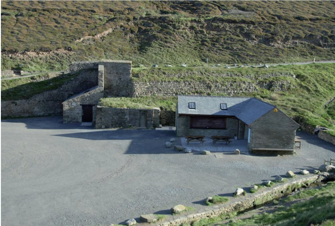
Fig 116. The modern café at Chapel Porth [190500] constructed in 1984 and partially rebuilt after a fire in 2007. HE Archive.
