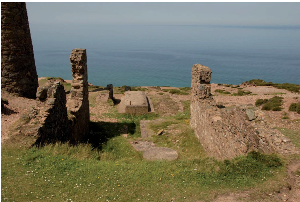
Fig 101. The producer gas generator house [190379] viewed from the east with the loadings for the gas engine (centre) and the site of the stamps and 20 th century dressing floors (upper right centre). HE Archive.
