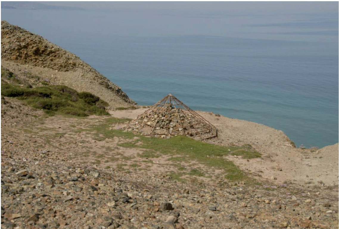
Fig 130. West Shaft [190555] in Great Wheal Charlotte, set on the cliff edge above Porthgvidden Cove, and fitted with a two part Clwyd Cap. HE Archive.
