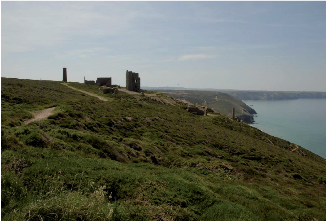
Fig 70. The Wheal Coates complex from the north, looking across the site of the original water-powered dressing floors [190299]. Again the buildings are prominent in the landscape. HE Archive.
