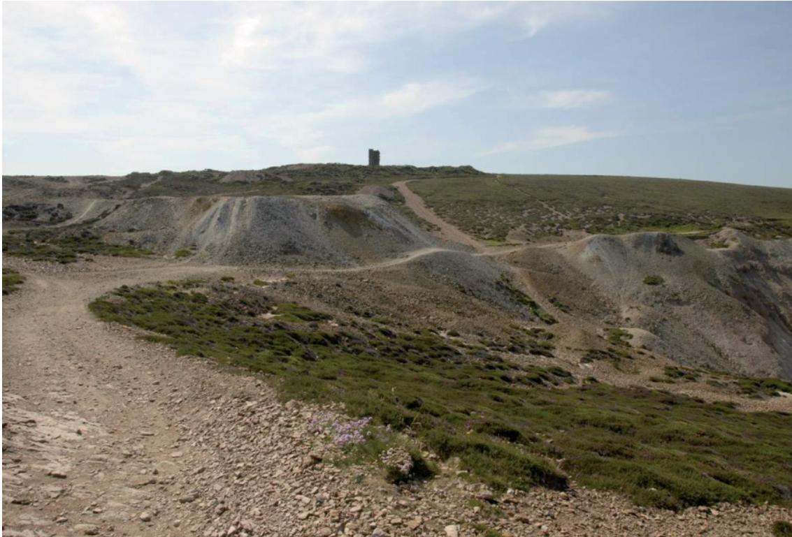
Fig 132. A view of the coastal section of Great Wheal Charlotte seen from the coast path, the bob wall of the pumping engine house [190567] being a prominent skyline feature. HE Archive.
