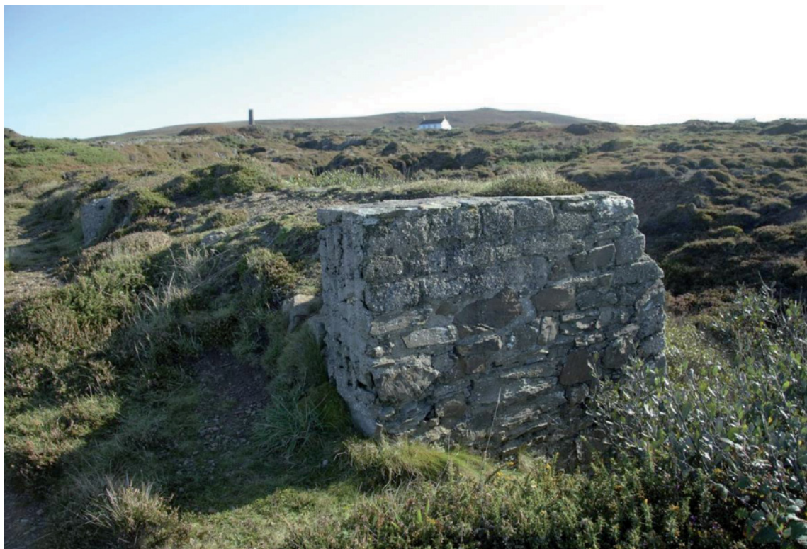
Fig 103. The mortared masonry base of the 20 th century stone crushing plant [190294] set up to rework the dumps deriving from the Wheal Coates openwork [190289]. The material produced here was probably used as hardcore or as gravel for roads. HE Archive.
