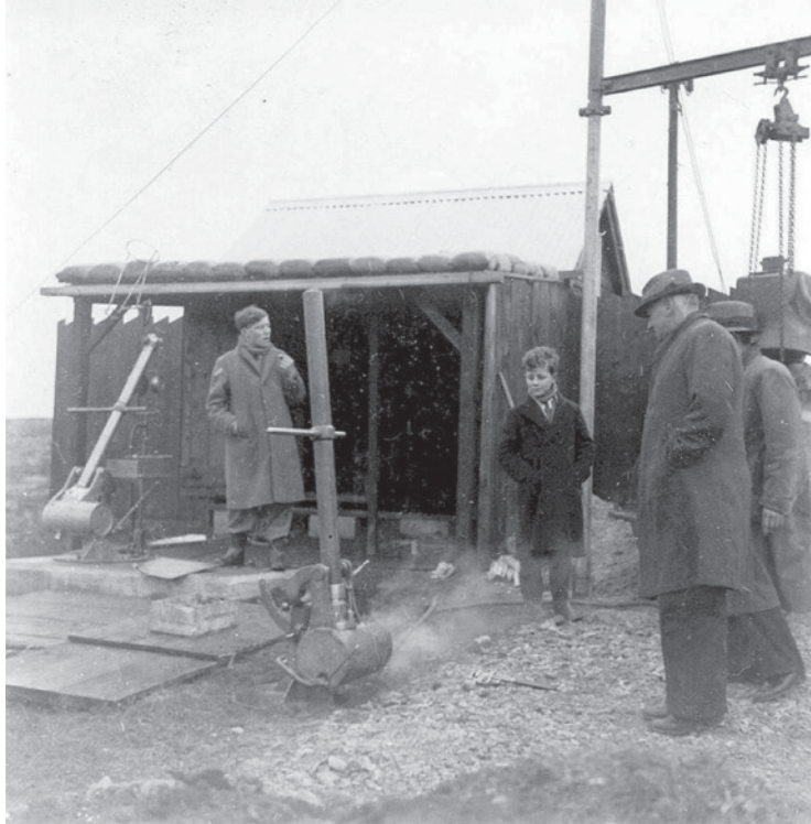
Fig 143. Cooking up a Mills Bomb in an experimental steam-powered Holman Projector. No-one gathered round seemed particularly perturbed by the possible consequences. Holman Archive, Trevithick Society Collection.
