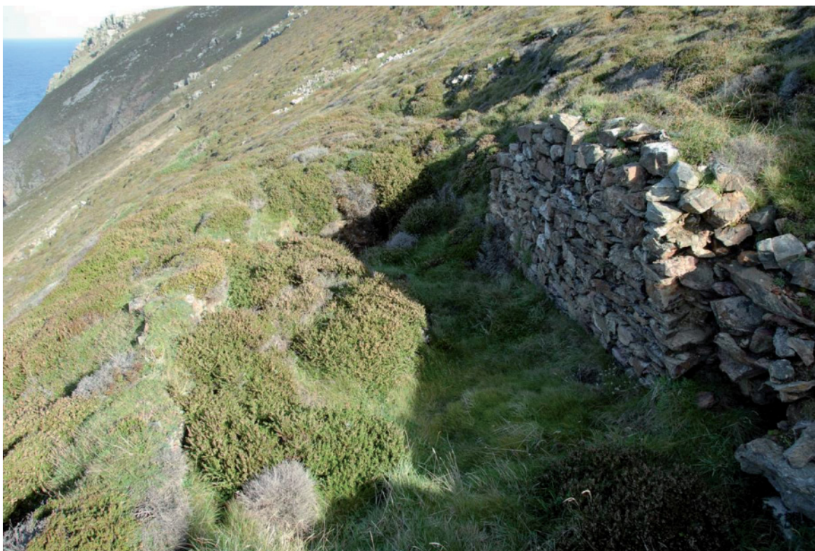
Fig 62. The remains of the early mine building [96764] to the north of Tubby's Head. The probable footway shaft [96765] lies at the northern (furthest) end of the building. HE Archive.
