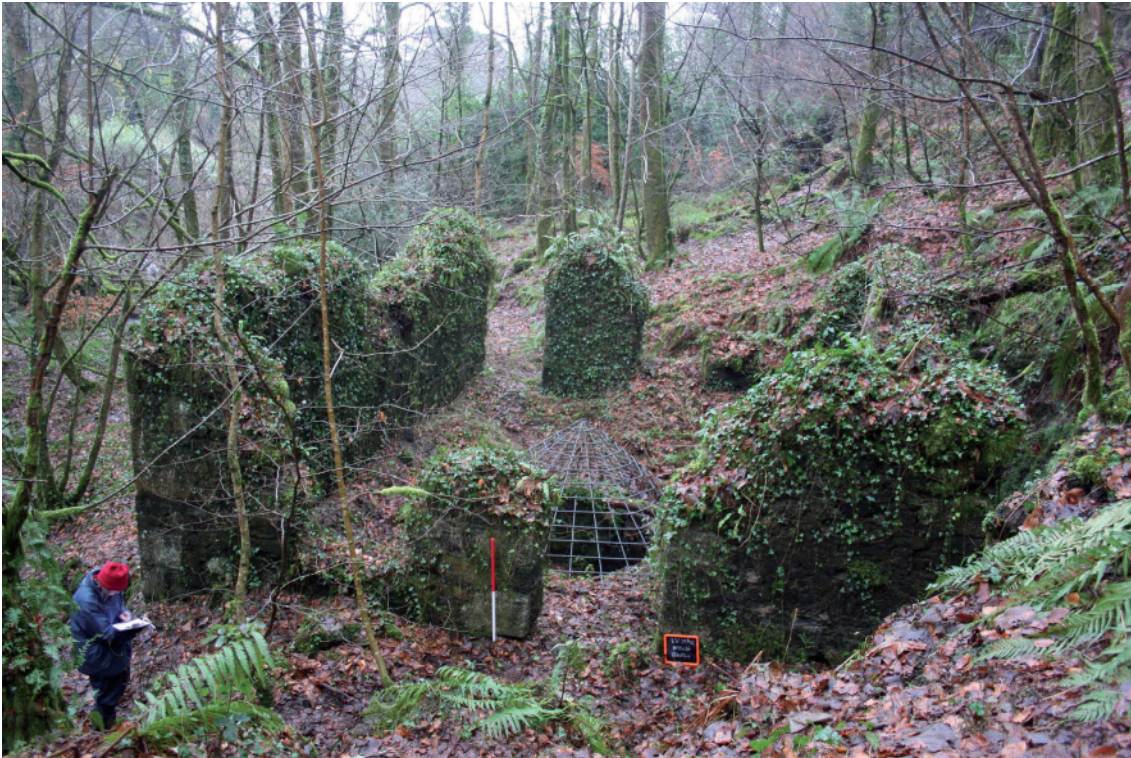
General view from the west
