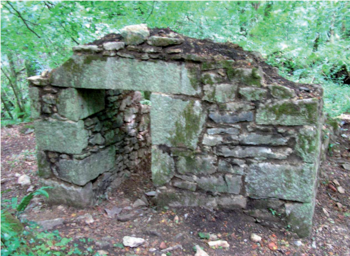
Fig 14 Cask house SW wall after consolidation
