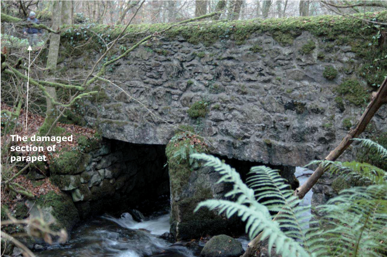
Fig 17 West face of bridge
