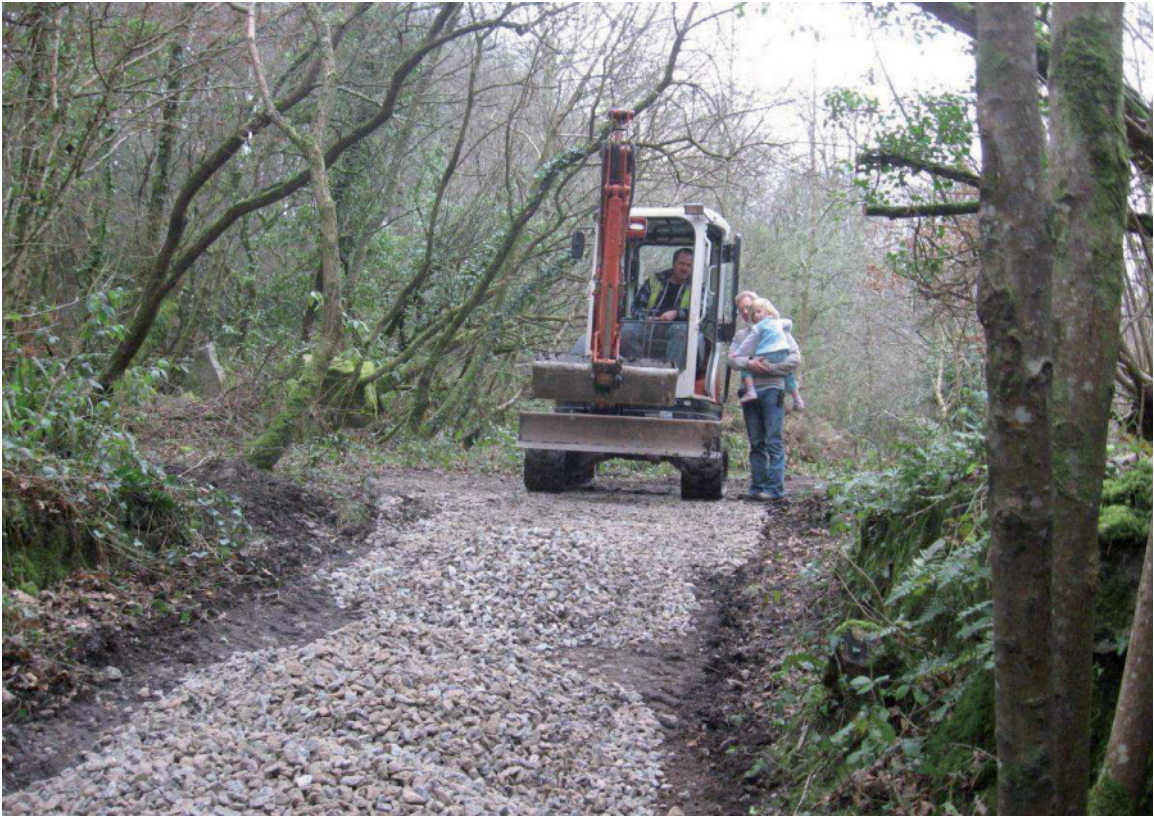
Fig 29 New granite chippings being laid to surface track
