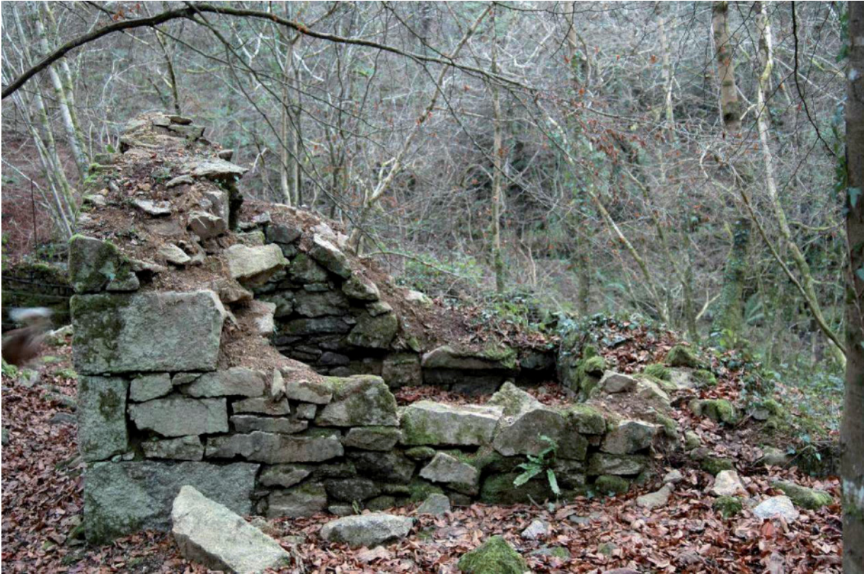
Fig 10 North-west (above) and south-east (below) walls of cask house
