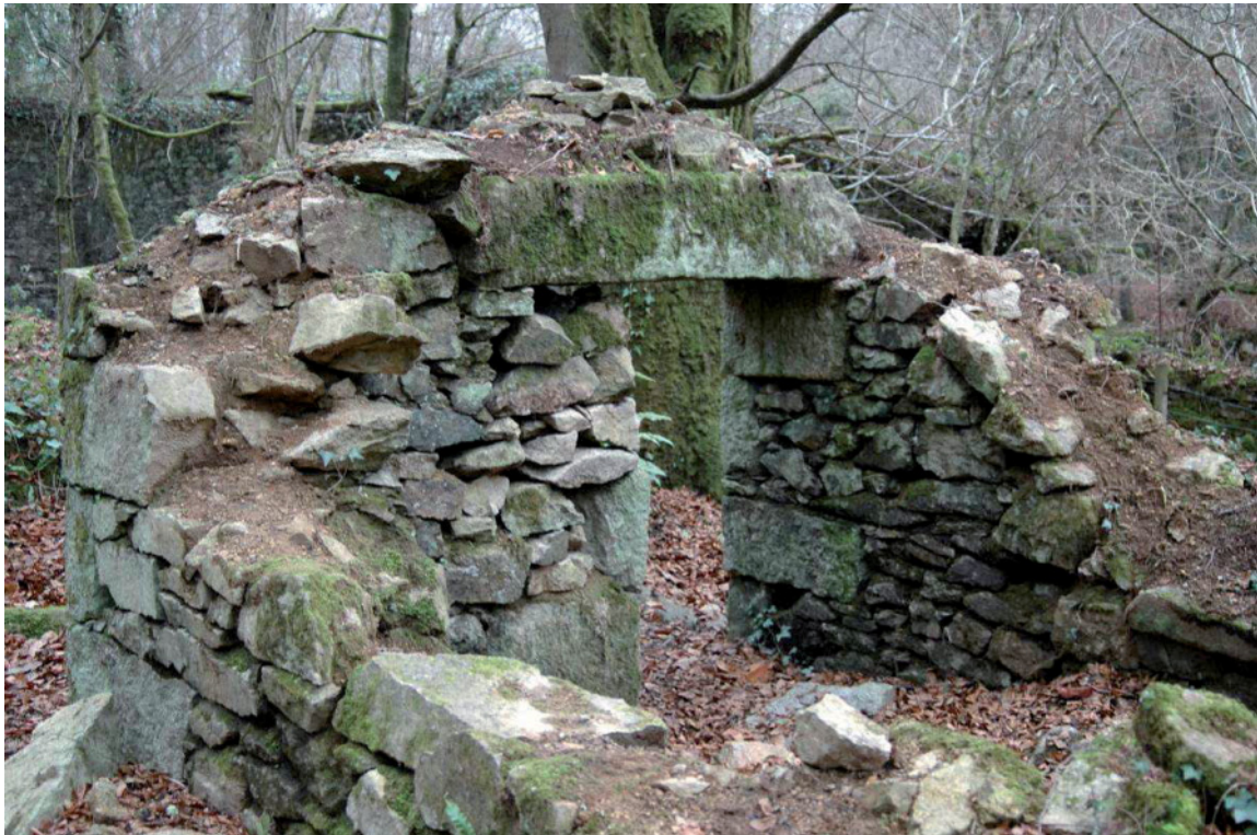
Fig 9 Cask house, SW wall, from west (above) and east (below)
