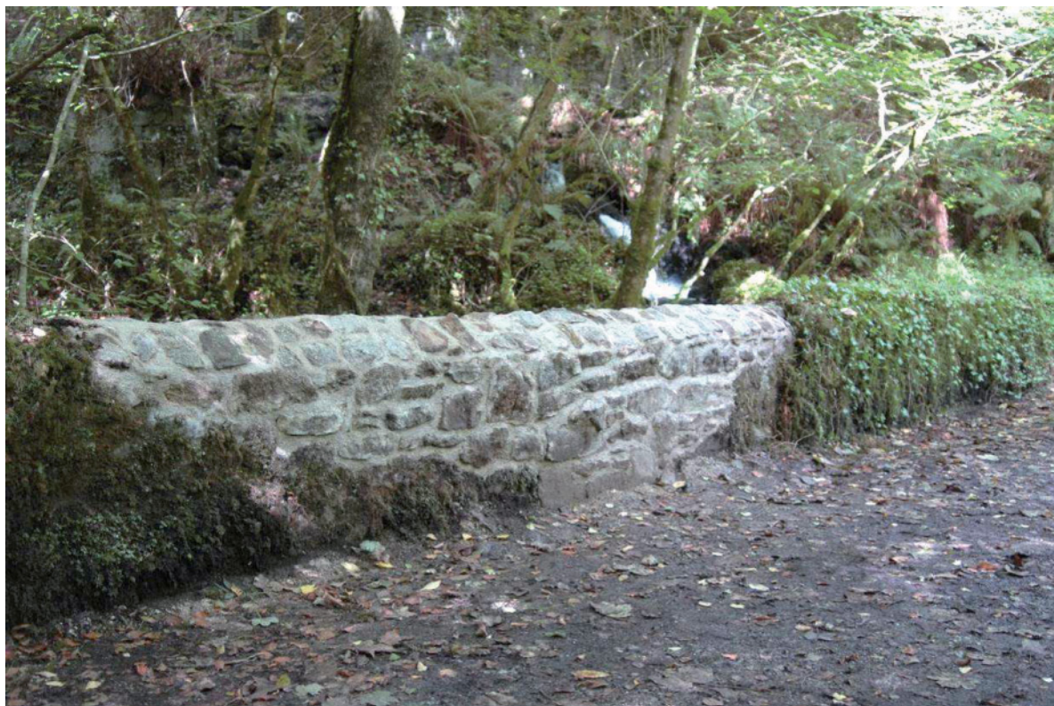
Fig 21 The rebuilt parapet
