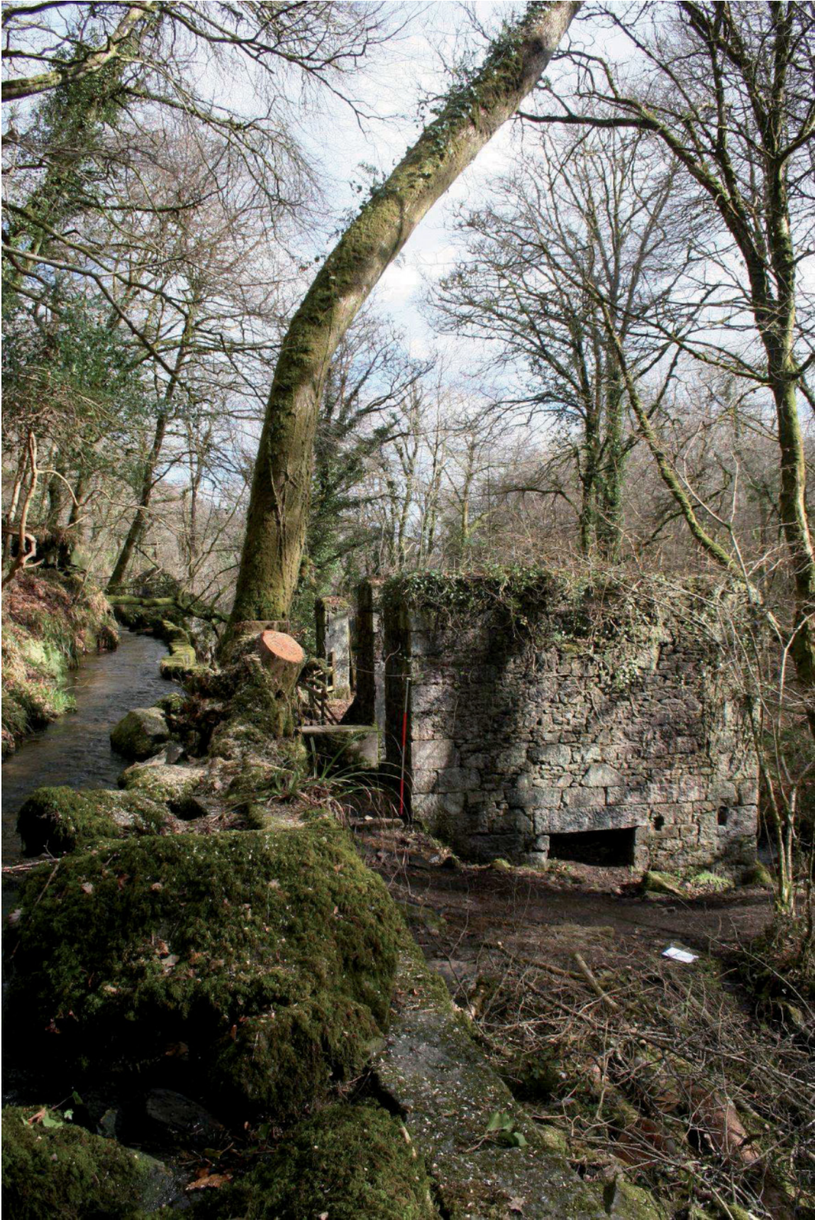
Fig 26 Tree work in progress: one tree has been felled and the other leaning tree is about to go
