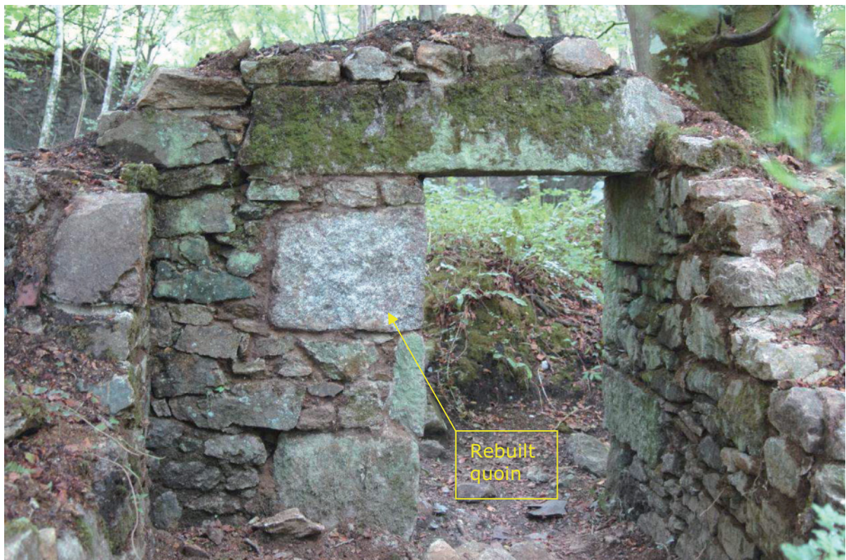
Fig 15 Cask house SW wall after rebuilding of door jamb
