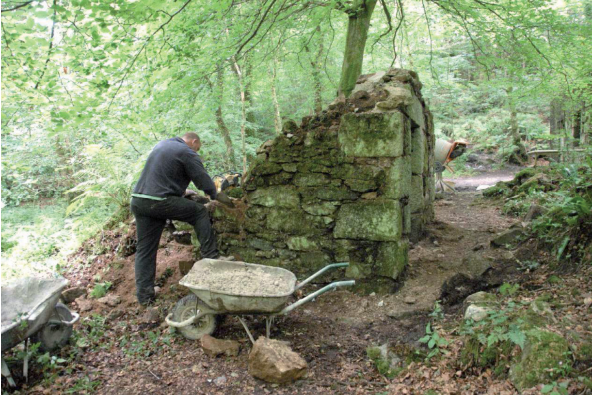
Fig 13 Work in progress on cask house
