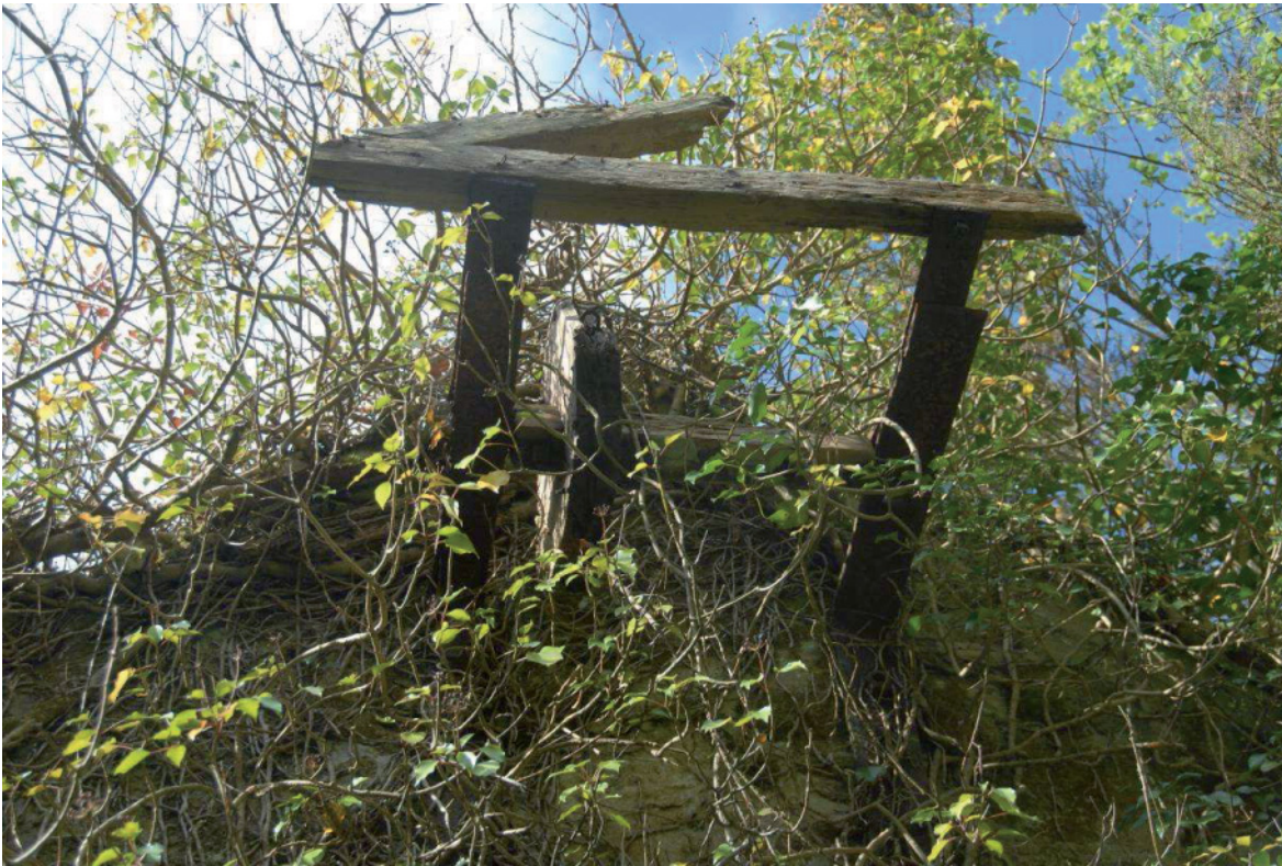
Fig 64. The remains of the timber canopy within which a bell was hung on the northern gable of Big Wheel Mill is typical of the detailing which could easily be lost if works are not undertaken. HE Digital Image Archive.
