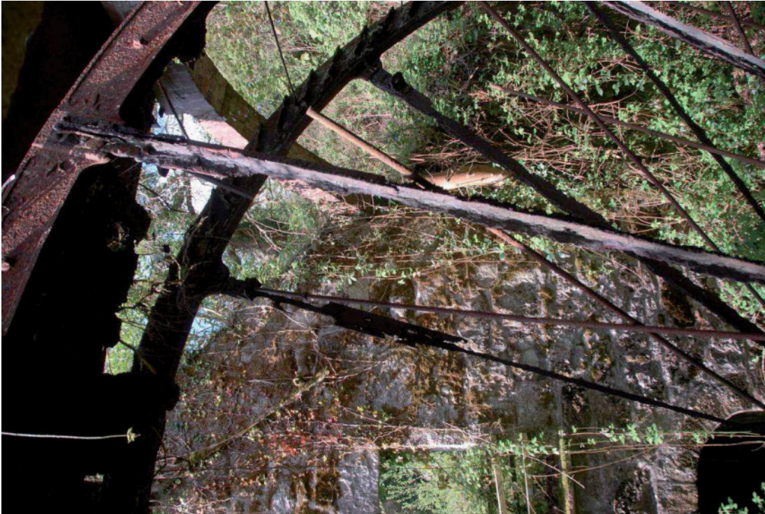
Fig 72. Another view of the very poor state of the water wheel spokes the Big Wheel Mill. HE Digital Image Archive.
