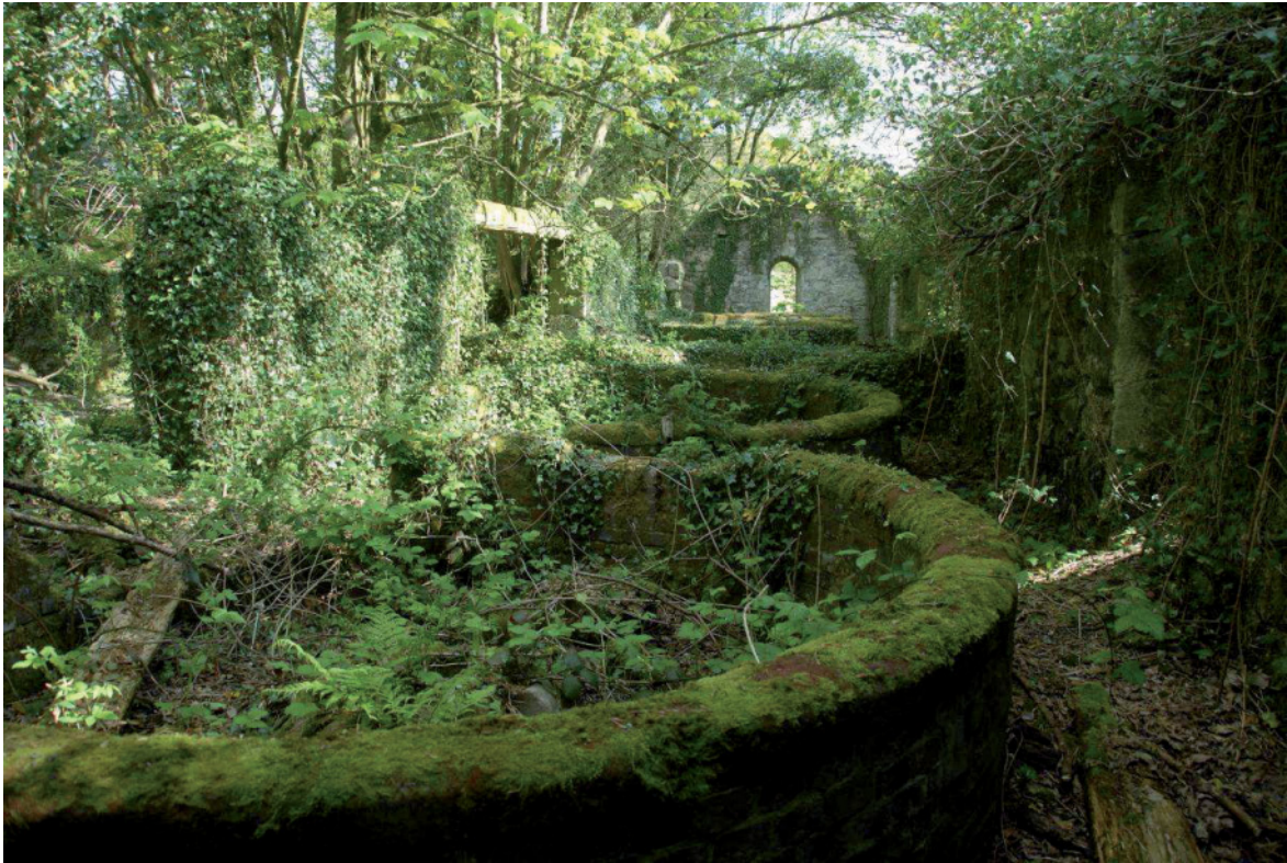
Fig 88. Looking north along the grinding floor in Mica Mill [39], showing the well-preserved brick-built grinding pans. HE Digital Image Archive.
