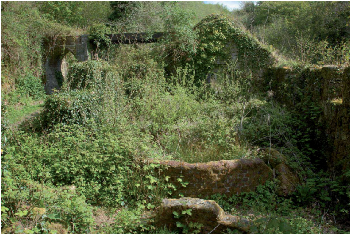
Fig 59. The remains of the brick-built grinding pans in the southern section of Big Wheel Mill [29]. HE Digital Image Archive.
