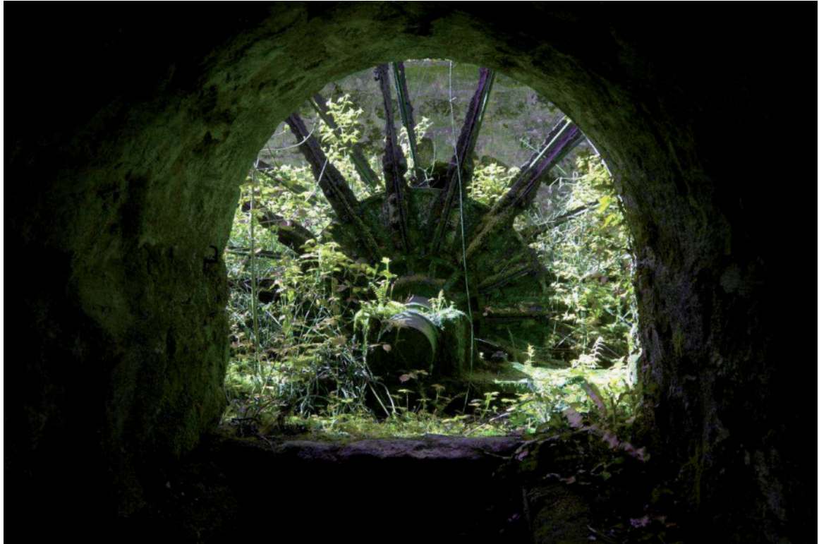
Fig 66. The hub of the Big Wheel Mill central water wheel, seen from the power vault running under the building. HE Digital Image Archive.
