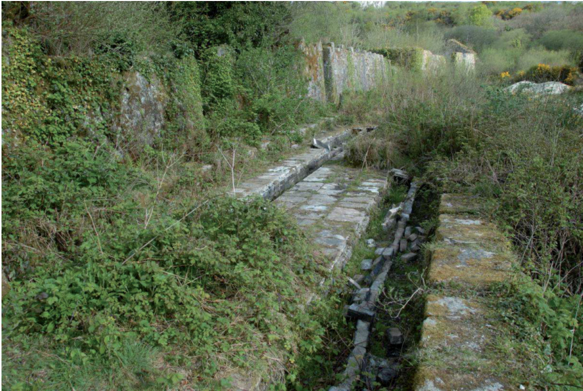
Fig 36. The interior of the Wheal Arthur pan kiln [11], showing the area from which the hypocaust tiles were recently removed. HE Digital Image Archive.
