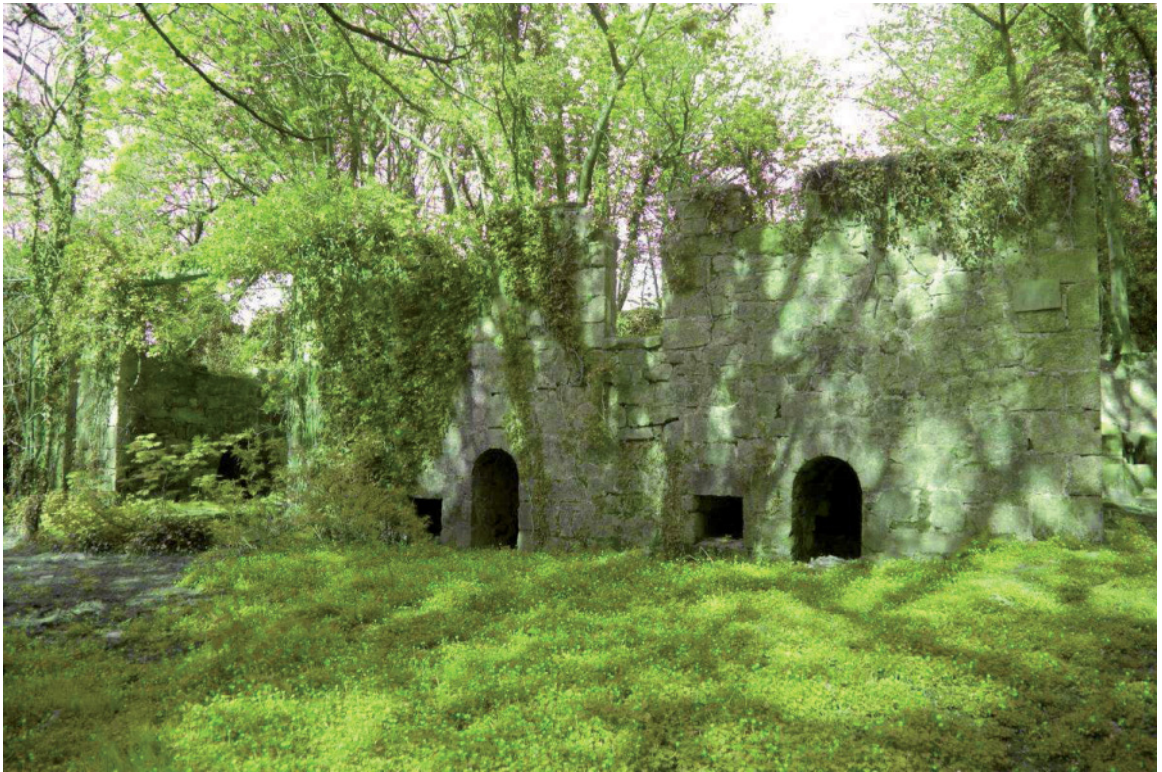
Fig 86. The northern section of Mica Mill [39] seen from the north-east. The massive central wheelpit can be seen to the left. HE Digital Image Archive.
