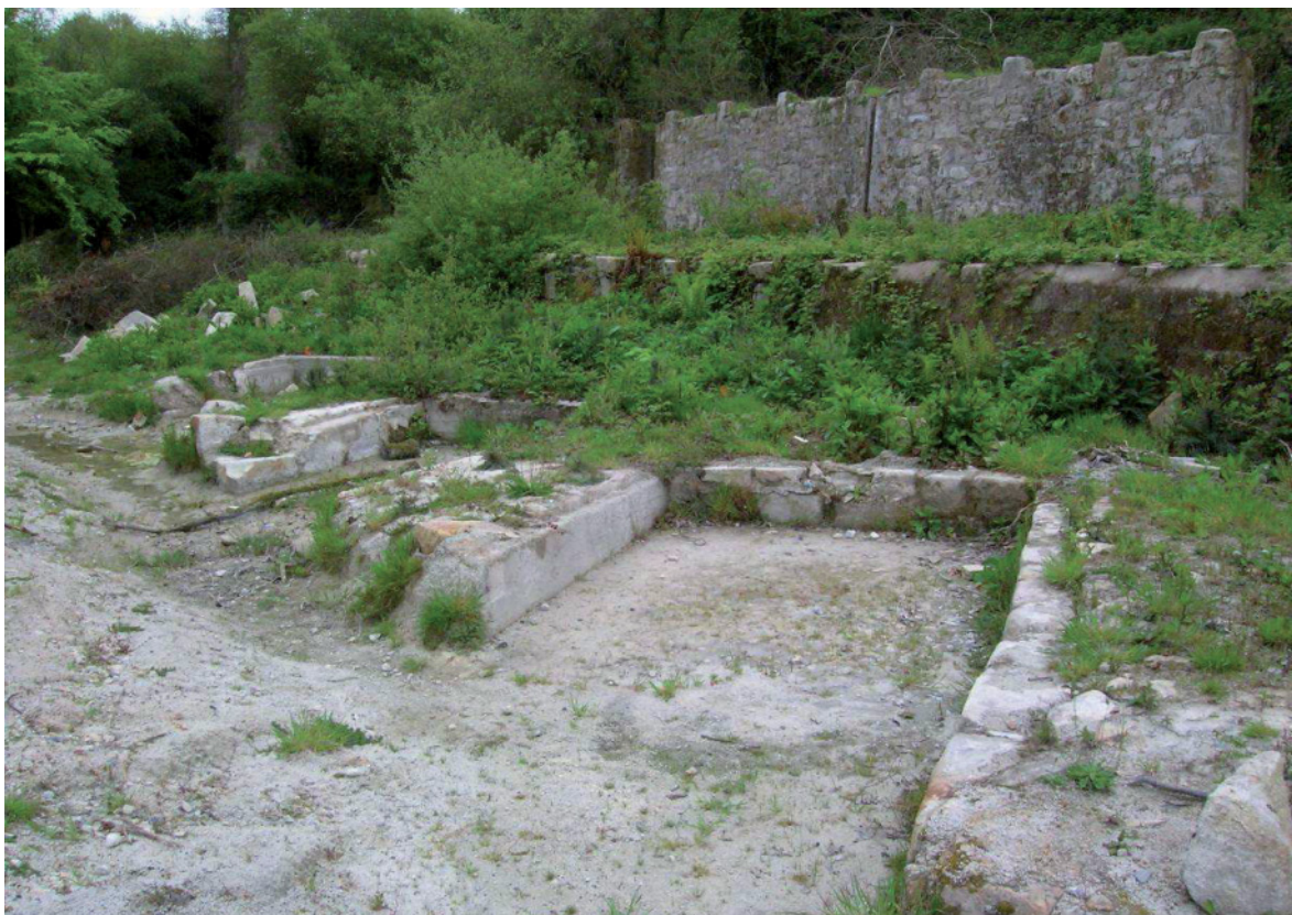
Fig 37. The linbay [12] to the east of the Wheal Arthur dry [11], showing one of the bays which has been cleared out by the Tregargus Trust. HE Digital Image Archive.
