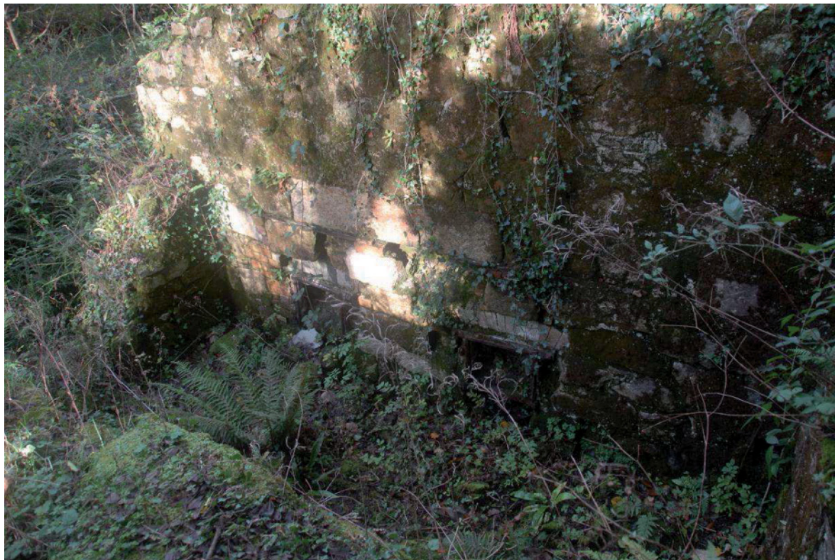
Fig 79. The southern end of the Trevear Mill dry, with its paired stoking doors. HE Digital Image Archive.
