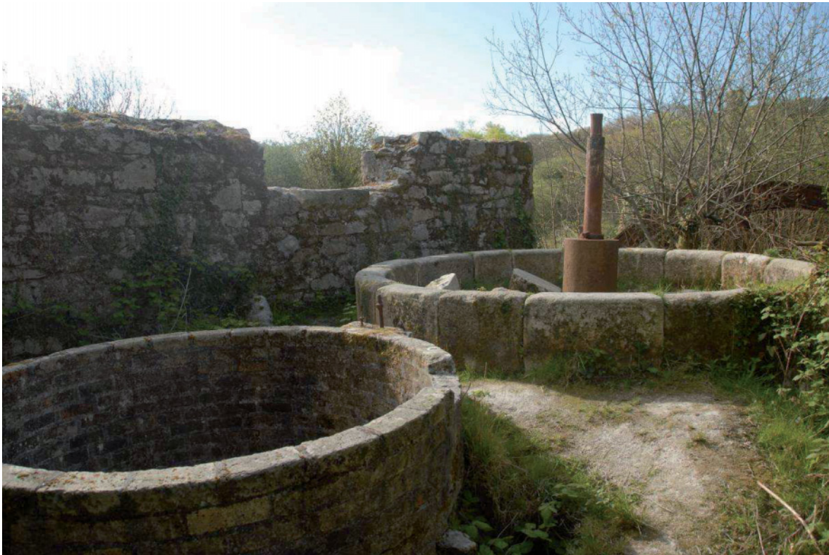
Fig 34. The brick-built grinding pans in the northern section of Wheal Arthur china stone mill [10]. The crown of the central waterwheel can be seen in the background. HE Digital Image Archive.
