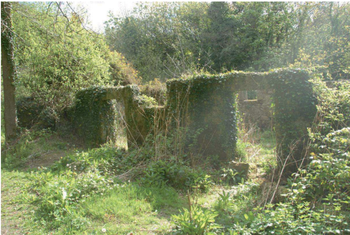
Fig 61. The northern section of the grinding floor of Big Wheel Mill [29] seen from the south-east. HE Digital Image Archive.
