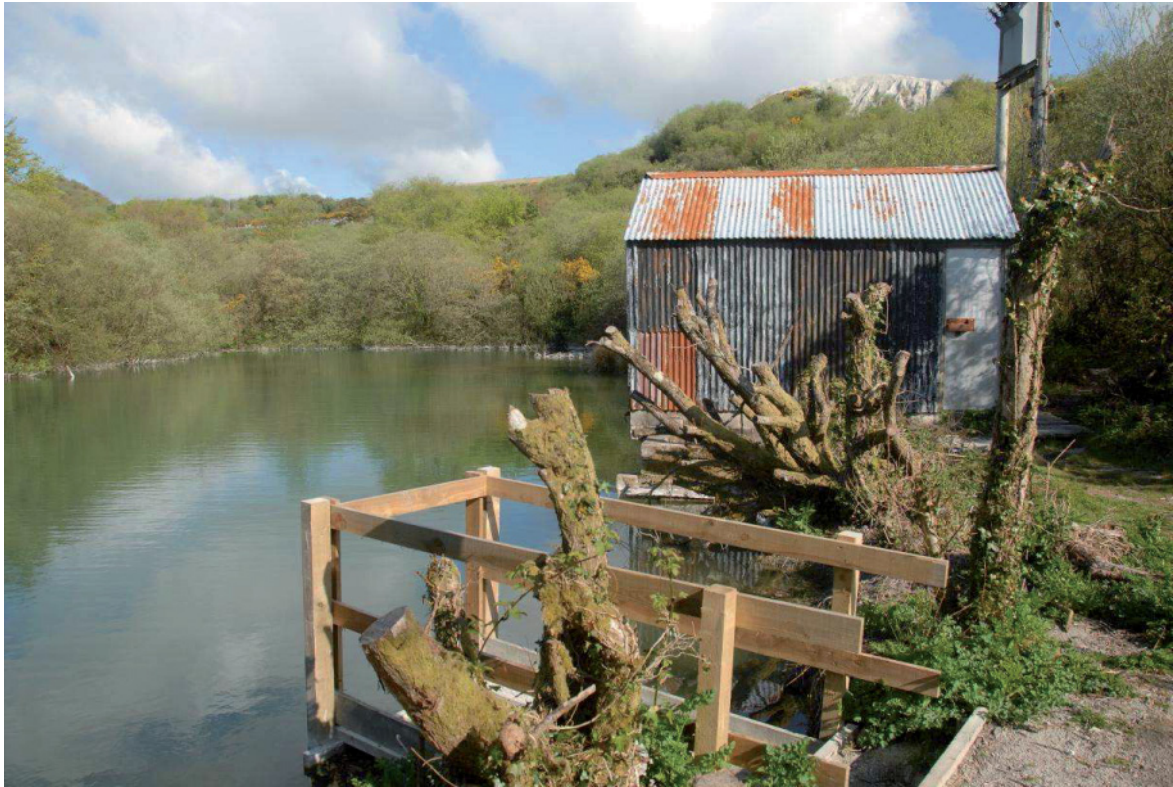
Fig 29. The pond and pump house just to the north of the Wheal Arthur complex. This site is just to the north of the area managed by the Tregargus Trust. HE Digital Image Archive.
