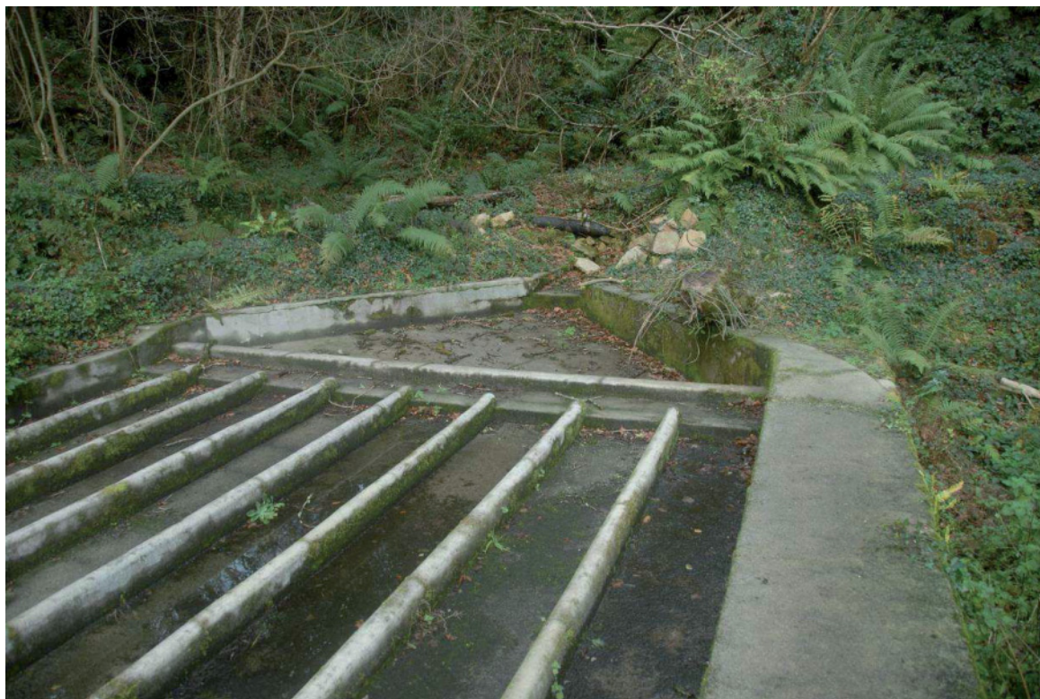
Fig 43. The northern end of the mica drags [19]. The entrance to its Adit [17] lies just beyond the clump of ferns. HE Digital Image Archive.
