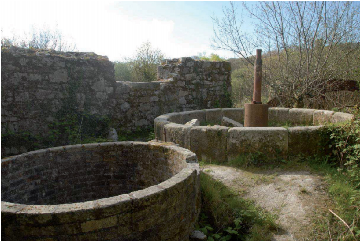
Fig 34. The brick-built grinding pans in the northern section of Wheal Arthur china stone mill [10]. The crown of the central waterwheel can be seen in the background. HE Digital Image Archive.
