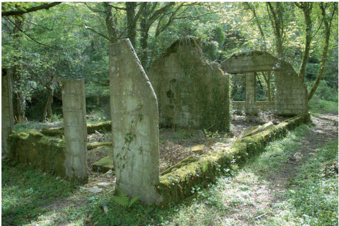
Fig 47. The remains of the blockwork-built crib hut [31] to the east of Big Wheel Mill. HE Digital Image Archive.
