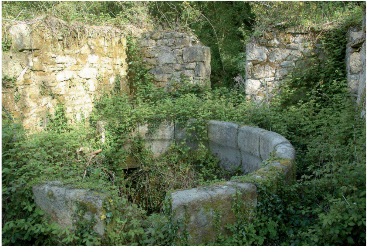
Fig 78. A stone-constructed grinding pan at Trevear Mill, showing the characteristic wear on its inner face. HE Digital Image Archive.
