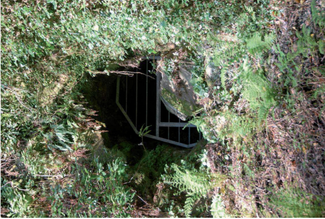
Fig 28. One of the bat-friendly galvanised steel grilles [3] fitted in the adits in Wheal Arthur Quarry [1]. The quarry is outside the area managed by the Tregargus Trust. HE Digital Image Archive.
