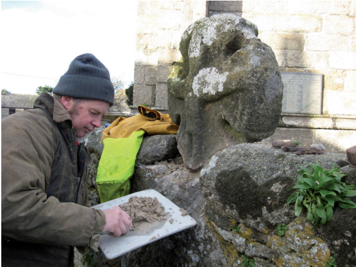
Fig 13 Repointing with lime mortar
