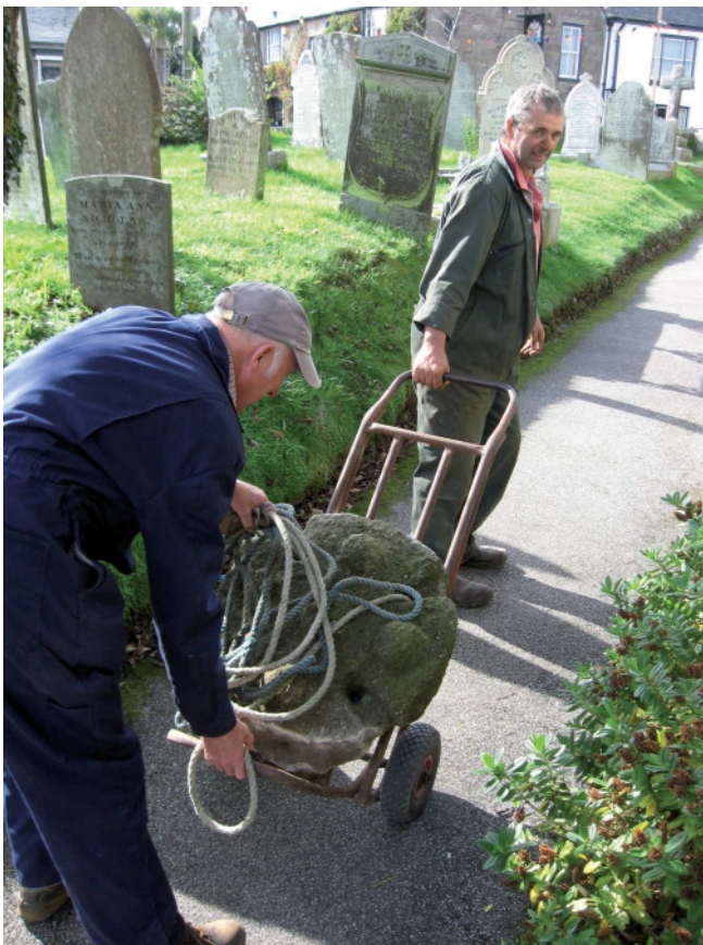
Fig 23 Removing the cross-head from the church prior to final restoration
