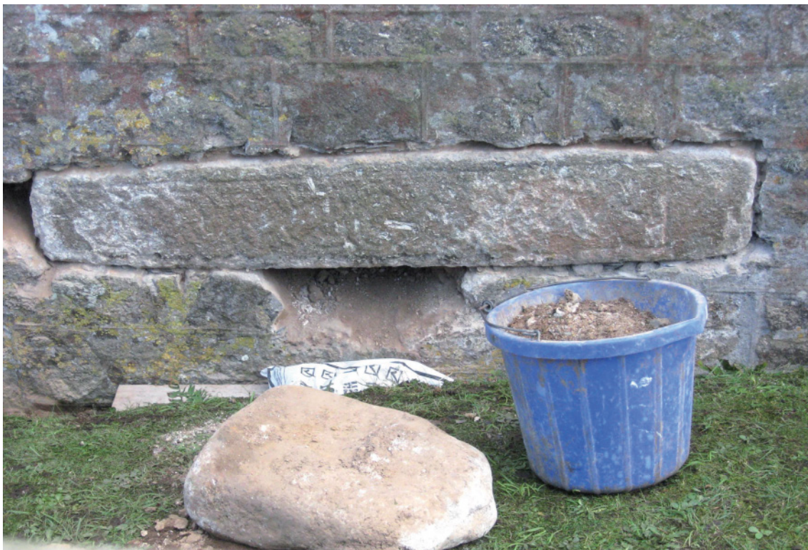
Fig 17 The shaft fully exposed
