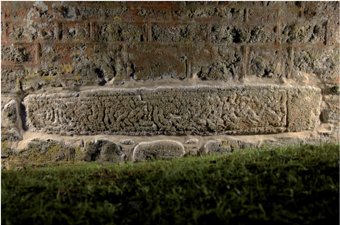
Fig 18 The shaft after re-pointing
