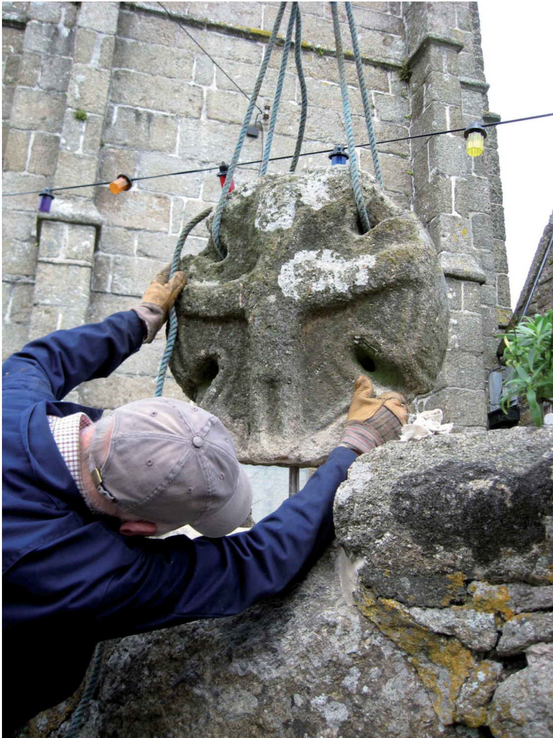
Fig 24 Replacing the cross-head
