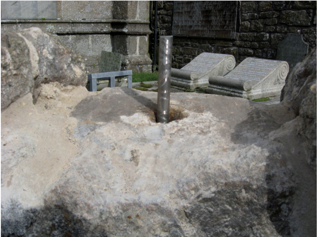
Fig 22 The new stainless steel pin in position in the boulder-base
