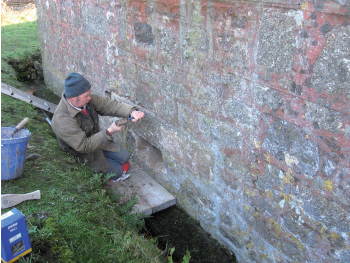
Fig 16 The mortar being removed from around the cross-shaft
