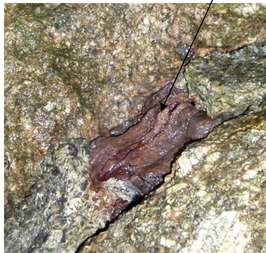
Fig 10 Detail of the ironwork visible in the mortar around the cross-head
