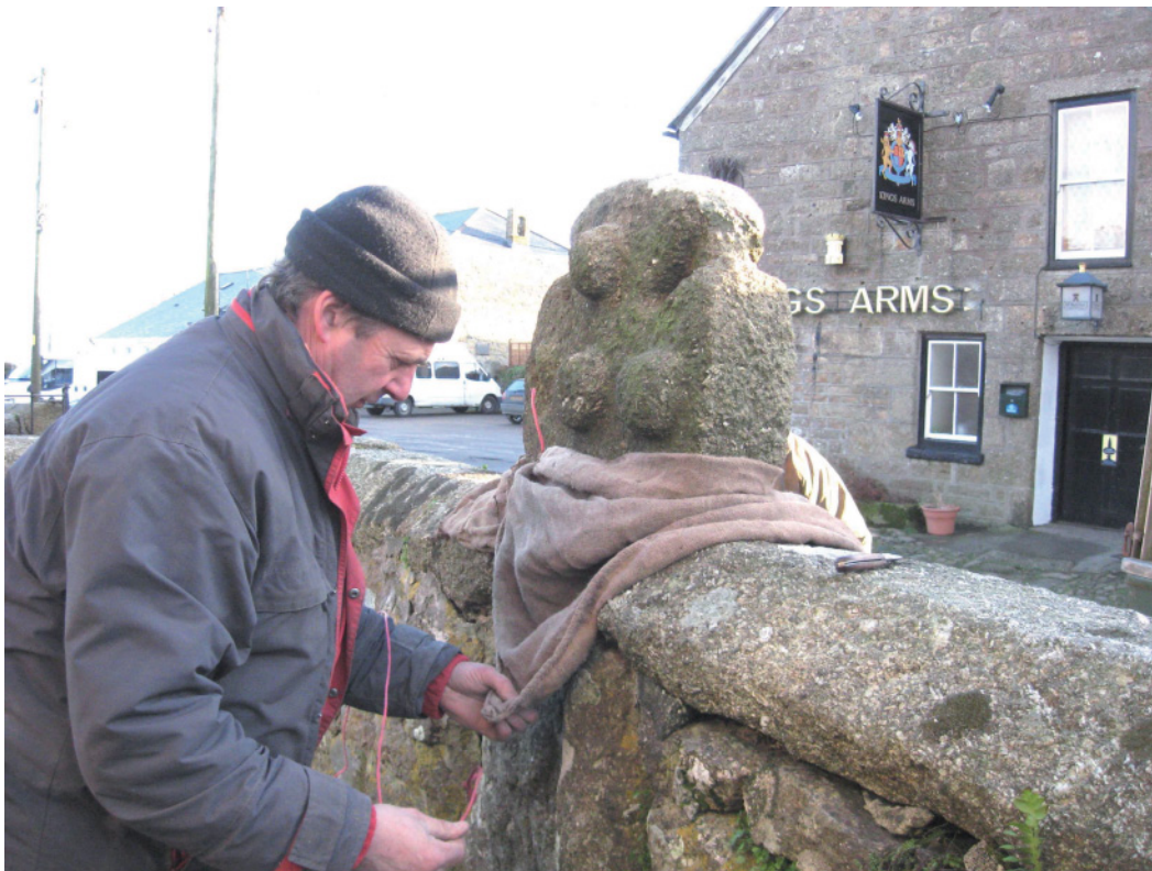
Fig 14 Mortar being protected with hessian
