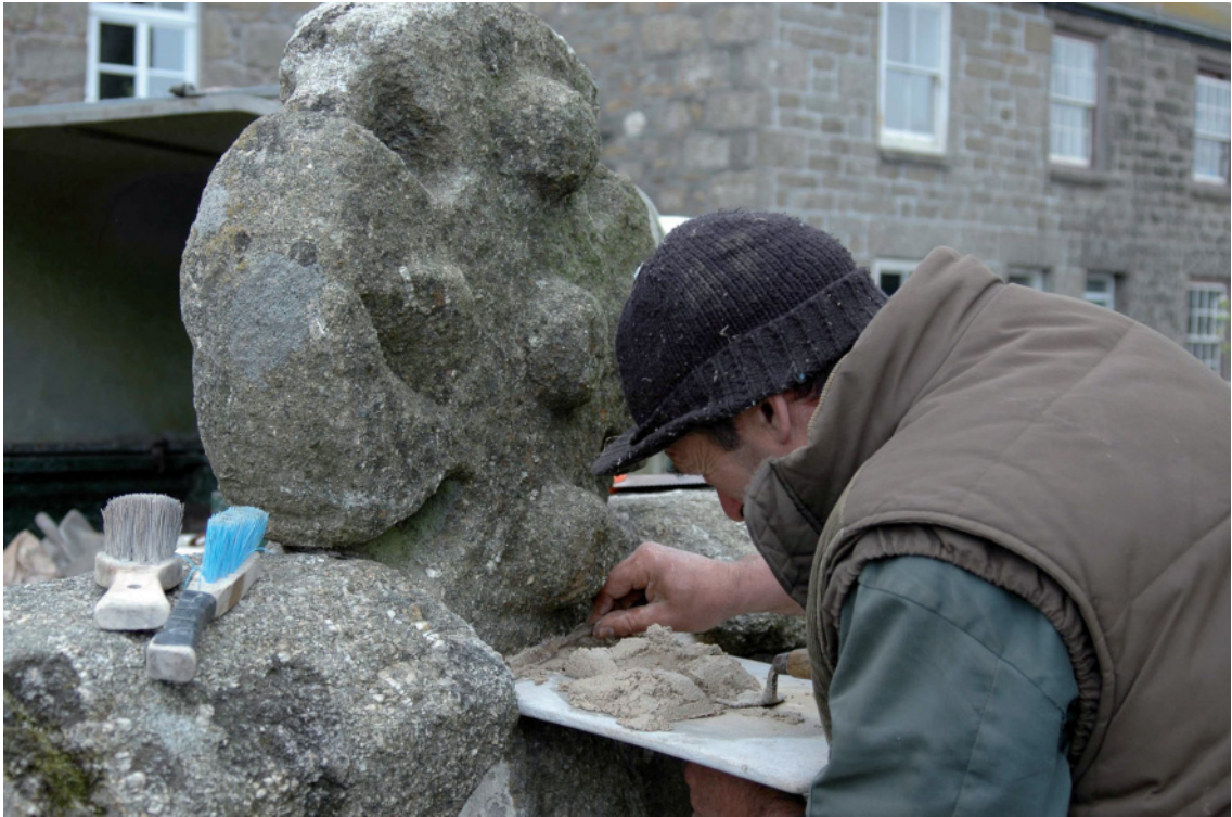
Fig 25 Final repointing of the joint between the head and the boulder
