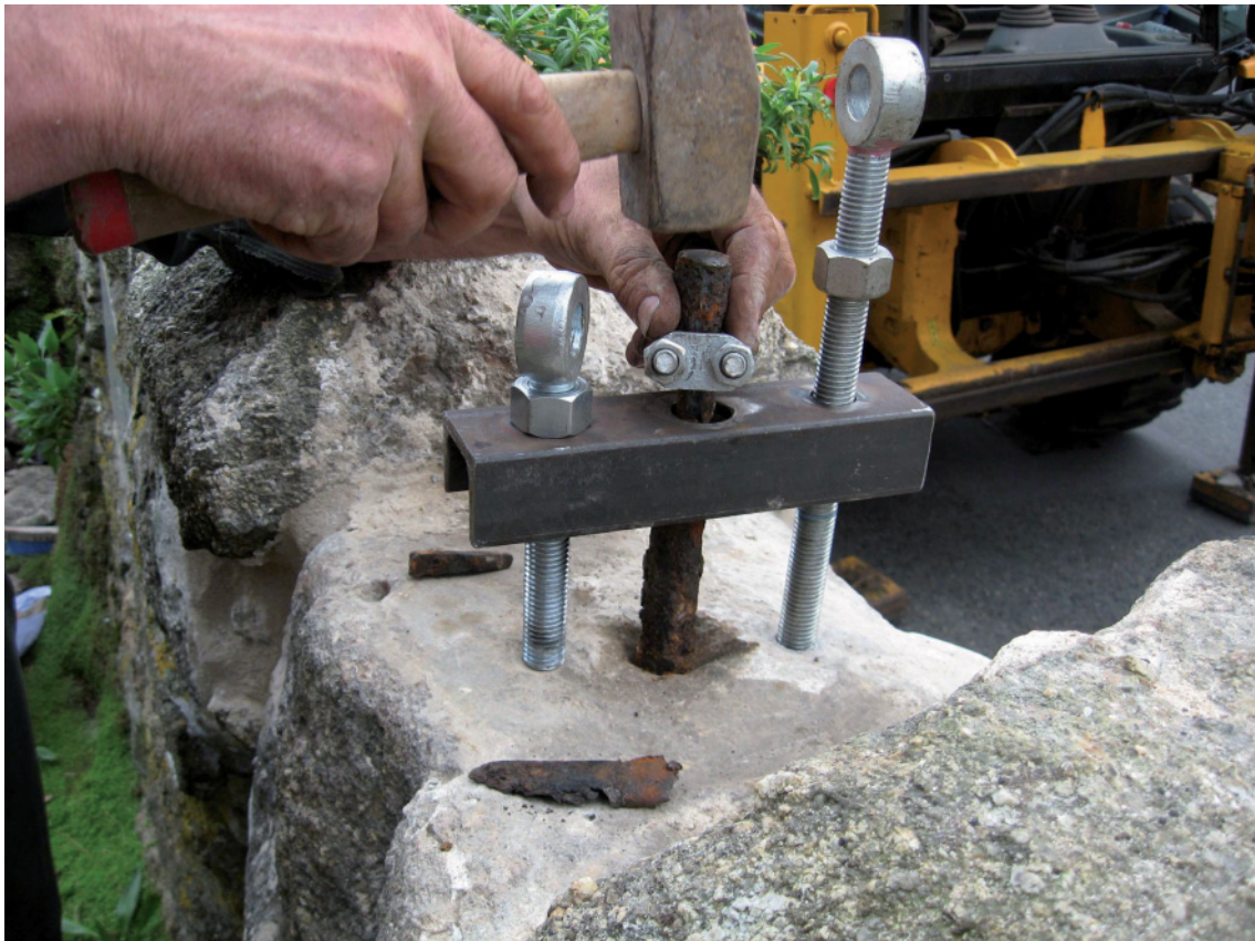
Fig 21 Removing the pin with a specially-designed puller
