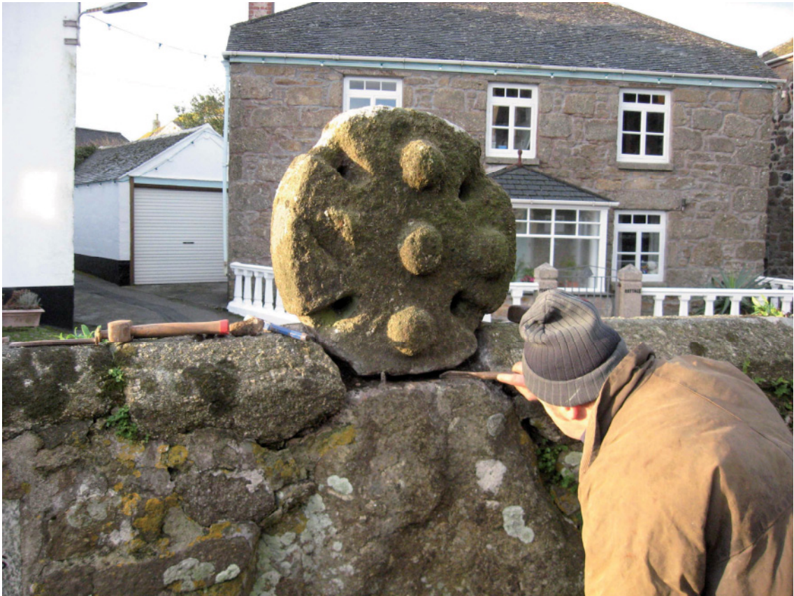
Fig 11 Removing cement pointing from around the cross-head
