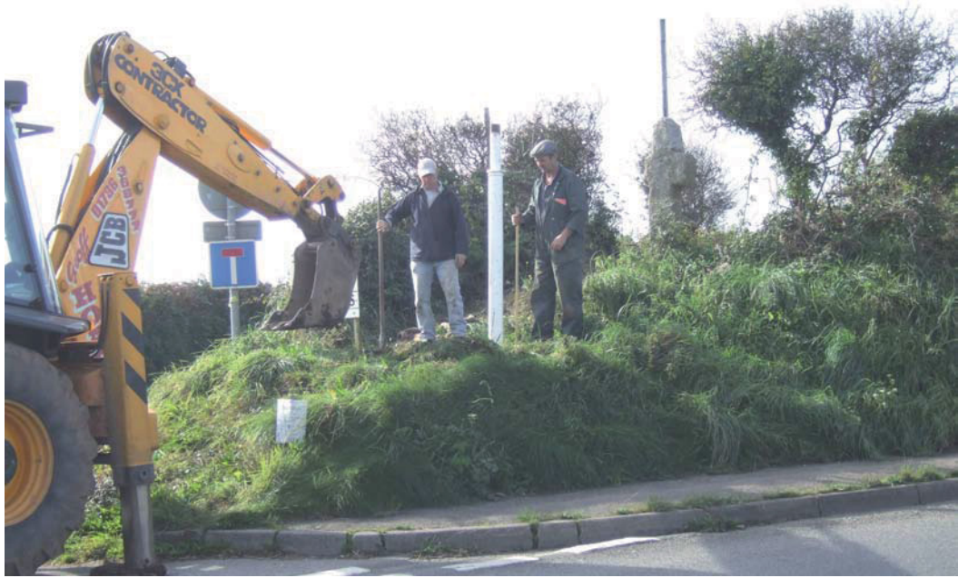
Fig 25 The finger post is restored (note the restored cross behind it)
