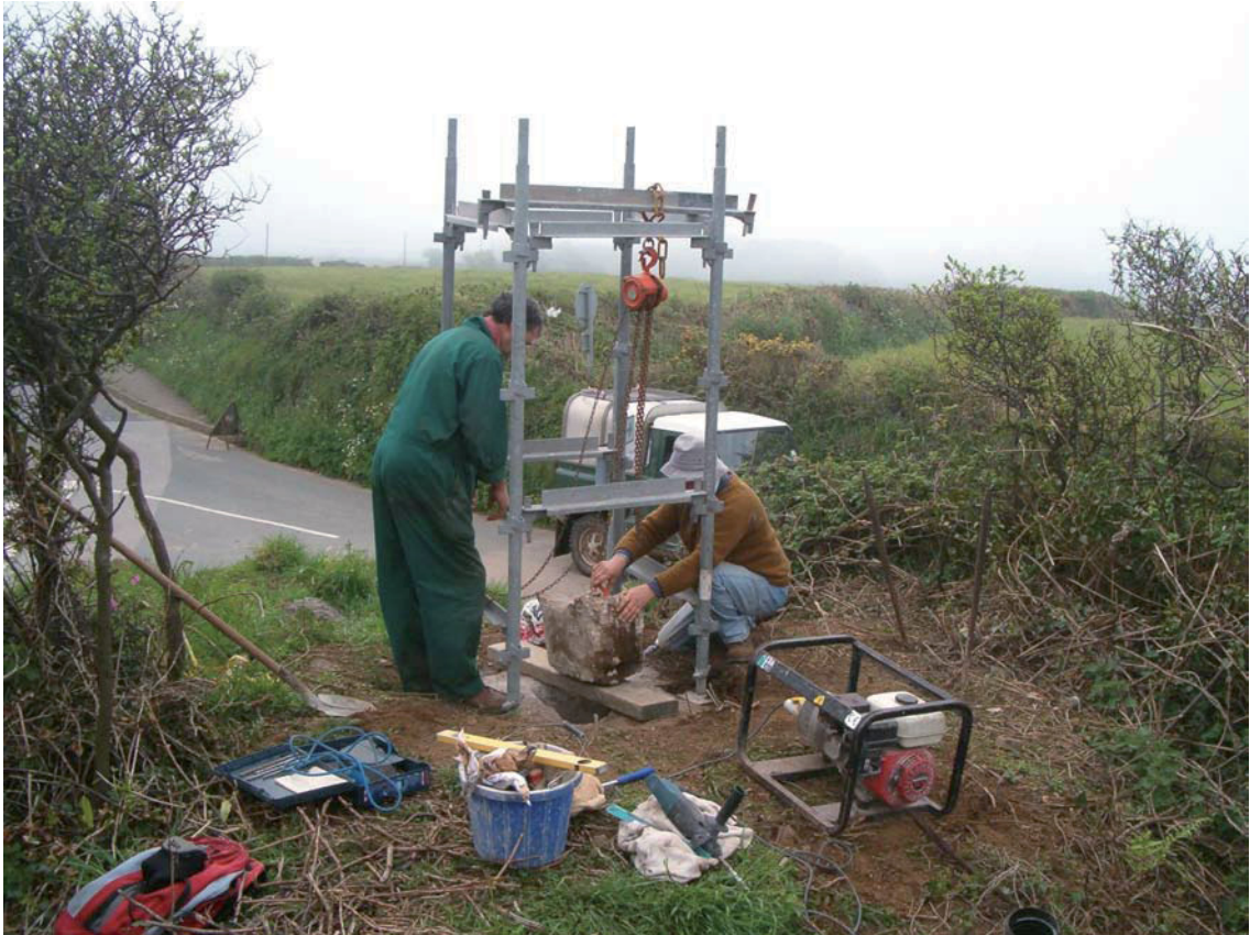
Fig 14 Removing the bottom of the cross-shaft from the base
