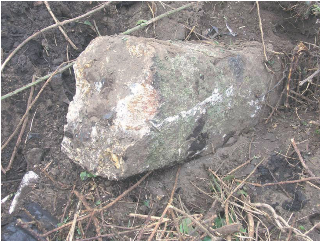
Fig 11 The damaged cross: the shaft lodged in the rubble ploughed up by the lorry
