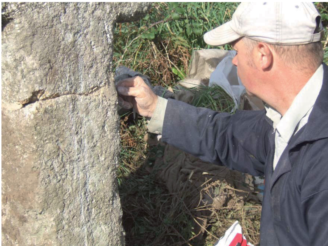
Fig 23 Pointing the joint in the shaft with lime mortar
