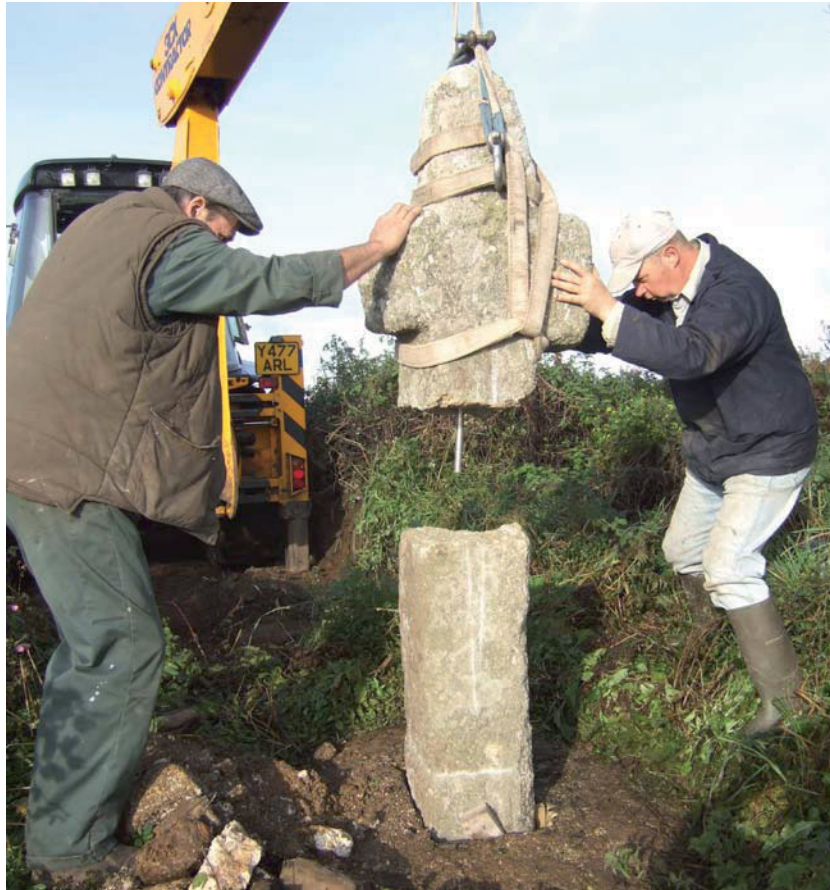
Fig 22 Restoring the cross: the cross-head is lifted back
