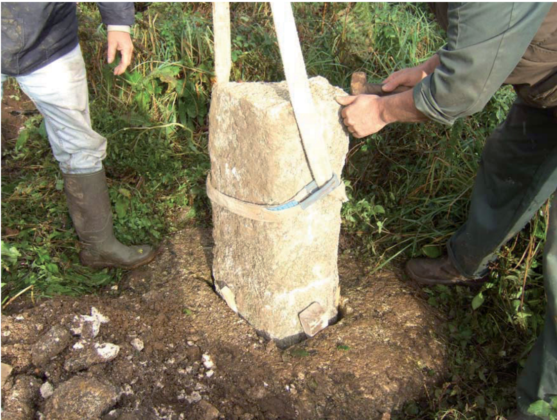
Fig 21 Restoring the cross on site: the shaft is put in position
