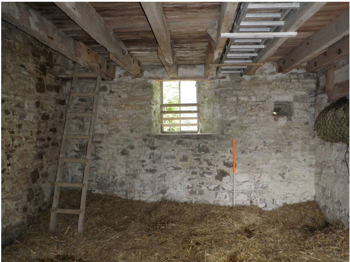
Fig 14: Rear wall inside stable showing a partially blocked original window opening and an opening for a drive shaft to the north of it
