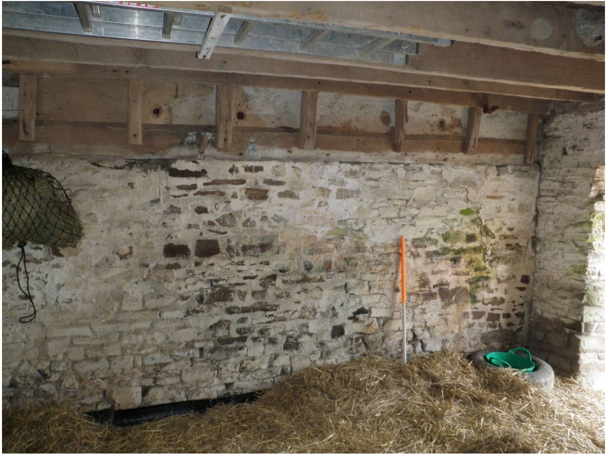
Fig 13: Partition wall inside the stable showing ground floor stone rubble wall with remains of timber stud wall extending up to the first floor
