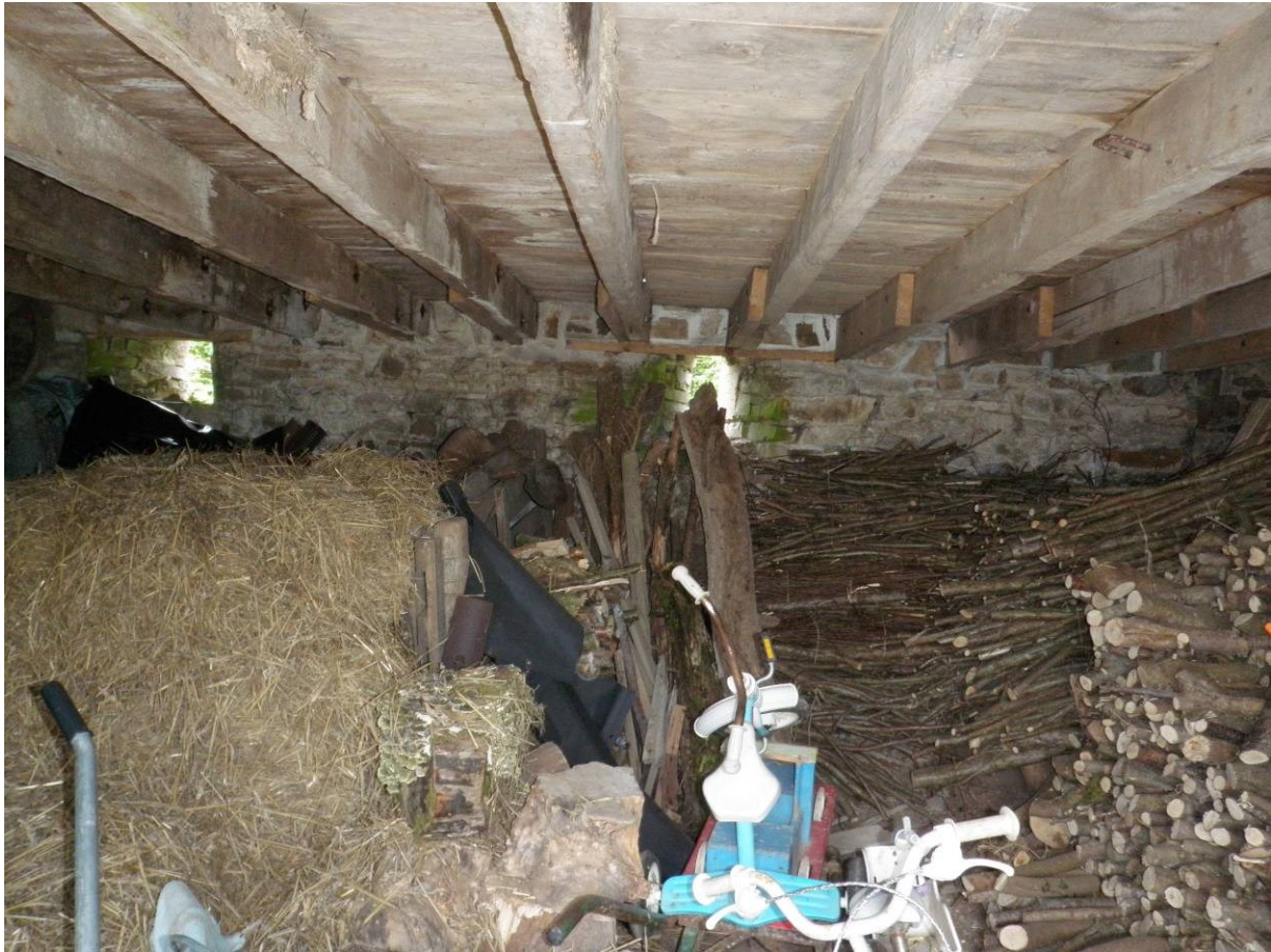
Fig 15: Rear wall inside cow-house showing two internally splayed ventilators and threshing floor above
