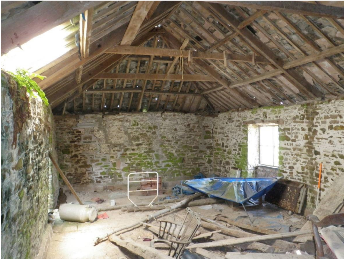
Fig 17: First floor interior looking north into former threshing barn showing the location of a former stud wall as a shadow on the east wall and the remains of studs attached to the truss
