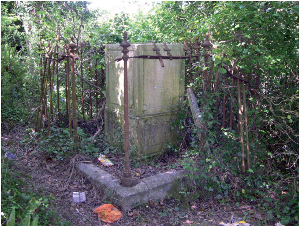
Fig 10 Ornate tomb of the Poat family, in the south west corner of the Congregationalist ground, damaged by woody growth and by vandalism; the top slab of the central structure has been recently displaced (right)
