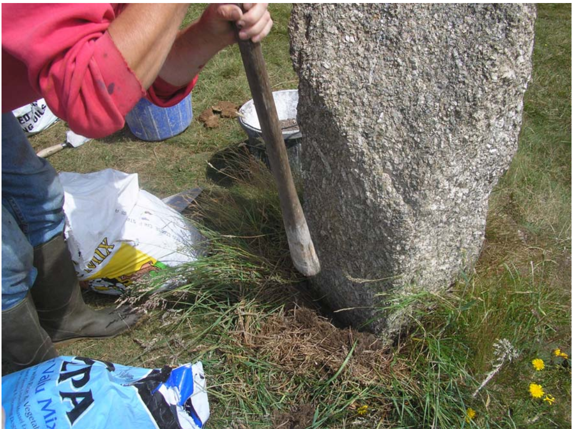
Fig 10 Stabilising the stones by tamping rab into the cracks between the stones and the ground
