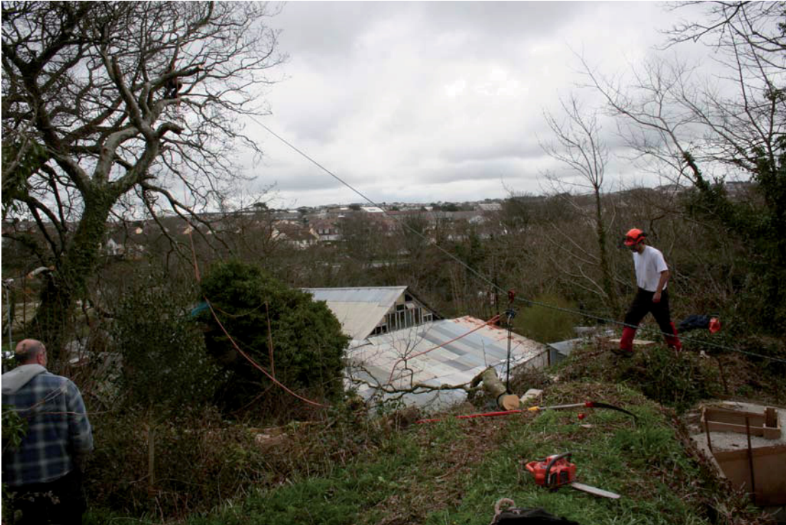
Fig 3: Initially branches were lowered carefully towards the mill pond
