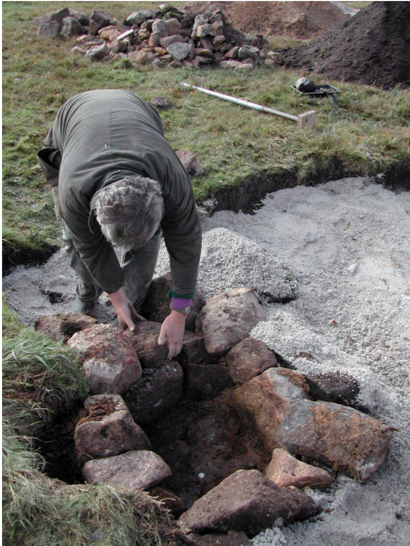
Fig 10. Construction of the new stone-lined socket for recumbent stone 19.
