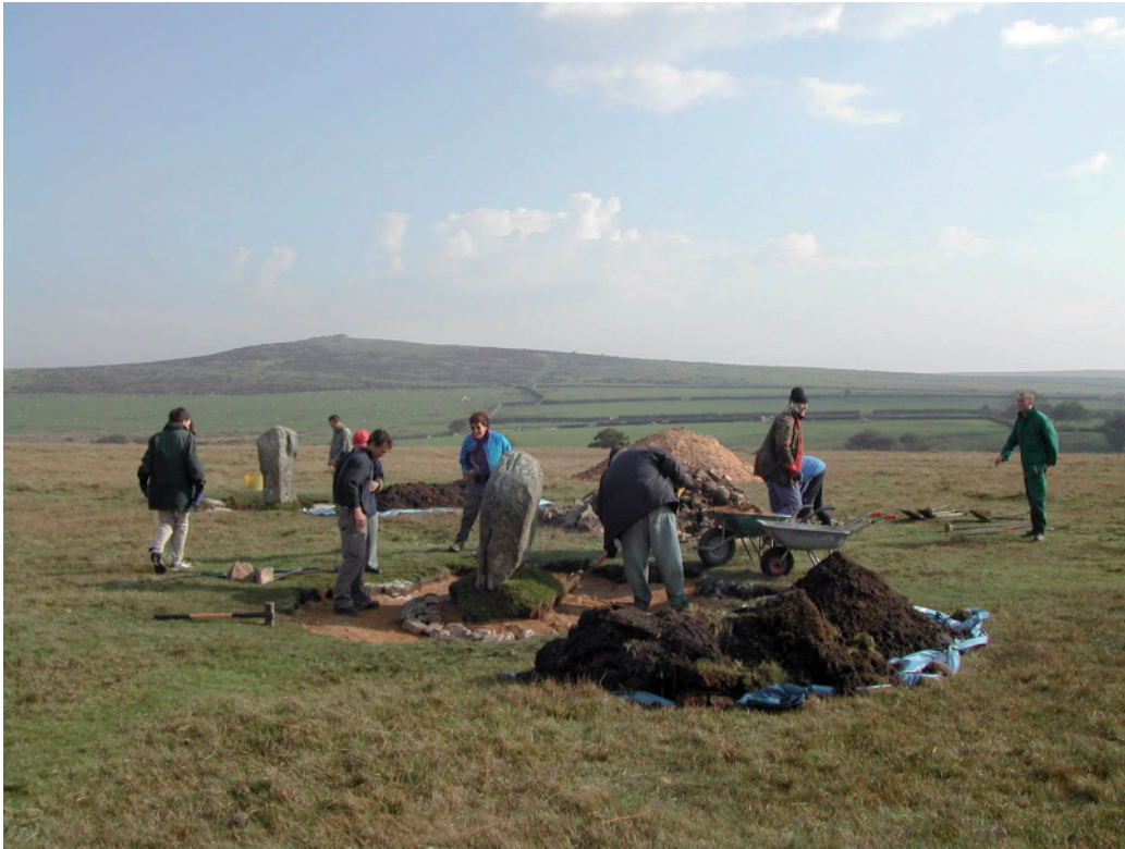
Fig 4. The Trippet Stones Stone Circle, repairs underway.
