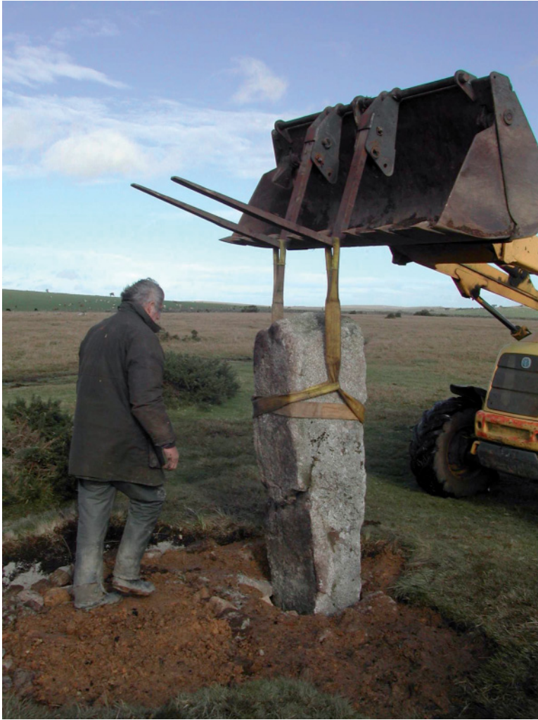
Fig 11. Re-erection of recumbent stone 19
