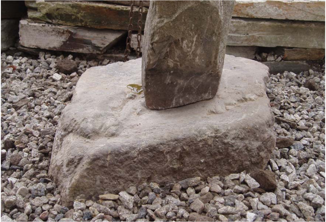
Fig 14 Detail of the sloping joint between cross and its base
