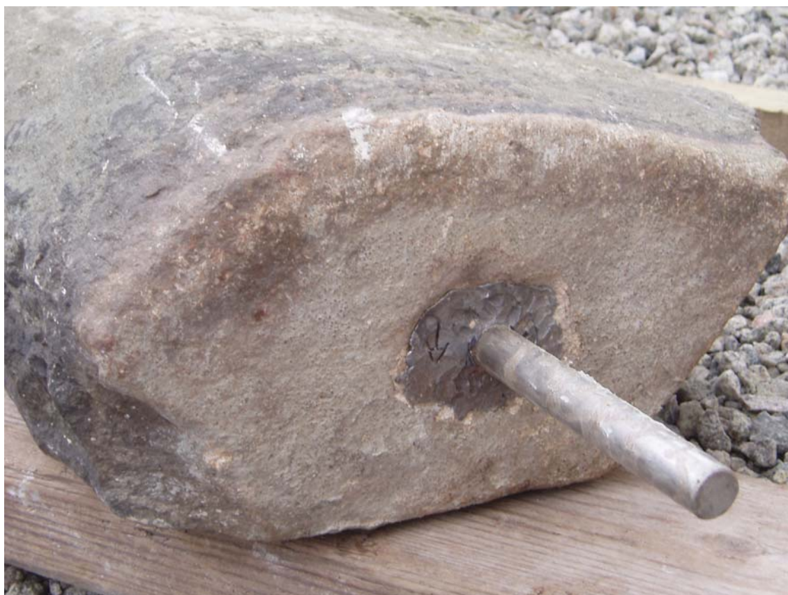
Fig 12 The new pin, leaded into place
