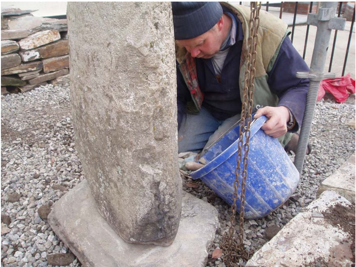
Fig 15 Mortaring the joint at the base of the cross
