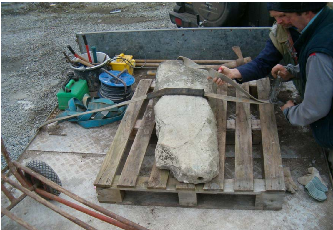
Fig 10 Lifting the cross for removal to St Just for drilling and pinning
