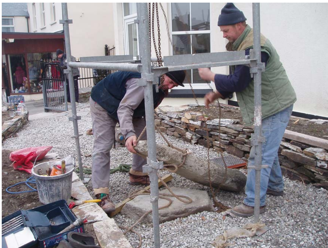
Fig 13 Lifting the cross back into position
