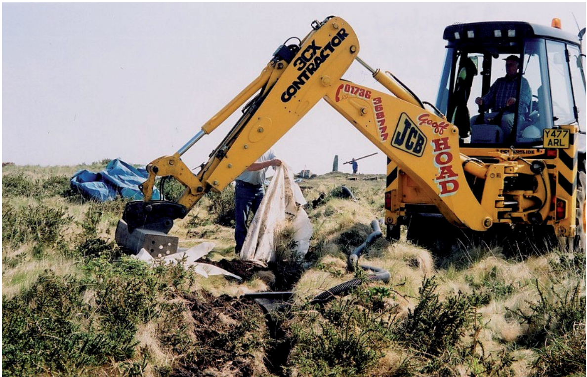
Fig 27 Drainage work underway at the Nine Maidens in May 2004
