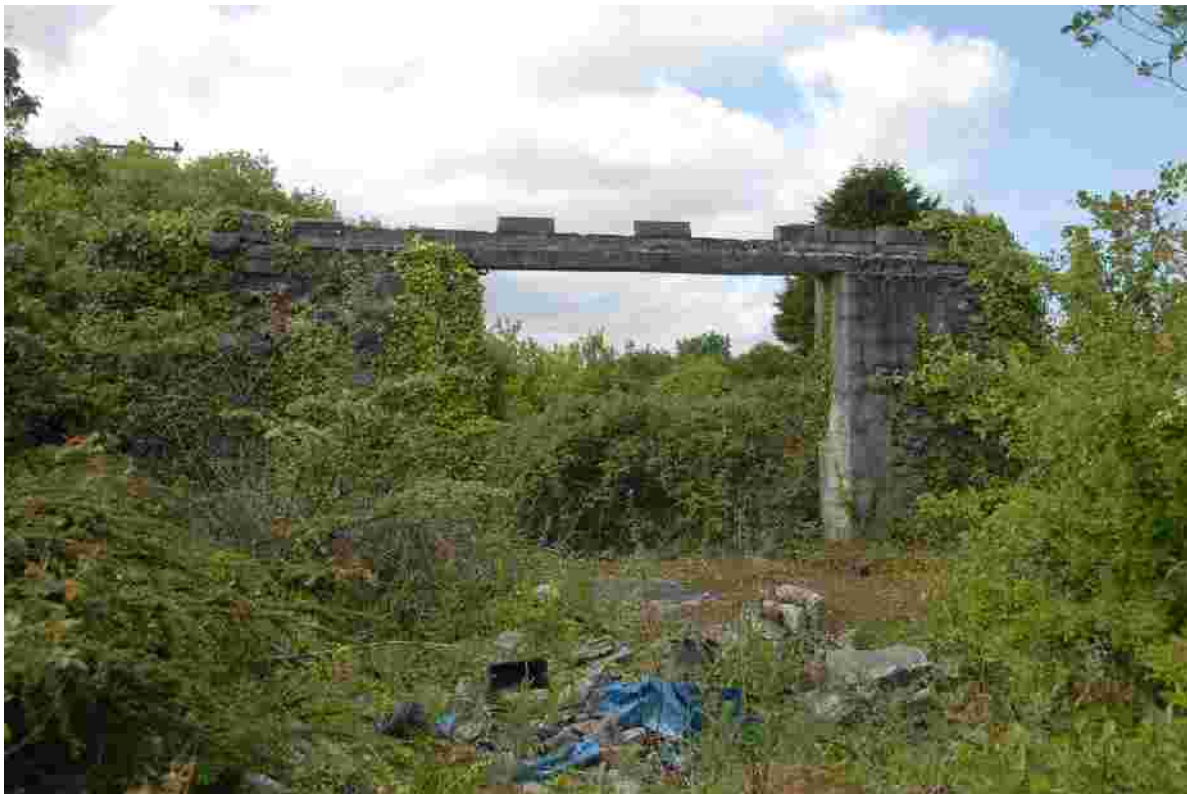
Fig 48. All that remains of the L-shaped mid-19 th century mine building [41] at the southern end of the Hallenbeagle site.
