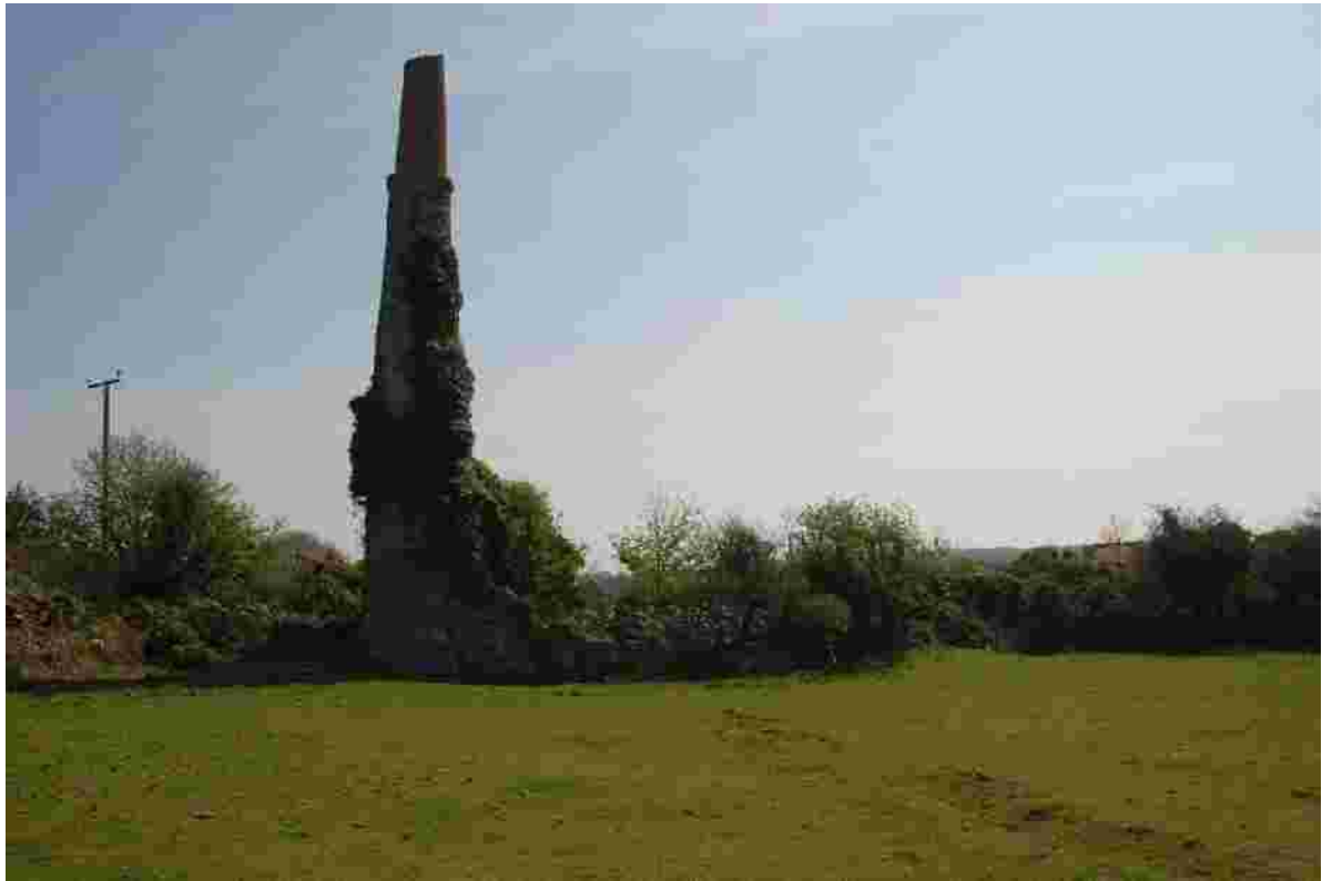
Fig 35. Reade's whim engine house [16] seen from the east. The forward part of this Listed Building, together with its boiler house and loadings have been demolished. A shallow trench runs across the nearby field to this building.
