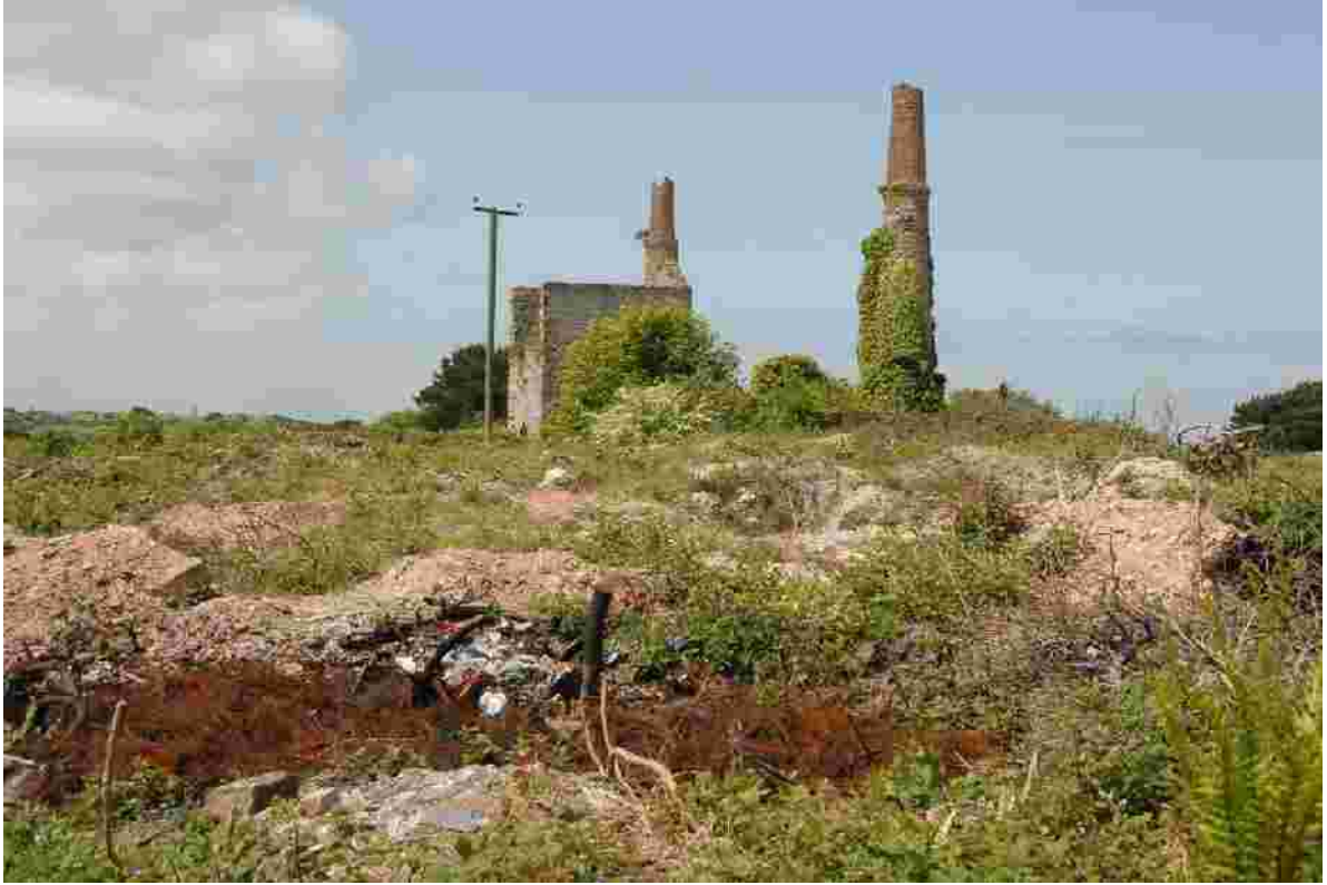
Fig 29. Looking towards the buildings at Reade's Shaft from the edge of the spoil dump associated with Jeffrey's [18] and Oat's [19] Shafts.
