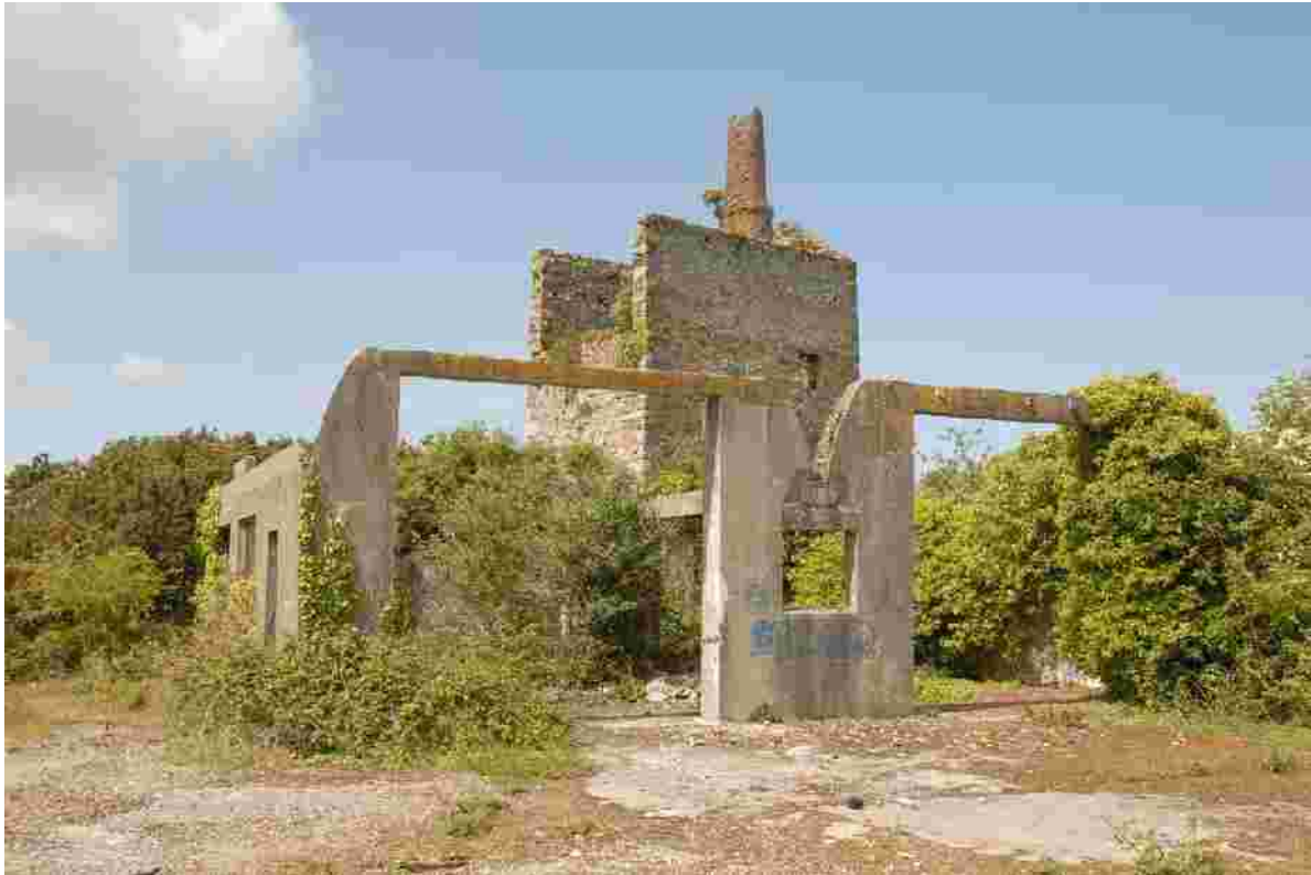
Fig 37. The concrete plant vehicle maintenance building [28] adjacent to Reade's Shaft.
