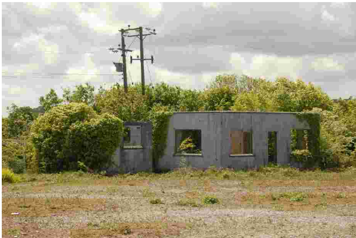
Fig 36. Two of the abandoned concrete plant buildings [30/31] to the south of Reade's Shaft.
