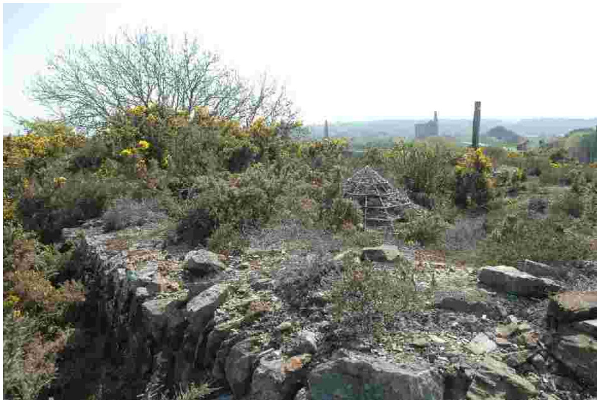
Fig 24. The Clwyd Cap on Whim Engine Shaft [5] on the top of the spoil dump on the western part of the site at its northern end.
