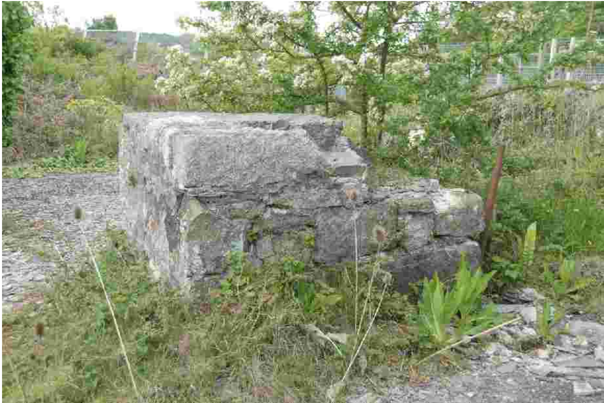
Fig 47. A substantial masonry plinth at the western end of the central sawmill building [40]. A large threaded metal fixing protrudes from the ground adjacent to this.
