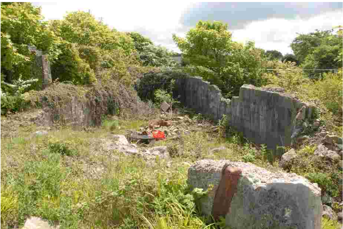
Fig 38. The masonry and concrete tank [38] in the south-eastern part of the site, almost certainly constructed as part of the sawmill complex.
