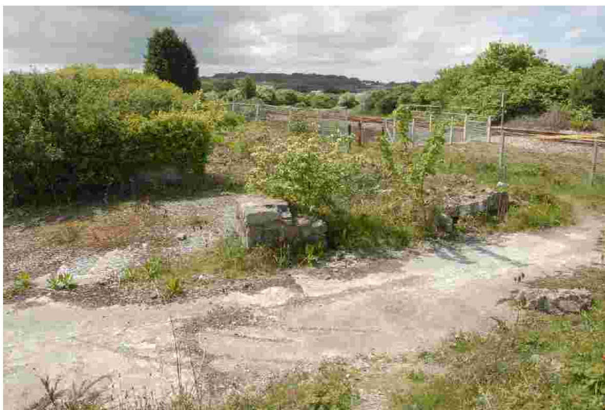
Fig 46. A view of the southern side of the western end of the elongated sawmill building [40]. Only foundations now remain of this building.
