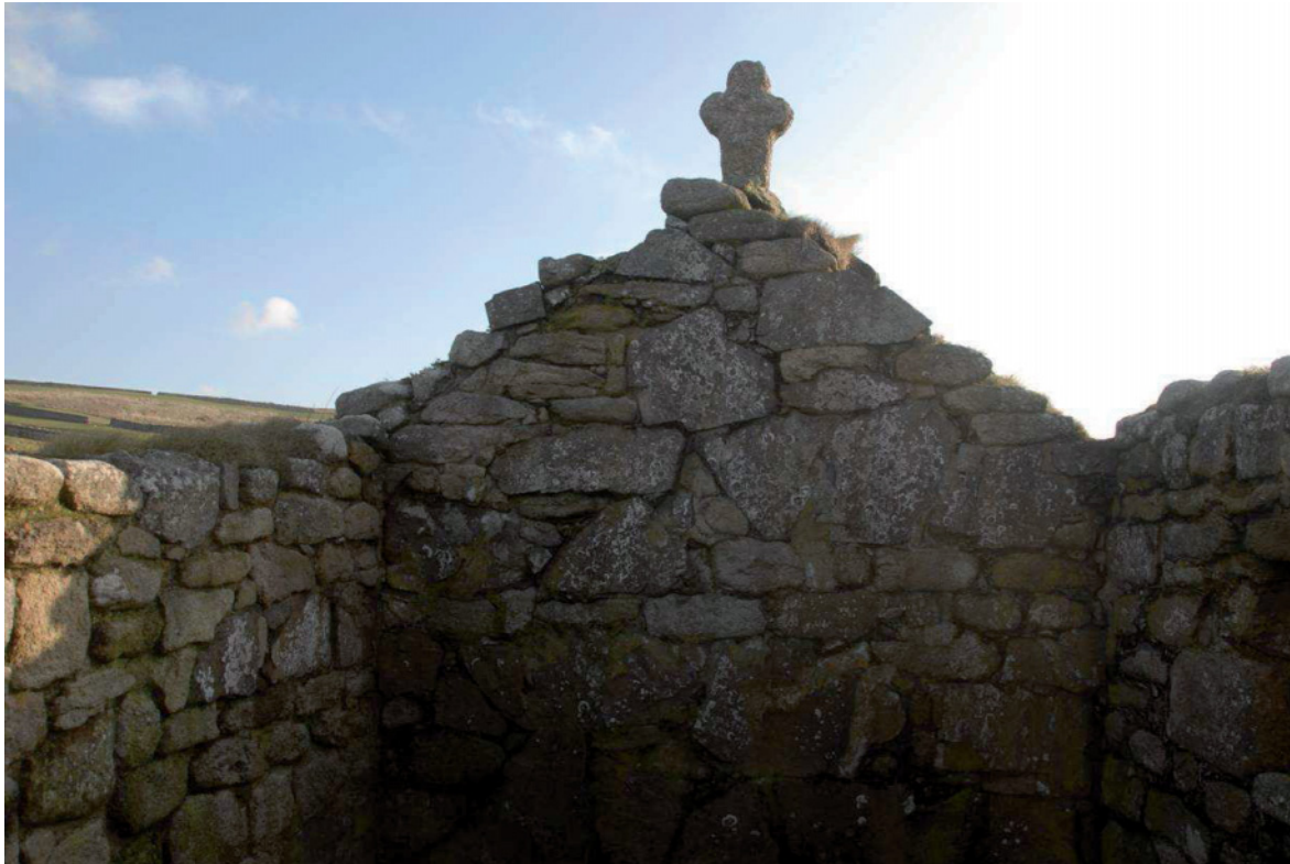
Fig 26. The internal elevation of the southern wall of St. Helen's Chapel in late 2009. HE Digital Image Archive.
