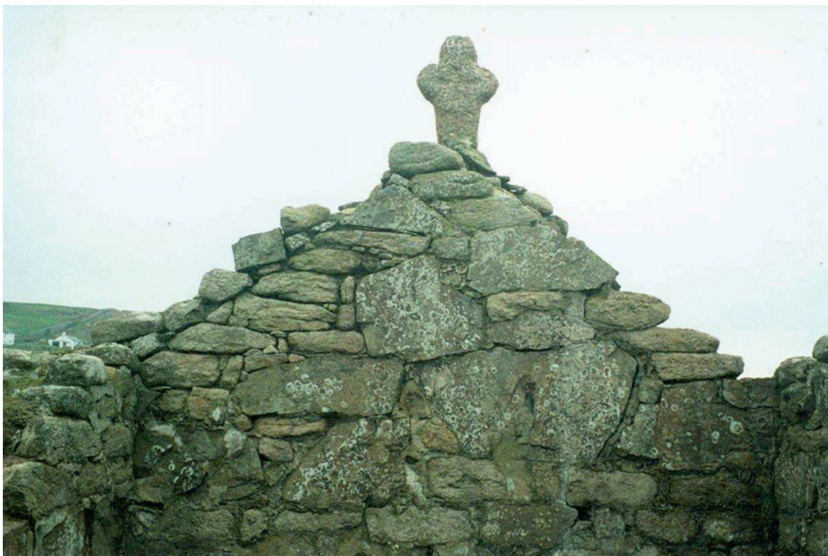
Fig 15. The internal elevation of the southern wall of St. Helen's Chapel before works, showing some evidence for the original gable line having been raised in smaller stone (left). HE Digital Image Archive.
