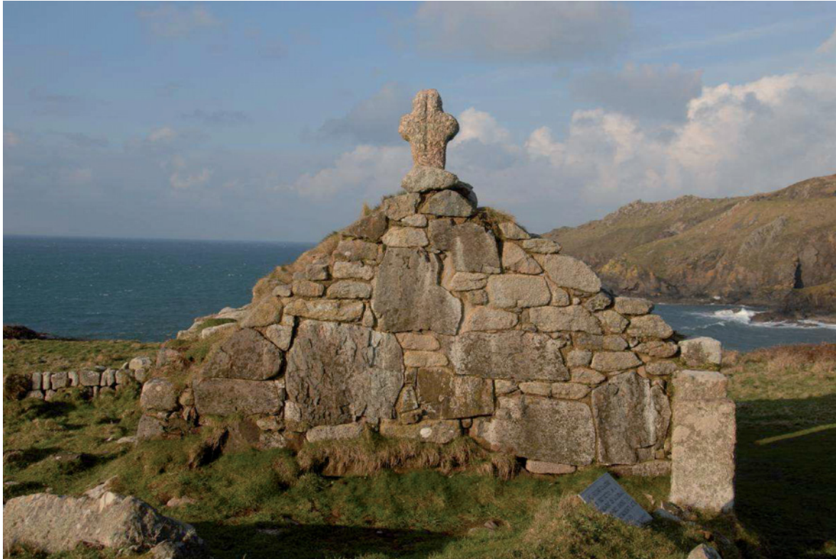
Fig 23. The southern elevation of St. Helen's Chapel in late 2009. HE Digital Image Archive.
