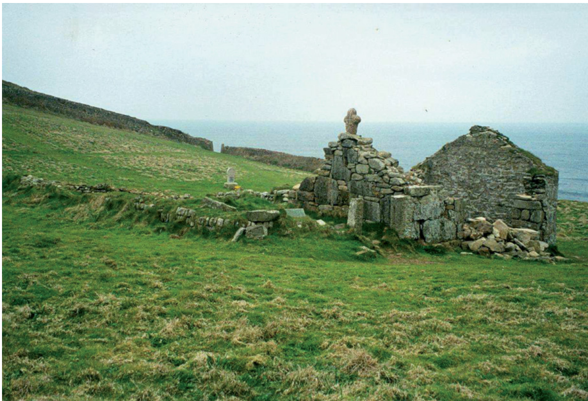
Fig 11. St. Helen's Chapel from the south-east prior to works, showing the collapsed masonry adjacent to the doorway, and the low walls forming the enclosures to the west. HE Digital Image Archive.
