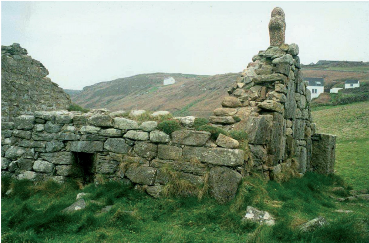
Fig 12. St. Helen's Chapel from the west-south-west before works, showing the window, the smaller size of masonry used in this wall and the deterioration of the southern wall head. HE Digital Image Archive.
