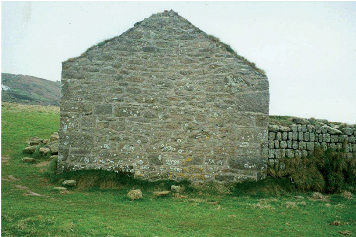
Fig 14. St. Helen's Chapel from the north before works, showing the markedly different style of stonework used in the construction of this wall. HE Digital Image Archive.
