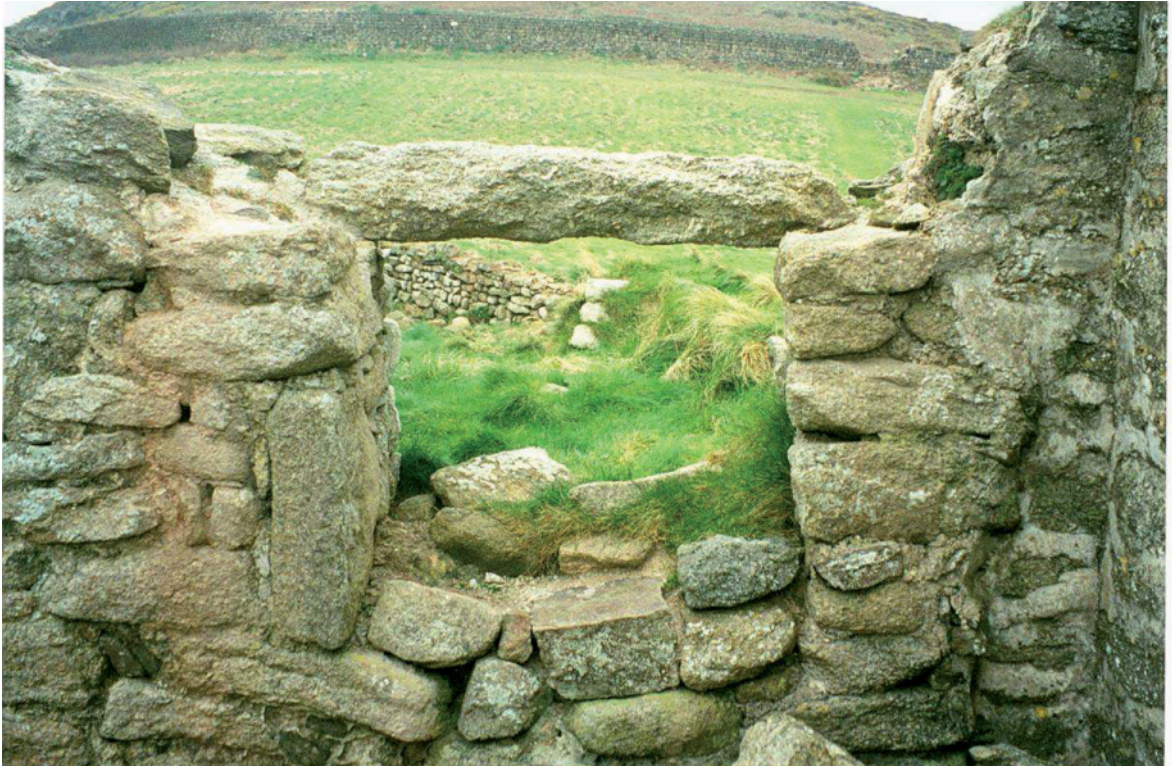
Fig 16. The small window in the eastern wall of St. Helen's Chapel before works, showing the lost inner lintel. HE Digital Image Archive.
