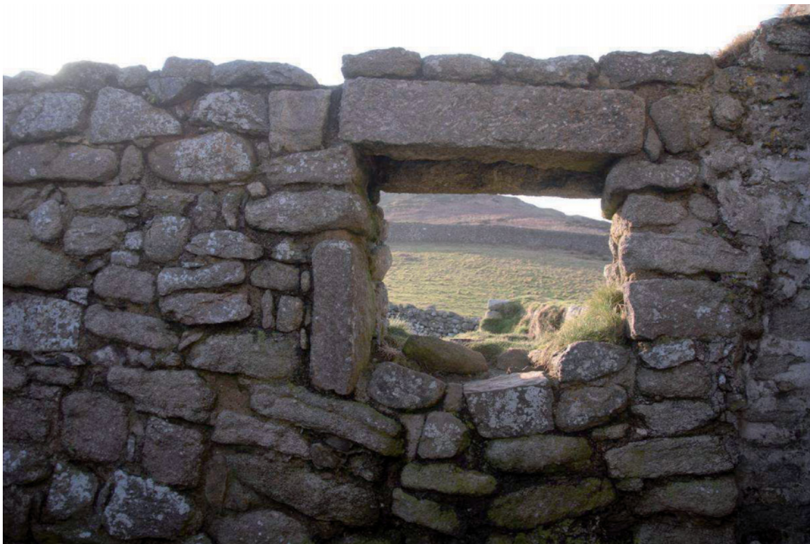
Fig 27. The internal elevation of the small window in the western wall of St. Helen's Chapel in late 2009. HE Digital Image Archive.
