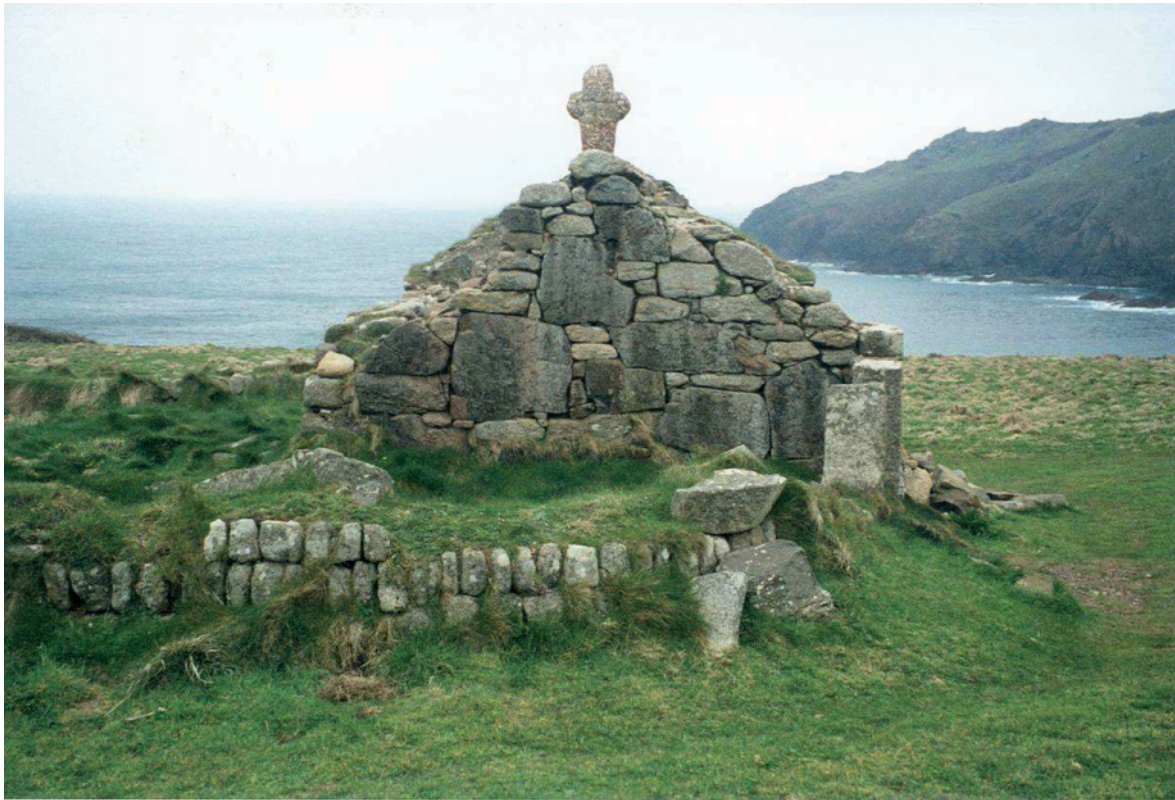
Fig 10. St. Helen's Chapel from the south prior to works showing the massive stones used in the construction of this wall and the cross re-erected on its gable. HE Digital Image Archive.
