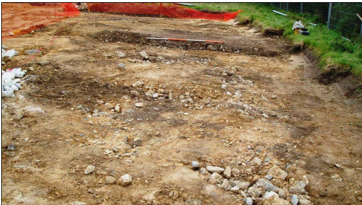
Fig 15 The eastern end of the poor house site, looking east, after stripping.
