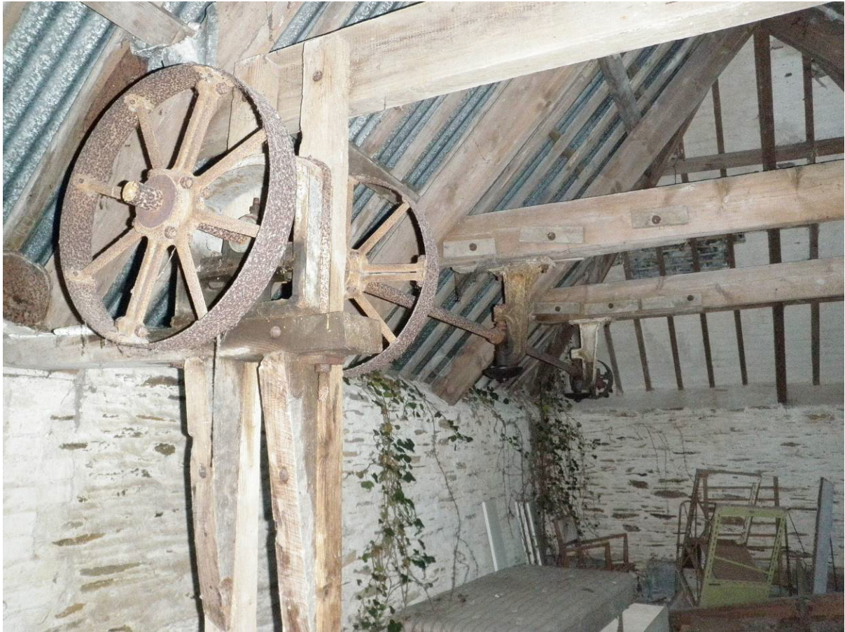
Fig 21: First floor in east range (former threshing barn) showing belt drive wheel for threshing machine/ chaff cutter
