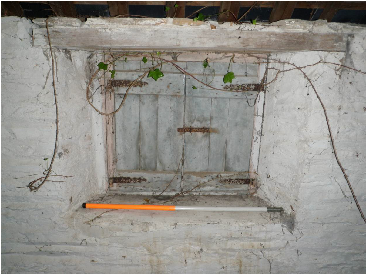
Fig 19: First floor in west range (former hayloft) phase 3 shutters in window
