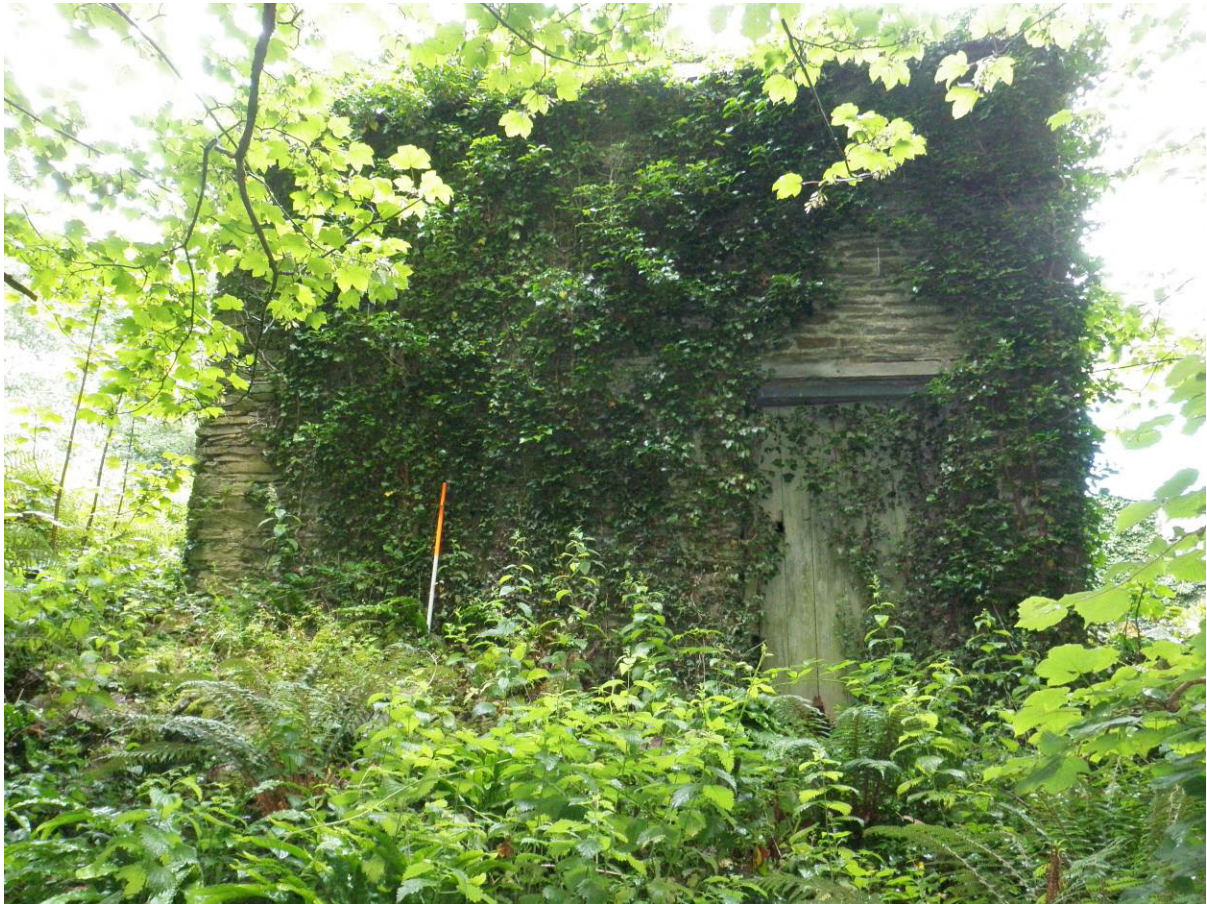
Fig 12: South-west end elevation of west range
