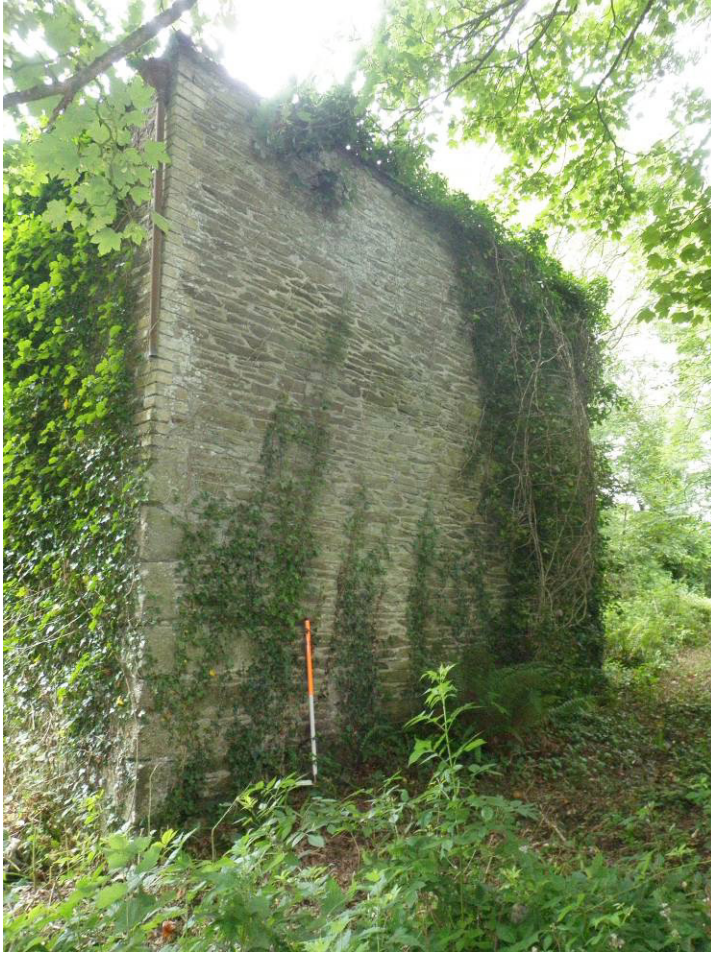
Fig 7: South-east elevation of the east range
