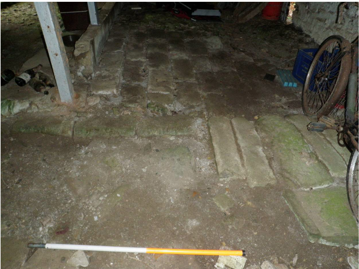
Fig 16: Ground floor in west range (former cow-house) showing granite flooring
