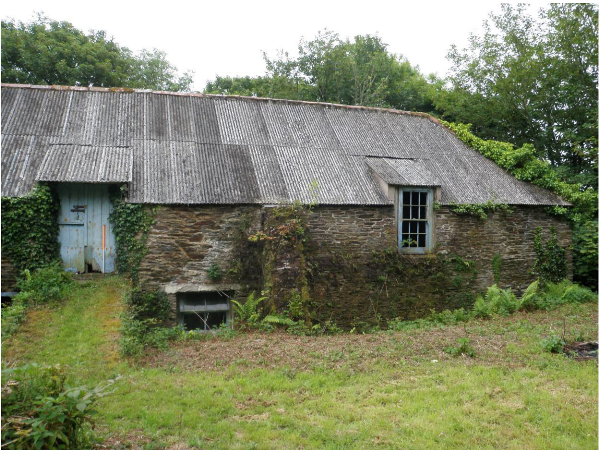
Fig 10: South-west half of north-west elevation
