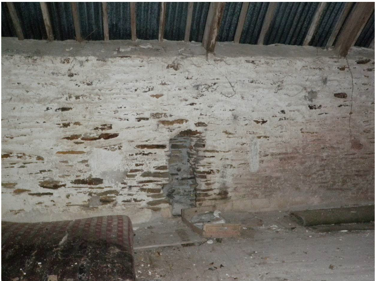
Fig 22: First floor in east range (former threshing barn) showing belt drive opening in north-east wall
