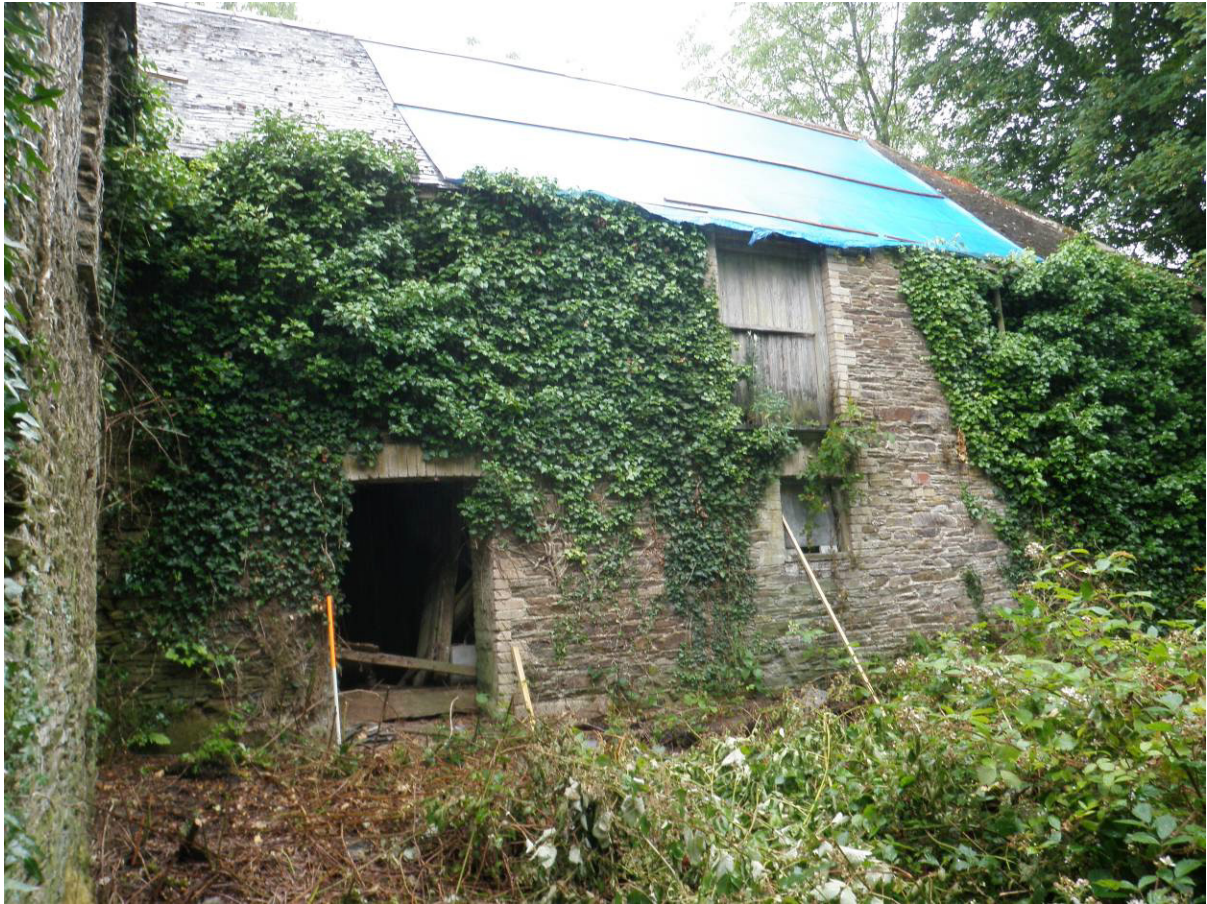
Fig 11: South-west elevation of east range
