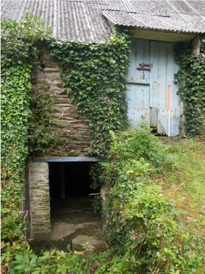
Fig 9: Door openings in north-west elevation
