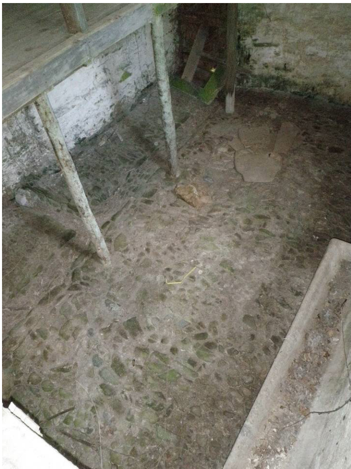
Fig 14: Cobbled floor inside former stables in the west range
