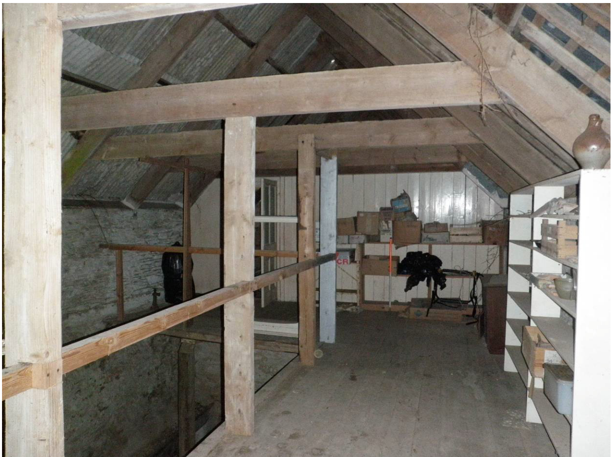
Fig 18: First floor in west range (former hayloft) looking north-east
