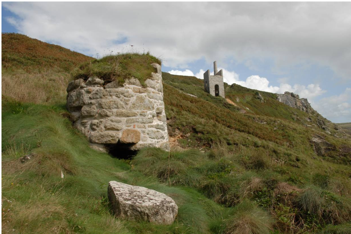
Fig 31. The chimney stump at Old Engine Shaft which may be the only surviving remains of a shaft sinking engine house on this part of the site.
