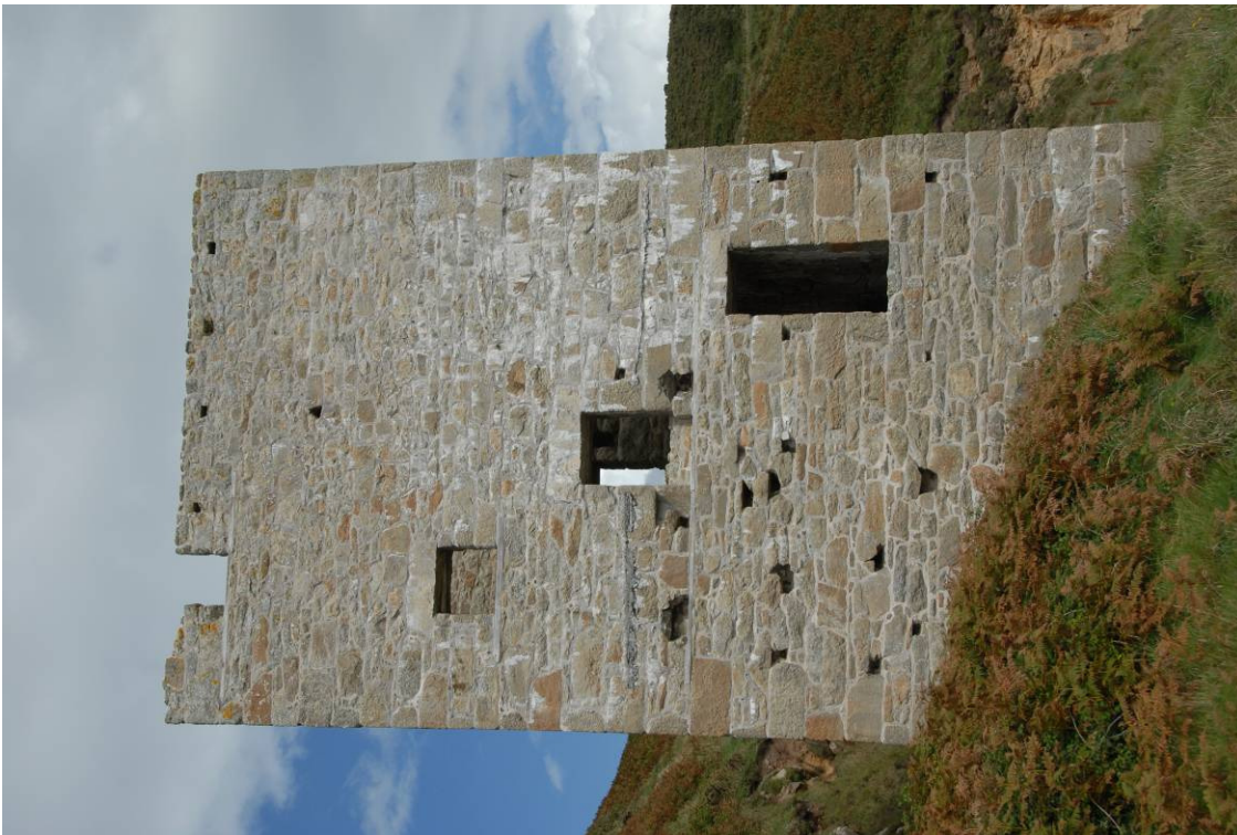
Fig 34. The engine house on Old Engine Shaft from the west, showing the boiler house door and the flashing line of its roof midway up this elevation.
