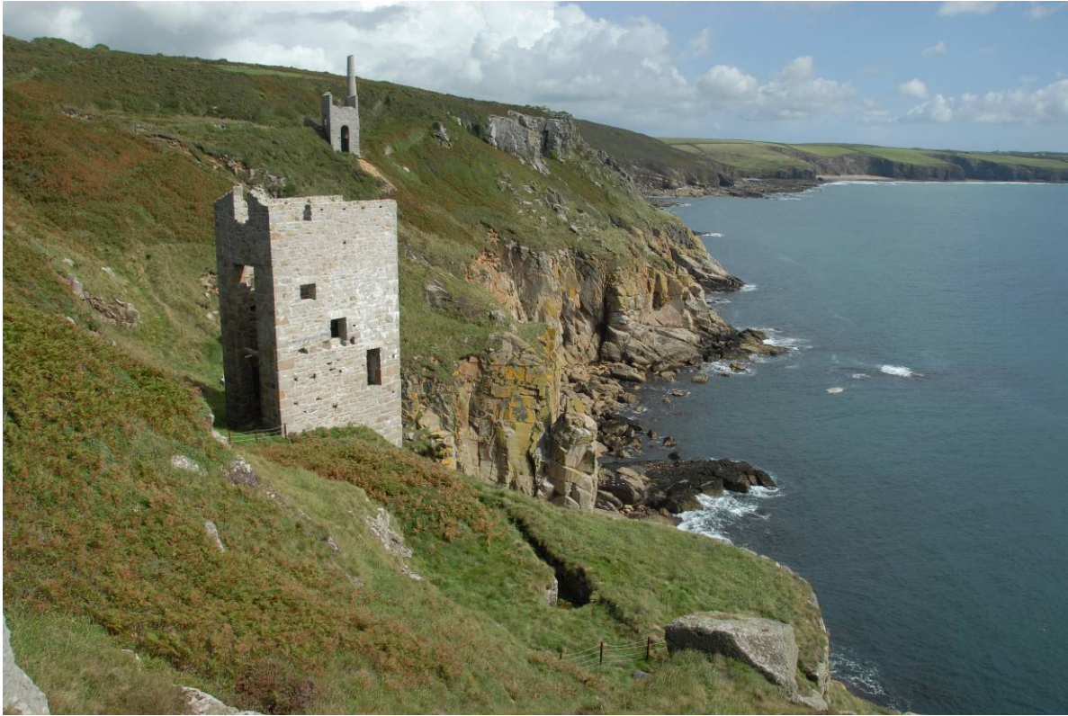
Fig 30. Trewavas mine from the west, with Old Engine Shaft, its engine house and capstan plat in the foreground and New Engine Shaft engine house and chimney in the background. Note the extensive bracken cover on the upper cliffslopes.
