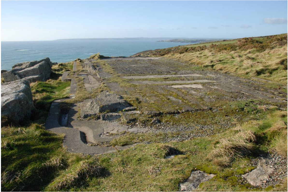
Fig 28. The main building of the Trewavas CHL radar station site seen from the east, showing its concrete floor and plinth (with its gutter), and the remains of one of the buttresses in its near left hand corner.
