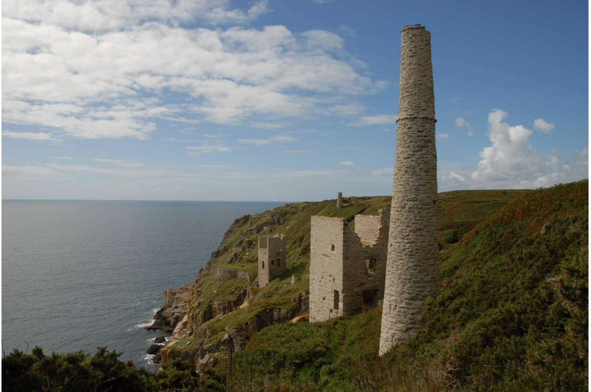
Fig 36. Looking west from the head of the inclined mine trackway past the New Engine shaft chimney and engine house towards the structures at Old Engine Shaft.
