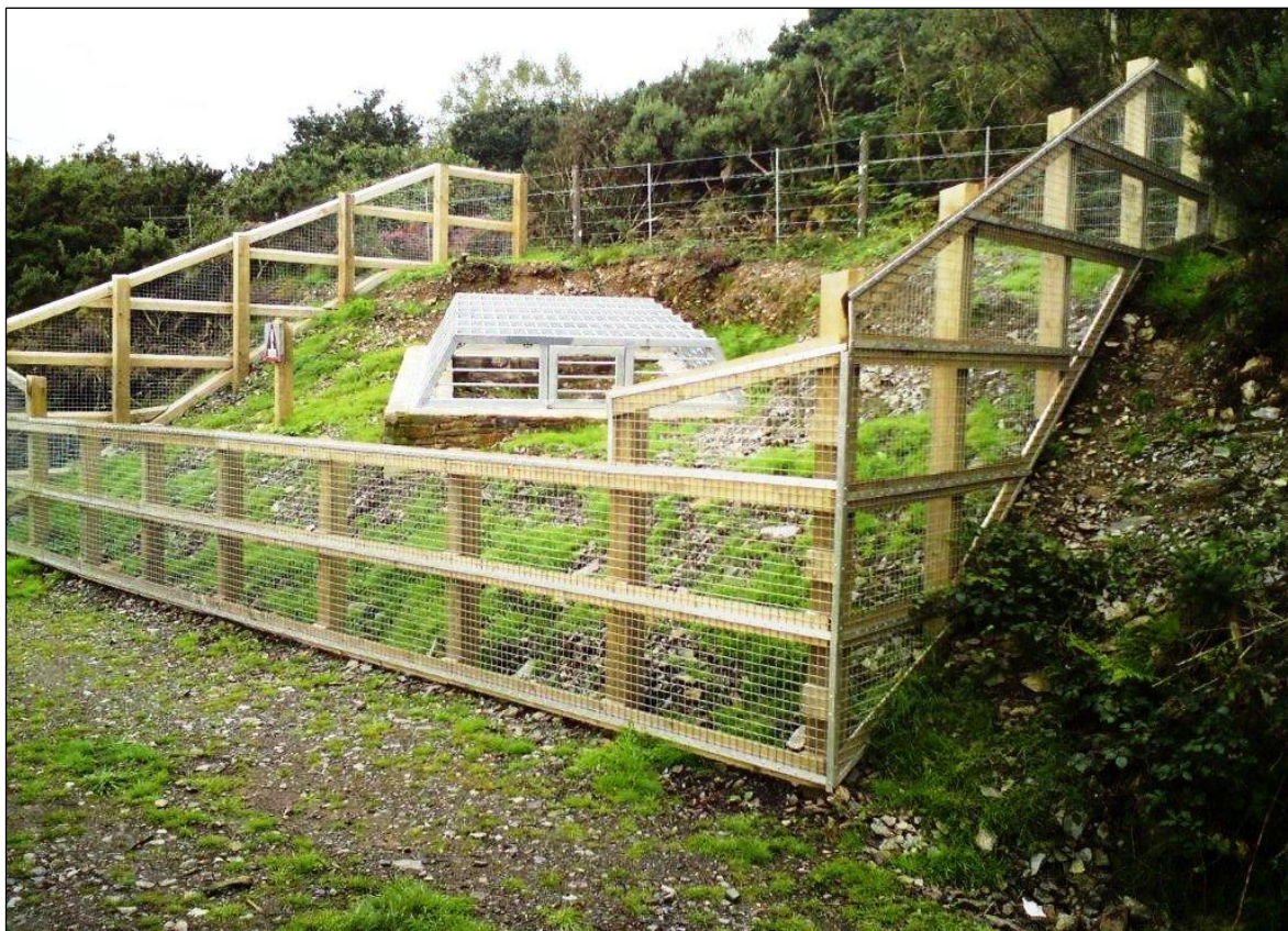
Figure 9 View of Unnamed Shaft after grilling/fencing works (© RG 2009)
