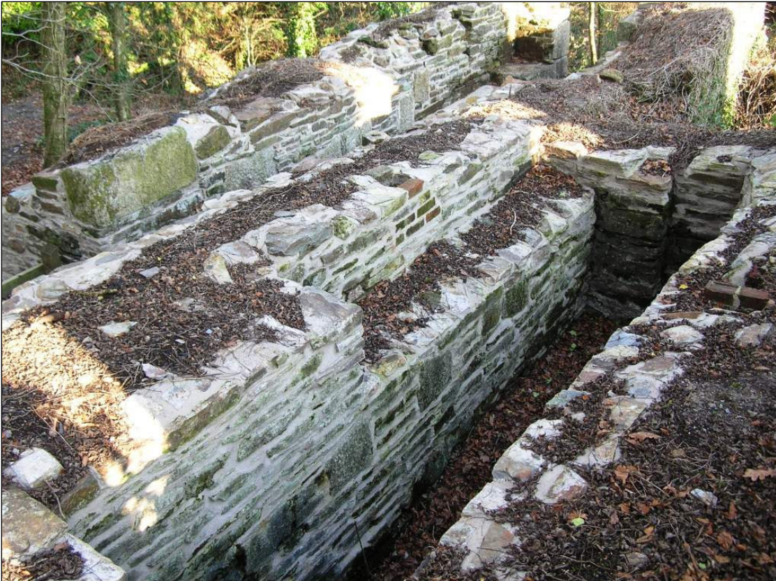
Fig 17 View of the copper crusher flywheel loadings (after works)
