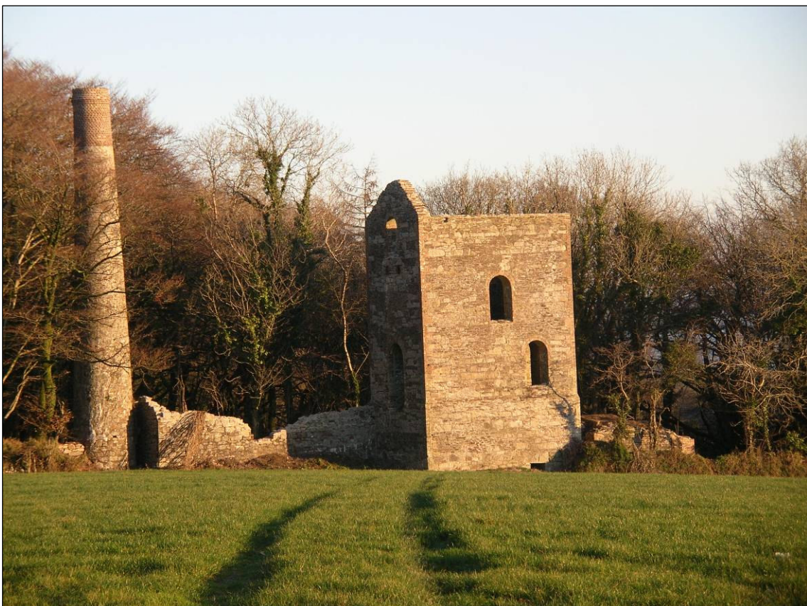
Fig 25 View of the south side of the winding engine house (after works) C Buck 2008 © CC HE Projects
