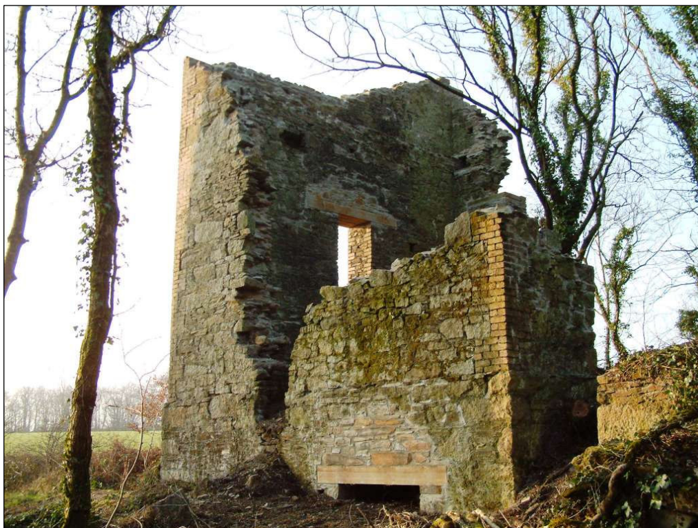
Fig 13 View of the copper crusher (after works) C Buck 2001 © CC CAU
