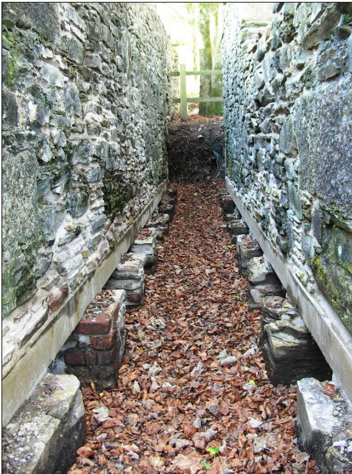
Fig 18 Photograph of the wheelpit (after works)
