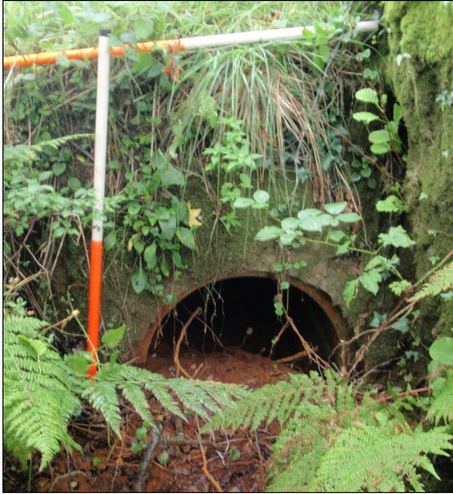
Fig 16 Culvert from the north west
