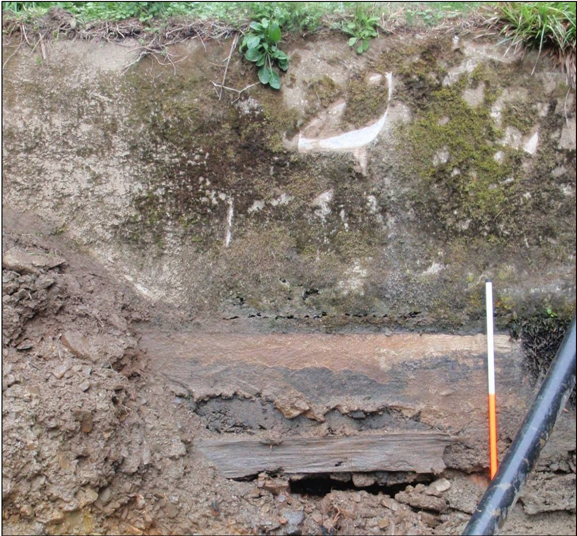
Fig 9 Remains of timber at the wall base
