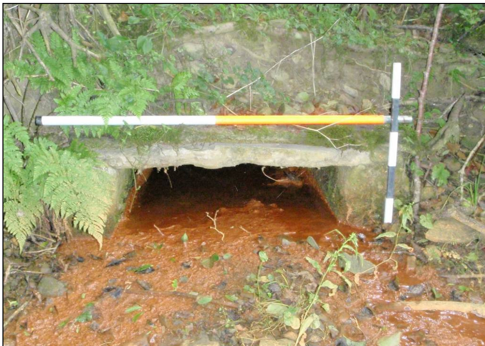
Fig 17 Culvert from the south east
