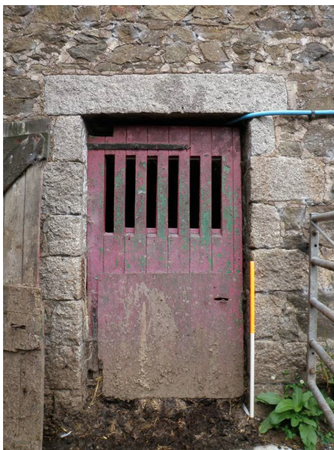
Fig 20: Building 3, original 'hit and miss' ventilated door at west end of south elevation
