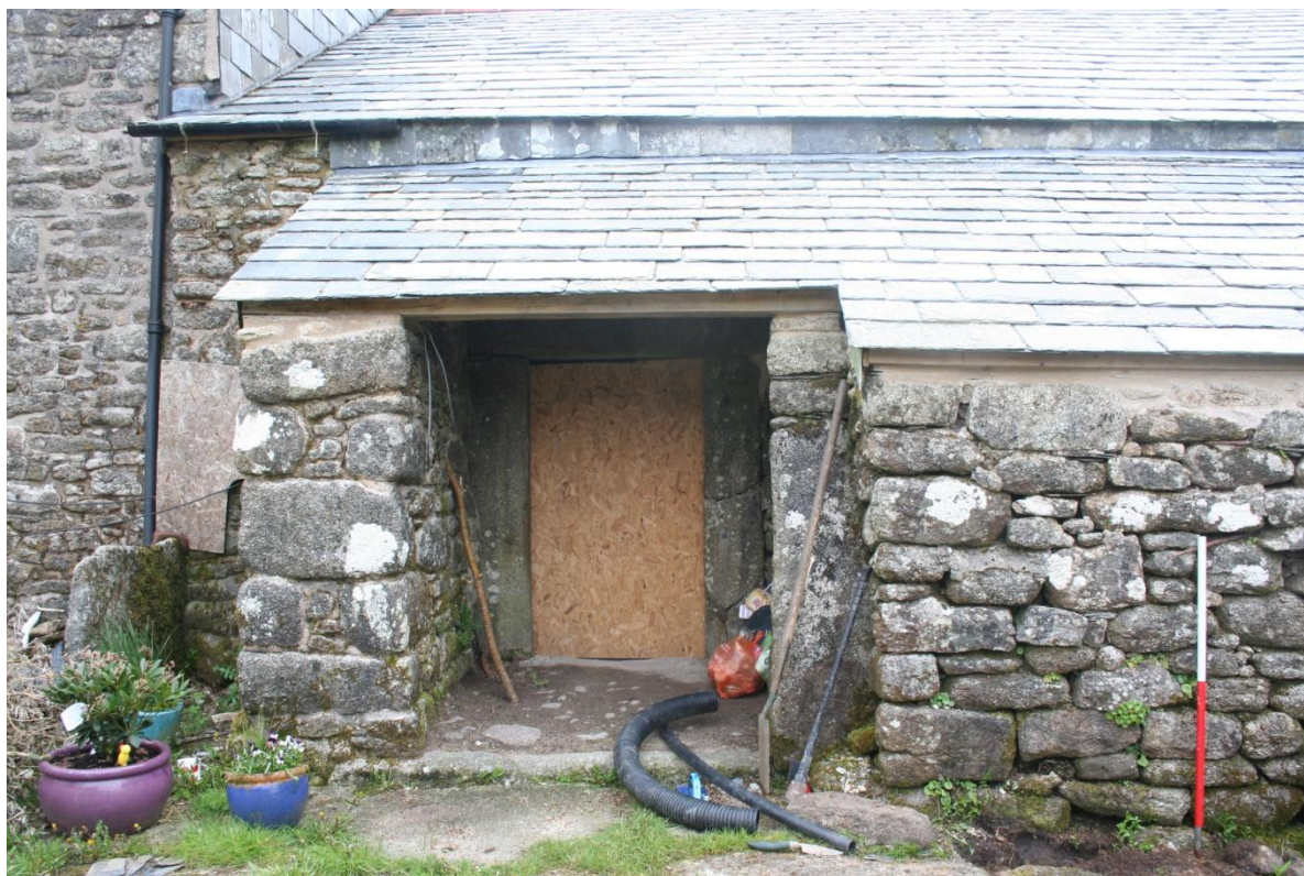
Fig 25 Re-roofed front porch, 2014.
