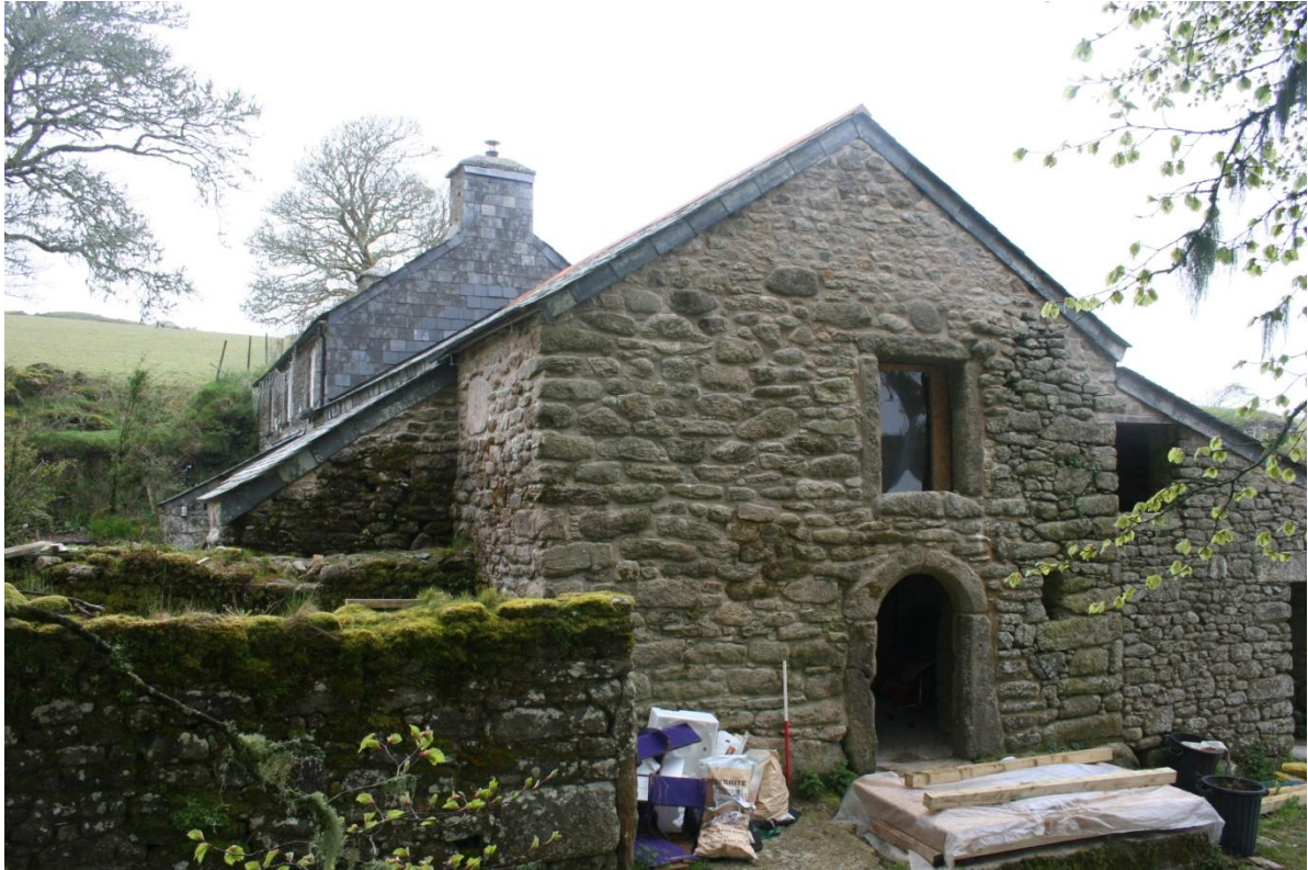
Fig 22 Overall view of the rebuilt lower end in 2014.
