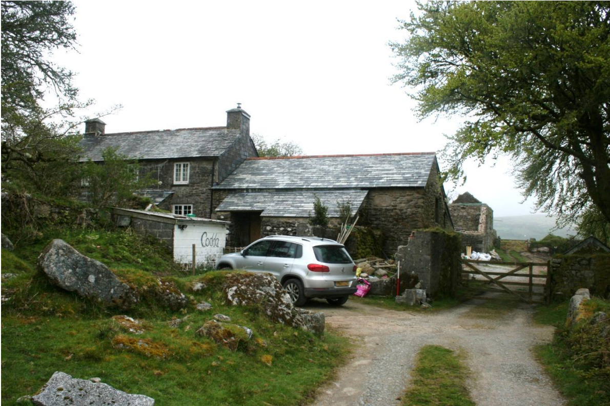
Fig 20 Front view of Codda in 2014, showing new roof on lower end.
