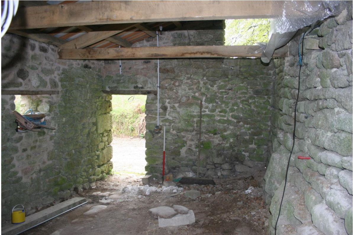
Fig 35 Interior of northern lean-to, looking SE.
