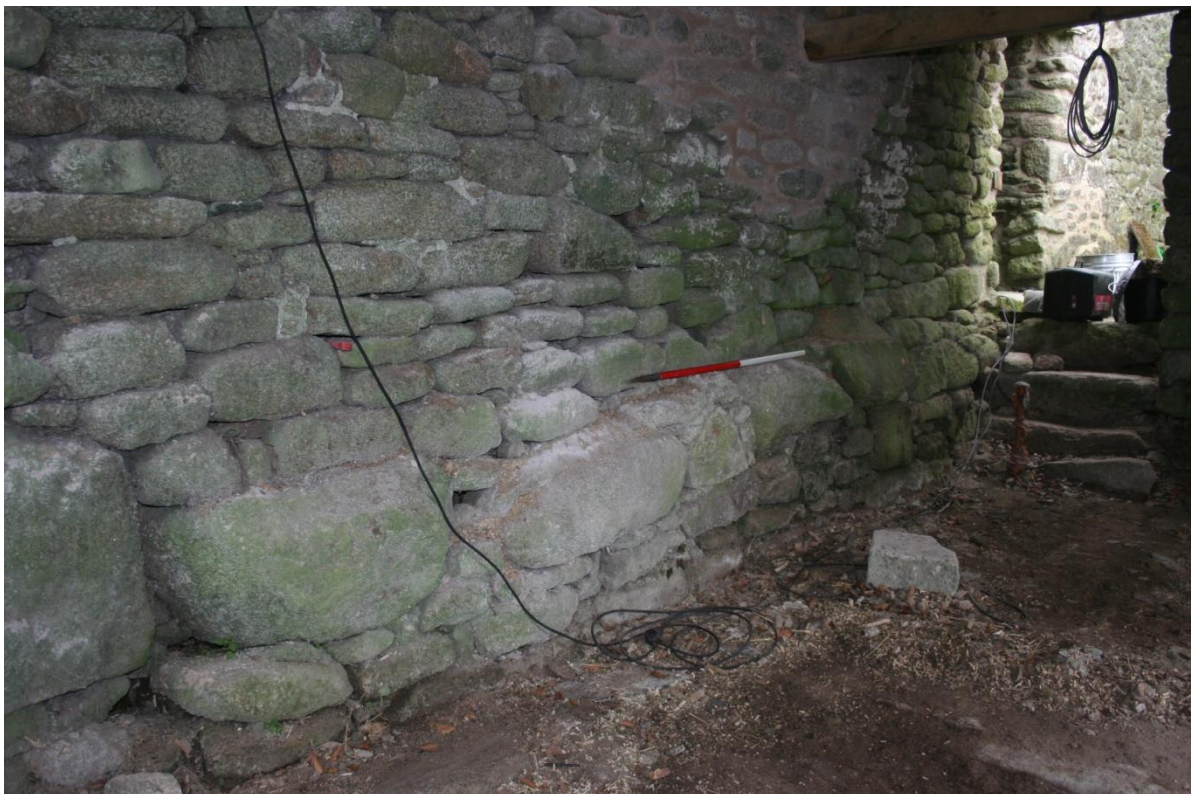
Fig 38 Plinth masonry at base of lower end wall.
