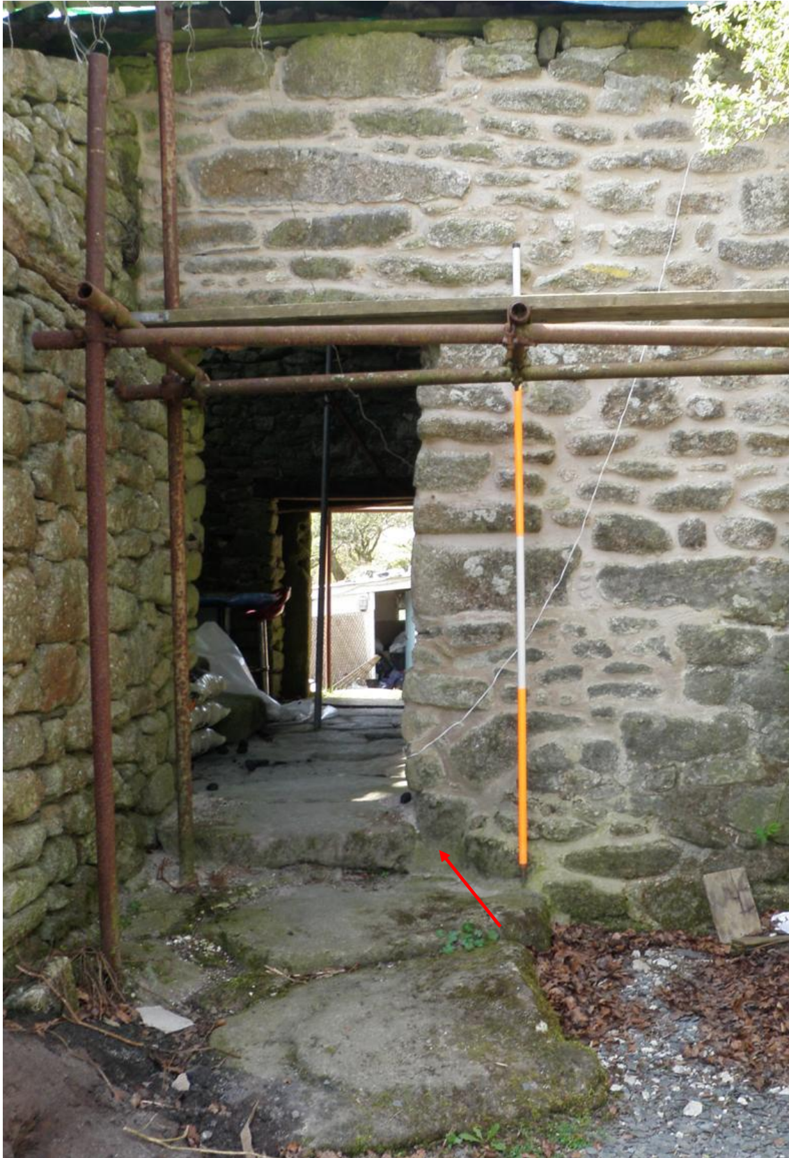
Fig 18 The rear doorway to the through-passage.
