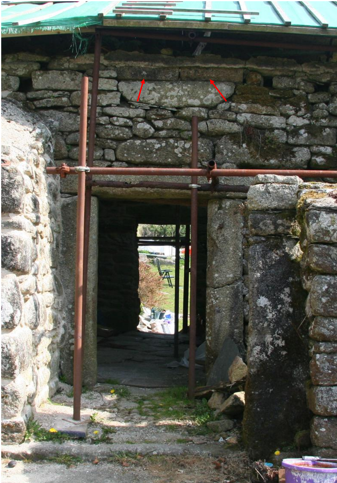
Fig 17 The front entrance to the through-passage
