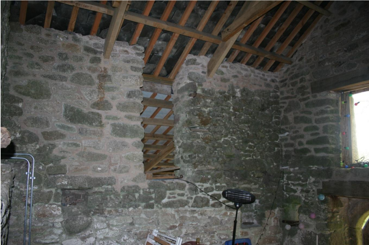
Fig 33 Rebuilt doorway into loft above northern lean-to.
