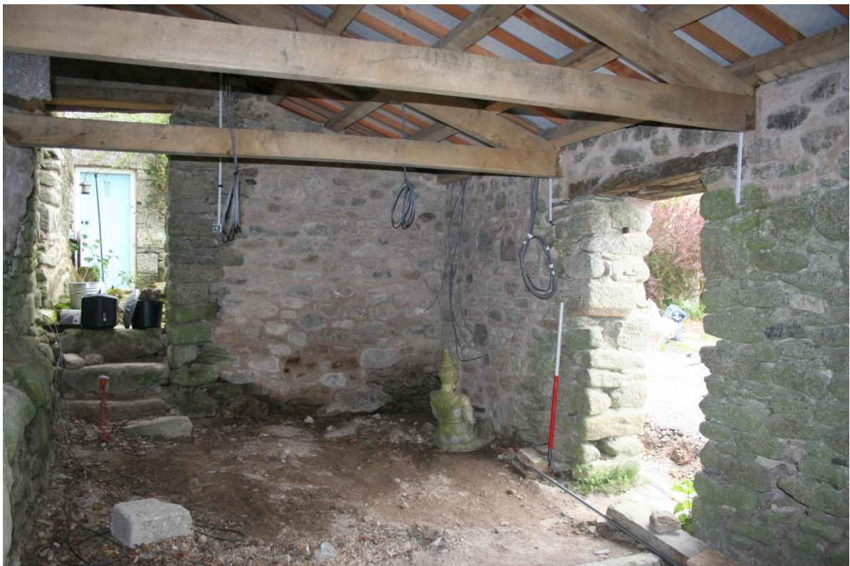
Fig 36 Interior of northern lean-to, looking NW.
