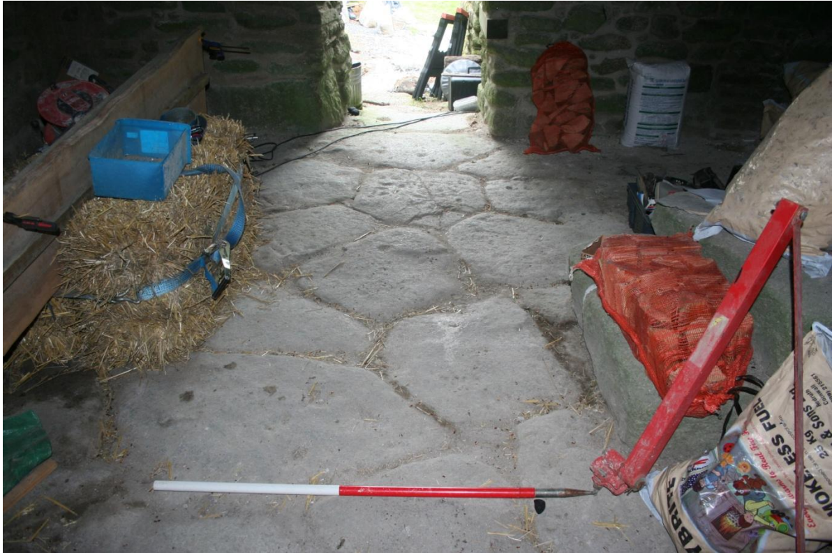
Fig 29 Granite paving in through-passage.
