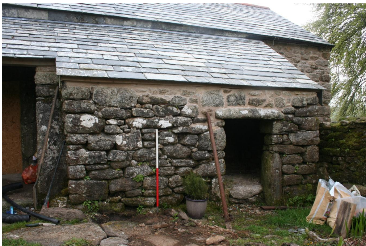
Fig 26 Re-roofed front lean-to, 2014.
