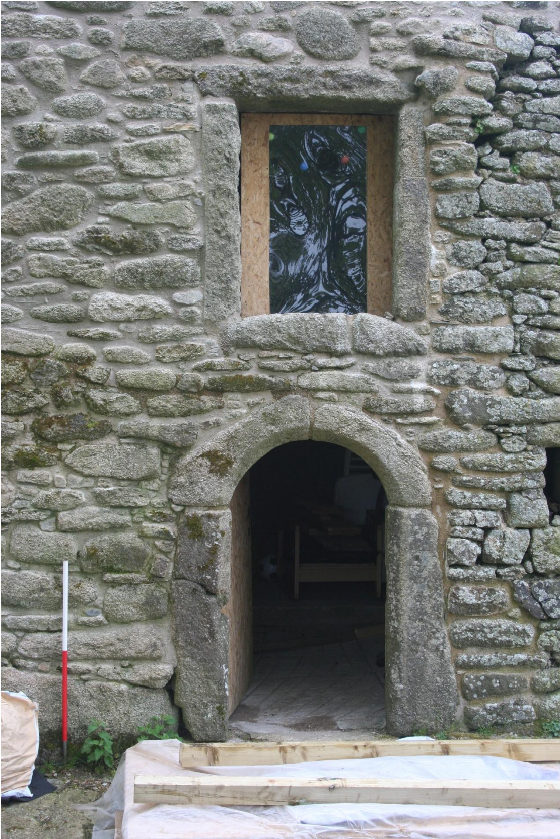
Fig 24 Detail of the rebuilt lower end openings, April 2014.
