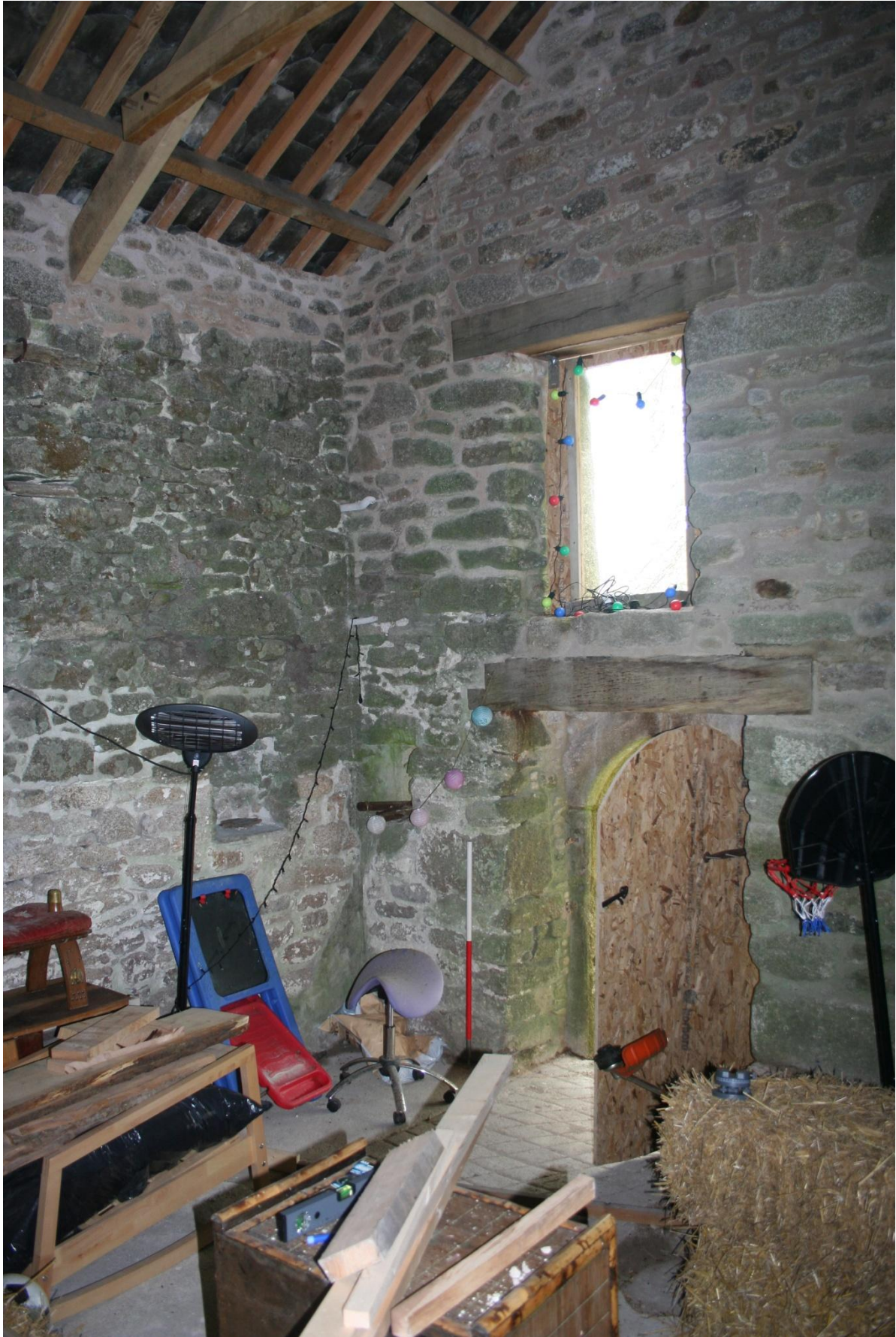
Fig 32 View of interior within rebuilt lower end, 2014.
