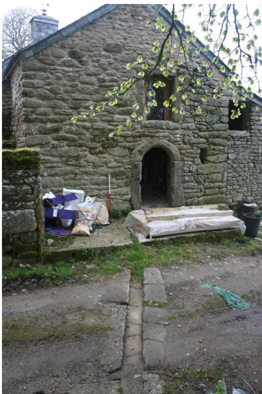
Fig 23 Drain from lower end.
