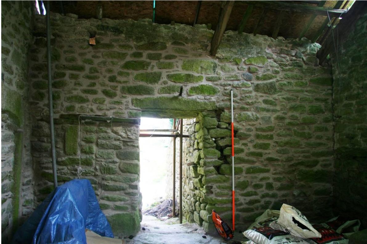
Fig 19 The interior of the through-passage, looking towards the rear doorway.
