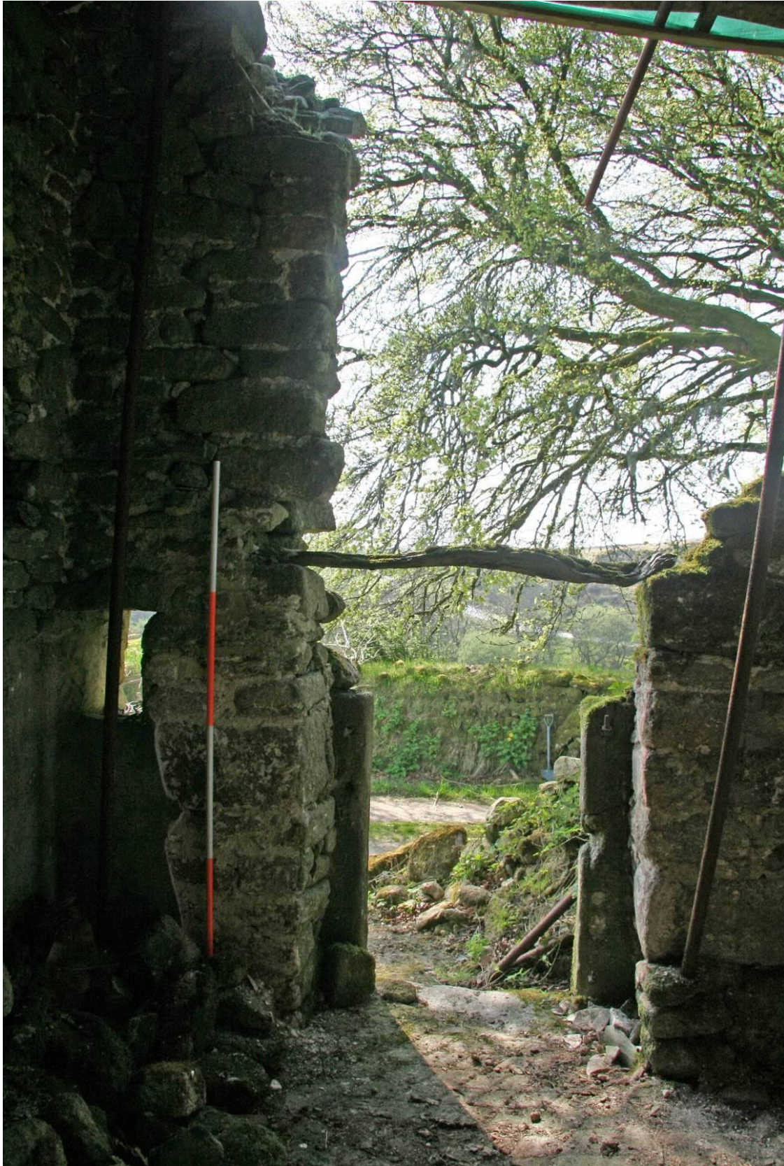
Fig 15 Inside view of the lower end openings.
