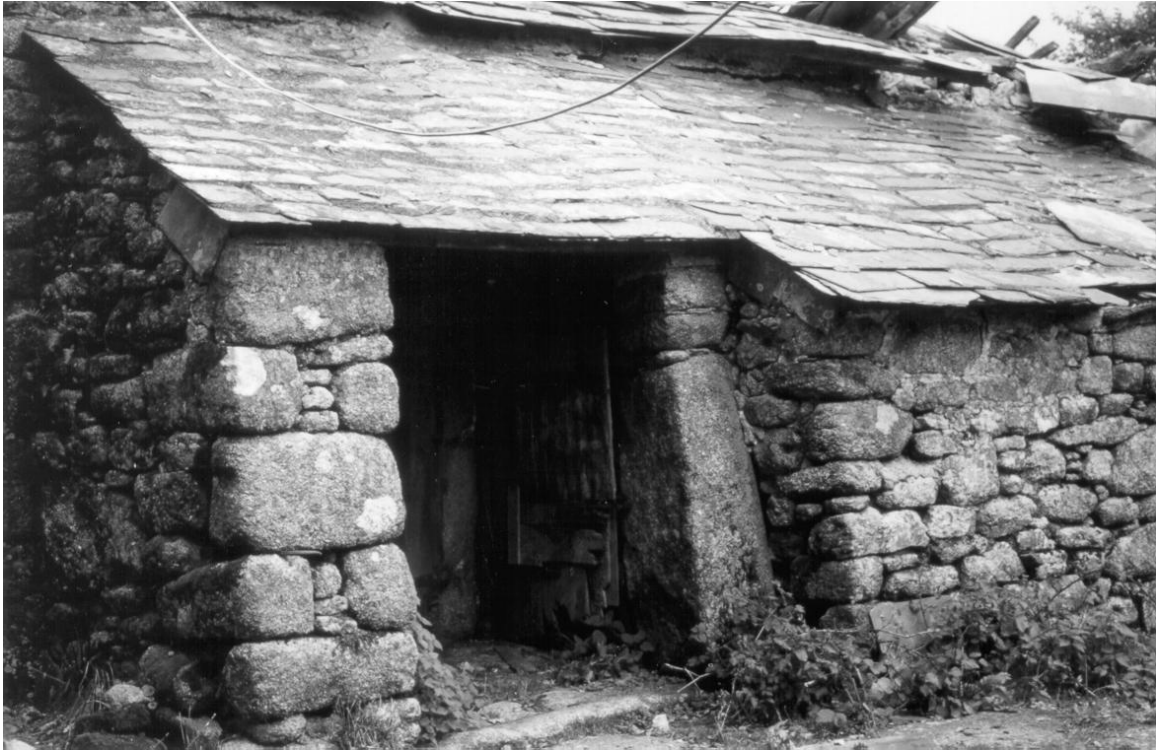
Fig 10 Surviving porch roof in 1981. (Photograph kindly supplied by Peter Herring)
