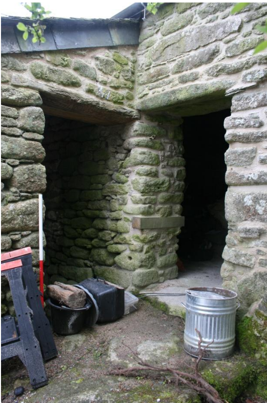
Fig 28 Rear through-passage doorway (right) and re-opened doorway into lean-to (left).
