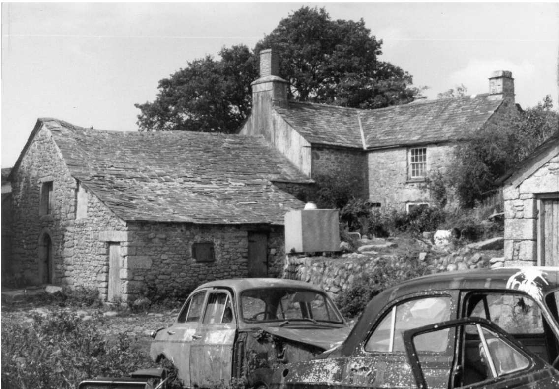
Fig 11 Rear view of the farmstead in 1981, when the roof of the lower end and lean-to were decaying but relatively intact.
