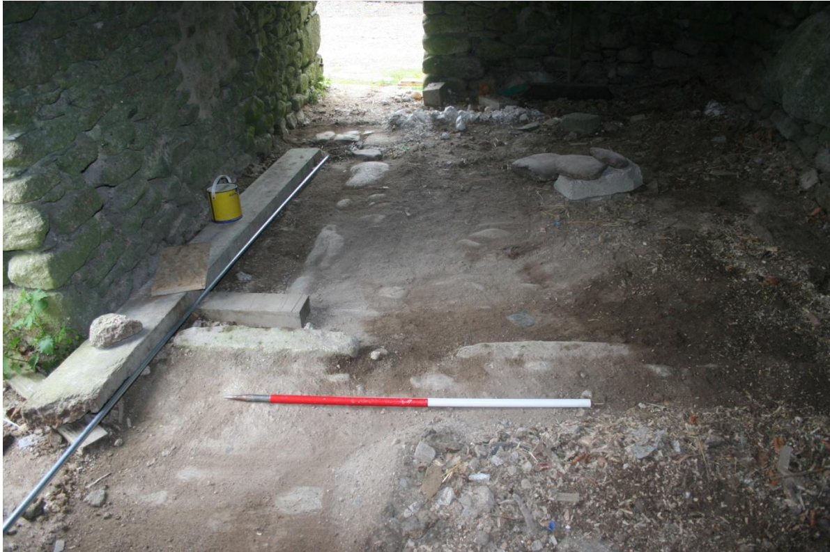
Fig 37 Floor of northern lean-to, showing stall division and part of a drain towards the lower doorway.
