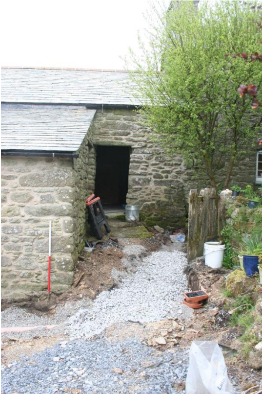
Fig 27 Rear through-passage doorway, 2014.
