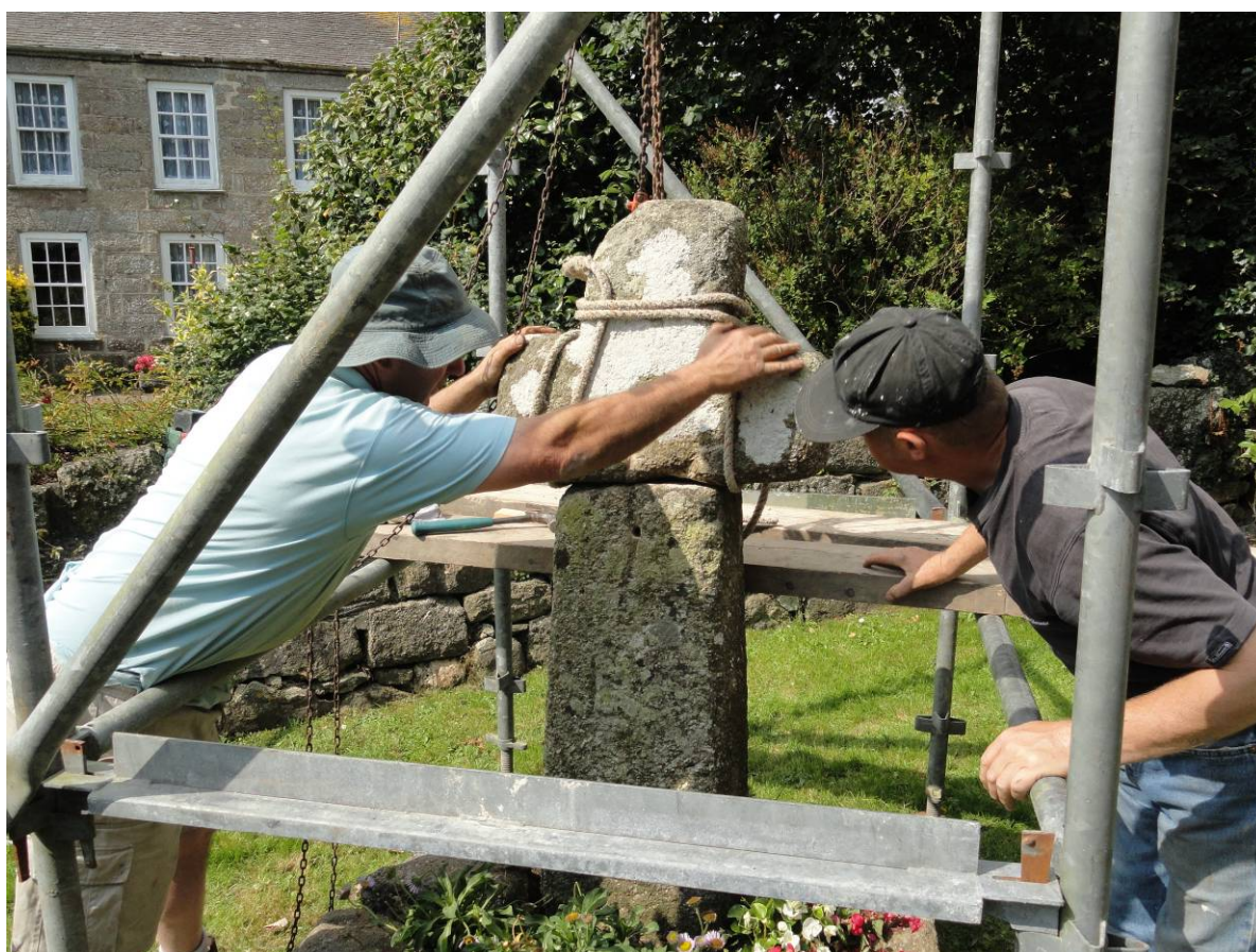
Fig 16 Lowering the cross-head onto the new pin
