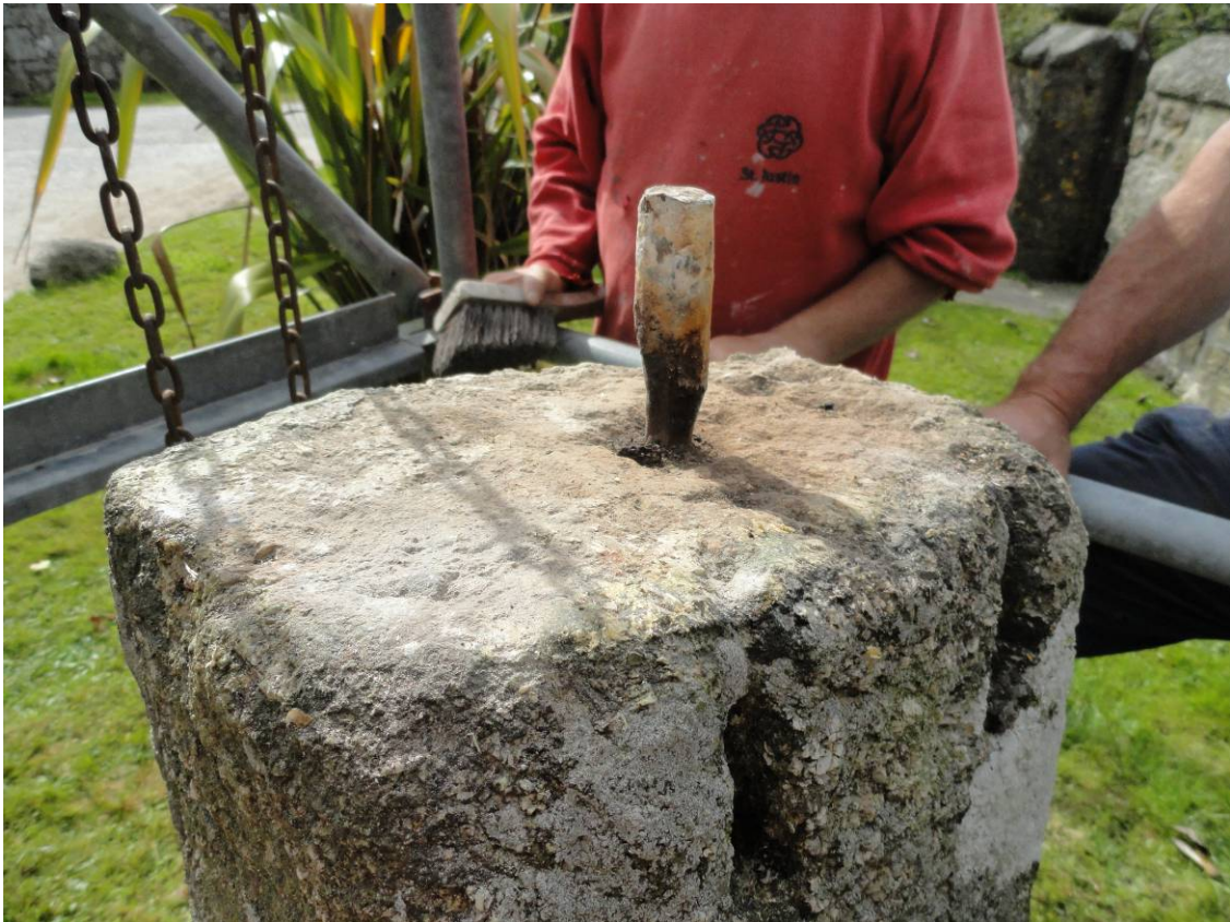
Fig 11 The iron pin, showing corrosion at the centre
