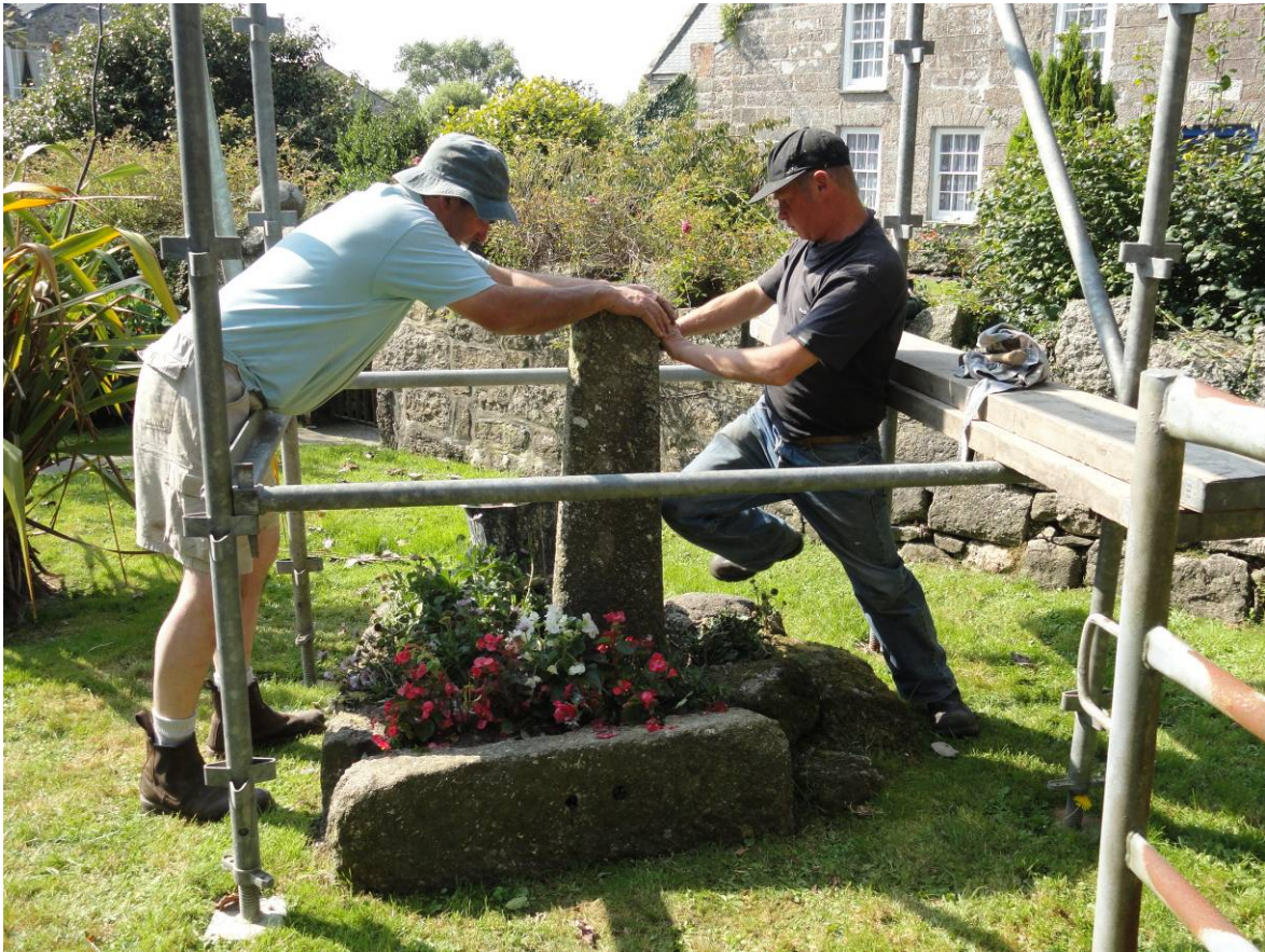
Fig 15 Straightening the cross-shaft
