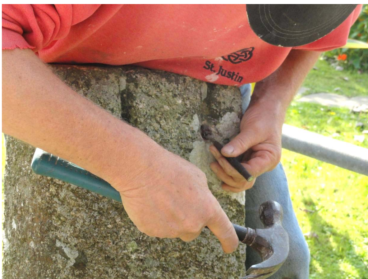
Fig 13 Removing the stub-ends of the staples
