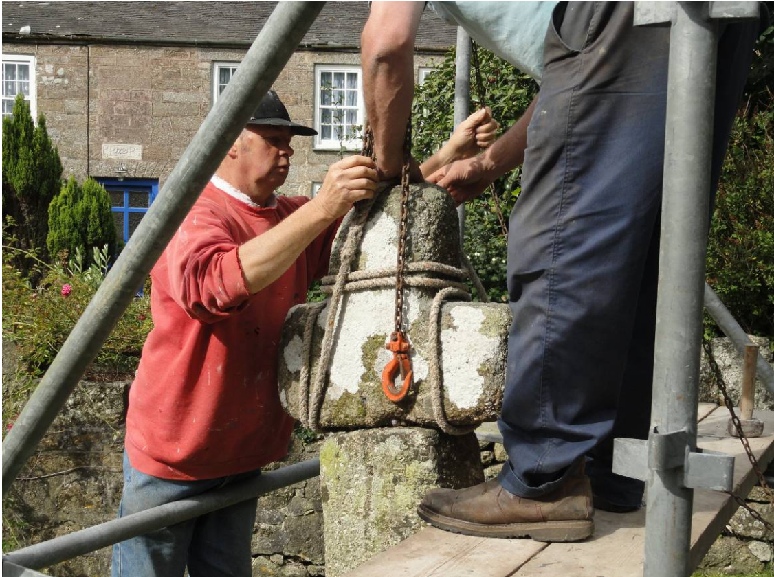
Fig 10 Removing the cross-head
