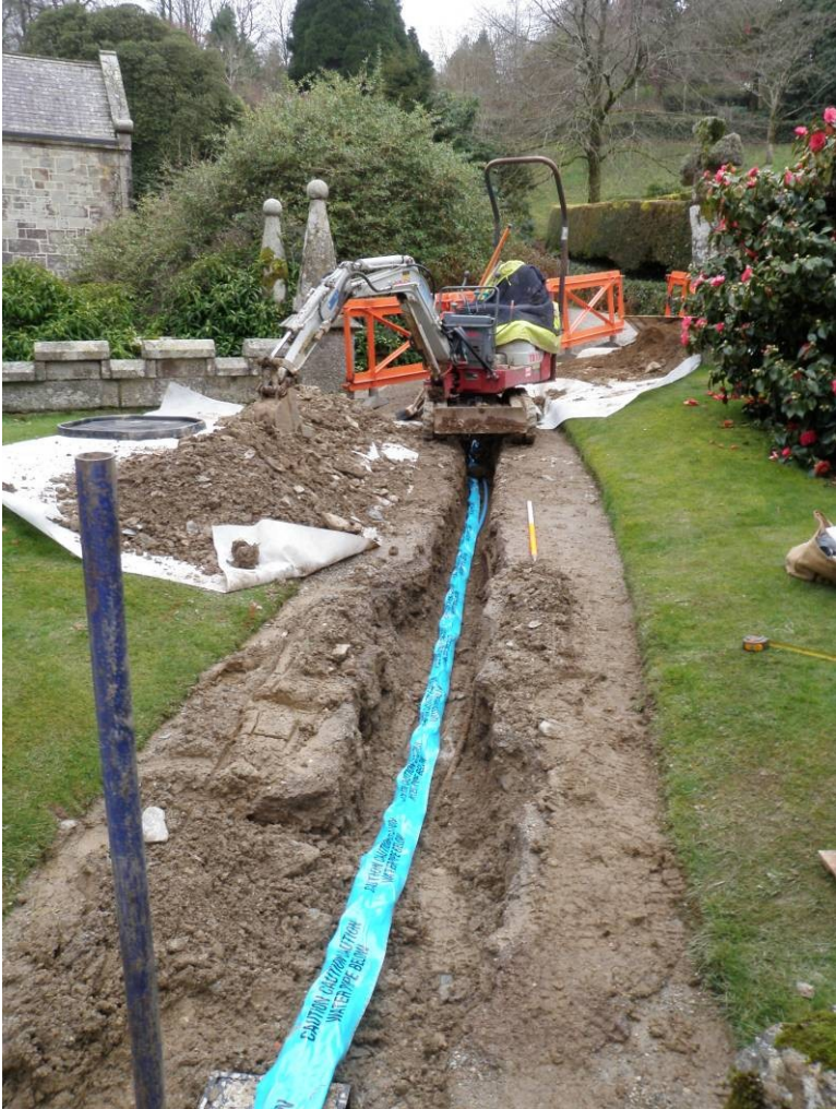
Fig 29 Area D, Trench 13 through churchyard, looking south-west
