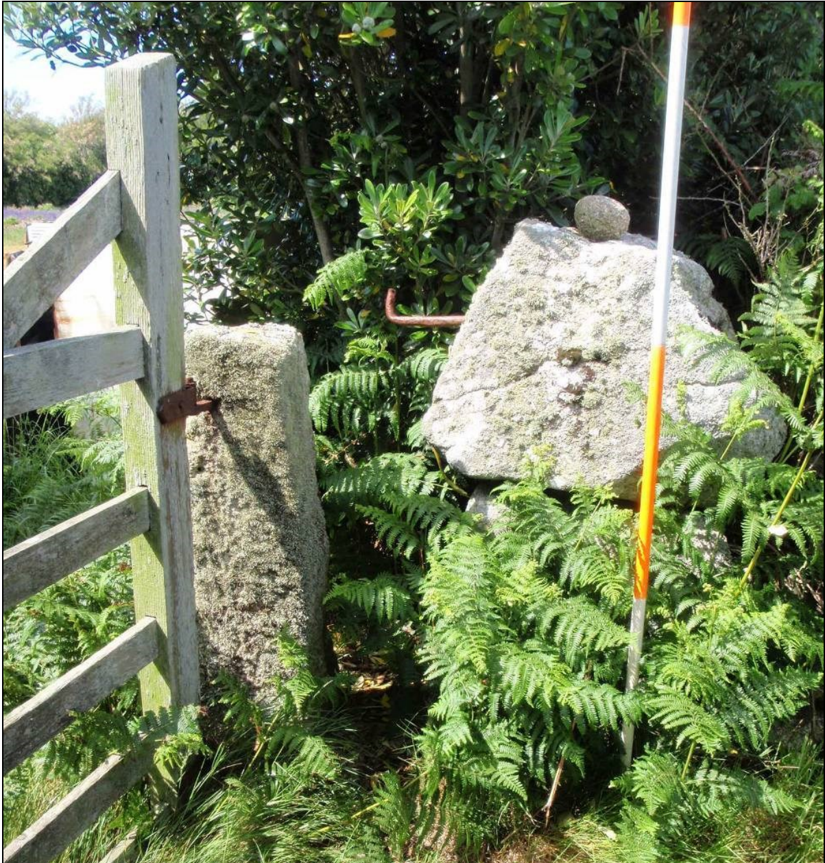
Fig 43 Two phases of stone gate supports in a boundary adjoining Barnaby Lane, St Agnes. To the left a squared and roughly dressed gatepost, with an earlier provision for gate-hanging in the form of a large boulder with an iron gate support set in it perched on the end of a stone boundary. (Photograph: Historic Environment, Cornwall Council.)
