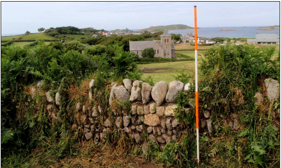
Fig 40 Tresco 3 boundary 13 has clearly slumped a little and undergone some minor repair or patching since it was built in the mid nineteenth century (cf Fig 39), making the original regular coursed form of its facing stonework less obvious. (Photograph: Historic Environment, Cornwall Council.)
