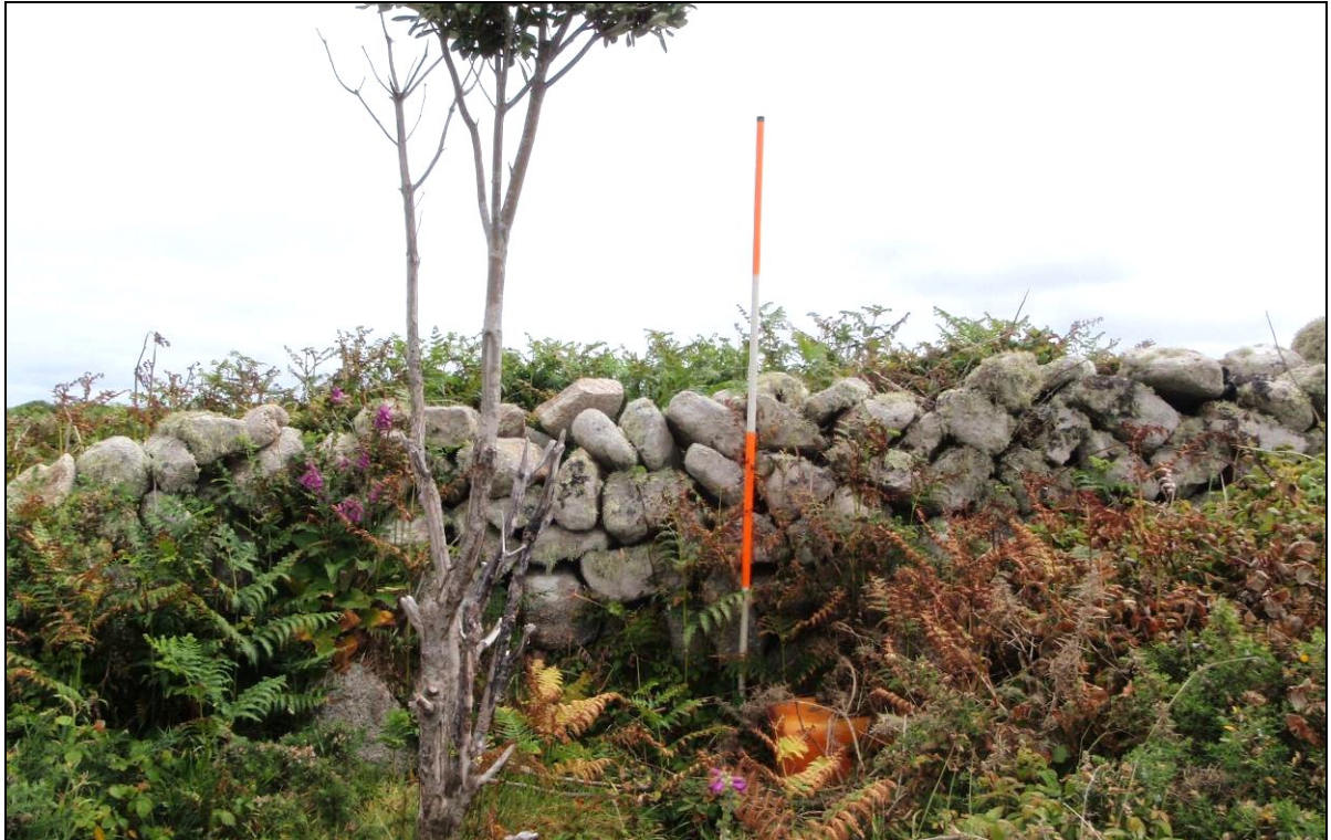
Fig 21 St Agnes 2 boundary 75 is the stone-faced stone wall immediately behind the girls in the historic photograph reproduced as Fig 20. The difference in vegetation cover resulting from the cessation of rough ground grazing and reduced intensity of exploitation of the enclosed area is readily apparent. The boundary remains in good condition over at least part of its length. (Photograph: Historic Environment, Cornwall Council.)
