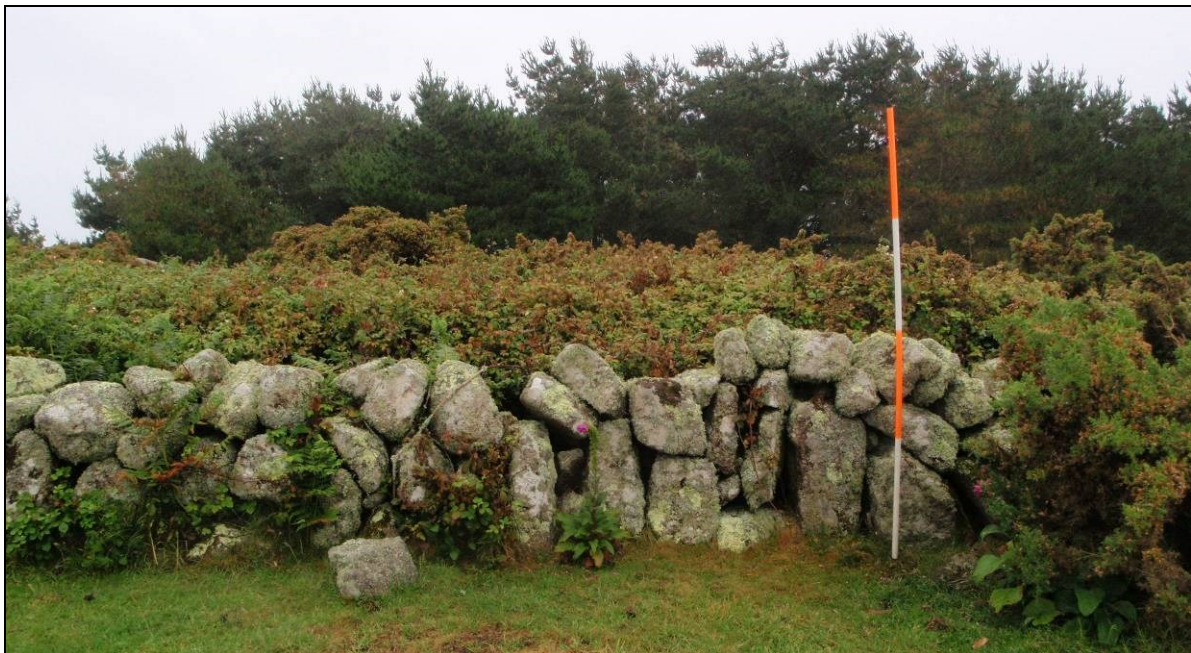
Fig 31 St Mary's 3 boundary 53: the dry-stone wall dividing the enclosed land from adjacent rough ground incorporates some earth-set orthostats. (Photograph: Historic Environment, Cornwall Council.)
