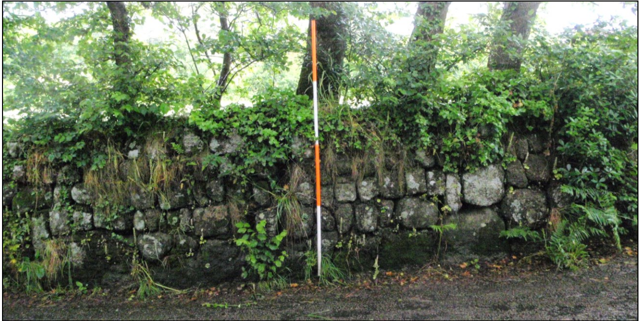
Fig 30 St Mary's 2 boundary 39, a stone-faced earth wall bordering the public road, is of fairly regular coursed stonework based on substantial horizontally-laid grounders. (Photograph: Historic Environment, Cornwall Council.)
