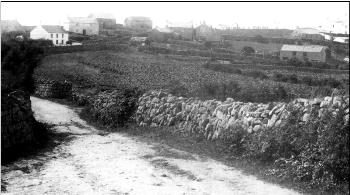
Fig 24 A Francis Frith photograph of St Agnes in 1892. The random stonework of the 'traditional' stone-faced stone wall in the foreground contrasts with the boundary of gradated, coursed stones and transversely-set capstones visible in the middle distance. The latter is probably to be attributed to the Augustus Smith period on Scilly. (Photograph: © Francis Frith Collection. Reproduced from Cowan 2001, 62-3.)
