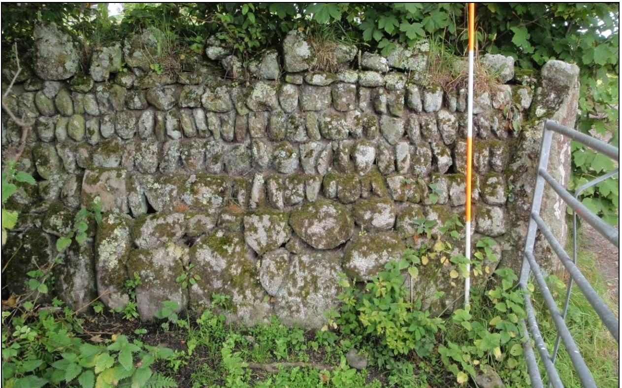
Fig 42 A granite orthostat used as a gatepost and the terminal for a stone-faced earth wall at Borough Farm, Tresco. (Photograph: Historic Environment, Cornwall Council.)
