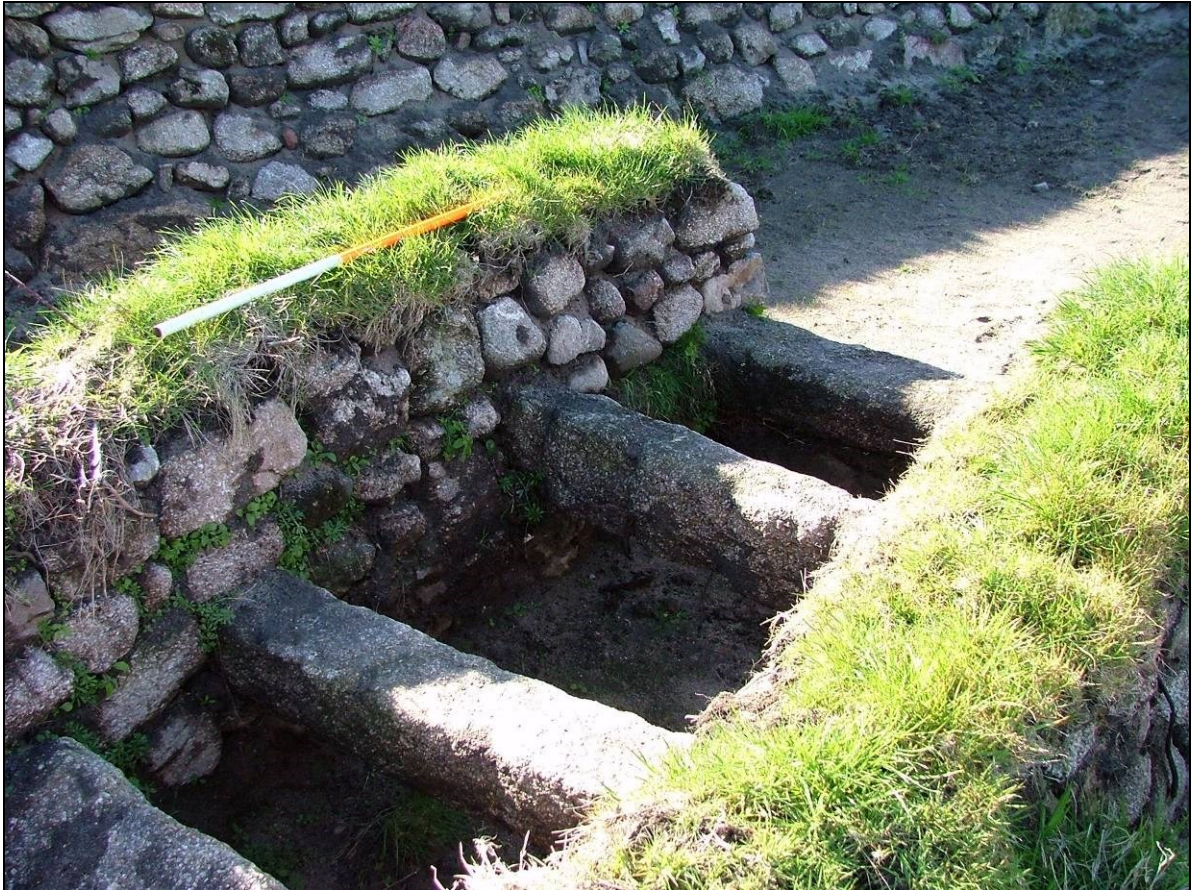
Fig 46 Tresco survey area 3: the restored cattle grid in boundary 31 with modern boundary 32 behind; photographed after reconstruction in 2003. (Photograph: Historic Environment, Cornwall Council.)
