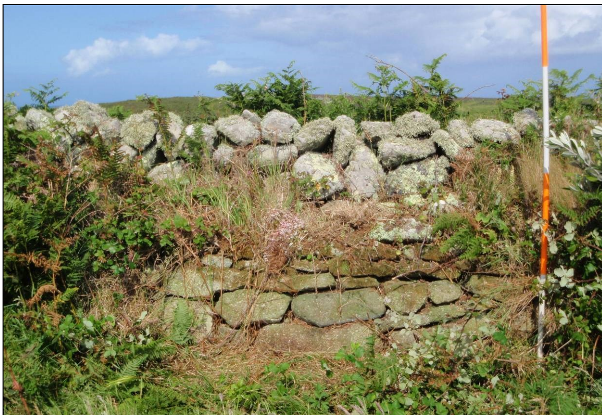
Fig 27 St Martin's 2a, boundary 41: a dry-stone wall imposed on an unusual stone-faced earth wall of semi-coursed horizontally-laid stonework. (Photograph: Historic Environment, Cornwall Council.)
