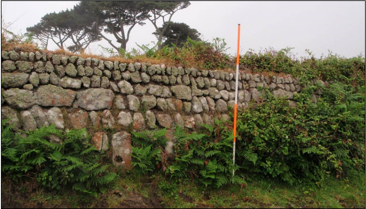
Fig 32 Mount Todden Farm (St Mary's 3), boundary 8. This is one of the stone-faced earth walls attributed to the work of Charlie Guy in the inter-war period (Arthur Swift, pers comm). (Photograph: Historic Environment, Cornwall Council.)
