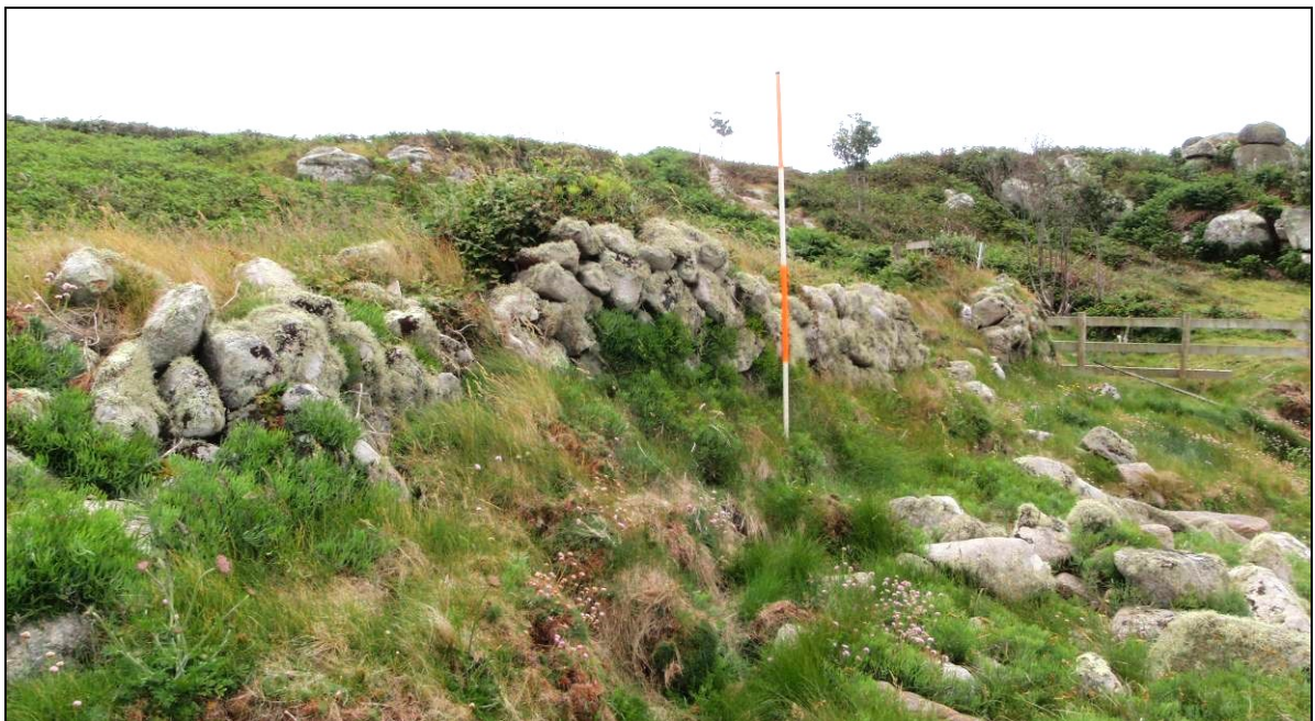
Fig 22 St Agnes 2 boundary 76 is visible in the middle distance on the left hand side of Fig 20. It has survived less well than boundary 75 and now needs extensive repair. Its location alongside the coast path means that it is a highly visible element in this distinctive landscape. (Photograph: Historic Environment, Cornwall Council.)
