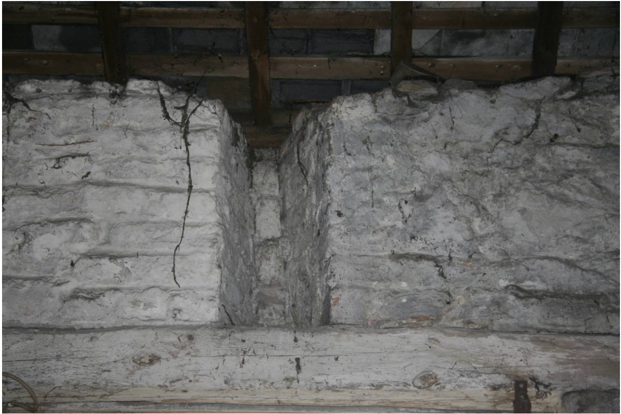
Fig 14 Detail of the ventilation slit above the doorway
