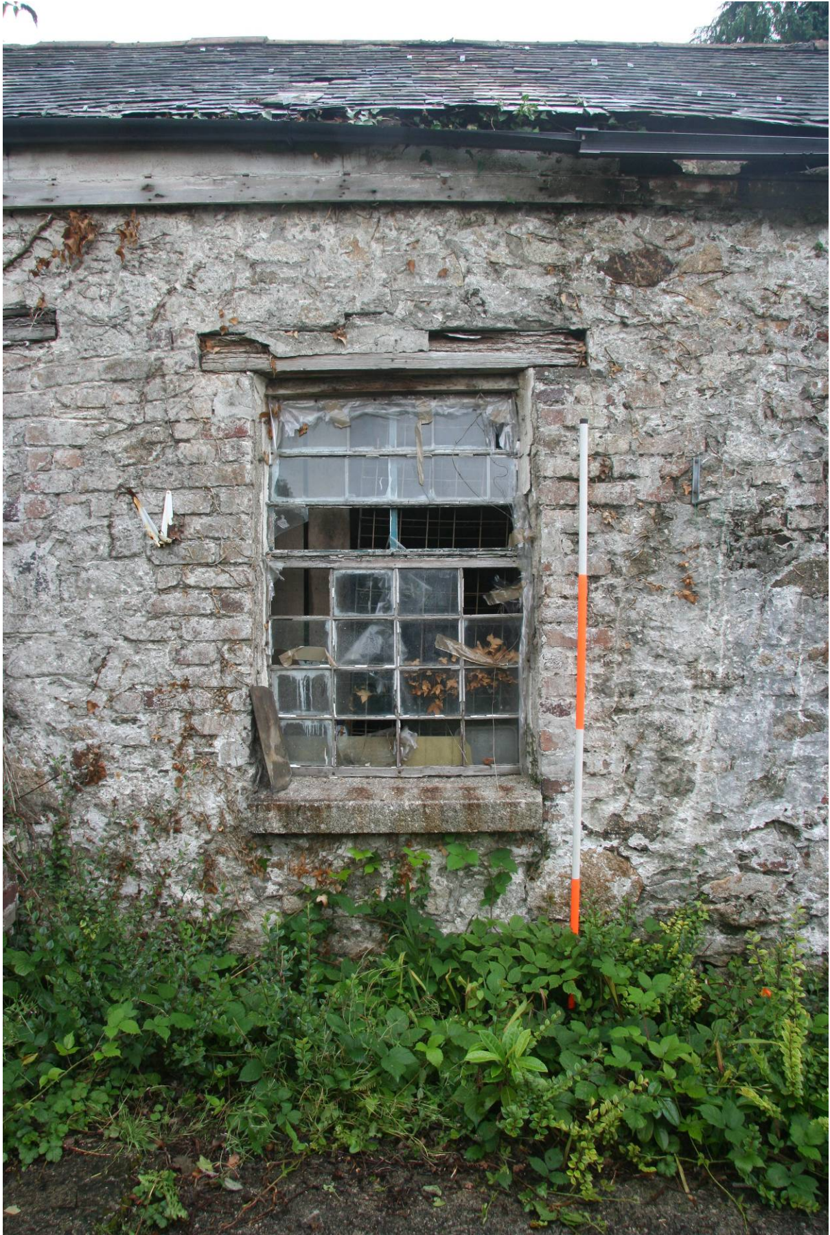
Fig 9 Window lighting upper (western) end of building, with original granite sill Window frames and glazing are earlier 20 th century replacements
