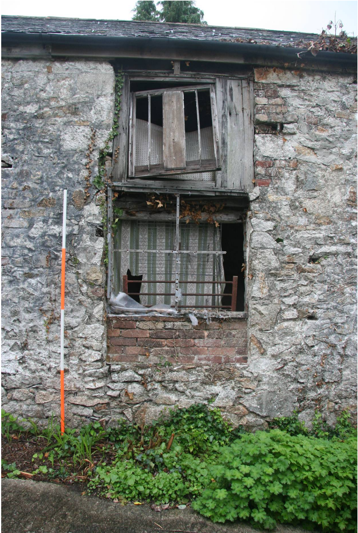
Fig 11 Pair of openings in south wall
