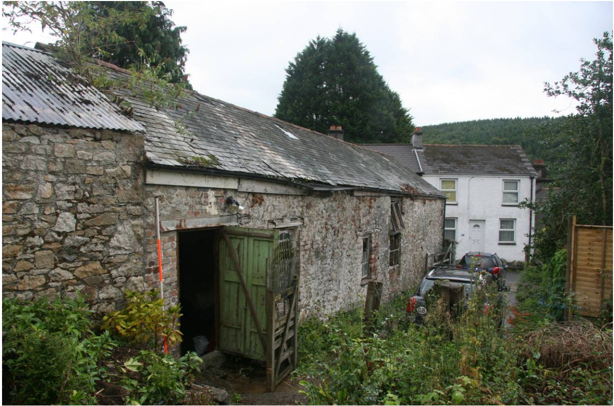
Fig 7 A view along the south elevation, looking NE
