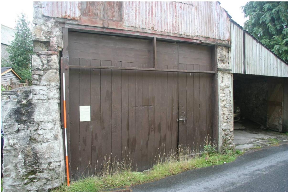
Fig 8 Eastern gable end and principal entrance, fronting onto Under Road
