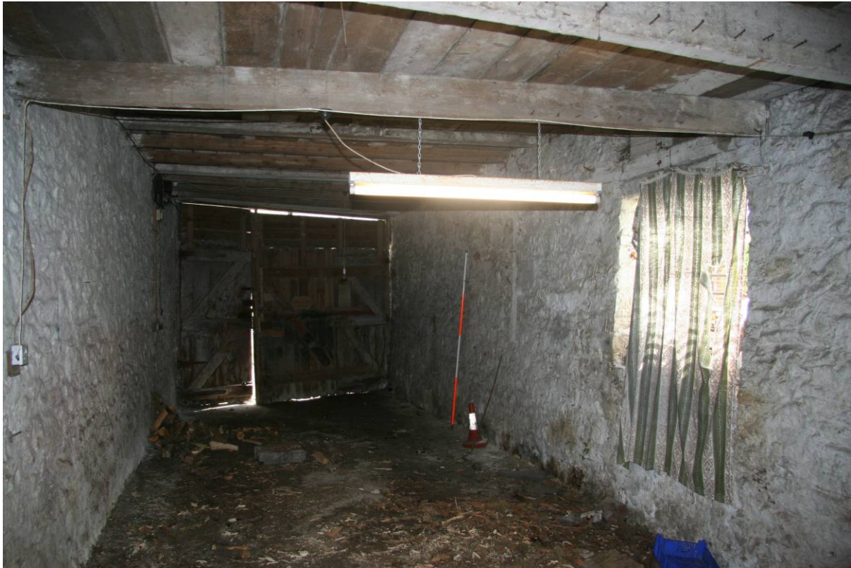
Fig 16 Interior of the eastern room, looking E towards the main doorway A blocked original window opening is located to the right of the ranging pole. The loft floor joists and planking are late 20 th century
