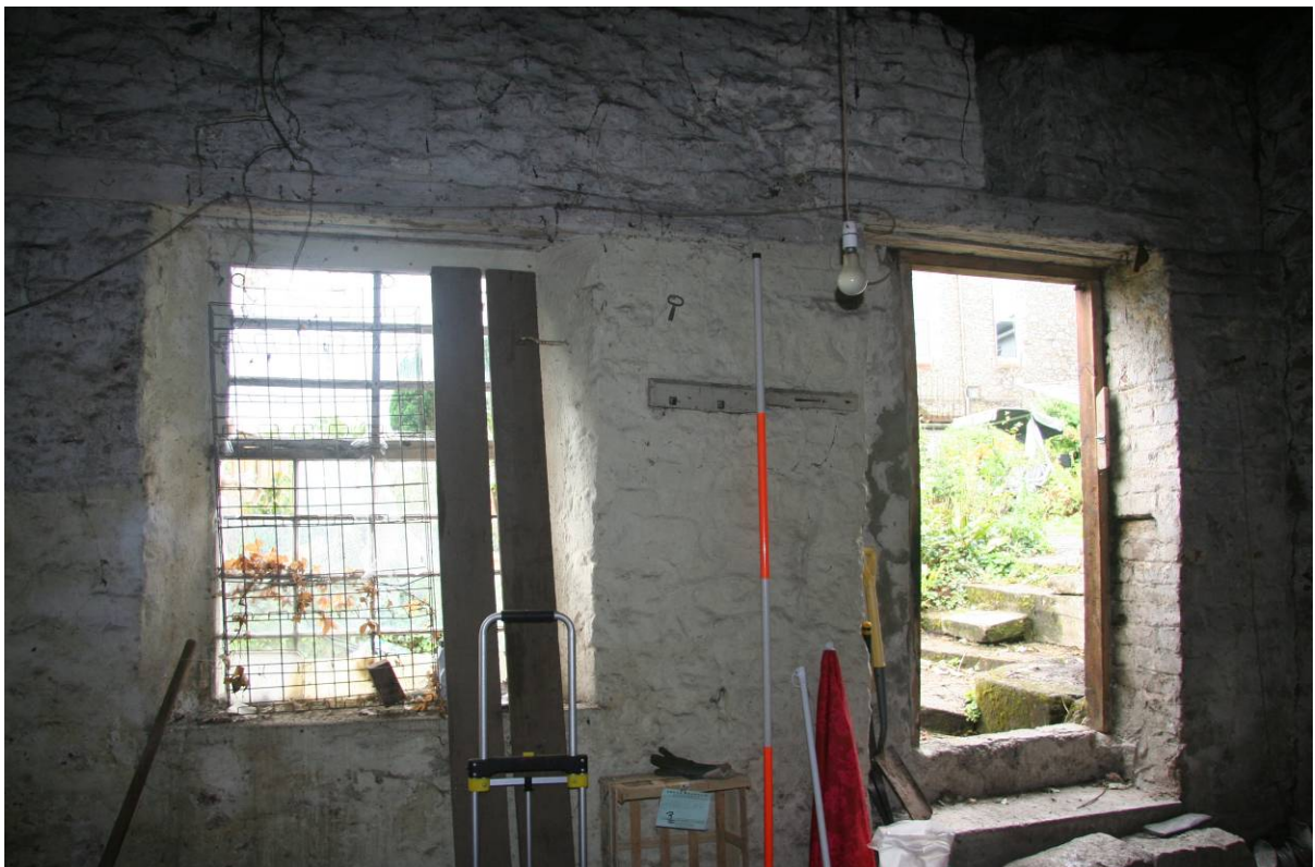
Fig 13 Interior of the west end Note the doorway, which has been reduced in width and its threshold raised, also the ventilation slit above
