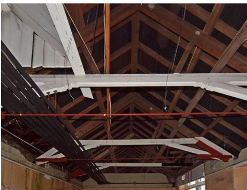
Fig 34: Room 2 roof structure
