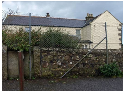
Fig 24: Blocked gate from east side of playground to school master/mistress's house 'Shalom'
