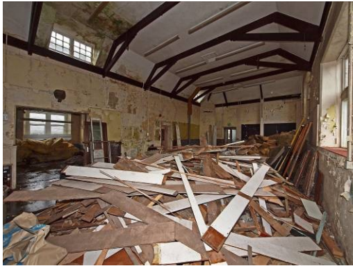
Fig 49: Room 5 looking south-west
