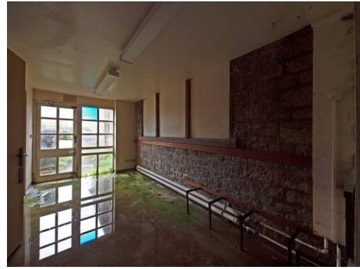
Fig 58: Room 7 looking south-east
