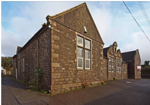
Fig 13: South and west elevations of school
