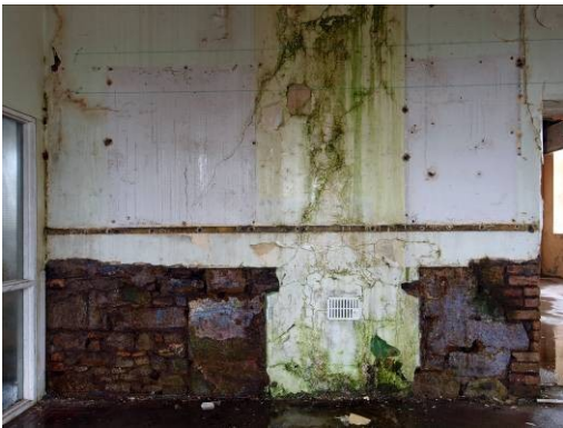
Fig 27: Blocked inserted fireplace in east wall of room 1
