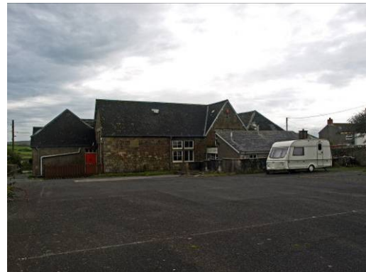
Fig 17: North (rear) elevation of school
