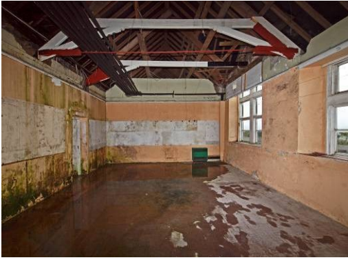
Fig 31: Room 2 looking east
