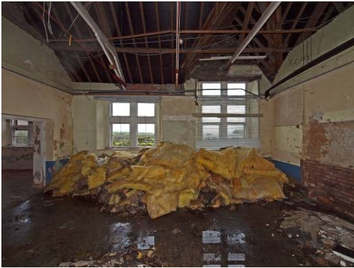
Fig 37: Room 3 looking south
