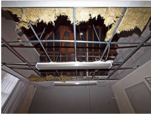
Fig 56: Room 6 roof structure
