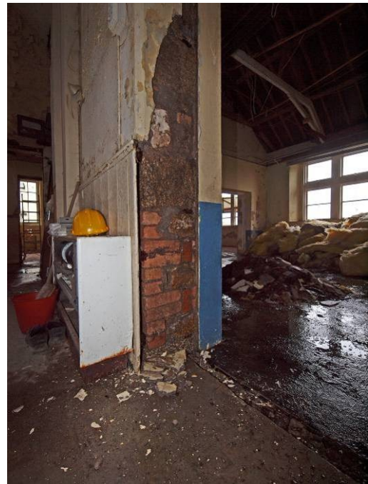
Fig 54: Room 5/3 looking south-east showing evidence for former window to side of door opening
