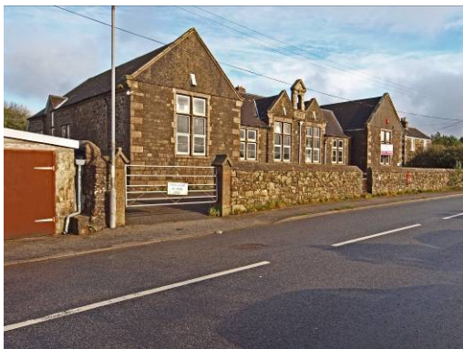
Fig 10: South (frontage) elevation of school
