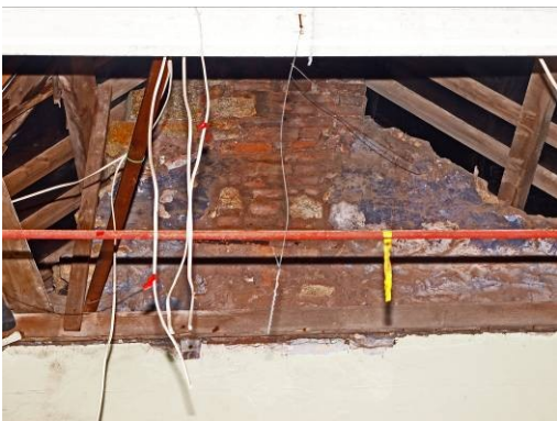
Fig 39: Room 3 remains of chimney in east gable end
