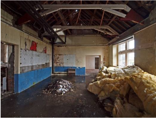
Fig 36: Room 3 looking east
