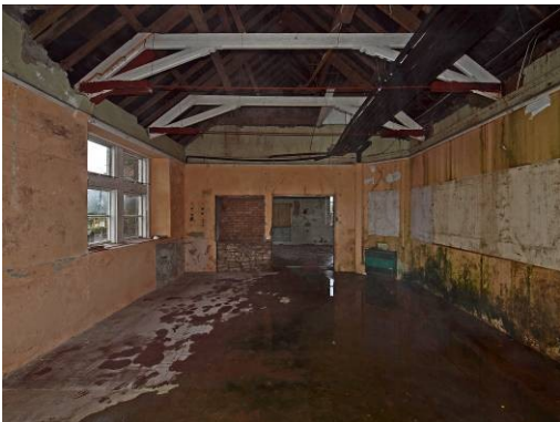
Fig 33: Room 2 looking west
