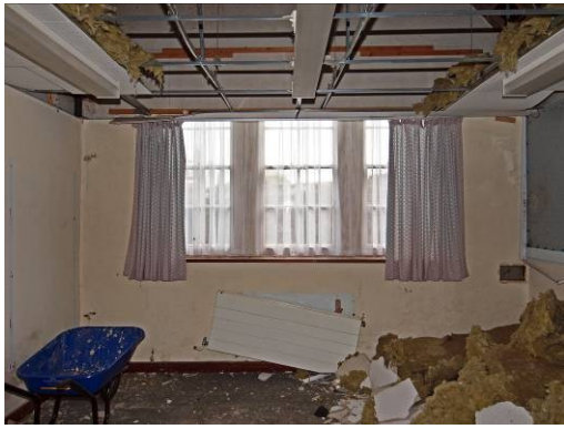
Fig 55: Room 6 looking west
