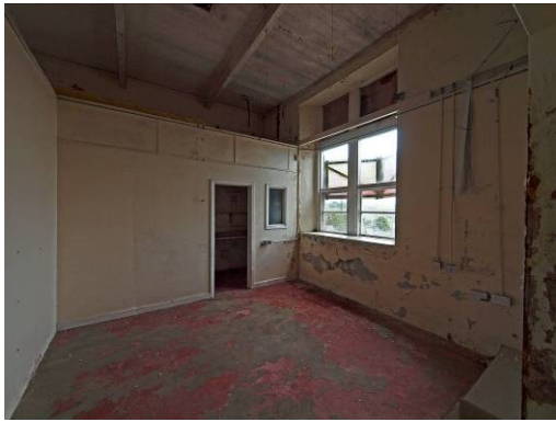
Fig 40: Room 4a looking south-east
