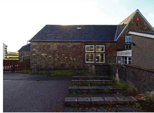
Fig 18: North (rear) elevation of school
