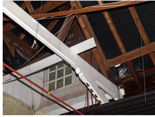
Fig 35: Room 2 dormer in north-west corner
