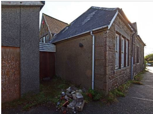
Fig 14: West and north elevations of school
