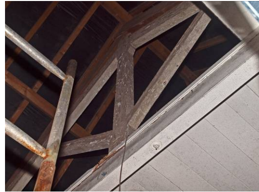
Fig 44: Room 4 roof structure
