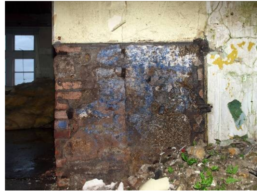
Fig 52: Room 5 south wall, blocked original rear door to 1842 building
