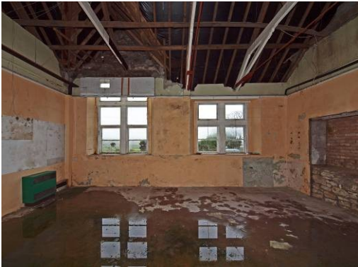
Fig 32: Room 2 looking south
