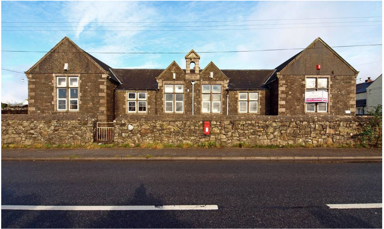
Fig 9: South (frontage) elevation of school
