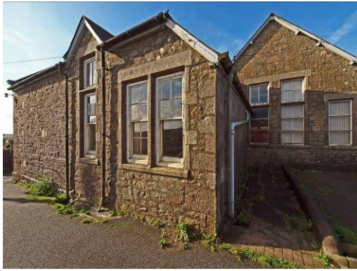
Fig 20: East elevation of school
