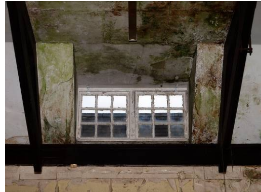
Fig 53: Room 5 dormer in centre of south wall
