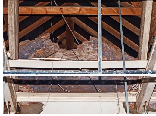
Fig 29: Top of 1842 gable end looking east from room 1
