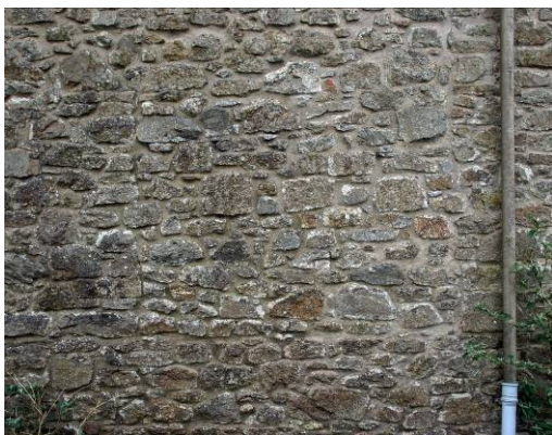
Fig 15: Blocked window at south end of west elevation
