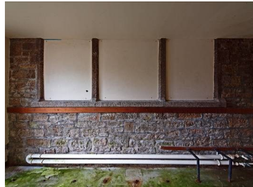
Fig 59: Room 7 blocked hall window in south wall
