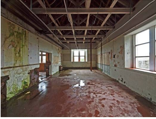
Fig 25: Room 1 looking south
