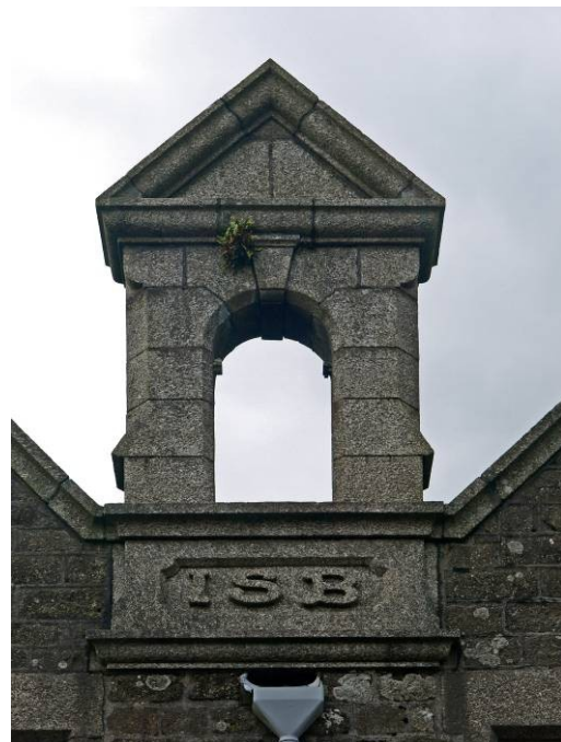
Fig 11: Bell-cote at centre of south elevation
