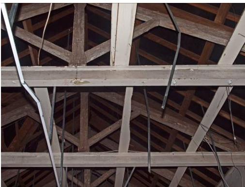
Fig 28: Room 1 roof structure
