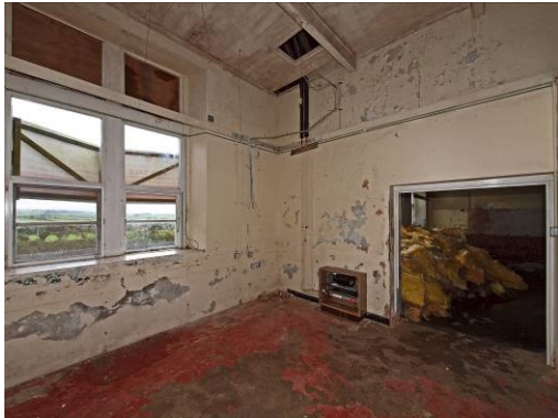
Fig 41: Room 4a looking south-west
