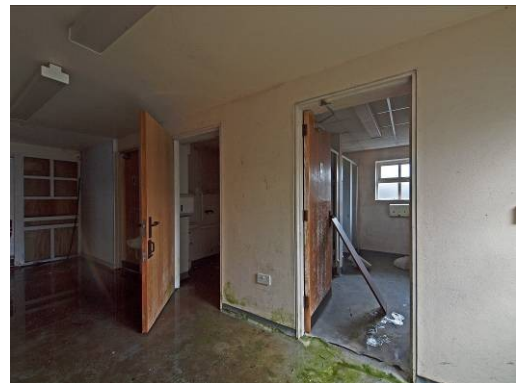
Fig 60: Room 7 looking north-west to toilet block
