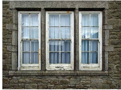
Fig 16: Window at east end of west elevation
