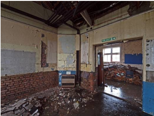
Fig 38: Room 3 looking north-west
