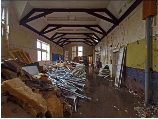
Fig 48: Room 5 looking east
