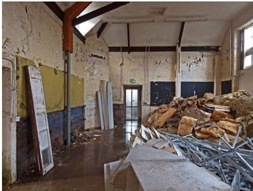
Fig 50: Room 5 looking west
