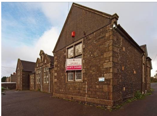
Fig 22: South and east elevations of school
