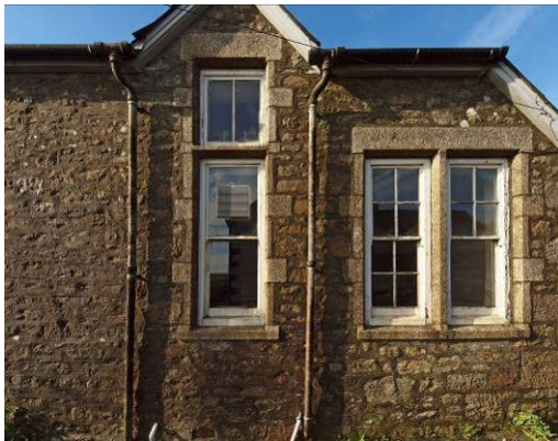
Fig 21: East elevation of school
