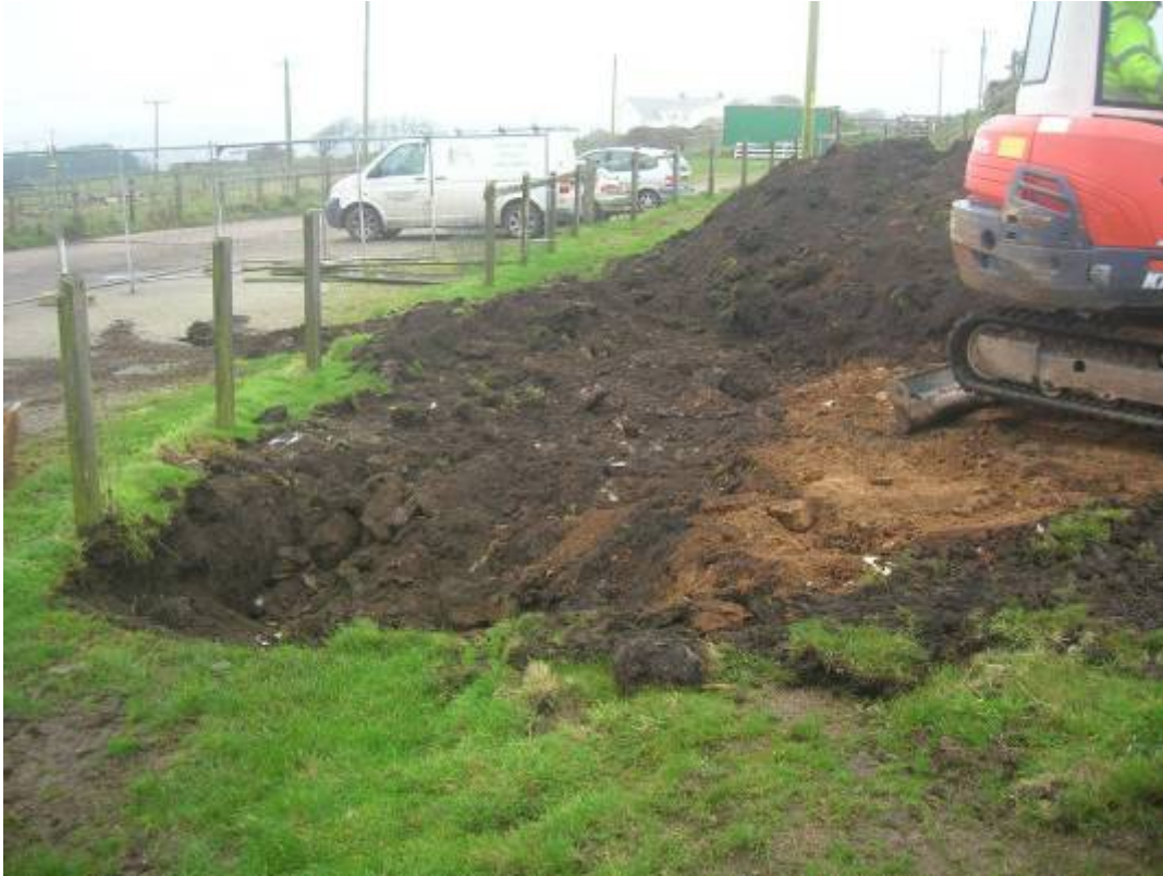
Fig 11 Line of trenched feature [9] as first exposed. View looking northeast.
