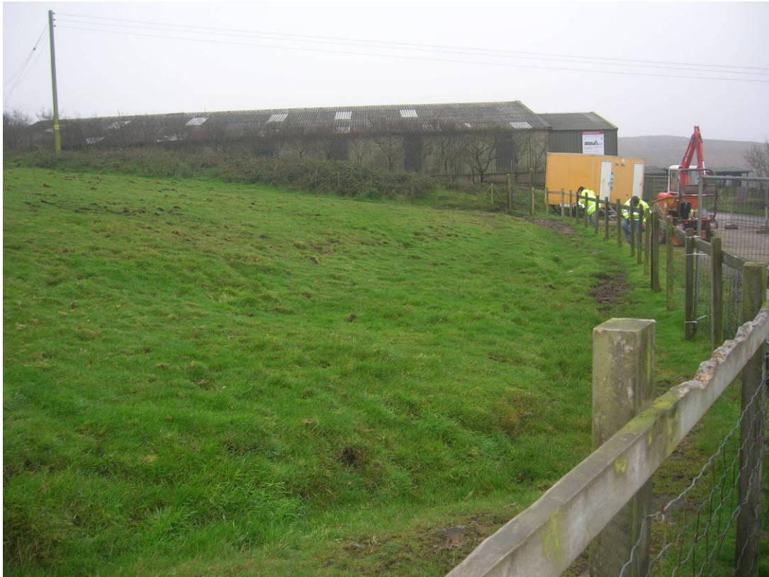
Fig 7 General view of site prior to commencement of work looking northwest.
