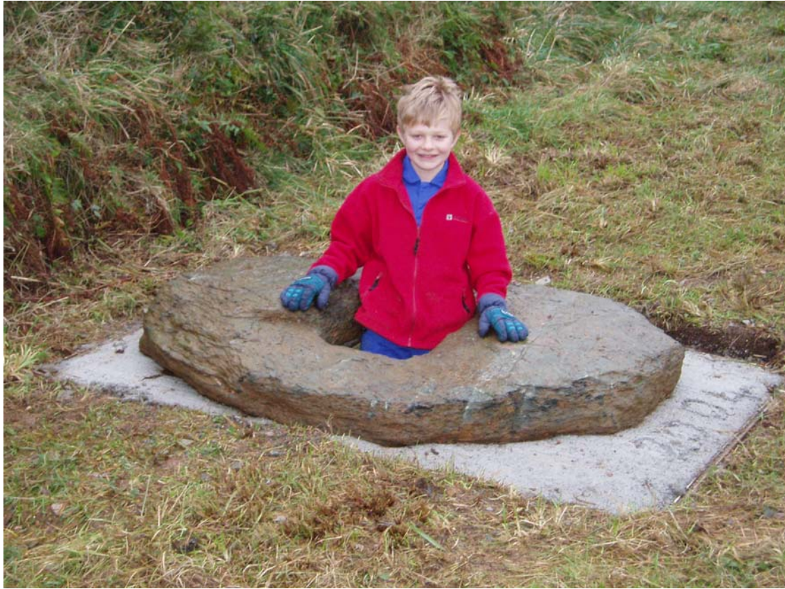
Fig 11 The original base, restored on a new concrete foundation
