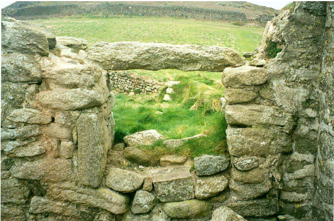
Fig 16. The small window in the eastern wall of St. Helen's Chapel before works, showing the lost inner lintel. HE Digital Image Archive.
