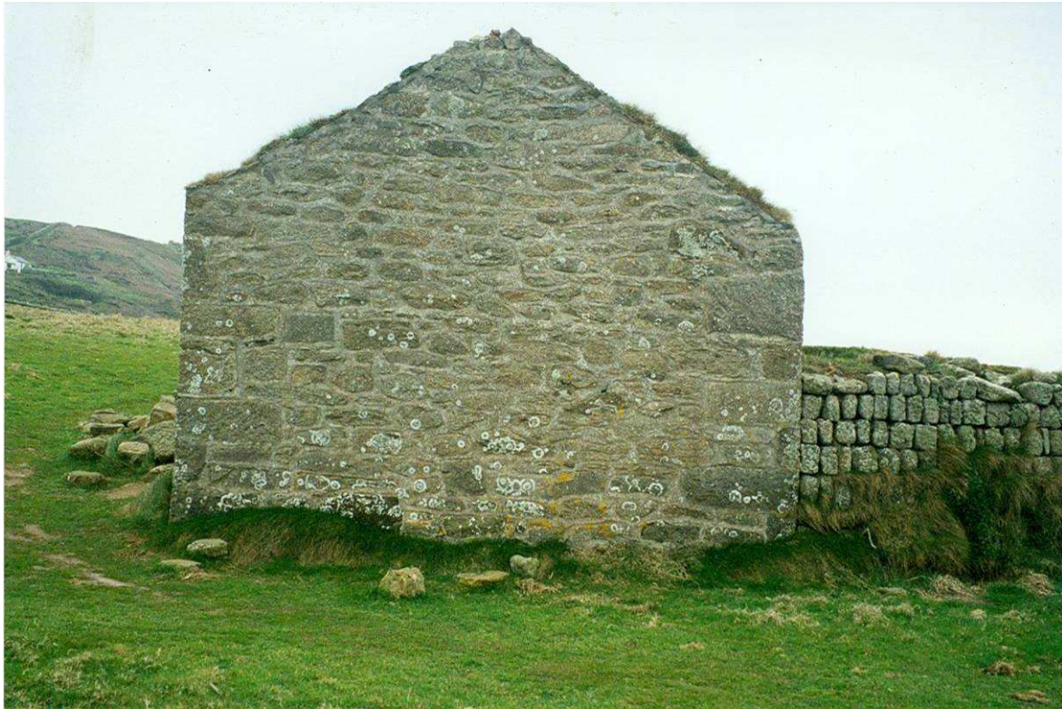
Fig 14. St. Helen's Chapel from the north before works, showing the markedly different style of stonework used in the construction of this wall. HE Digital Image Archive.
