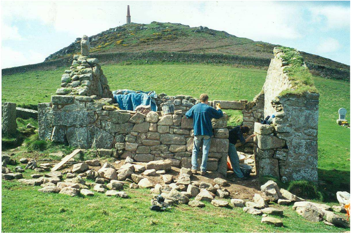
Fig 20. The reconstruction of the collapsed section of the eastern wall approaching completion. HE Digital Image Archive.
