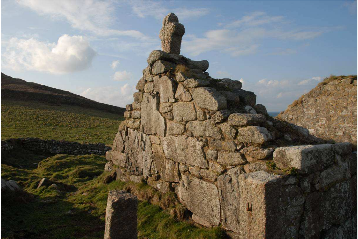
Fig 24. The southern wall of St. Helen's Chapel from the south-east in late 2009. HE Digital Image Archive.
