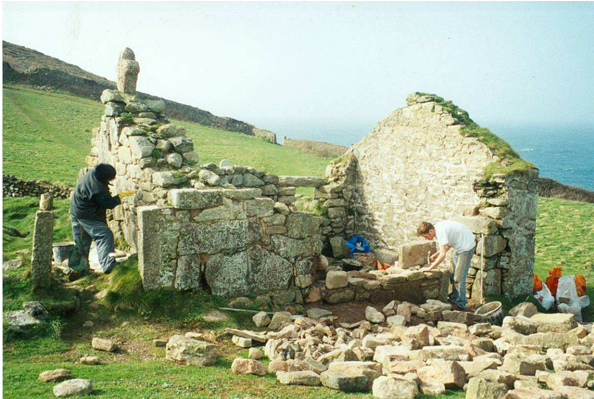
Fig 18. An early stage during the conservation works. The foundation courses of the collapsed walling have been reconstructed, whilst repointing is under way on the southern wall. HE Digital Image Archive.
