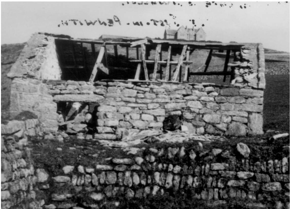
Fig 9. A view of the Chapel from the west, again probably taken during the early 1960s showing the severe deterioration of the roof structure at that date. NT Collection.
