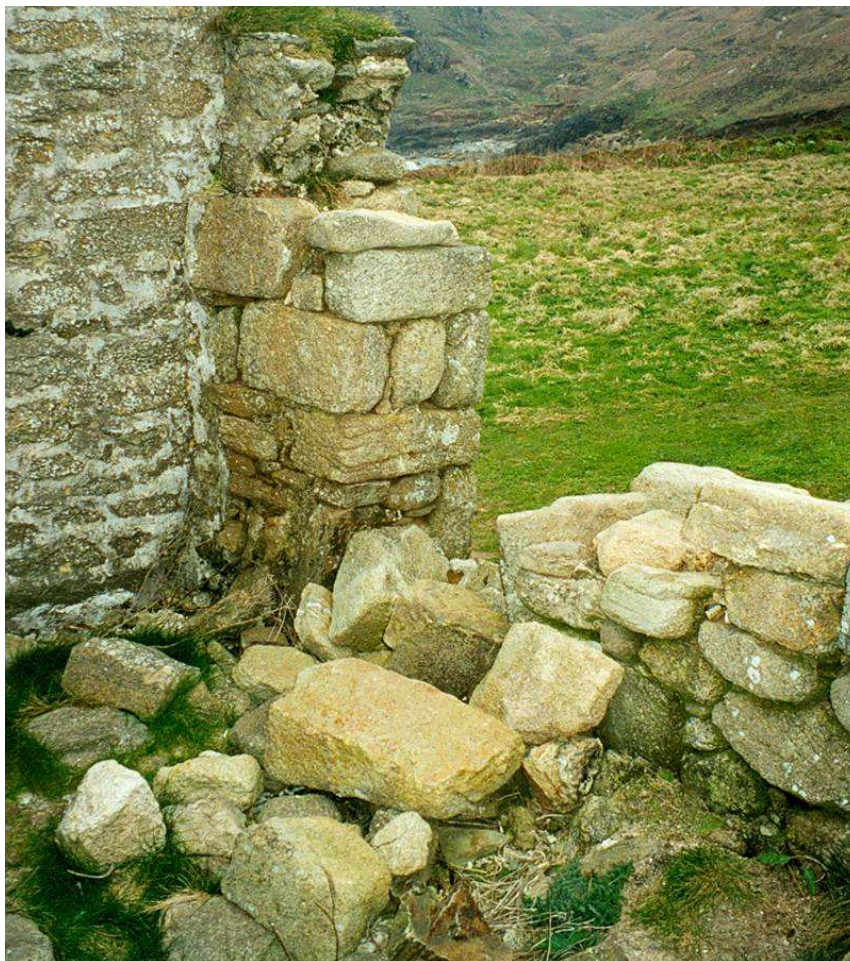
Fig 16. The small window in the eastern wall of St. Helen's Chapel before works, showing the lost inner lintel. HE Digital Image Archive.
