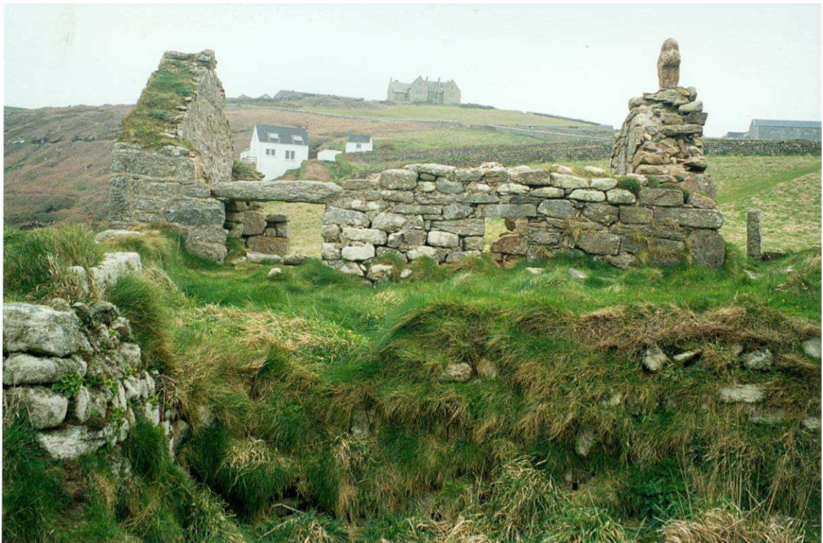
Fig 13. St. Helen's Chapel from the west before works, with the dividing enclosure wall in the foreground. HE Digital Image Archive.
