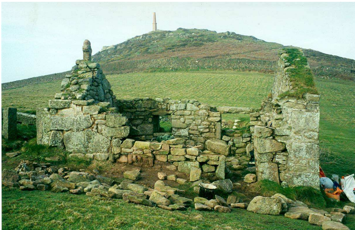
Fig 19. A later stage during the reconstruction of the eastern wall and doorway reveal. HE Digital Image Archive.
