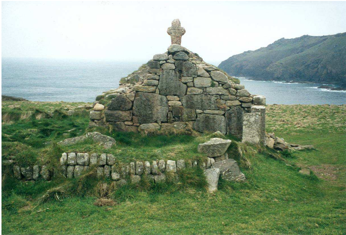
Fig 10. St. Helen's Chapel from the south prior to works showing the massive stones used in the construction of this wall and the cross re-erected on its gable. HE Digital Image Archive.
