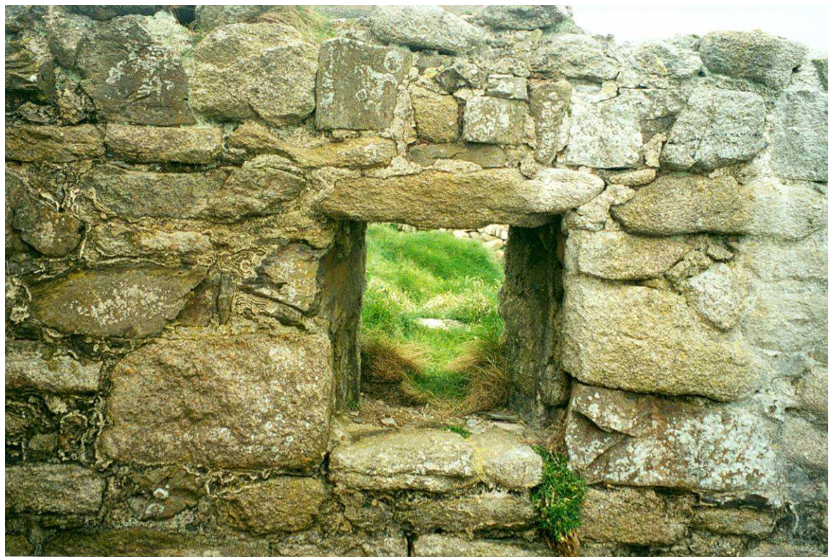
Fig 21. The masonry over the external face of the window in the western wall. HE Digital Image Archive.
