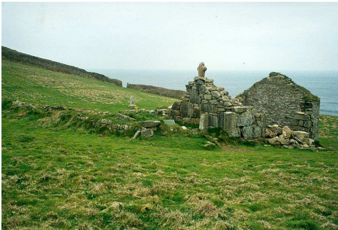
Fig 11. St. Helen's Chapel from the south-east prior to works, showing the collapsed masonry adjacent to the doorway, and the low walls forming the enclosures to the west. HE Digital Image Archive.
