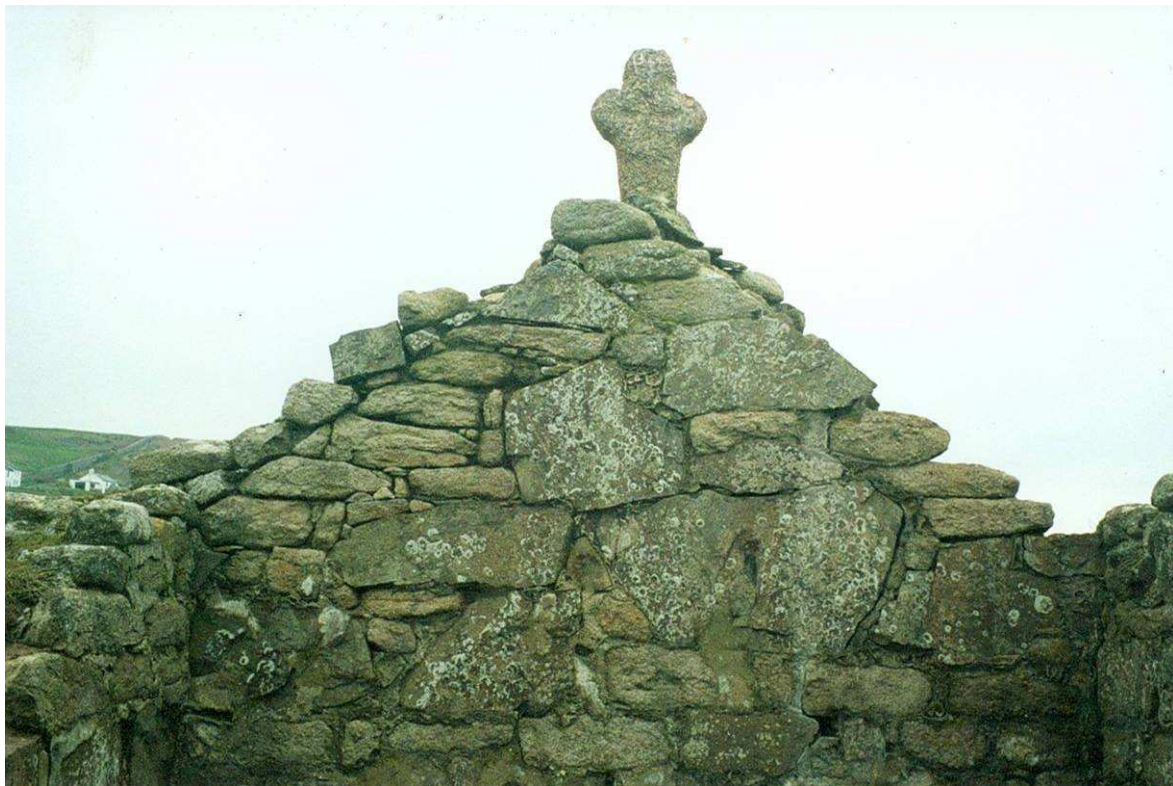
Fig 15. The internal elevation of the southern wall of St. Helen's Chapel before works, showing some evidence for the original gable line having been raised in smaller stone (left). HE Digital Image Archive.
