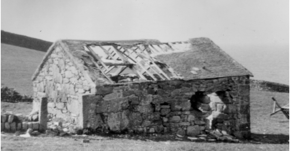
Fig 8. A view of the Chapel from the south-east, of unknown date but probably the early 1960s, when the structure still retained some of its roof, and when the area of the wall adjacent to the door had begun to collapse. NT Collection.
