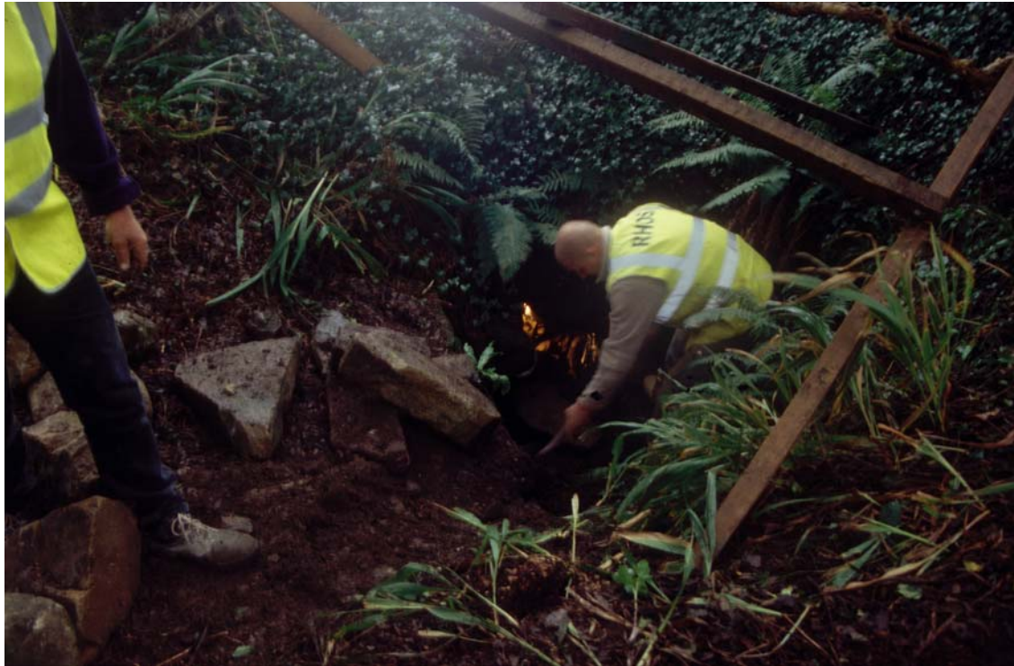
Fig 11 Blocking in progress (photo HES GCS 34698)
