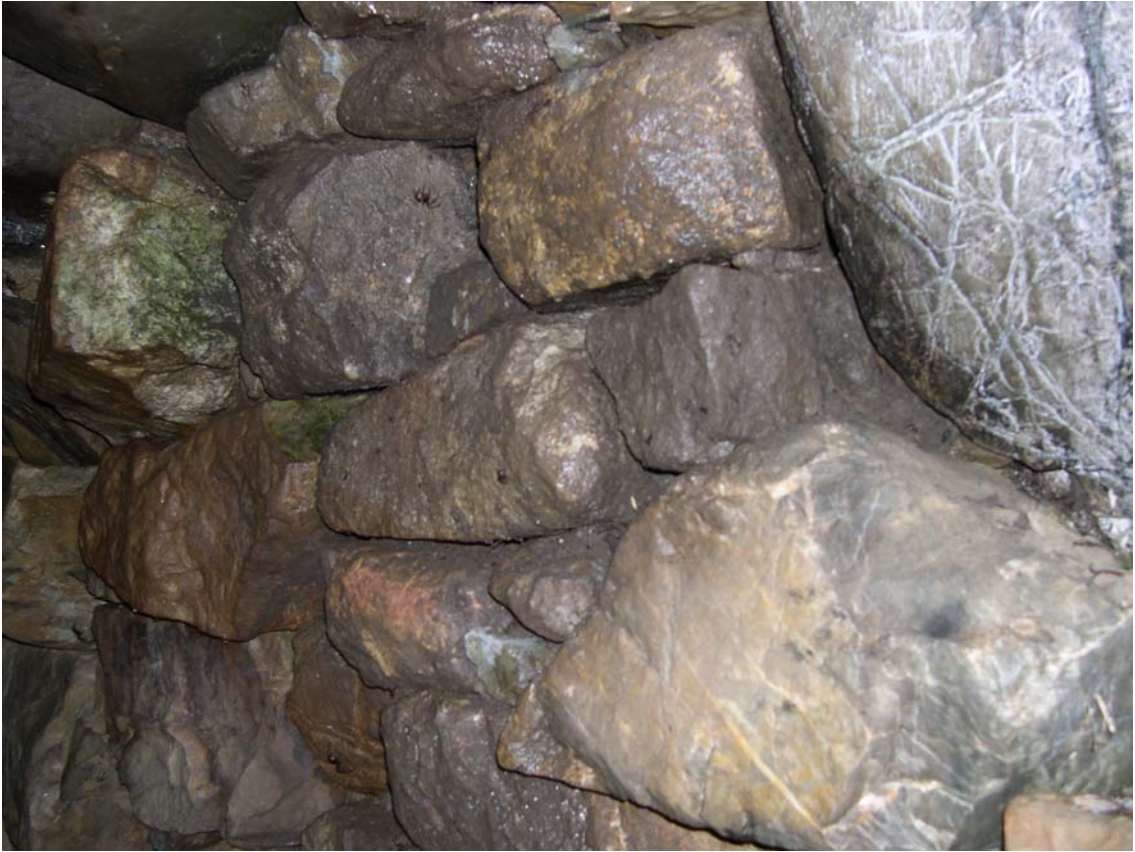
Fig 13 The stone blocking from inside the creep (photo HES GDP /0002)
