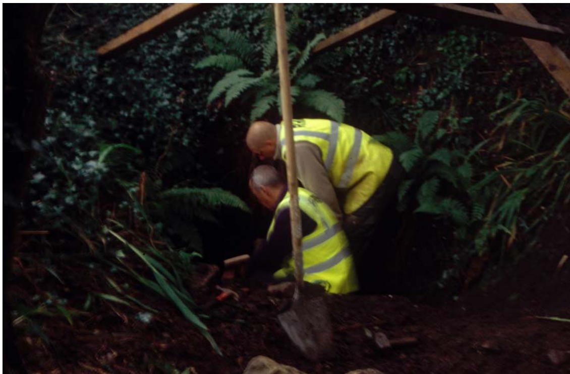
Fig 12 Blocking in progress (photo HES GCS 34696)
