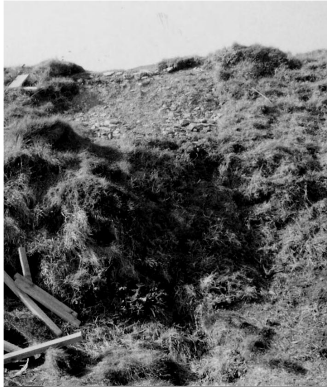
Figs. 13 and 14 Infilling of the rampart 2 in progress. Note how vegetation removed from the hollow has been replaced at the base of the scar.
