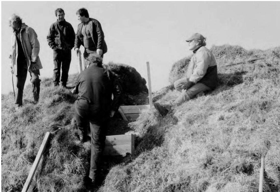
Fig. 12 Construction of wooden revetments into scar on rampart 2.
