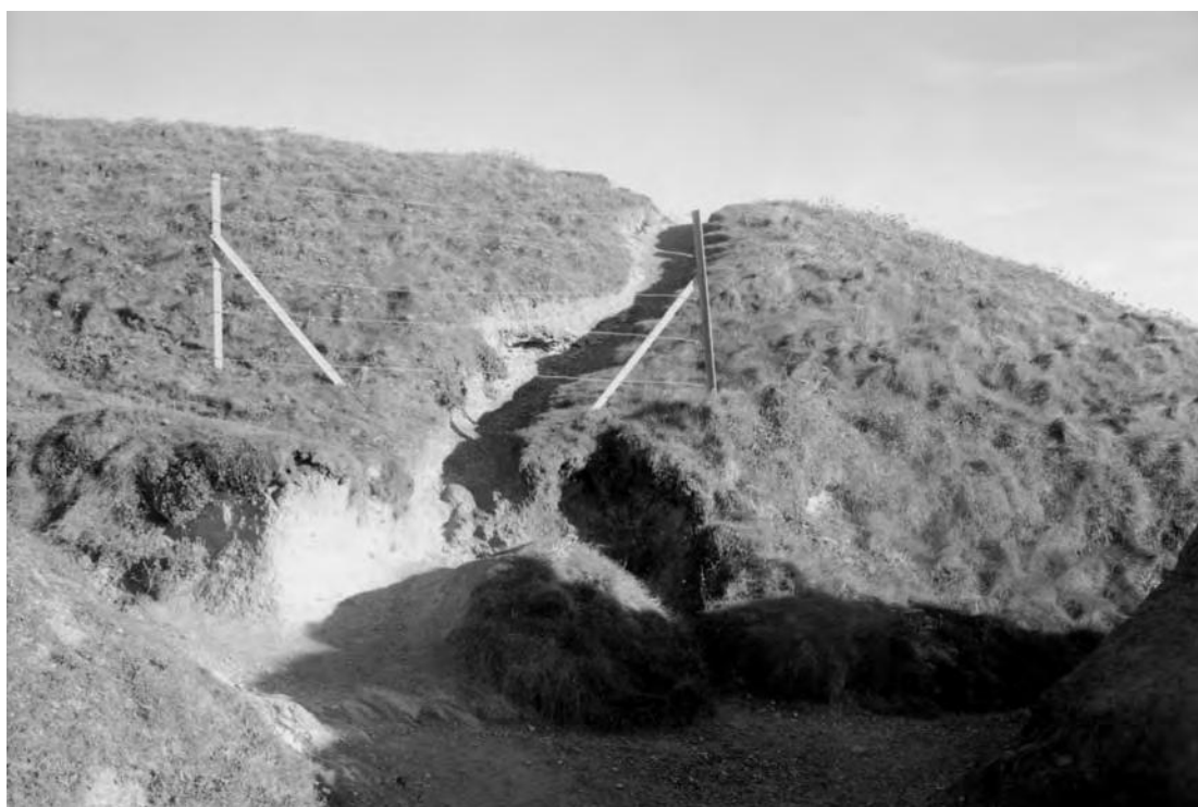
Figs. 17 Eroded scar across rampart 4, prior to works commencing. Photograph taken from the west.
