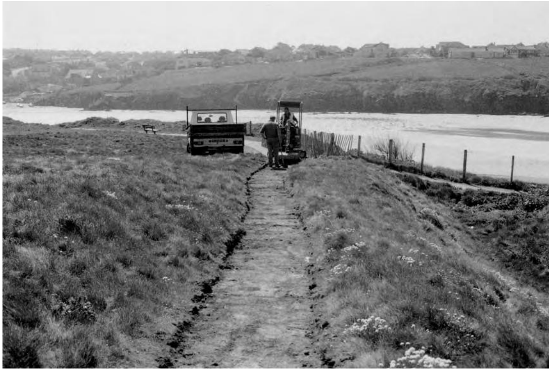
Fig. 31 Construction of new path to east of ramparts 3-5.
