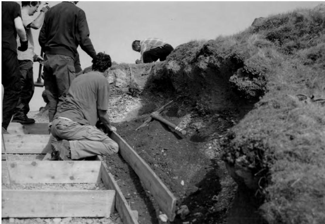
Fig. 28 Construction of steps through rampart 4.
