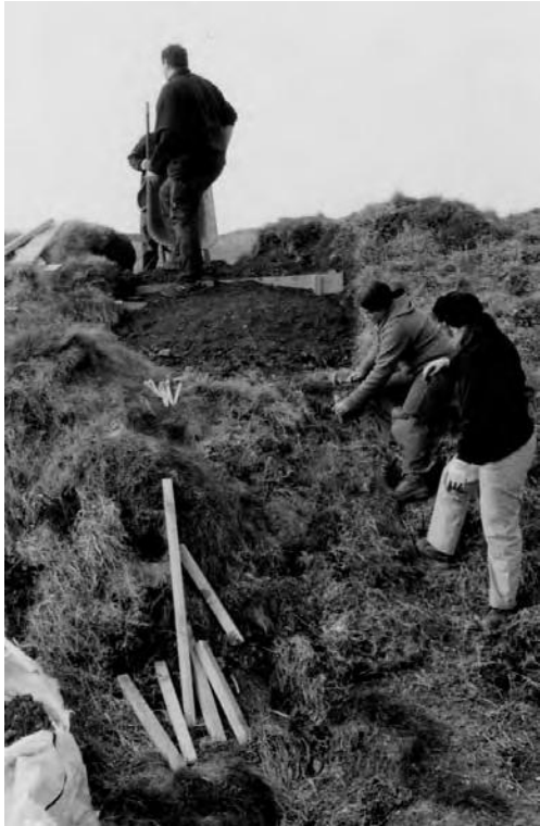
Figs. 13 and 14 Infilling of the rampart 2 in progress. Note how vegetation removed from the hollow has been replaced at the base of the scar.
