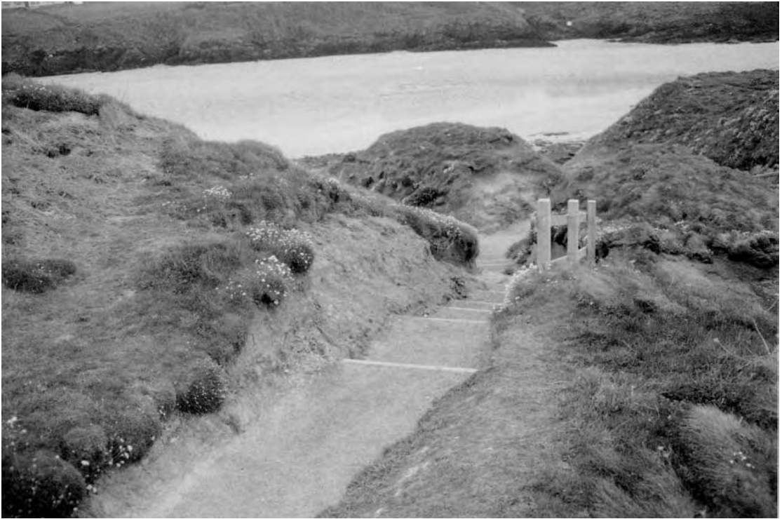
Fig. 29 Steps through rampart 4. Note infilled hollow to the left and safety fence to right of path.
