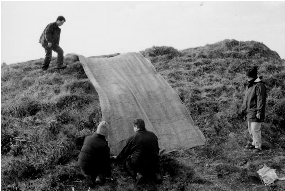
Fig. 15 Eroded scar following conservation, covered with bessian matting.
