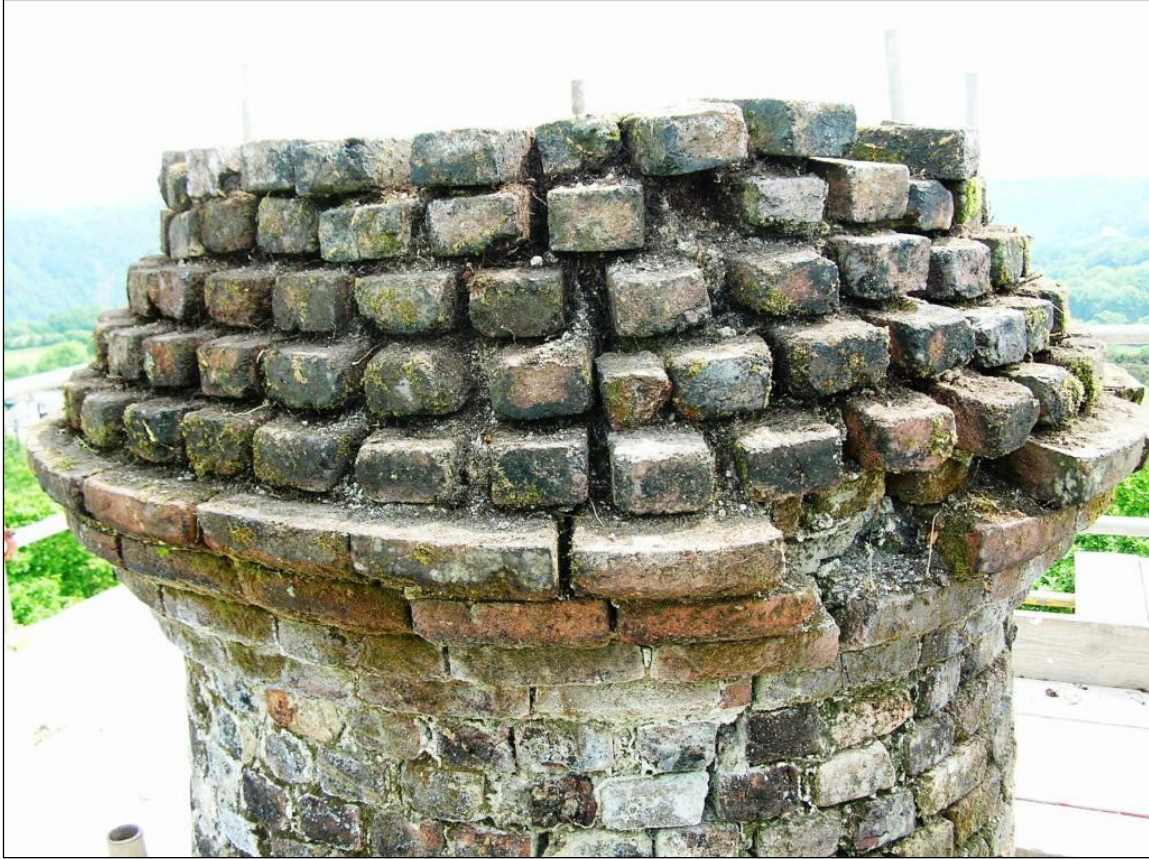
Figure 14 External view of the chimney top before works © CC HE Projects 2008
