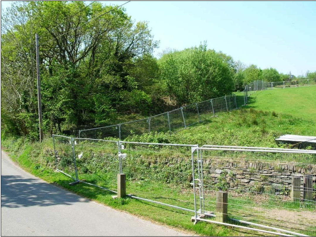
Figure 20 A view of the Tamar Valley Centre building site (from the northeast) © CC HE Projects 2008
