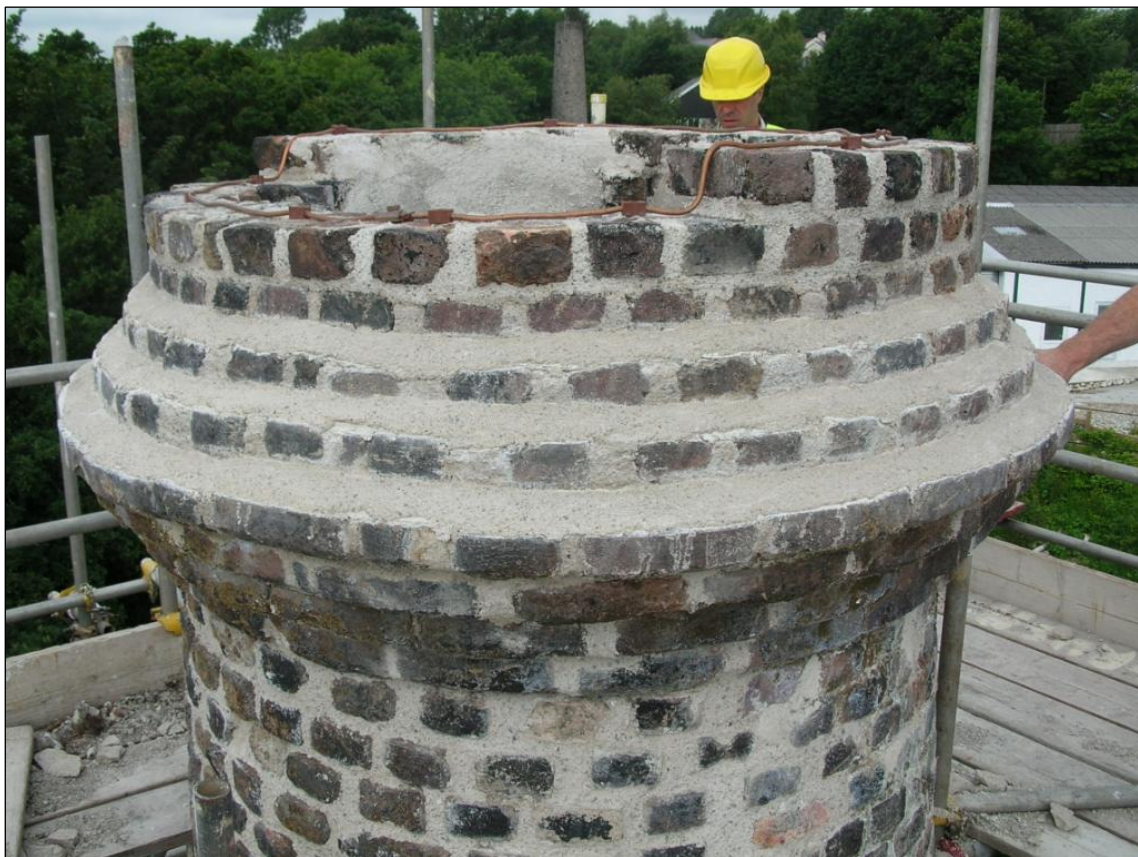
Figure 15 External view of the chimney top after works © CC HE Projects 2008
