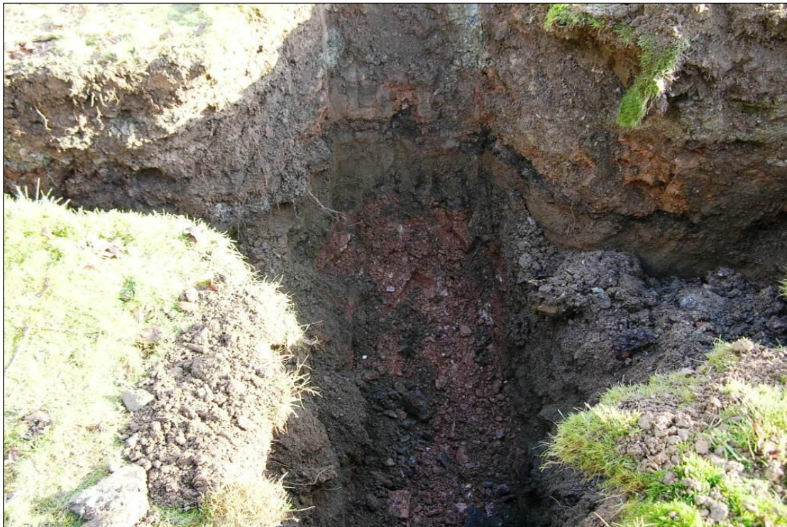
Figure 24 A view of excavated surface depression (from the north) © CC HE Projects 2009
