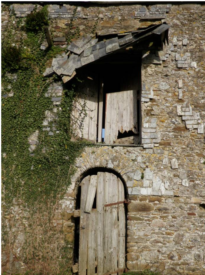
Fig 8 Exterior south elevation of central openings (ground floor cow house and first floor threshing door)
