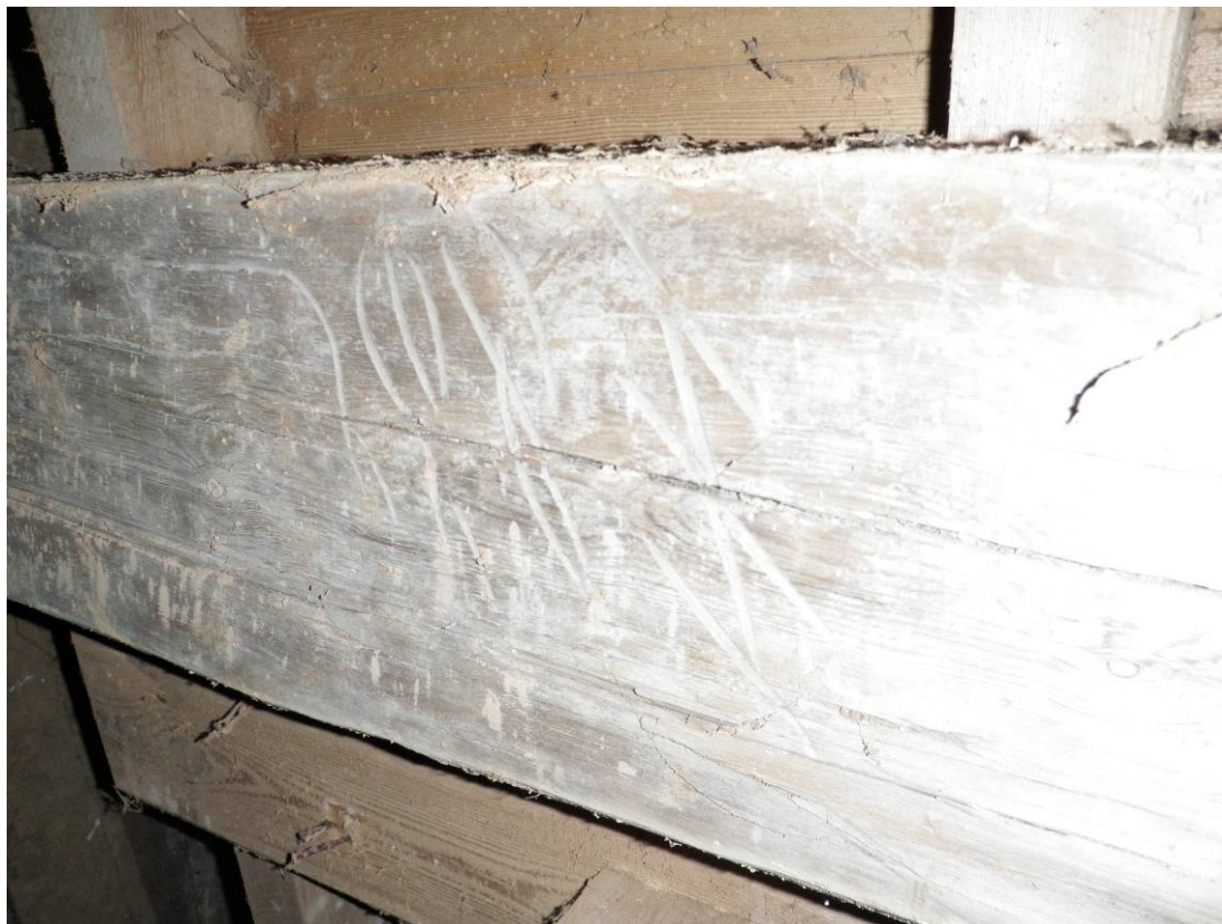
Fig 19 Carpenter's marks on joist in cow house
