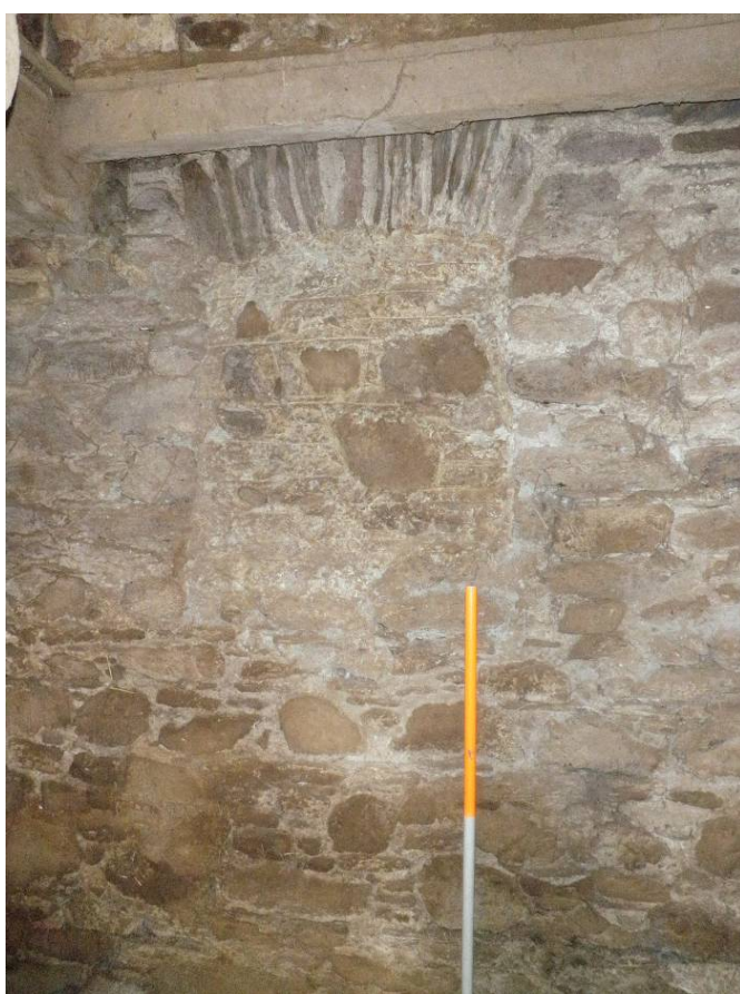
Fig 18 Blocked window in north wall of cow house
