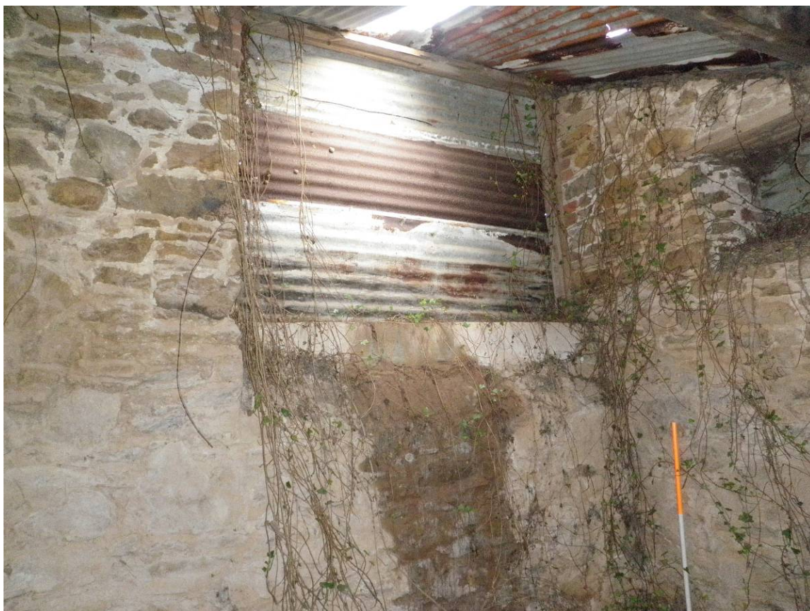
Fig 21 Interior of lean-to root house looking north-east showing chute and window openings
