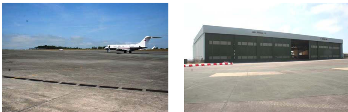
Fig 23 Apron (left) and Nimrod servicing hangar *31 (right)
