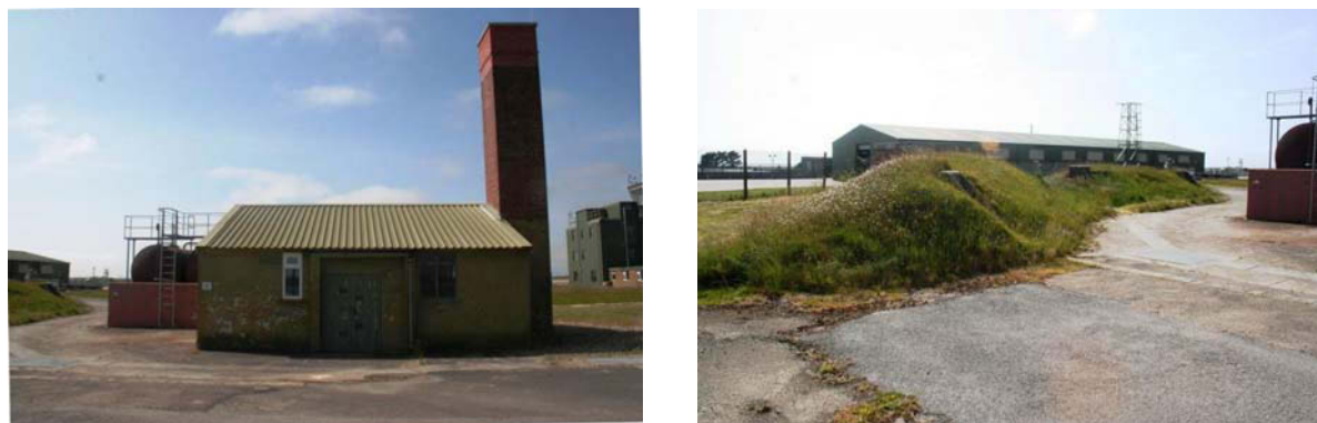
Fig 20 RAF boiler house *29 (left) and air raid shelters *19 and *20 (right)
