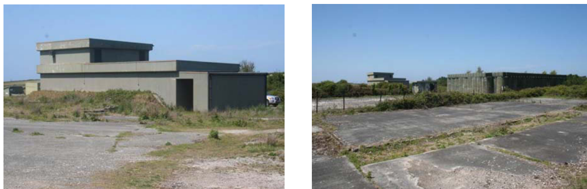
Fig 29 Communications building *84 (left) with HESCO Bastion building *90 and pill box*91 (right)
