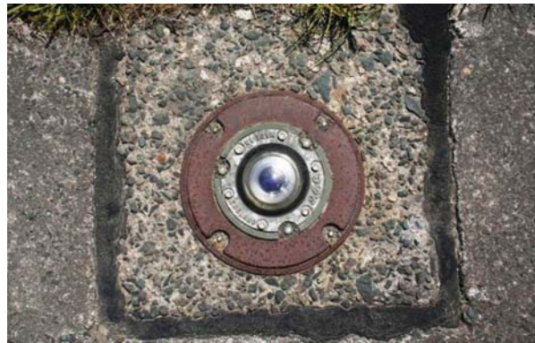
Fig 24 Apron detail: drain covers (left) and edge light (right)
