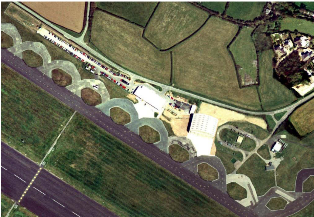
Fig 10 Excerpt from a Cornwall Council aerial photograph showing the terminal in the summer of 2000. Cornwall Council.
