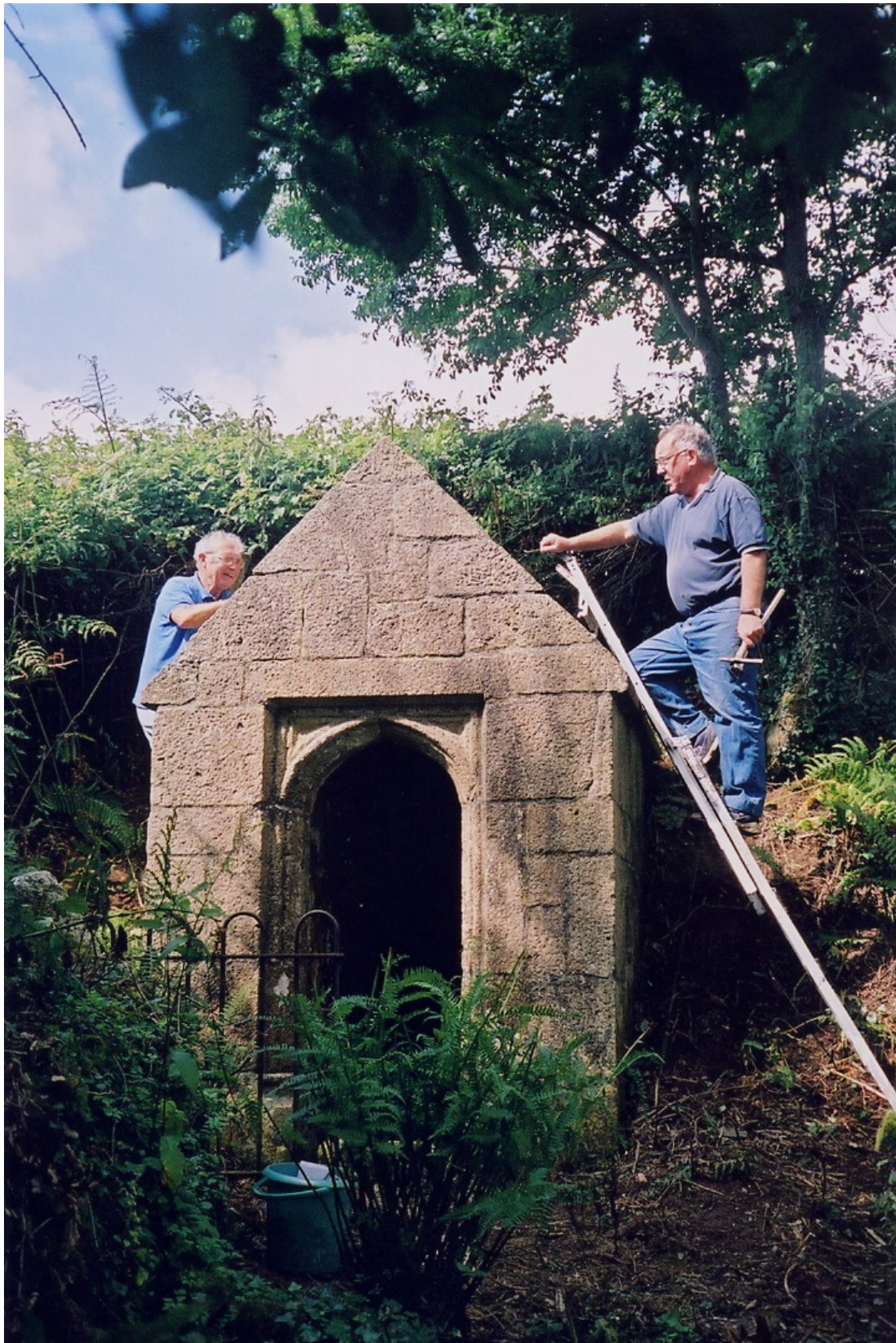
Fig 12 Graham Honey and Geoff Prettyman of Pentewan Old Cornwall Society, repointing Towan Well
