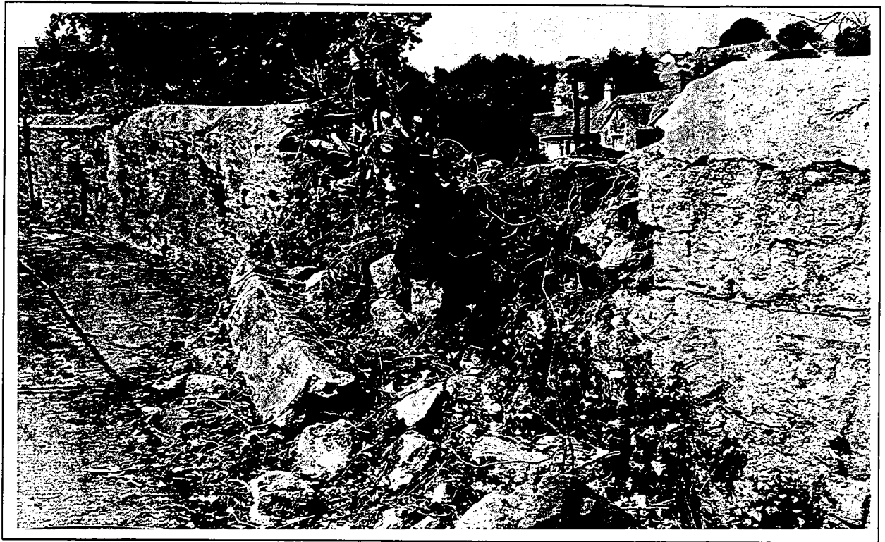
Fig. 6 Photograph of collapsed walling.
