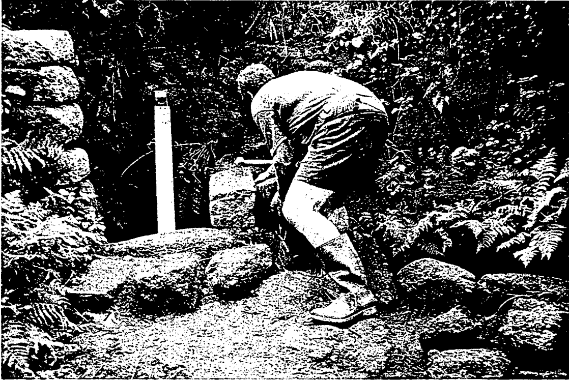
Fig 7. Work in progress
