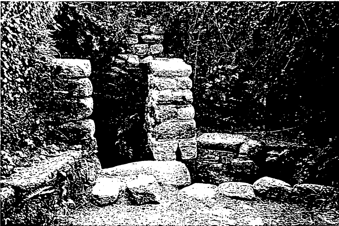
Fig 8. The repaired wall and bench
