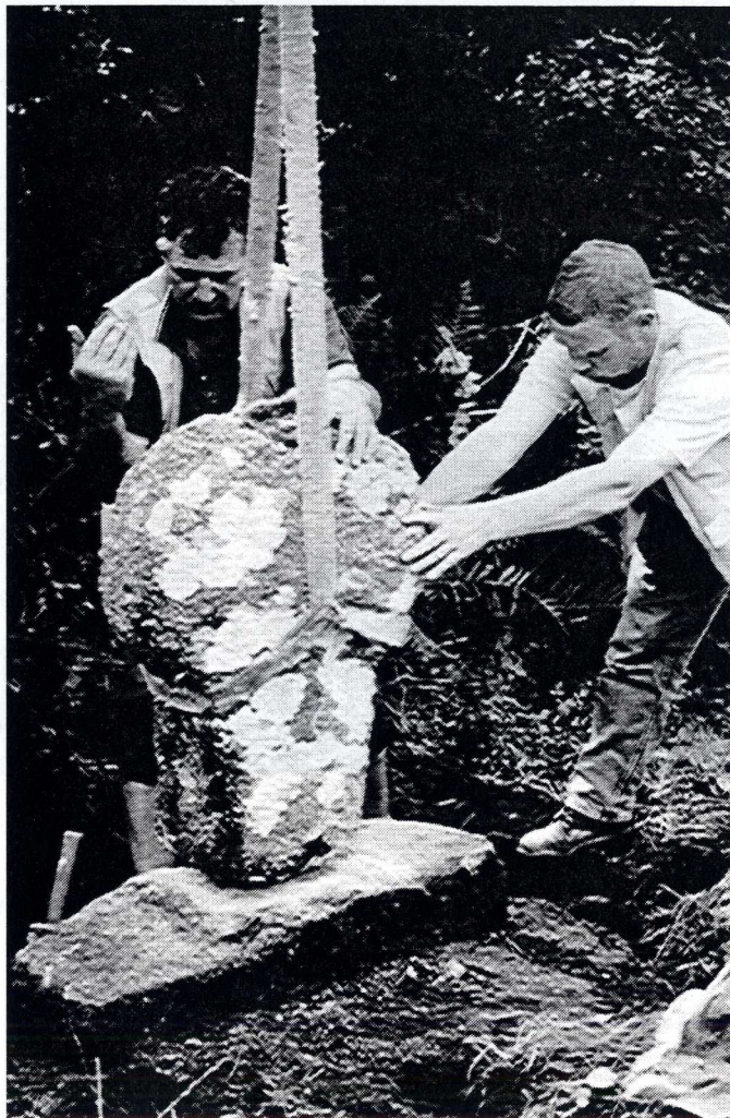
Fig 7. Restoration work in progress
