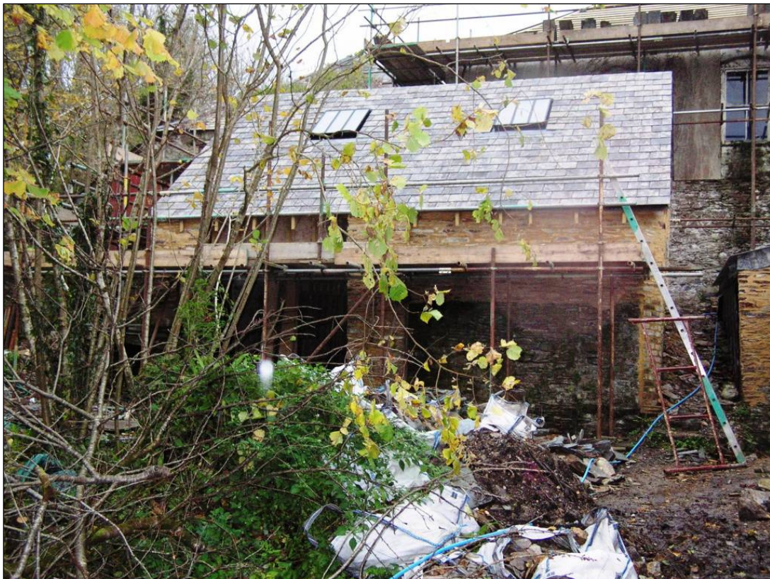
Figure 7 Photograph (from west) of Site 25 with new roof © CC HE Projects 14/11/09
