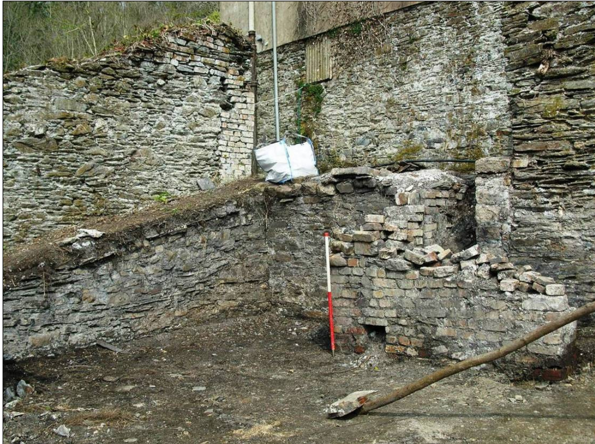
Figure 5 Photograph (from west) of the revealed brick feature (within Site 26) after clearance works (before repointing) © CC HE Projects 3/4/2009
