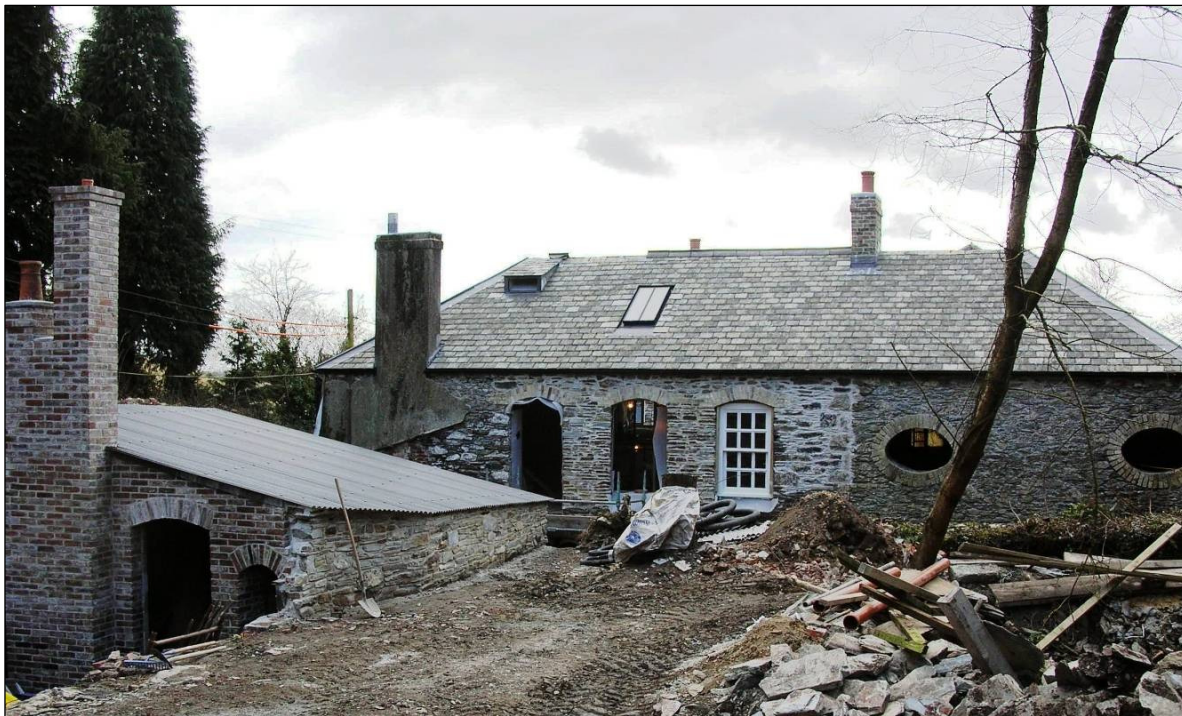
Figure 10 Photograph (from east) of Site 41 after major repair/building works
