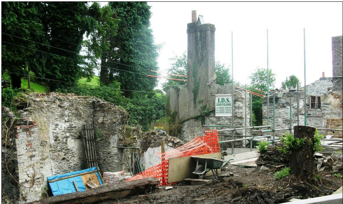
Figure 9 Photograph (from east) of Site 41 during rebuilding works
