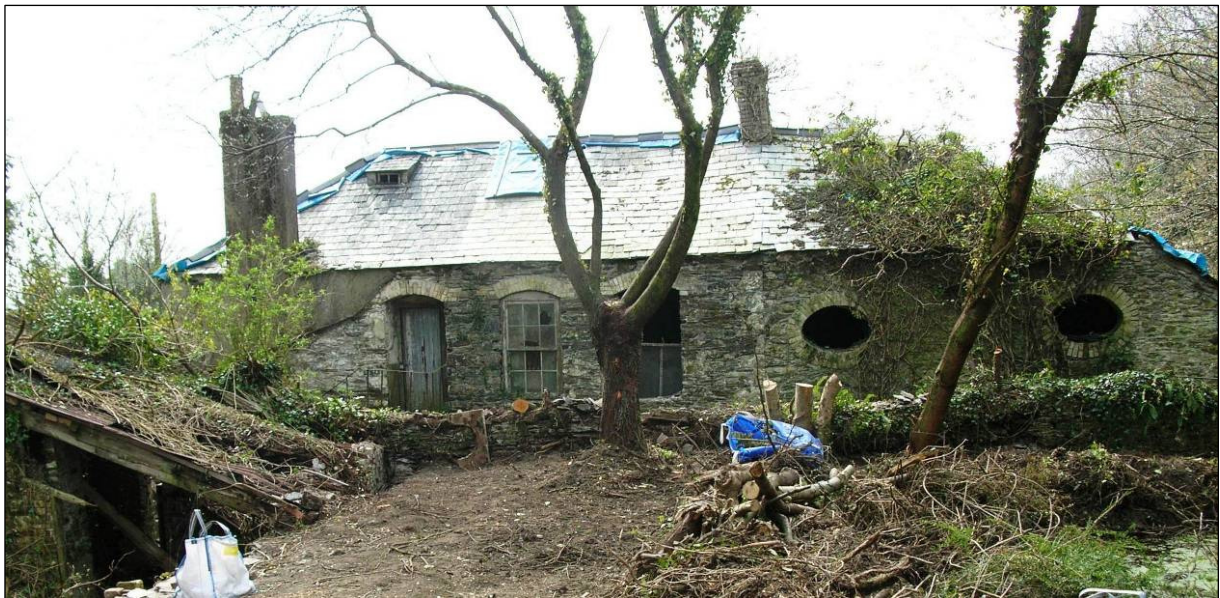
Figure 8 Photograph (from east) of Site 41 at the start of works
