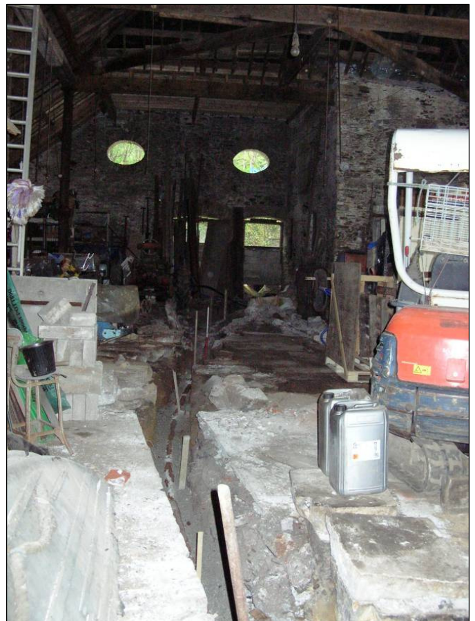
Figure 21 Photograph (looking east) of the excavated and partially infilled service trench across the former tin smelter floor © CC HE Projects 19/5/2010
