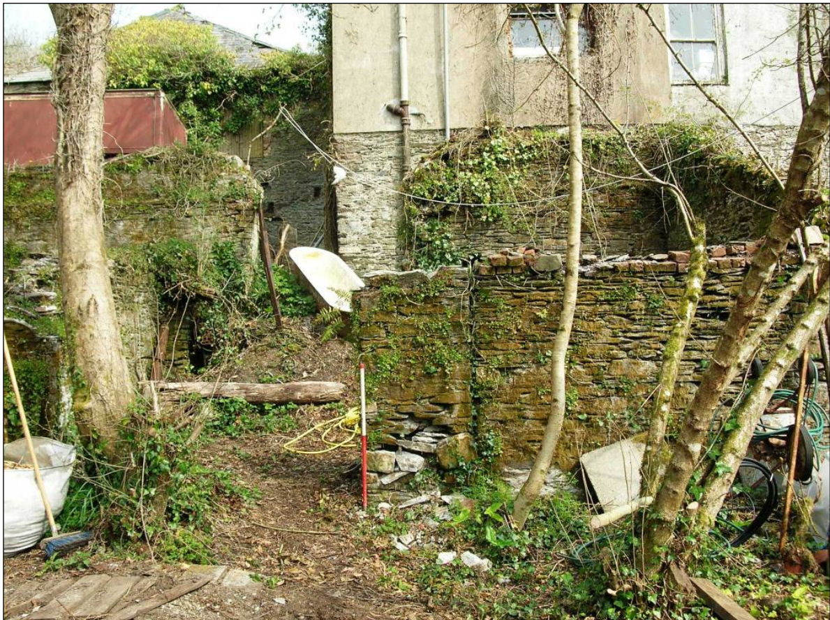
Figure 6 Photograph (from west) of Site 25 before works © CC HE Projects 3/4/09
