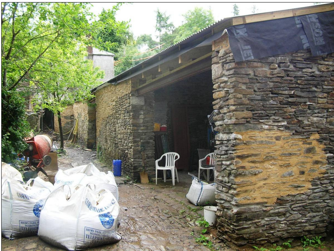
Figure 4 Photograph (from west) of the outbuildings (Sites 26 and 33) during works (repointing shown in places) © CC HE Projects 24/7/2009
