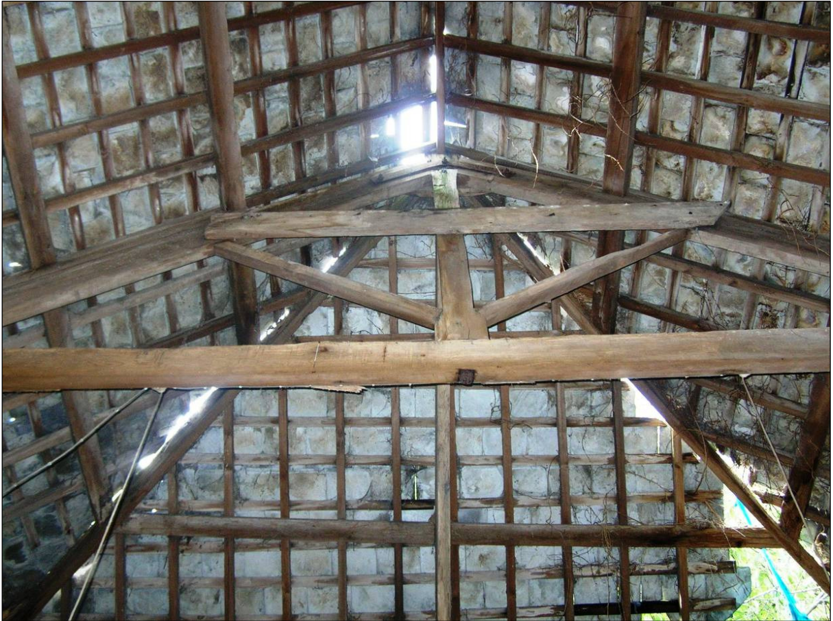
Figure 11 Photograph (looking north upwards) of Site 16 (Smelter roof 'A' frame truss) before major roof rebuilding works © CC HE Projects 14/7/2009
