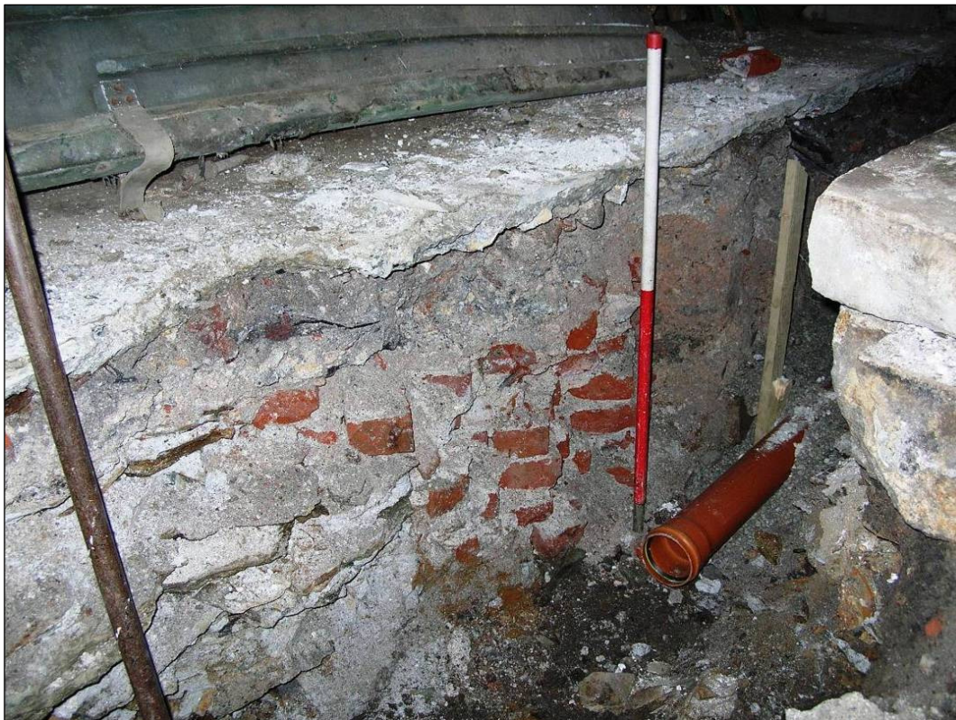
Figure 22 Photograph (looking north) of Section C © CC HE Projects 19/5/2010
