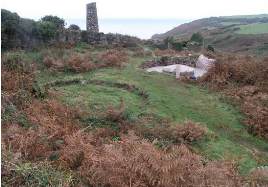
Fig 12. A view over the Porthmeor Stamps dressing floor in 2005 during the conservation of one of its buddles.
