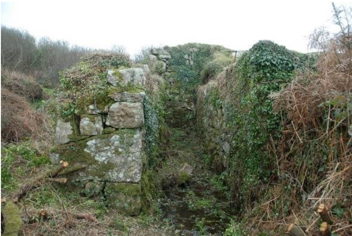
Fig 21. The interior of the wheelpit from the north following vegetation clearance.
