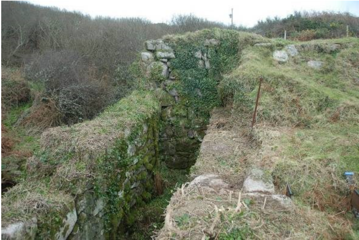
Fig 22. An overview of the wheelpit looking back towards the spalling floor. One of the stamps hold down bolts survives just to the rear of the location of the waterwheel axle.
