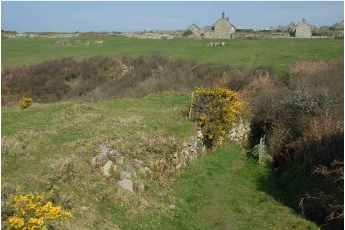
Fig 18. Looking east down the Zennor Church Path, with the spalling floor on its northern side.
