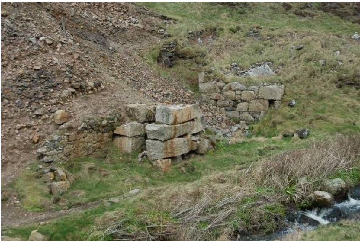
Fig 18. The angle bob loading adjacent to Engine Shaft (immediately to its right), with the remains of the pumping engine house bob wall to its right again.
