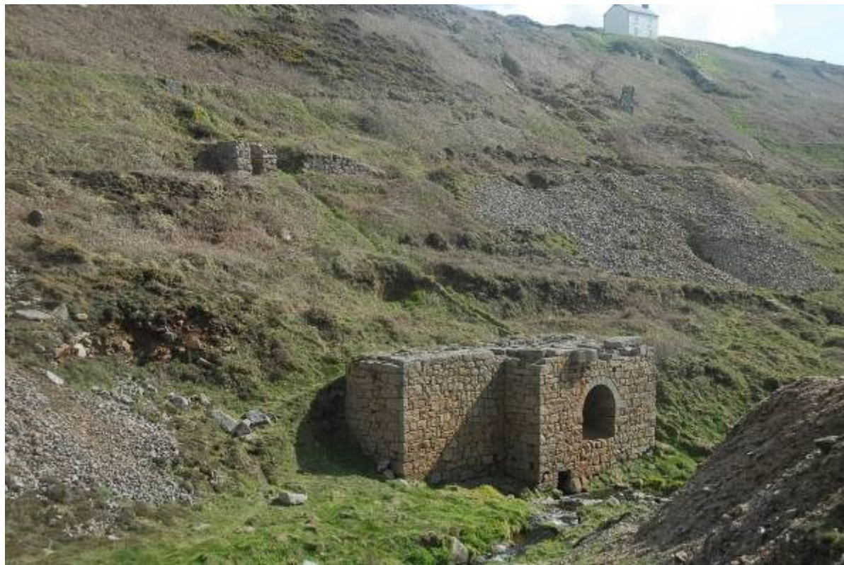
Fig 22. The free-standing pit for the Great Wheel which pumped Engine and Praze Shafts, with the pit for the winding water wheel and some of the mine leats clearly visible on the slopes above.
