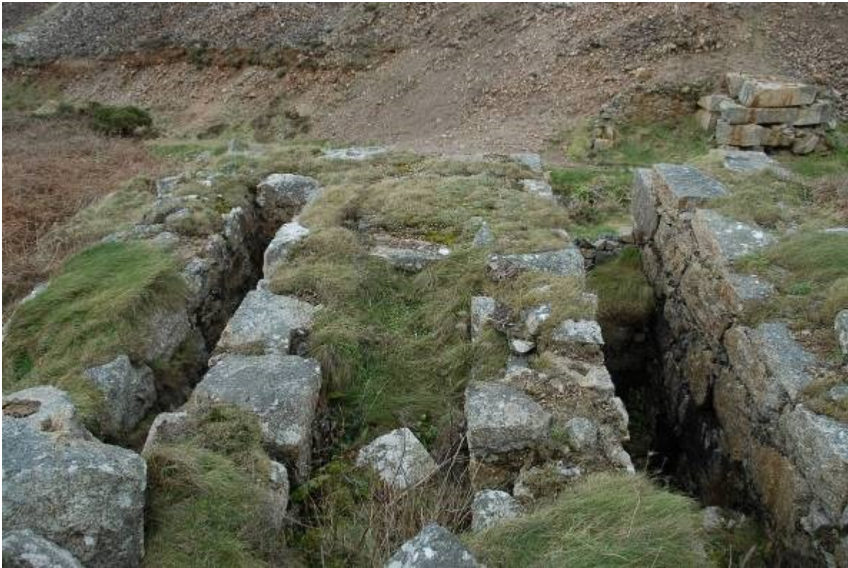
Fig 39. The paired flywheel slots and central crank slot in the loadings immediately to the north of the stamps engine house.
