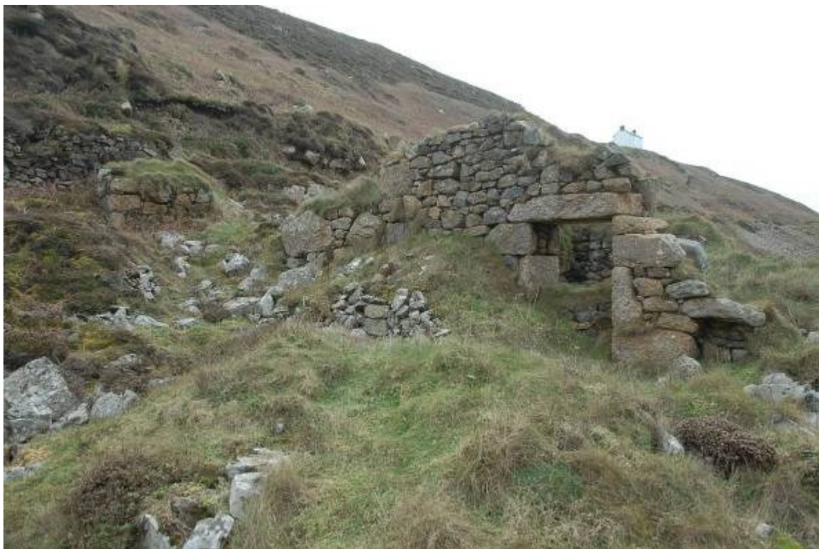
Fig 28. The eastern elevation of the reverberatory arsenic calciner, showing the part-blocked door, and the chimney stump (middle left).
