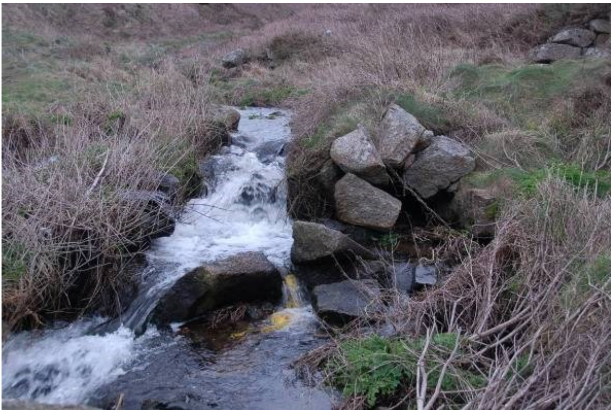
Fig 42. A collapsed section of the culvert which carried the Kenidjack Stream under the dressing floors, this part originally of arch headed form.
