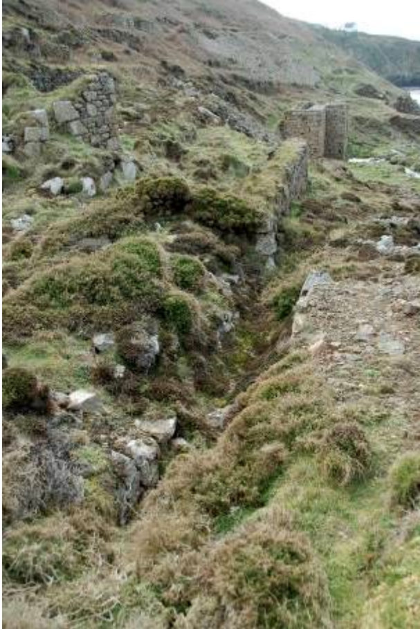
Fig 17. The flat rod trench running across the dressing floors from the Great Wheel. The collapsed end of the tunnel from the east is more or less at the point from which this photograph was taken.
