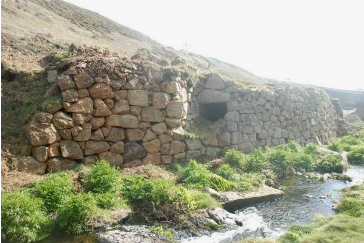
Fig 15. The dressing floor retaining wall from the north east, showing the entrance to the flatrod tunnel (centre).
