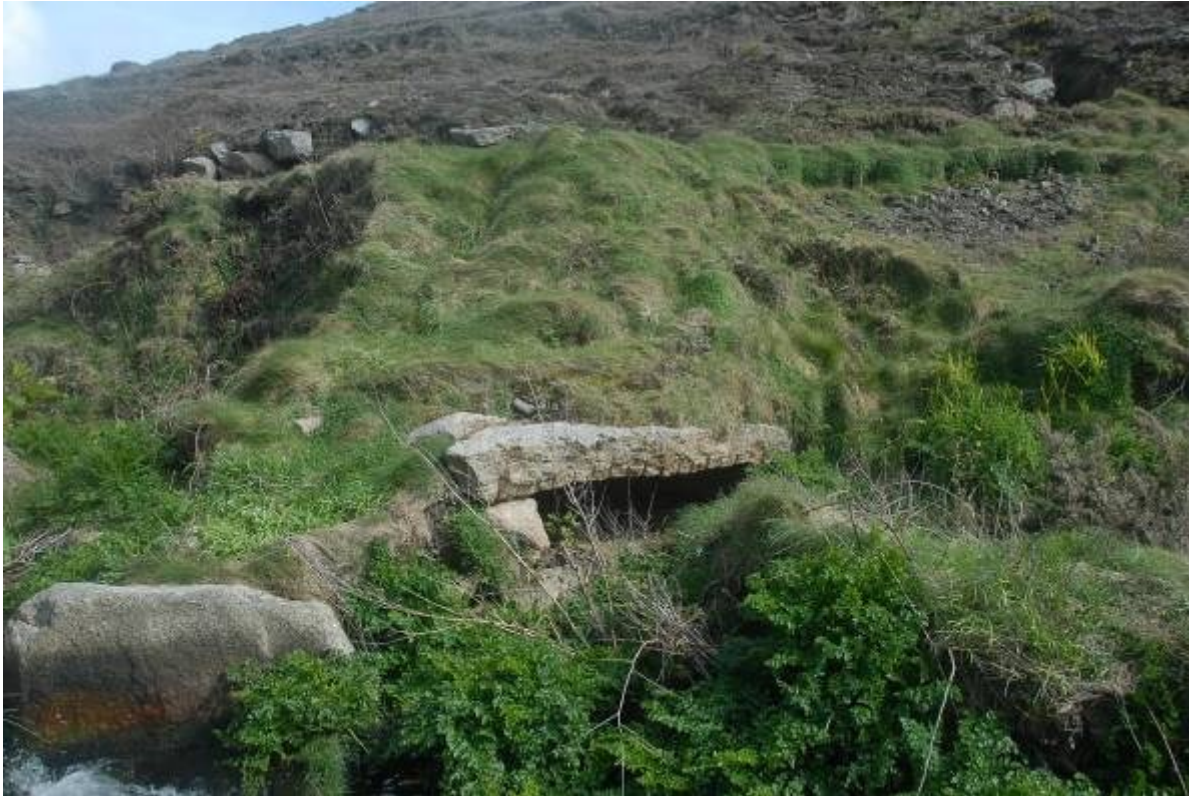
Fig 19. The entrance to the only surviving section of the culvert which originally carried the mine roadway across the valley from north to south.
