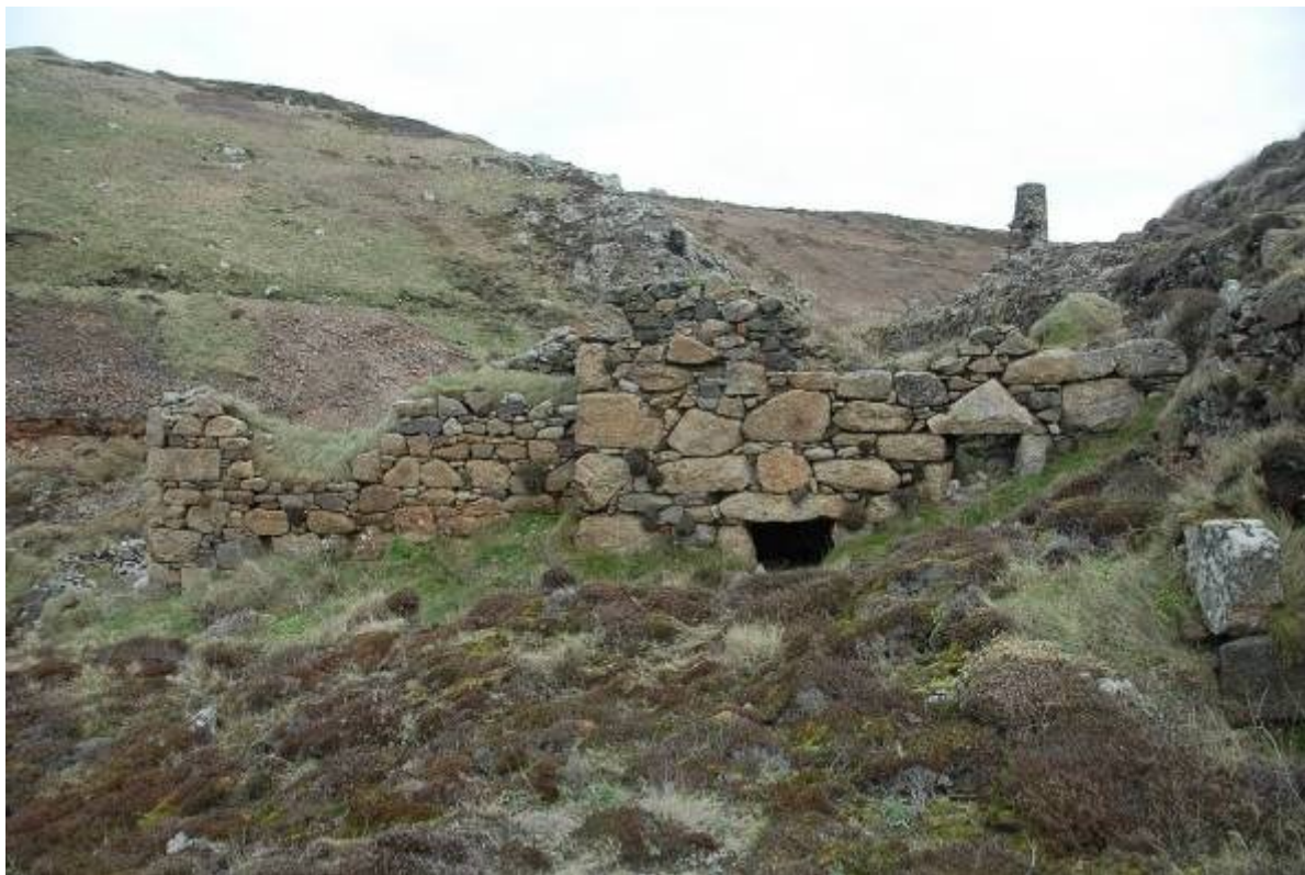
Fig 30. The reverberatory arsenic calciner from the west, showing the hearth opening (right) and discharge opening or wrinkle hole (left).
