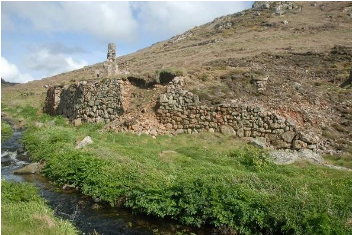
Fig 16. The dressing floor retaining wall from the north west, showing the area of collapse.
