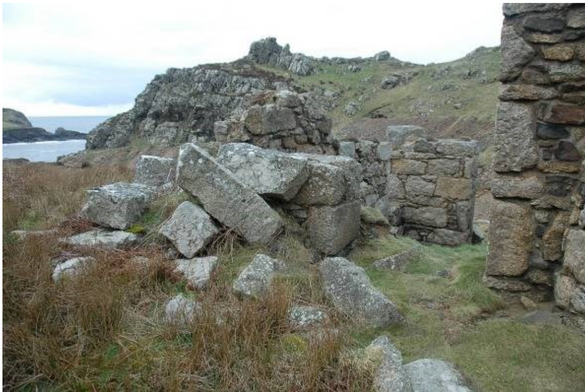
Fig 38. The remains of the substantially demolished rear wall of the stamps engine house, showing the remains of the original cylinder opening.
