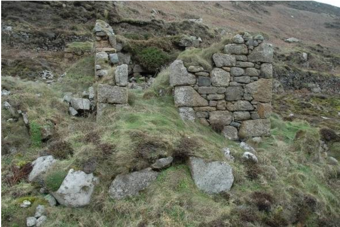
Fig 31. The northern elevation of the calciner, showing the offset doorway and the stamps mortarstone incorporated into the low wall in front (bottom left).
