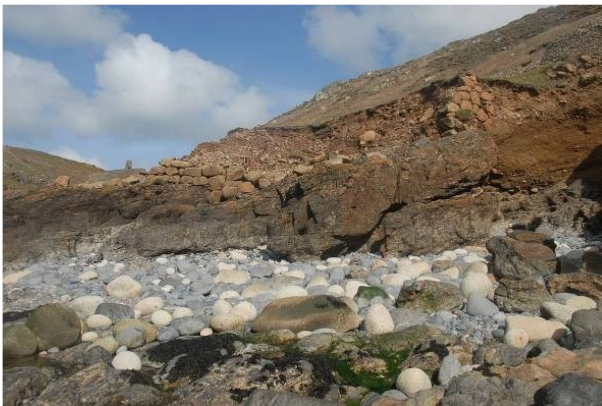
Fig 23. The remains of the boulder wall which formerly retained dressing floors above Porthledden, but is now very much eroded away.
