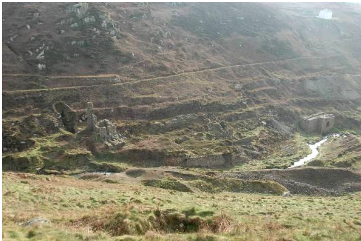
Fig 14. Looking down onto the Wheal Call dressing floors from the north, showing the stamps engine house to the left, the calciner at centre and the Great Wheel pit to the right.
