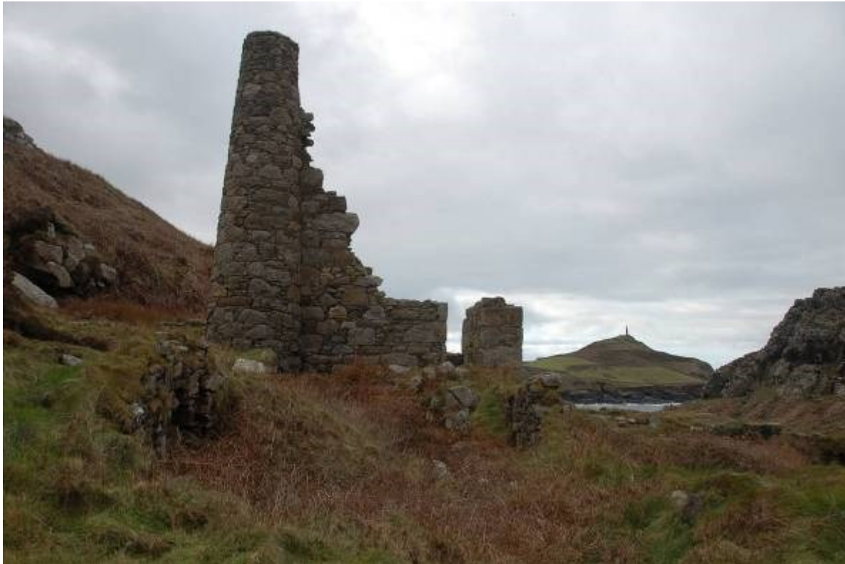
Fig 35. The stamps engine house from the east, with the remains of the boiler house walls in the foreground.
