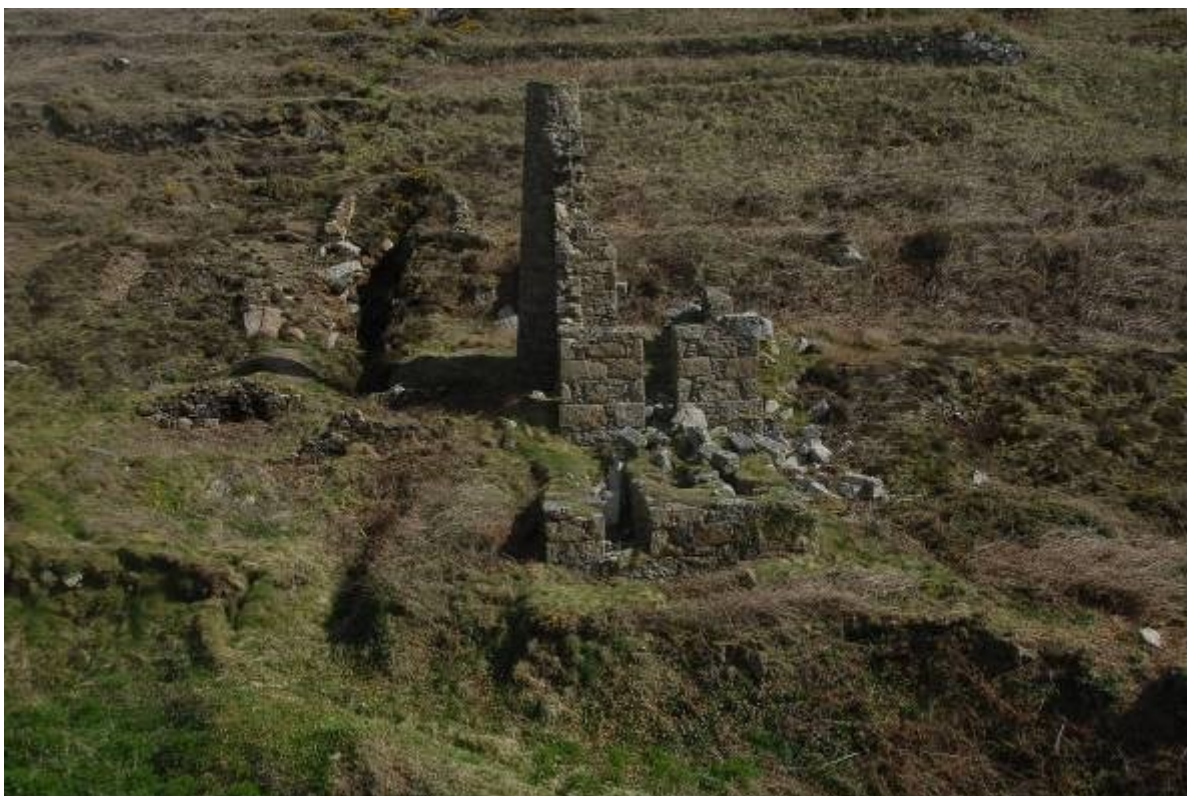
Fig 36. The stamps engine house from the north, showing the loadings to its north and workings on the outcrop of one of the Boswedden lodes to its left and running under its boiler house.
