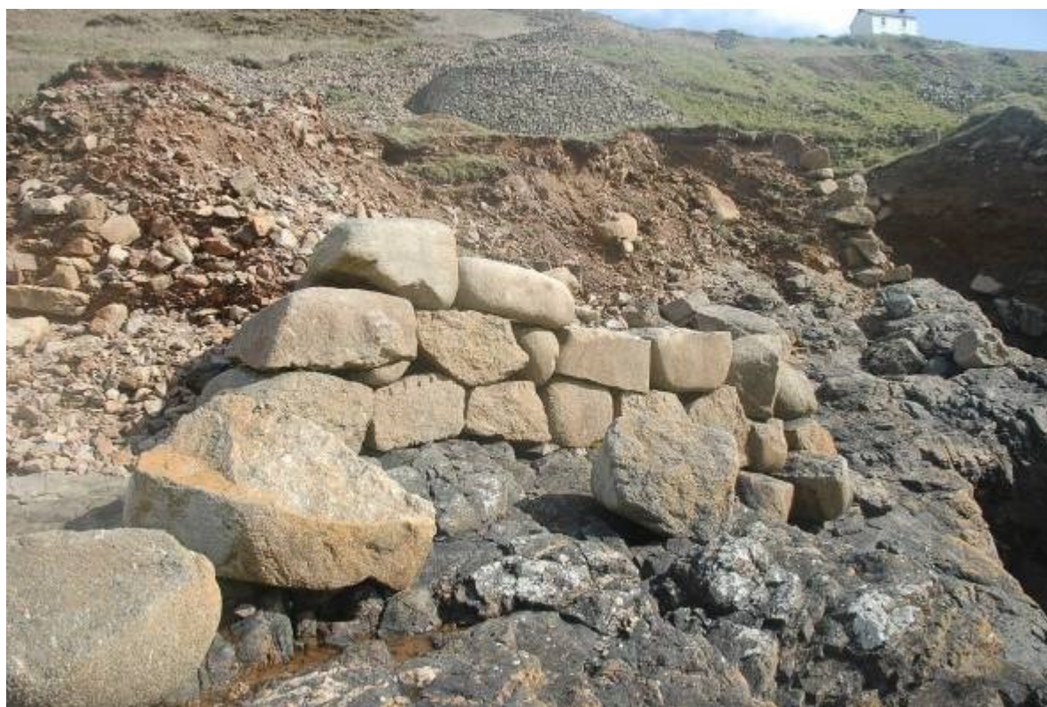
Fig 24. Another view of the remains of the boulder retaining wall, showing the substantial erosion which has taken place to the deposits which it formerly retained.
