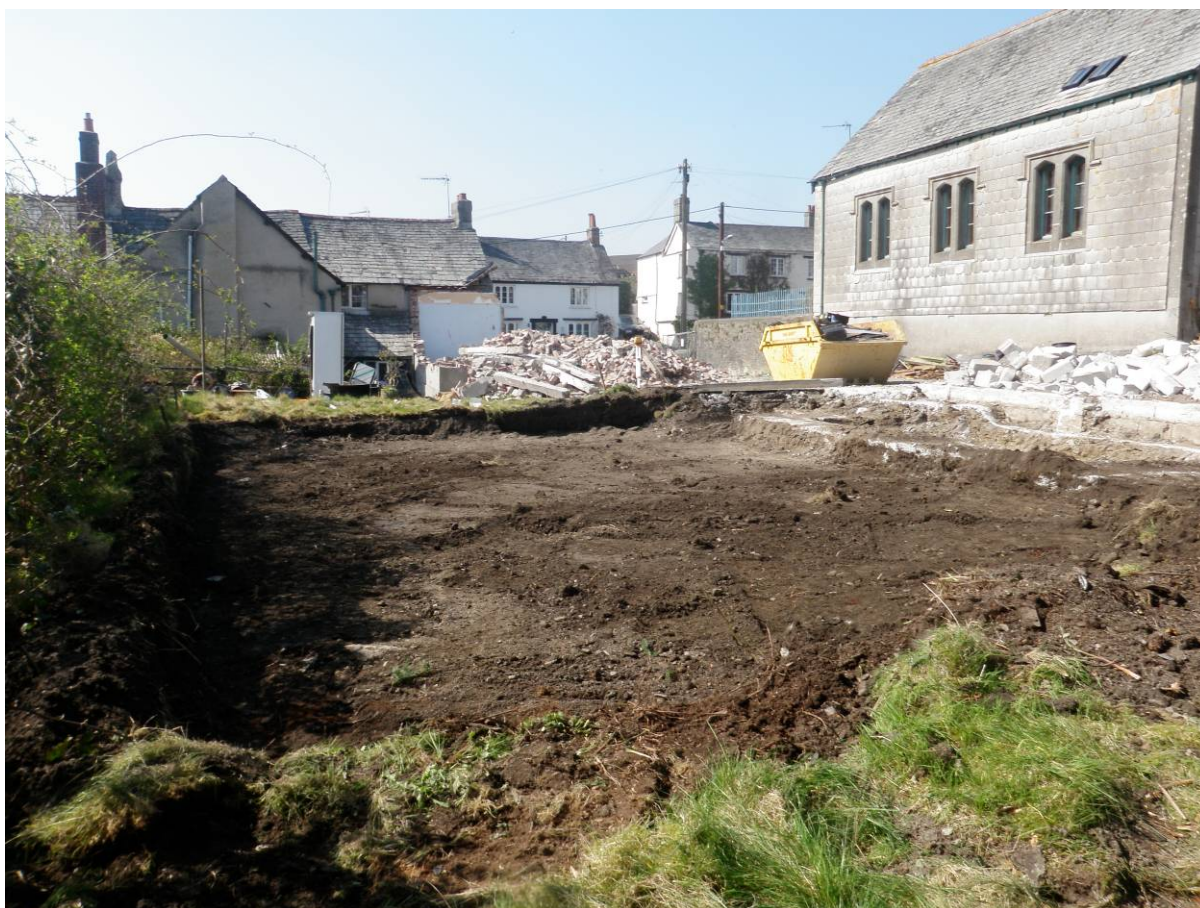
Fig 9 Excavation area looking west
