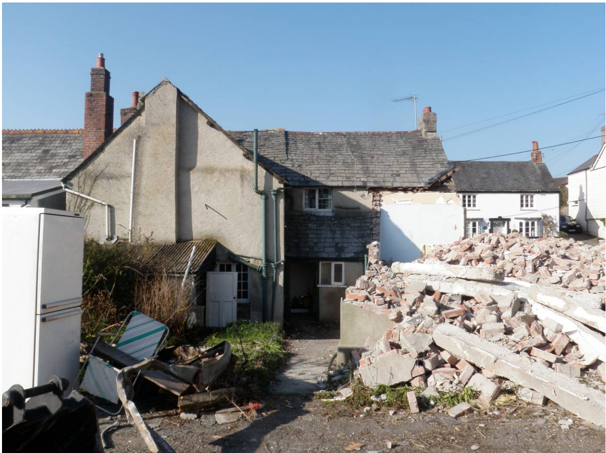
Fig 8 Rear of No 32 during demolition of No 32a
