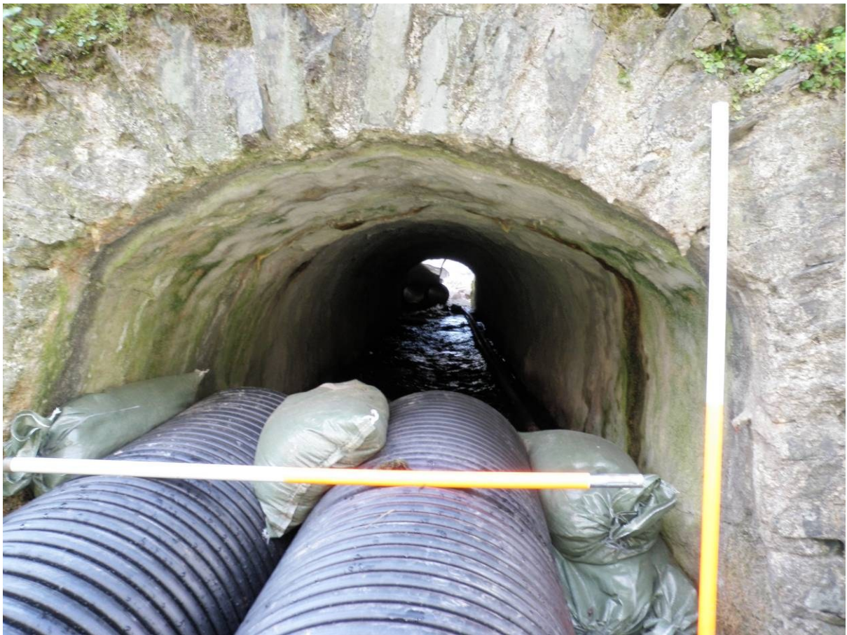
Fig 8 View inside the culvert from the north portal
