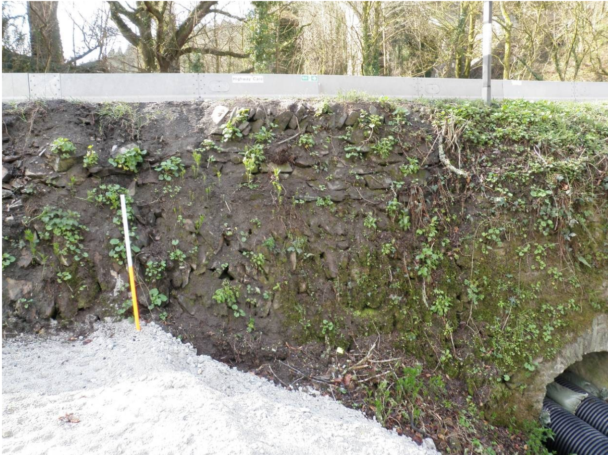
Fig 9 Revetment of the causeway east of the culvert
