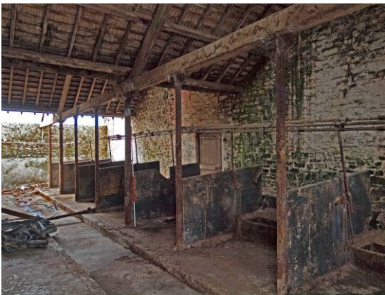
Fig 67 Building 5 (shippon) from south
