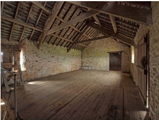
Fig 45 Building 1 room 7 (stable loft) from east
