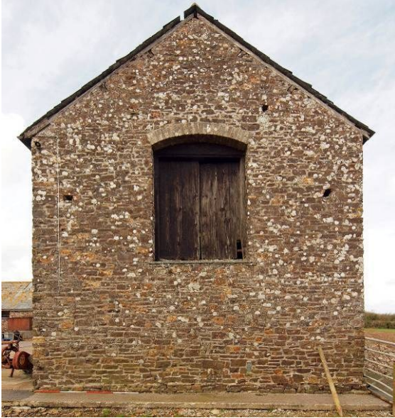
Fig 15 Building 1 from SE
