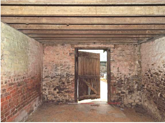
Fig 27 Building 1 room 2 from NE
