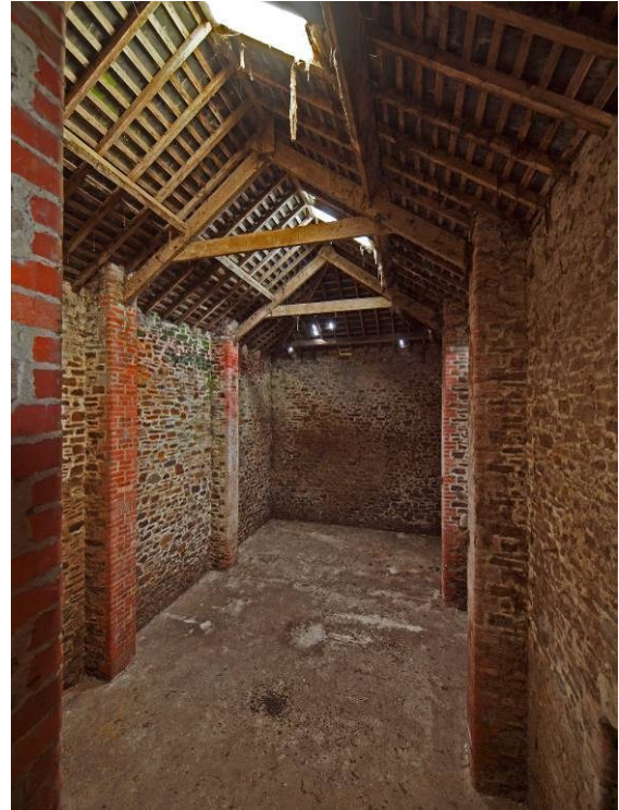
Fig 39 Building 2 room 5 (hay-barn)
