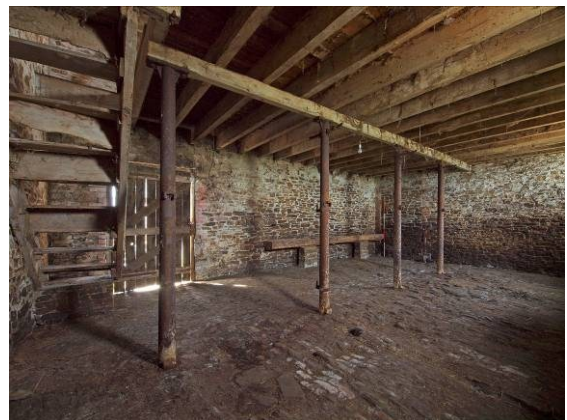
Fig 33 Building 1 room 4 (Stables) from east
