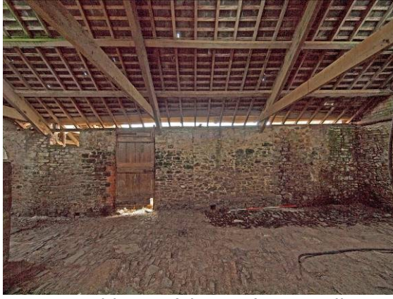
Fig 56 Building 3 (shippon) NW wall (right)
