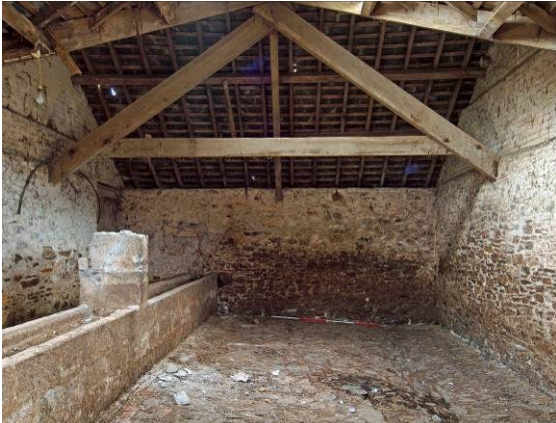
Fig 51 Building 3 (shippon), SW wall
