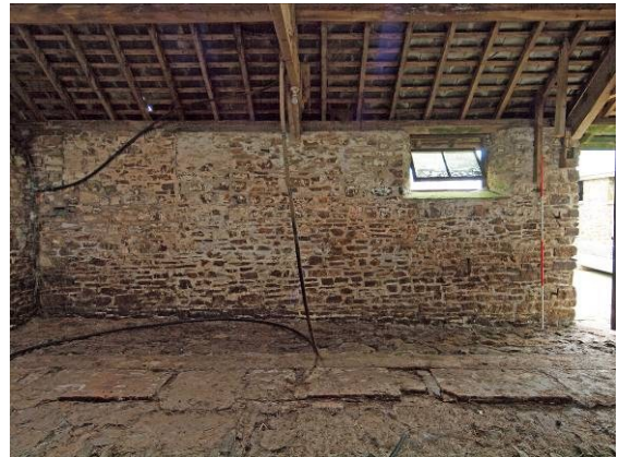
Fig 48 Building 3 (shippon), SE wall (left)
