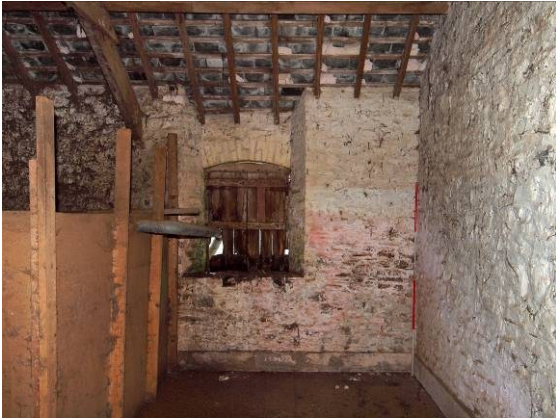
Fig 43 Building 1 room 6 NW end from NE
