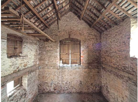
Fig 25 Building 1 (threshing barn) SE end
