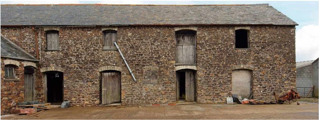
Fig 7 Building 1 from NW (threshing barn and stables)
