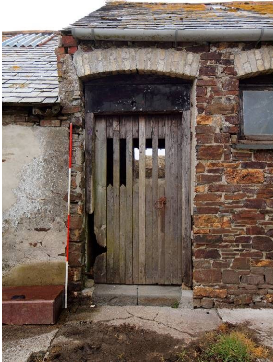
Fig 24 Building 5 (SE doorway)
