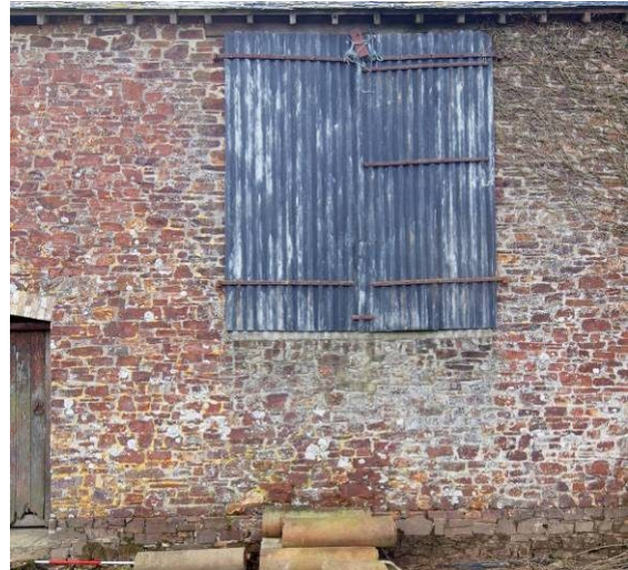
Fig 20 Building 2 Hay-barn NE loading doorway (reduced)
