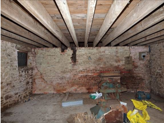
Fig 28 Building 1 room 2 from NW
