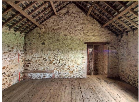
Fig 47 Building 1 room 7 Stable loft (inserted openings to later hay-barn (room 5))
