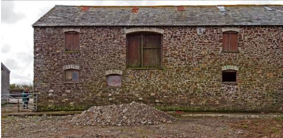
Fig 16 Building 1 (threshing-barn) from NE
