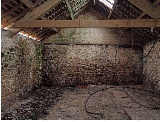
Fig 57 Building 3 (shippon), NE wall
