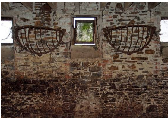
Fig 37 Building 1 room 4 Stable hay racks; window openings reduced
