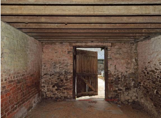
Fig 29 Building 1 room 3 from NE
