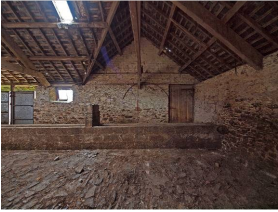
Fig 50 Building 3 (shippon), SE wall (right)
