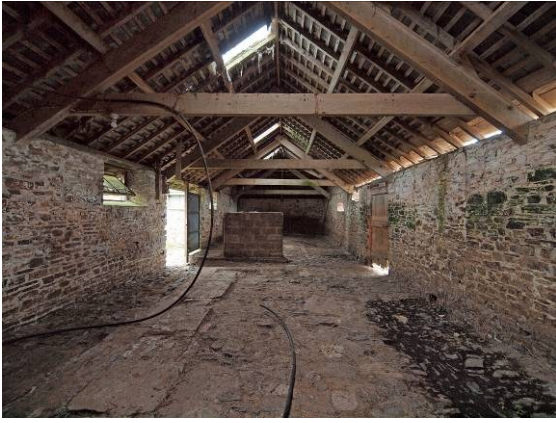
Fig 58 Building 3 (shippon) from NE
