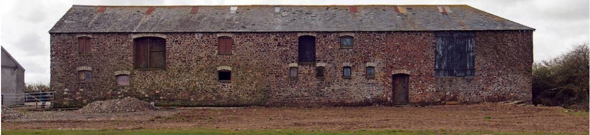
Fig 8 Buildings 1 and 2 from SE (threshing barn and stable barn, and later hay-barn)
