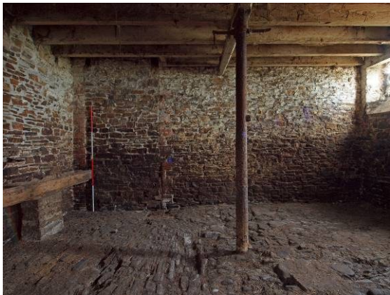
Fig 36 Building 1 room 4 (Stables) doorway cut through to later hay-barn and later blocked
