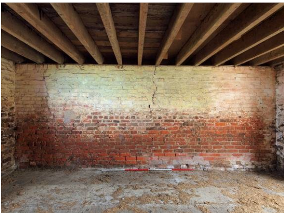
Fig 30 Building 1 room 3 from NW
