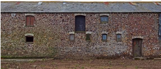
Fig 17 Building 1 (stables and loft) from NE
