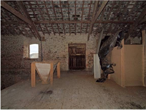
Fig 42 Building 1 room 6 Threshing floor from NE
