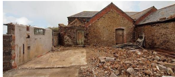
Fig 64 Building 4 site remains, also former bulk-tank room plus gables of Building 5 (shippon)
