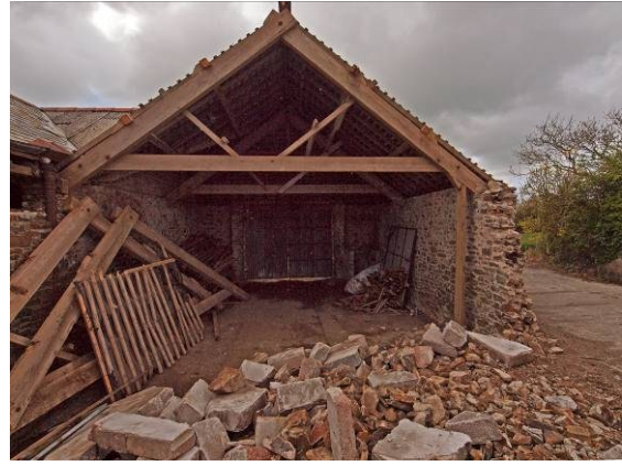
Fig 62 Building 4, cart-shed/implement store remains
