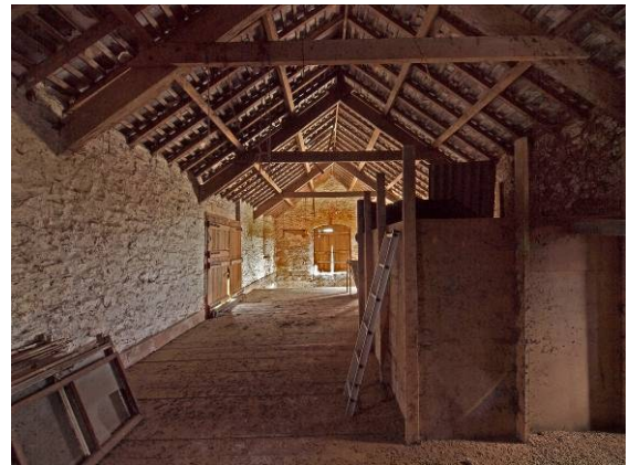
Fig 40 Building 1 room 6 (threshing floor) from NE
