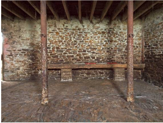
Fig 35 Building 1 room 4 (Stables) stall stanchion detail from NE
