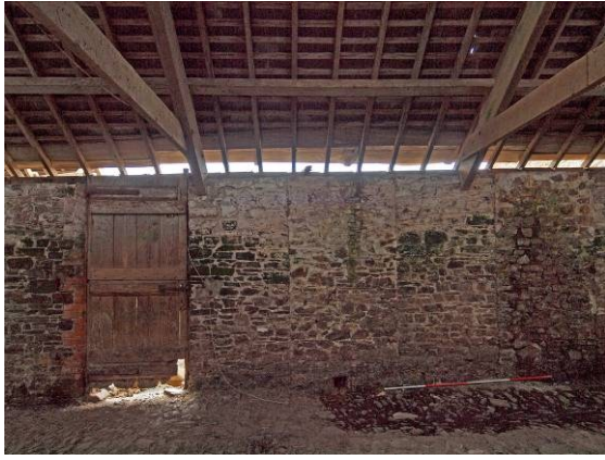
Fig 55 Building 3 (shippon), NW wall (centre)
