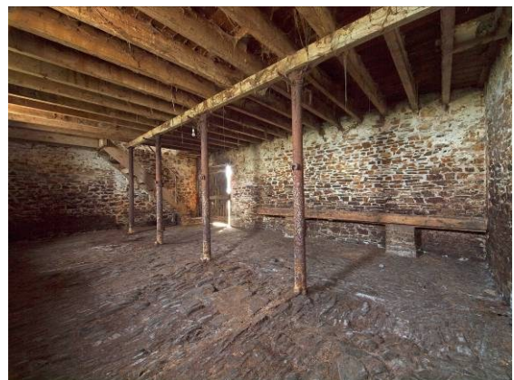
Fig 34 Building 1 room 4 (Stables) from north
