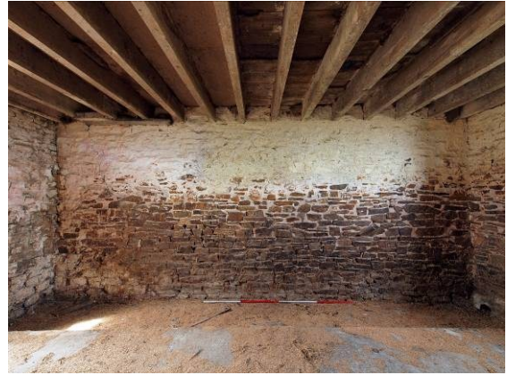
Fig 31 Building 1 room 2 from SE
