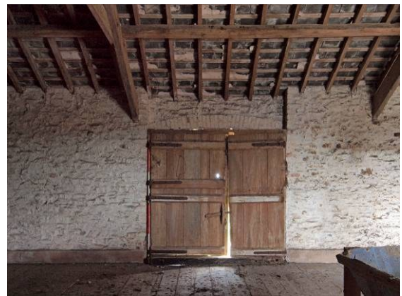
Fig 41 Building 1 room 6 Threshing floor NE doorway
