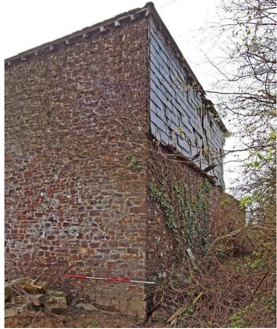
Fig 19 Building 2 (hay-barn) from NW
