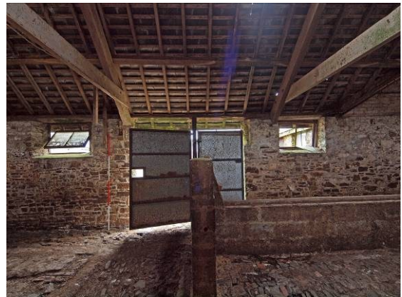
Fig 49 Building 3 (shippon), SE wall (centre)
