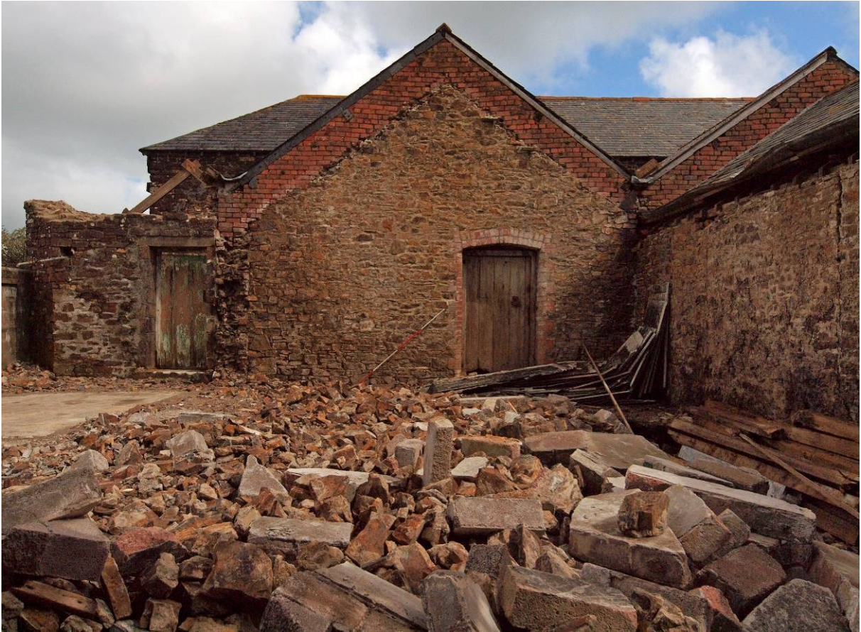
Fig 11 Building 5 (shippon); demolition remains of Building 4 in the foreground
